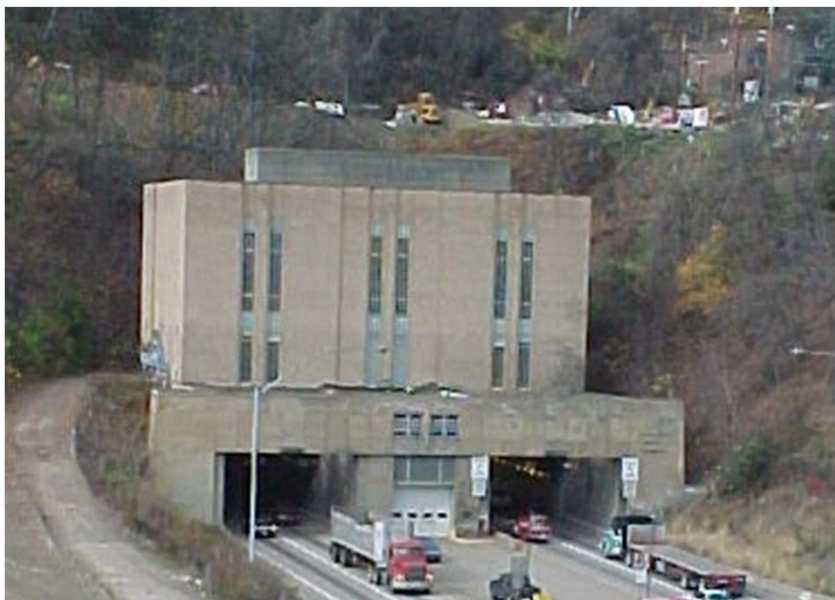
Squirrel Hill Tunnel on I-376 in Pittsburgh
