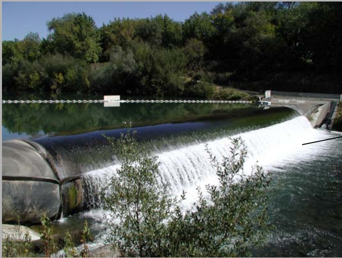
The inflatable dam is erected, May – Nov.
