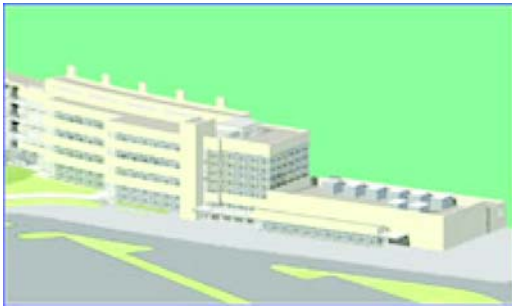
Center For Nanophase Materials Sciences at ORNL
