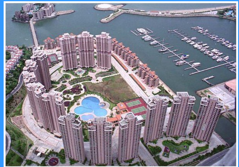
Marina and breakwater development
