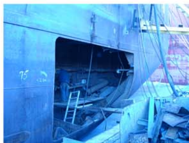
Workers weld shut the access hole cut into the M/V H. Lee White at Bay Shipbuilding in Sturgeon Bay, Wisconsin
