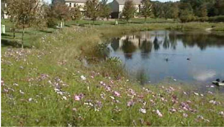
**Stormwater Basin:** A large excavated depression landscaped with native grasses or vegetation that temporarily detains stormwater and provide controlled stormwater flow. Infiltration can be design where feasible.
