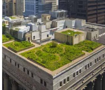
**Green Roof:** A vegetated surface installed over an existing roof surface. Vegetated roofs are effective in reducing the volume and velocity of stormwater runoff. A typical green roof consists of a waterproofing and root barrier layer, insulation, drainage and filter layer, growth media, and plants. Green Roofs can either be installed as a fixed structure or as a series of removable modules.
