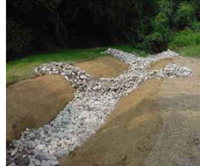
**Swale:** A vegetated basin designed to convey, attenuate and/or infiltrate stormwater runoff. In some cases, they are used to enhance water quality benefits. Porous media can be added to the swale base to enhance infiltration and water quality benefits.
