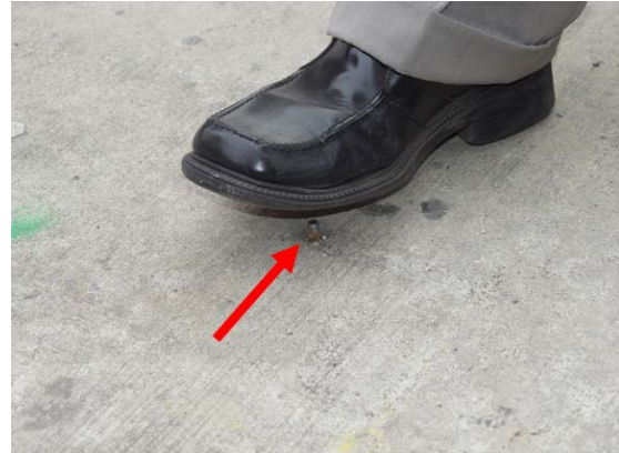
(4) Fastening screws left behind are a hazard to pedestrian traffic
