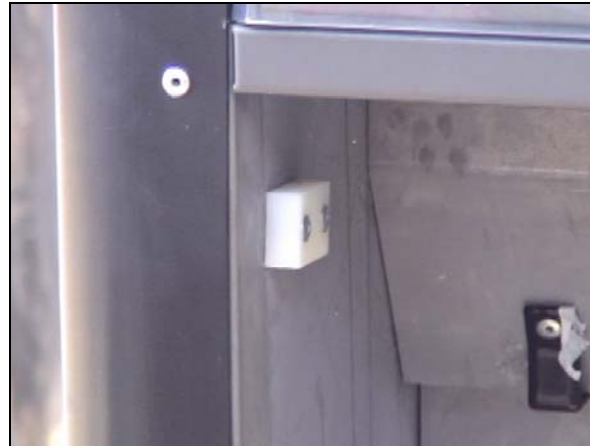
(35) New installed door stop
