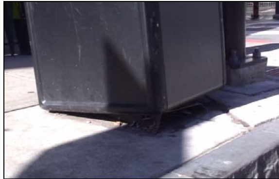
(26) A compactor unit that is not level
