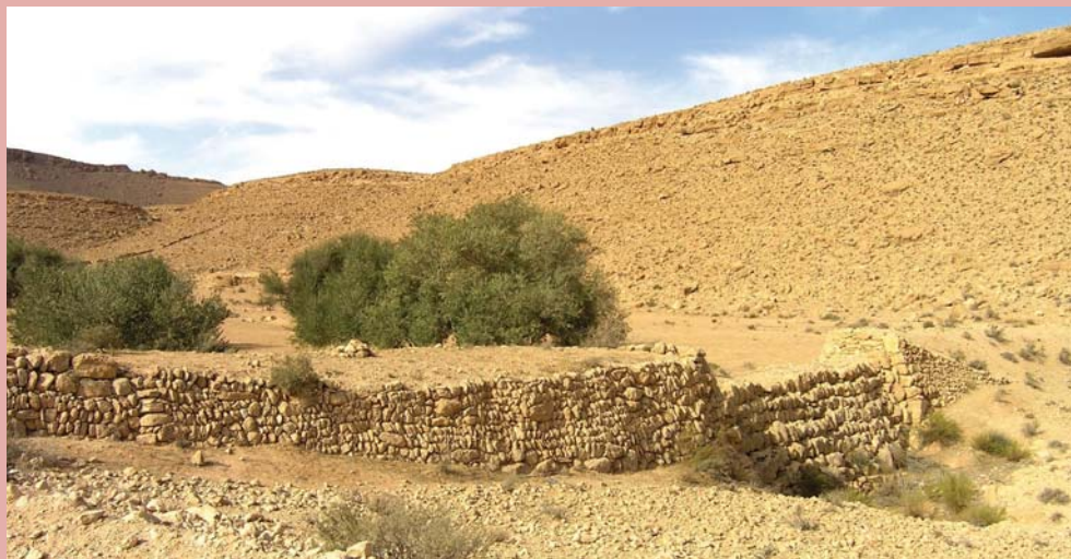
Traditional terracing to harvest water and control overland flow near Tataouine in Southern Tunisia.
