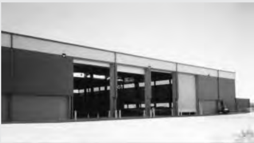
Transfer station structures require tall access doors to accommodate collection vehicles.
