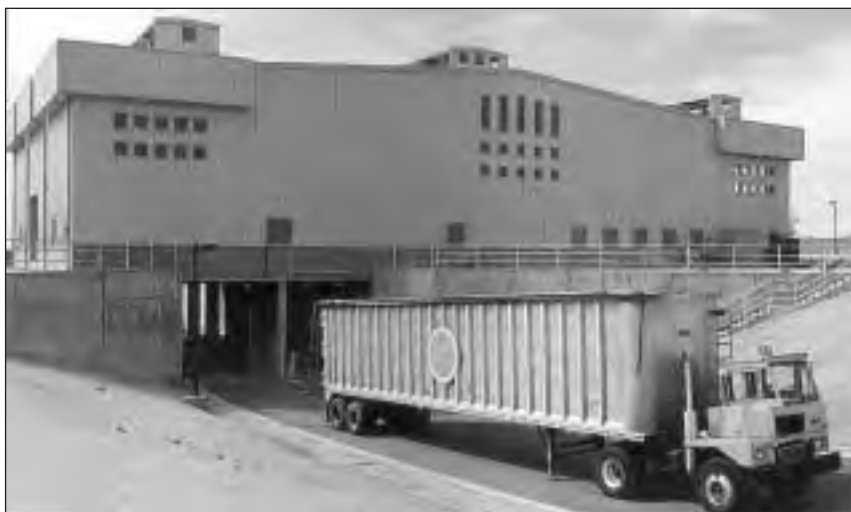
Many transfer stations are multi-level facilities that allow vehicle access at several levels.
