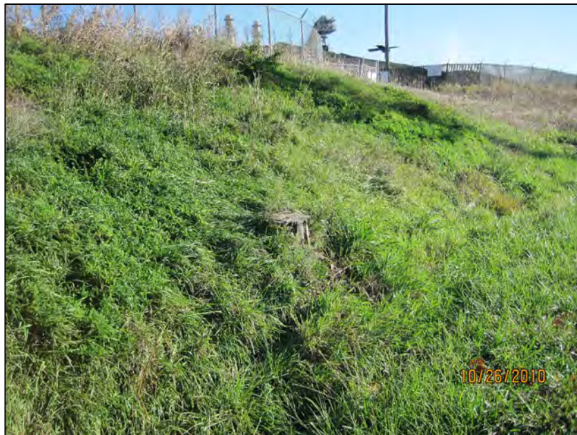
2-22 STUMP ON DOWNSTREAM EMBANKMENT FACE
