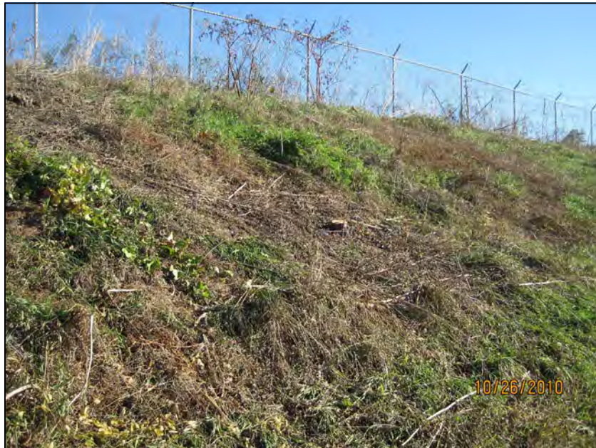
1-20 STUMP ON DOWNSTREAM EMBANKMENT FACE
