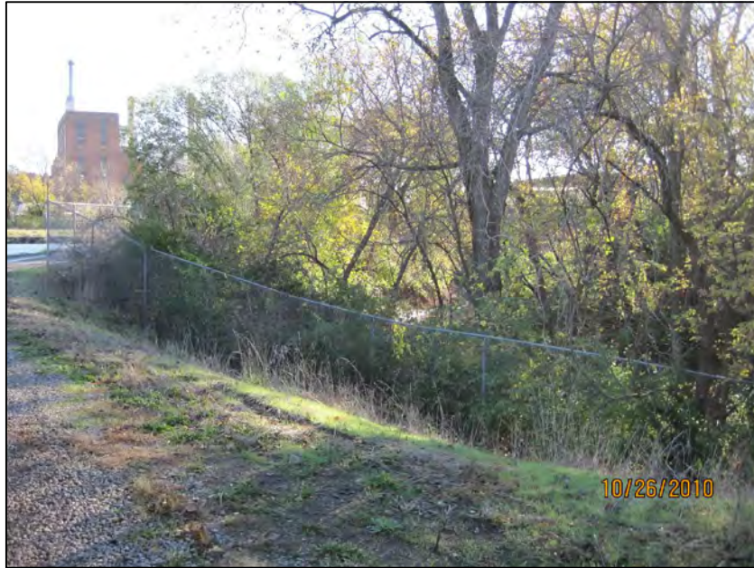
2-15 LOOKING EAST AT TREES/VEGETATION ON SOUTHERN DOWNSTREAM EMBANKMENT
