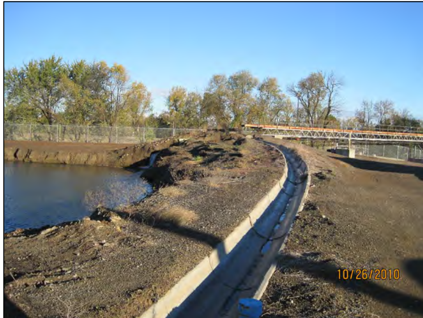
1-5 CENTRAL EAST SIDE LOOKING NORTH (UPSTREAM) AT SLUED ASH INFLUENT CHANNEL
