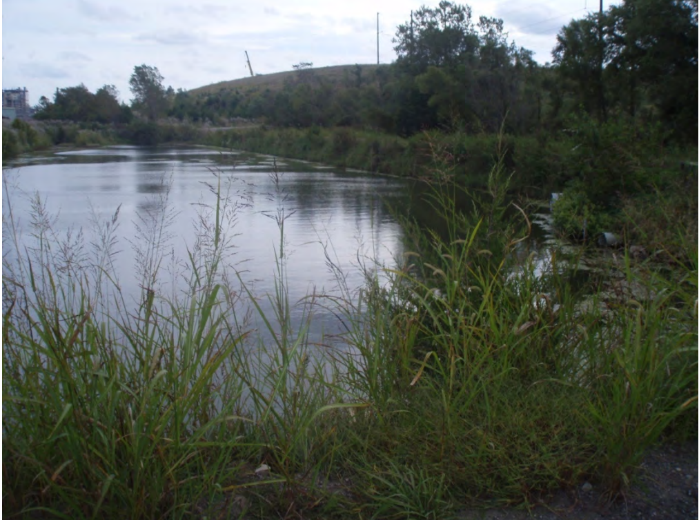
23. STORM WATERPOND AT SOUTH END OF ASH POND AREA/AREA 3 – TAKEN FROM WESTERN PORTION OF PERIMETER DITCH LOOKING EAST.
