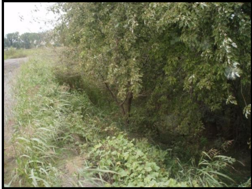
Figure 5.3.3-1: Typical Condition of Outside Slope of Western Portion of Perimeter Dike.
