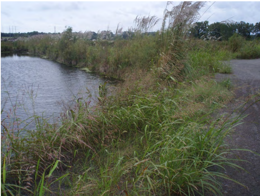
14. INTERIOR OF NORTHWESTERN PORTION OF PERIMETER DIKE (AREA 4)
