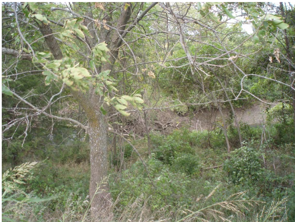
17. BALDWIN CREEK FLOWING NEAR TOE OF NORTHWESTERN PORTION OF PERIMETER DIKE (AREA 4)
