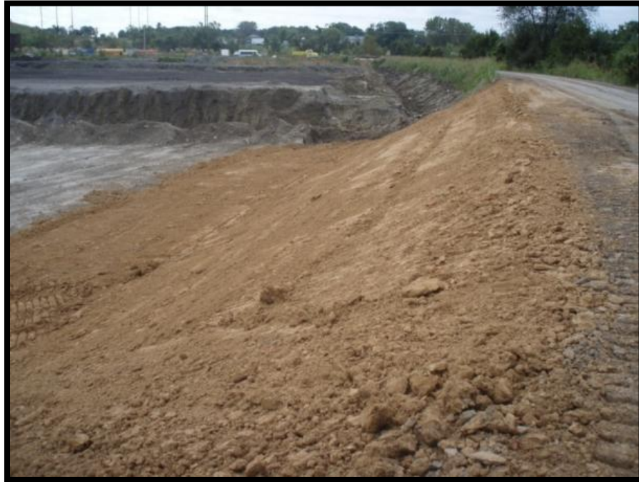
Figure 5.3.2-2: Inside Slope of Western Portion of Perimeter Dike (Area 3).
