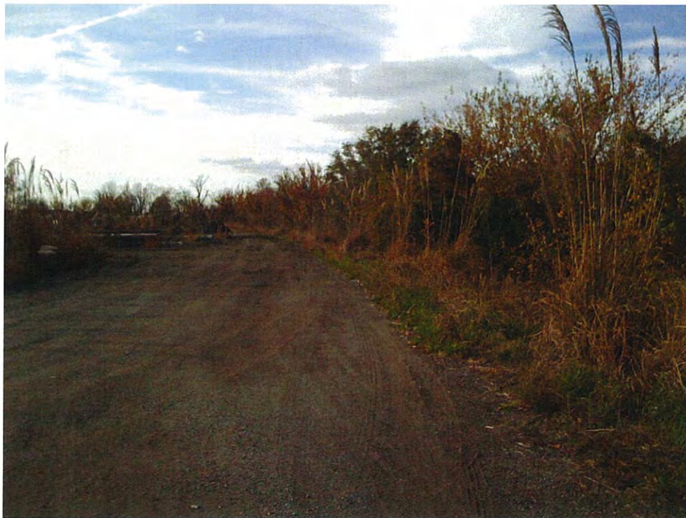
Photograph 4 – Berm crest near Borehole LEC-1 (looking northwest)
