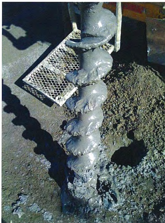
Photograph 6 – Soft saturated clay found in Borehole LEC-7 (looking northeast)
