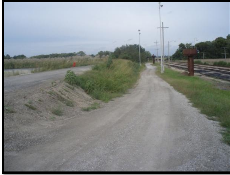
Figure 5.2.3-1: Outside Slope of Northeastern Portion of Perimeter Dike (Area 1).
