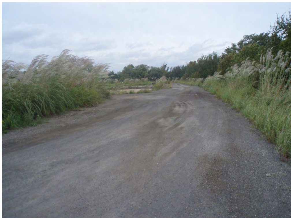
9. TOP OFNORTHEASTERNPORTIONOFPERMETERDIKE – TAKENFROM MIDPOINT BETWEEN AREA 1 AND 4 LOOKINGWEST
