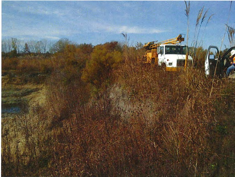
Photograph 5 – Drilling Borehole LEC-5 (looking west)
