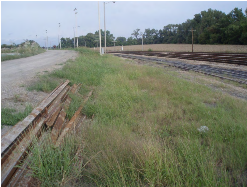
1. EXTERIOR OF NORTHEASTERN PORTION OF PERMETER DIKE – TAKEN FROM EAST END OF AREA 1, LOOKING WEST
