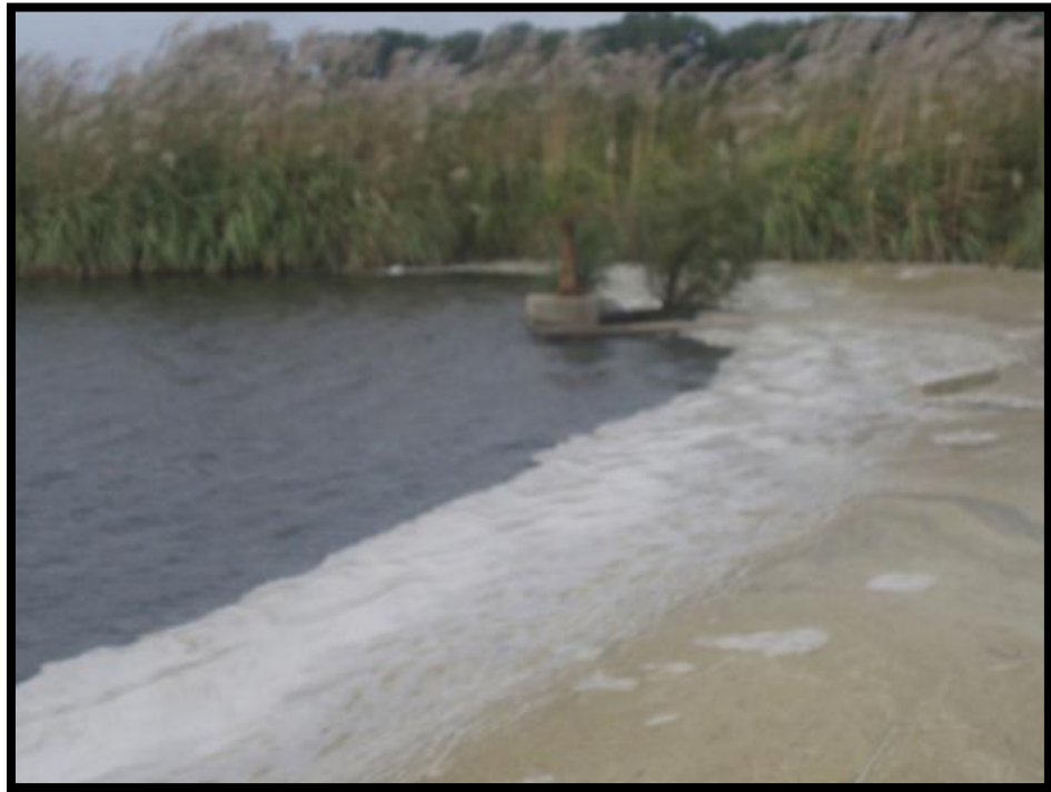
Figure 5.5.1-1: Overflow Outlet Structure (Area 1).
