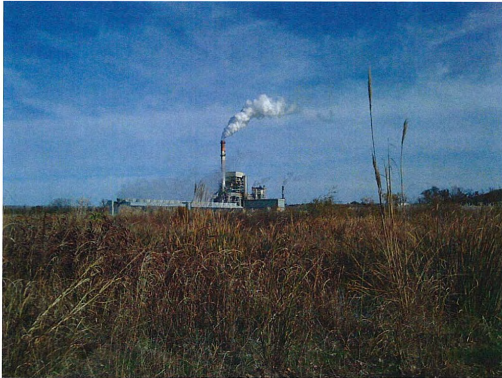
Photograph 3 – CCP storage facility (looking east)
