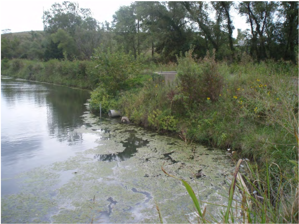
24. STORM WATERPOND DISCHARGE PIPE ON INTERIOR OF SOUTH SIDE OF AREA 3.
