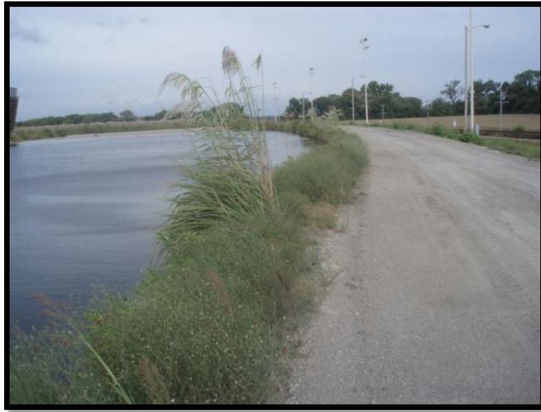
Figure 5.2.2-1: Inside Slope of the Northeastern Portion of the Perimeter Dike.
