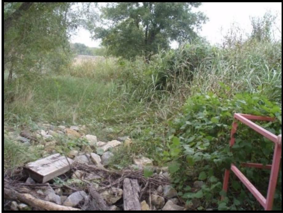
Figure 5.4.3-1: Outside of the Stormwater Pond Embankment on South Side.
