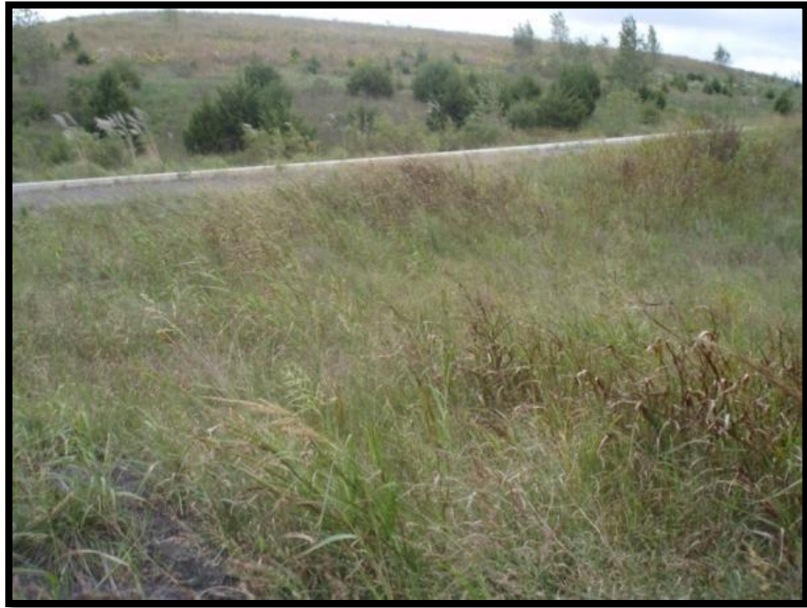
Figure 5.4.4-1: Tie-in of southern portion of perimeter dike to road embankment.
