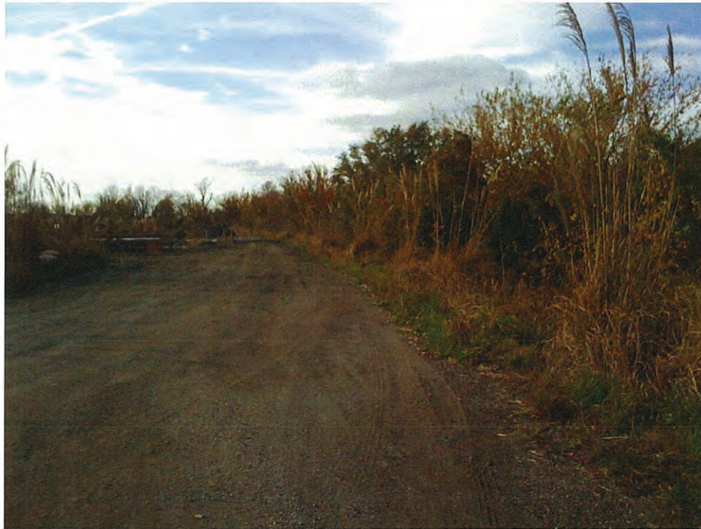
Photograph 5 – Berm crest (looking northwest)
