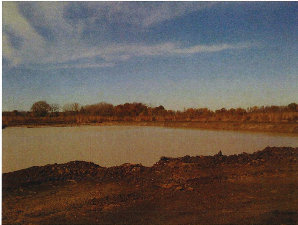
Photograph 1 – CCP storage facility (looking northwest)
