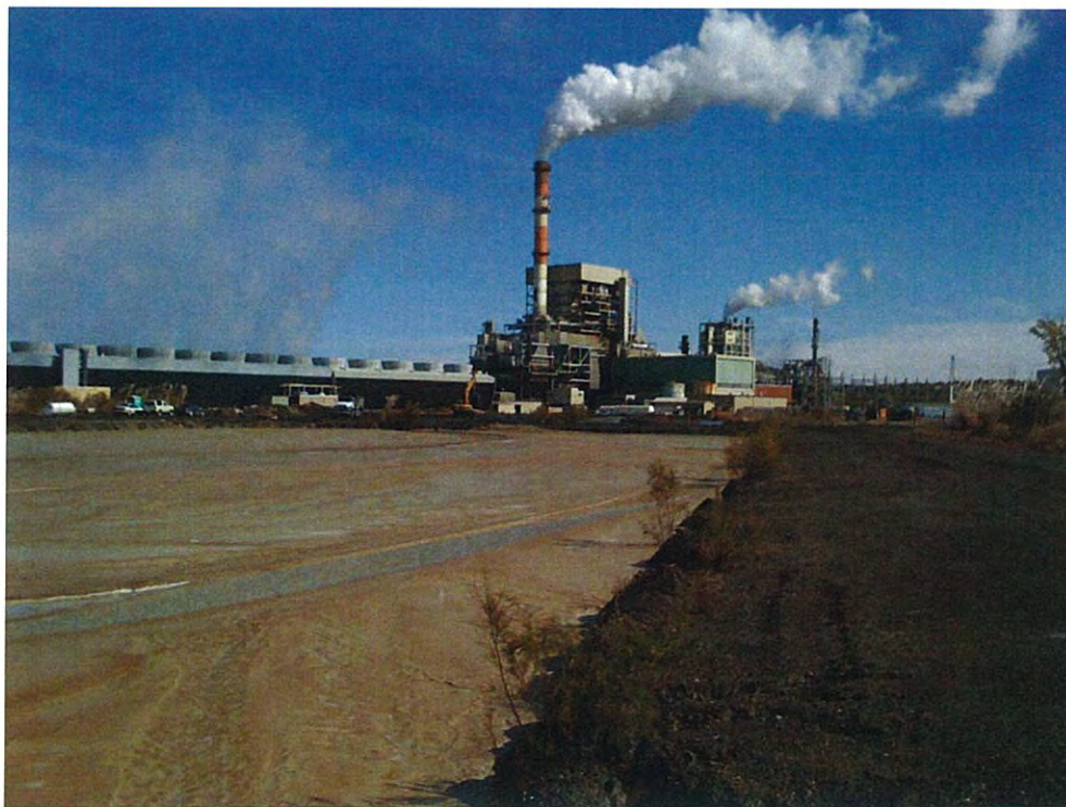
Photograph 2 – CCP storage facility (looking east)
