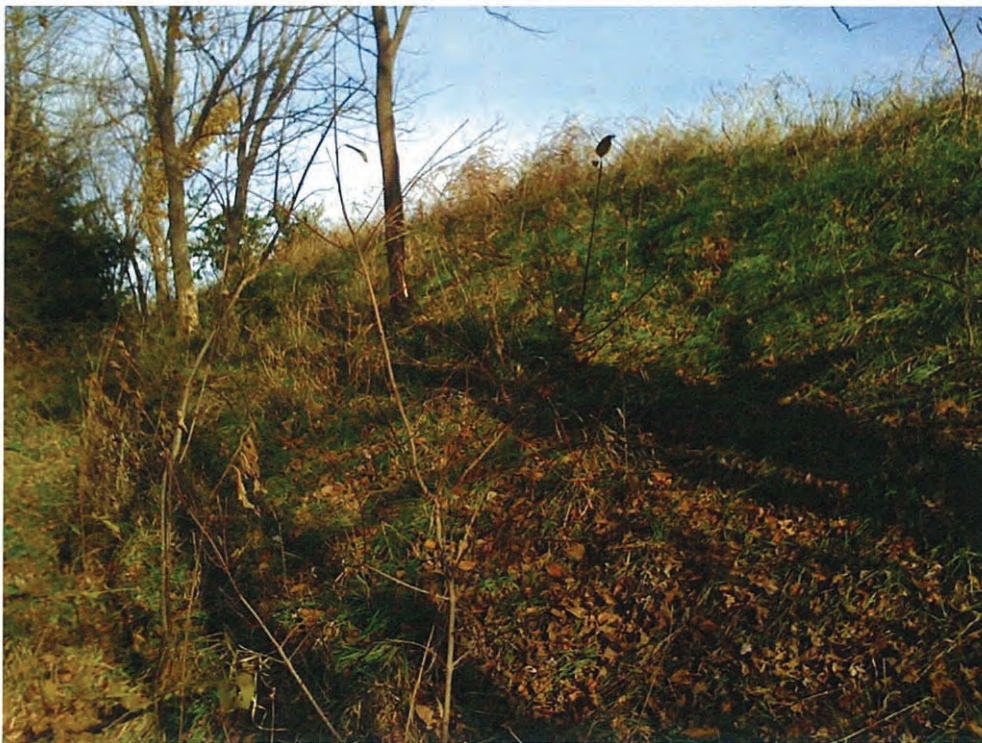
Photograph 6 – Downstream berm slope northwest of CCP storage facilities (looking east)
