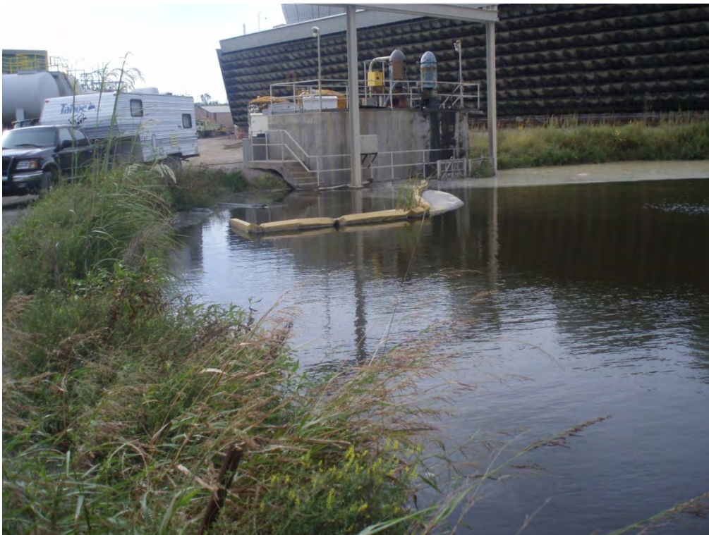
2. DISCHARGE PIPE AT EAST END OF AREA 1
