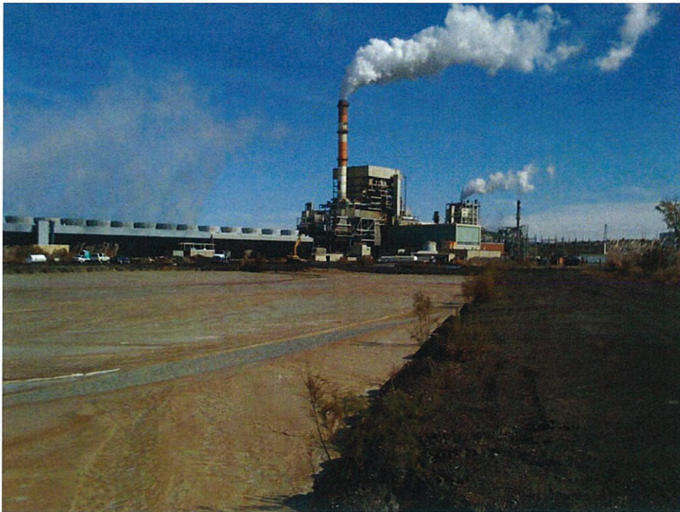
Photograph 2 – CCP storage facility (looking east)
