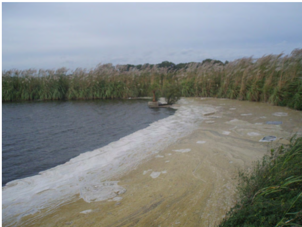
5. EMERGENCY OVERFLOW STRUCTURE – WEST END OF AREA 1
