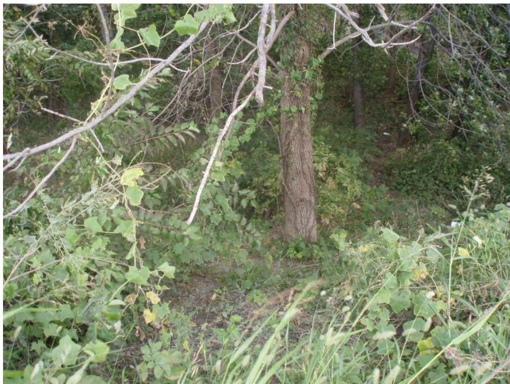
15. EXTERIOR OF NORTHWESTERN PORTION OF PERMETER DIKE (AREA 4) - 10" TREE OBSERVED AT TOE OF EMBANKMENT
