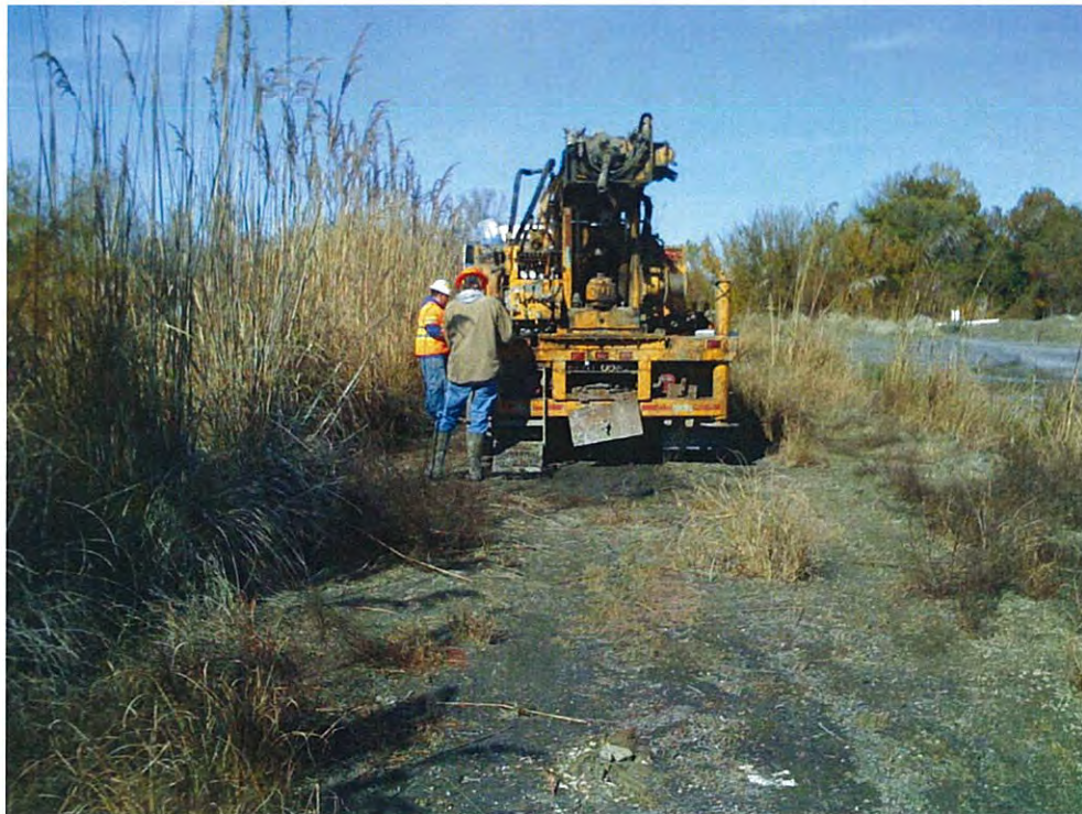
Photograph 8 – Drilling Borehole LEC-8 (looking north)
