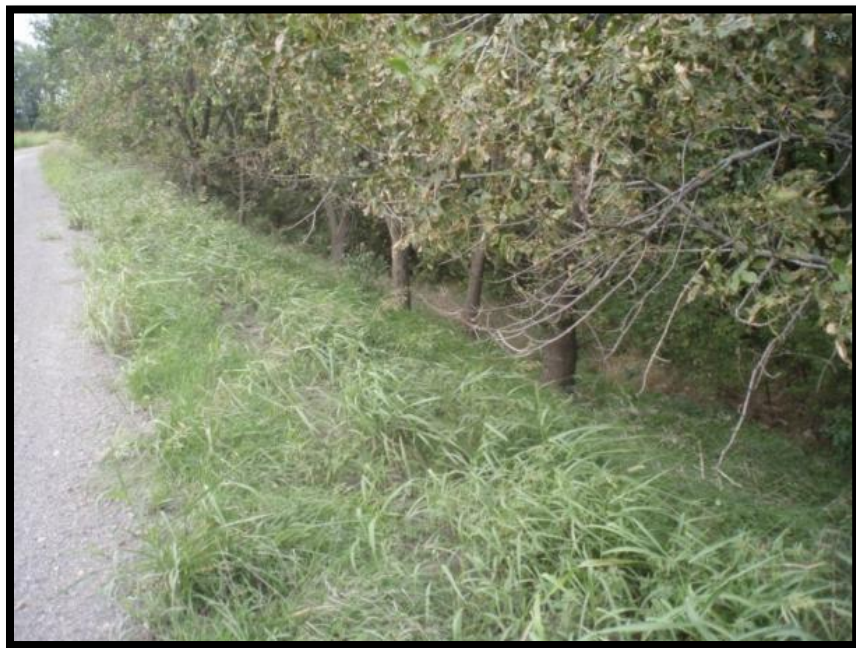
Figure 5.3.3-2: Trees on Outside of Western Portion of Perimeter Dike.
