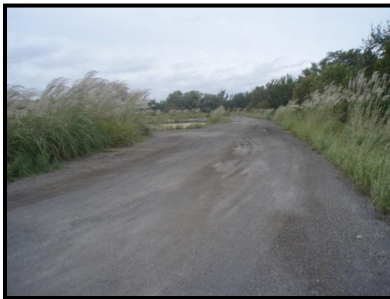
Figure 5.2.1-1: Crest of Northeastern Portion of the Perimeter Dike.
