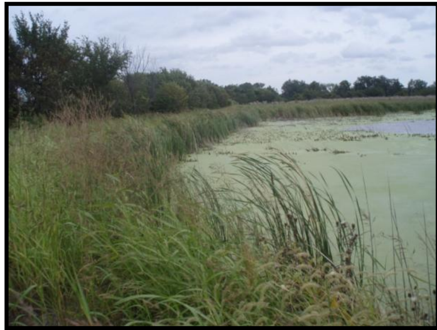
Figure 5.3.2-1: Inside Slope of Northwest Portion of Perimeter Dike (Area 4).
