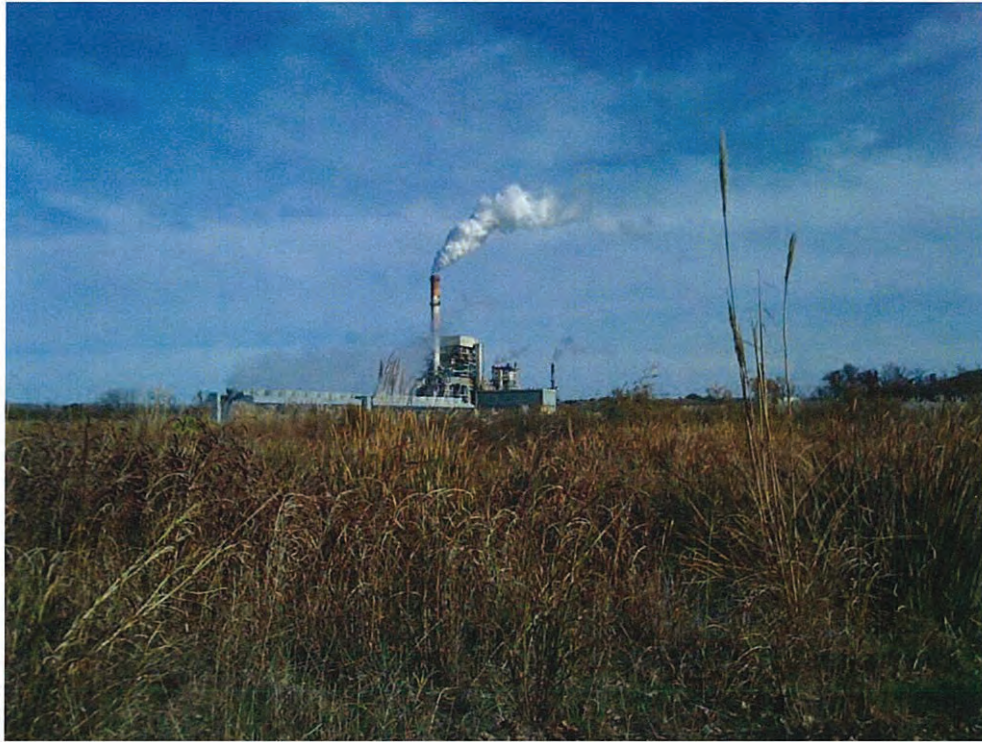
Photograph 3 – CCP storage facility (looking east)
