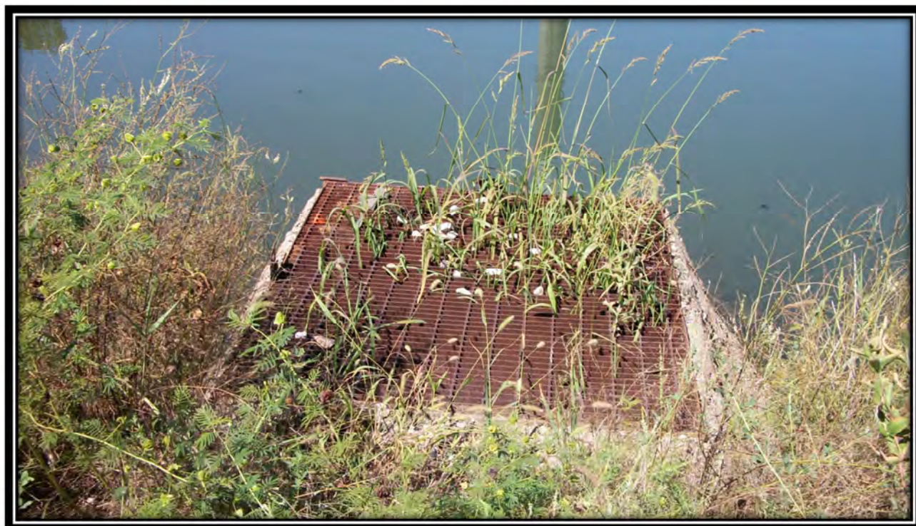
Photo 24 – Old overflow capped and plugged with concrete on east upstream bank
