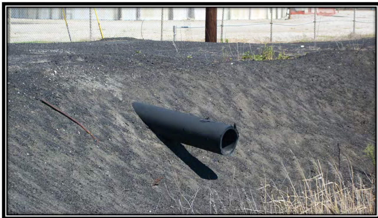
Photo 12 – Old ash line from neighboring site through west bank
