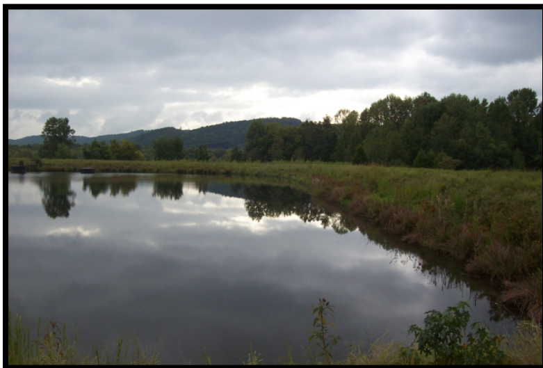
Figure 5.2.2-1: Inside slope of southern portion of embankment.
