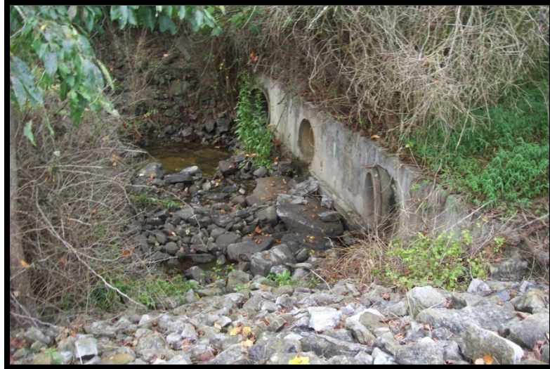
Figure 5.3.2-1: 3 - 36 inch outlet pipes discharging towards the Tennessee River.
