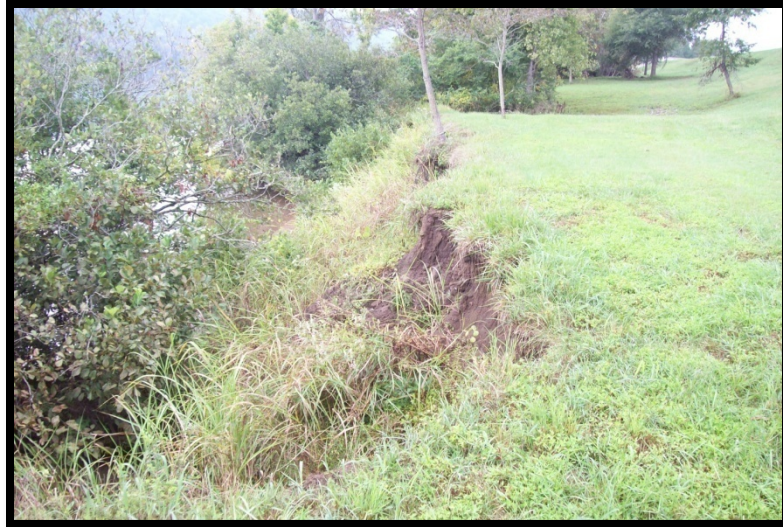
Figure 5.2.3-2: Outside toe of northeast portion of embankment. Note erosion.
