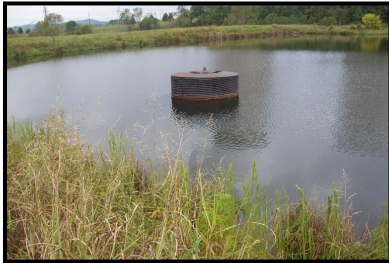
Figure 5.3.1-2: Riser structure.
