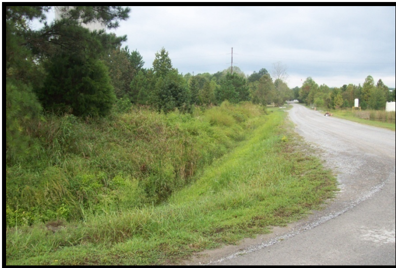
Figure 5.2.1-2: Crest of northern portion of embankment. The ash pond is to the left and the Watts Bar Fossil Plant is to the right.
