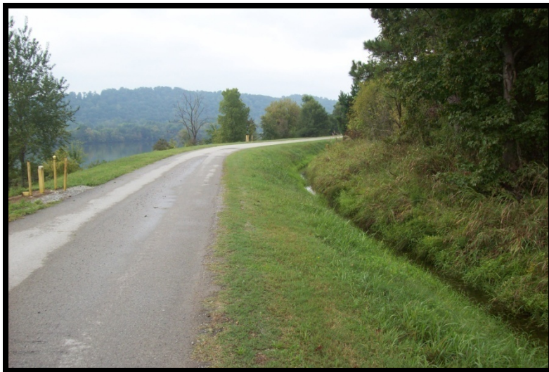
Figure 5.2.2-2: Inside slope of northeast portion of embankment.
