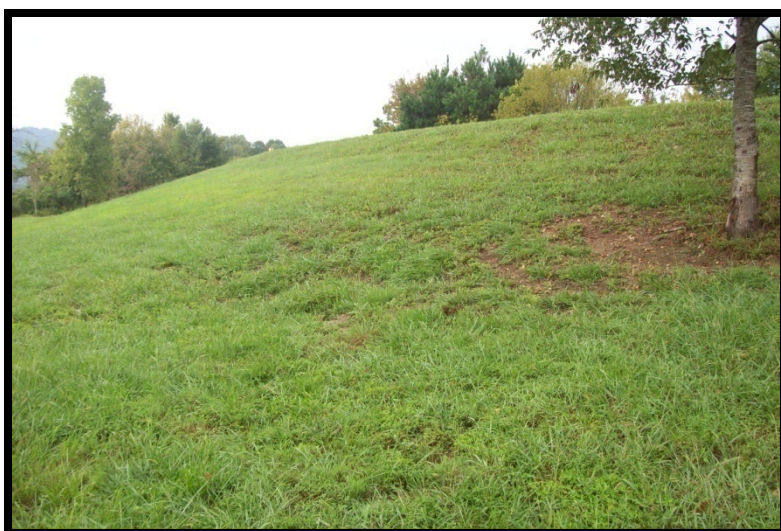
Figure 5.2.3-1: Outside slope of northeast portion of embankment. Note tree on embankment slope.
