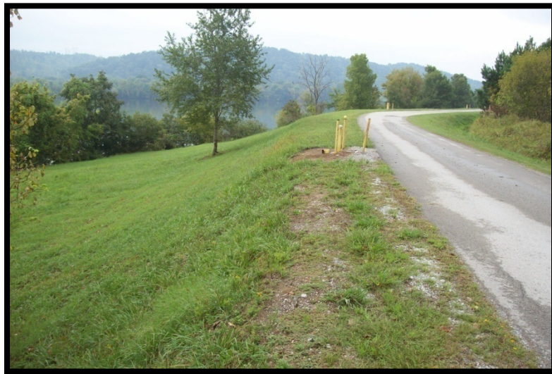
Figure 5.2.1-1: Crest of northeastern portion of embankment. The ash pond is to the right and the Tennessee River is to the left.
