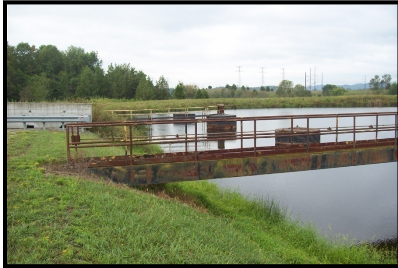
Figure 5.3.1-1: Riser structures. Picture taken from eastern portion of embankment.
