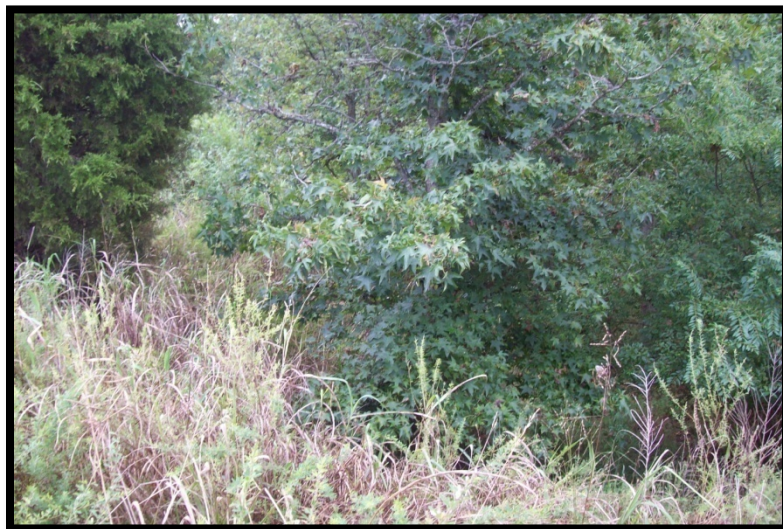
Figure 5.2.3-3: Outside slope of southern portion of embankment. Note tree growth and excess vegetation.
