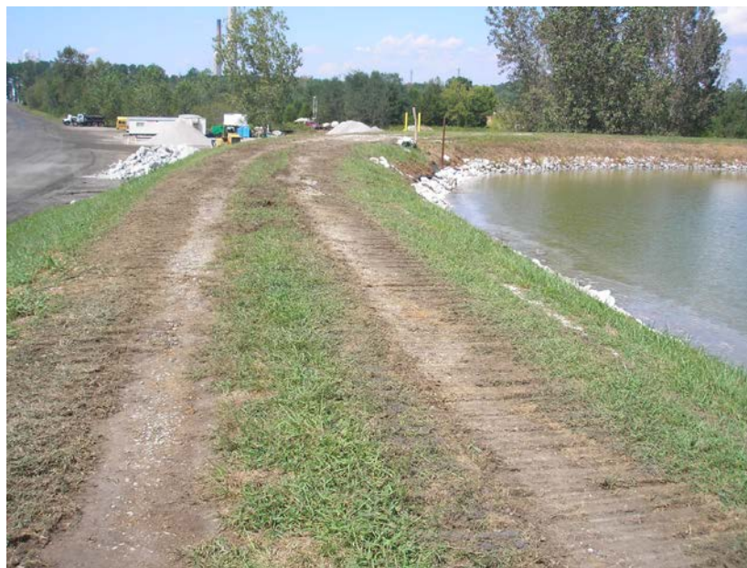
Photograph 5.3.4-1: Disposal Area 5 Drainage Basin Inside Groin at Southwest Corner
