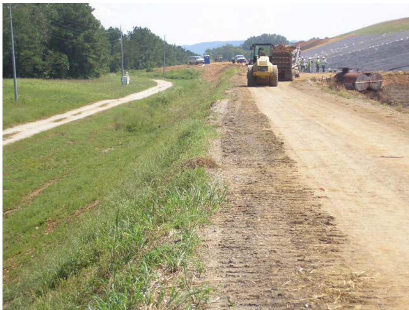
Photograph 5.3.3-1: Ash Pond 5 North Embankment Outside Slope with Fugitive Soil Adjacent to Construction along Ash Stack
