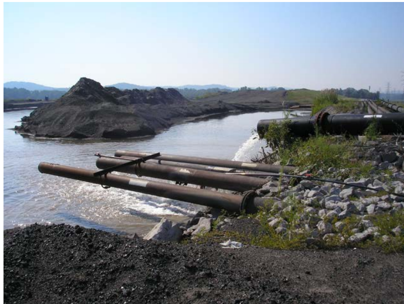
Figure 4.2.2-1: Sluiced Ash Discharge to Ash Pond 4. South Flowing Ditches through Stacked Ash in Background
