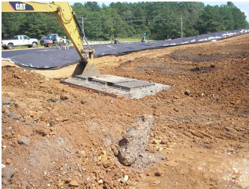
Photograph 5.4.1-2: Ash Stack Drainage System Outlet to Disposal Area 5 Drainage Basin
