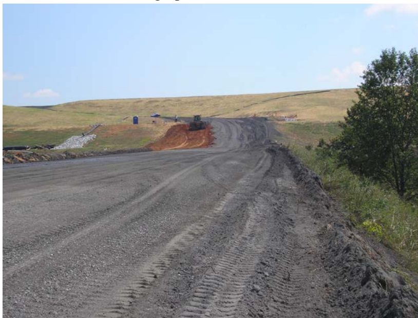
Photograph 5.3.2-2: Crest of Drainage Basin South Embankment with Compacted Ash Road Surface
