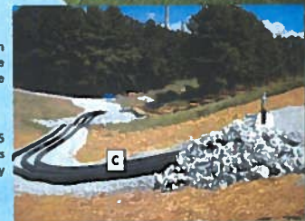
Siphons installed to lower normal pool in Ash Pond 4 stilling basin during spillway reconstruction.
