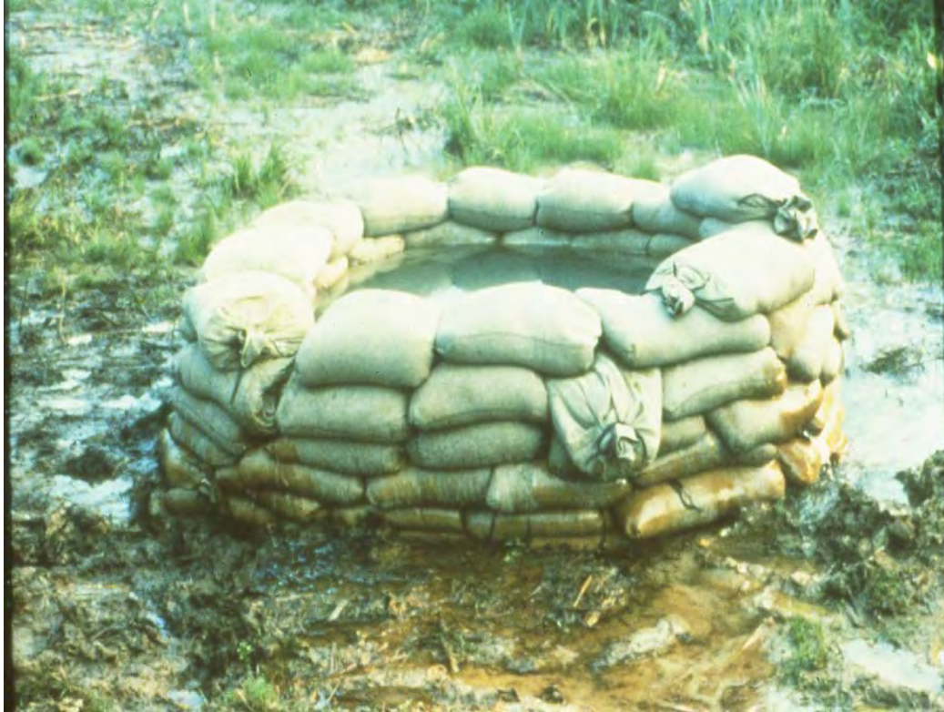
Figure 7. Sand Bag Treatment (Temporary)
