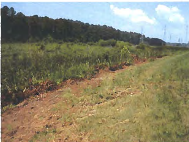
Photo 18 Recently trimmed vegetation along toe at southwestern edge of perimeter dike.
