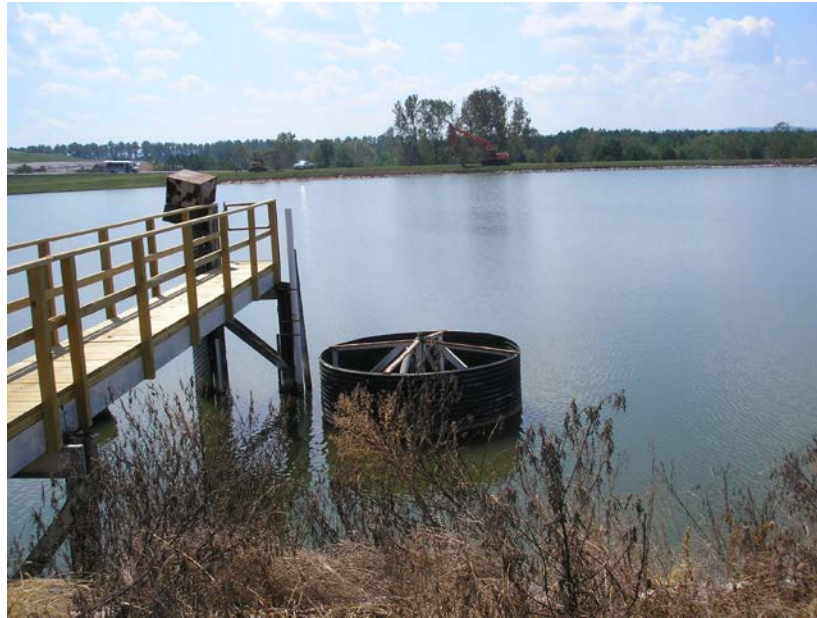
Figure 5.4.1-3: Ash Pond 5 Drainage Basin Rise Spillway
