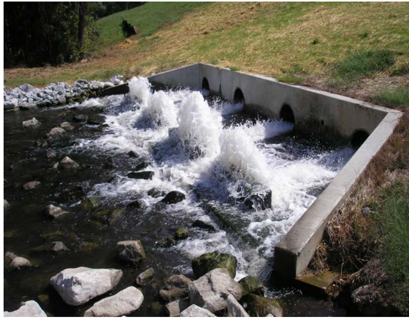
Photograph 5.4.2-1: Ash Pond 4 Spillway Conduits and Outlet Structure
