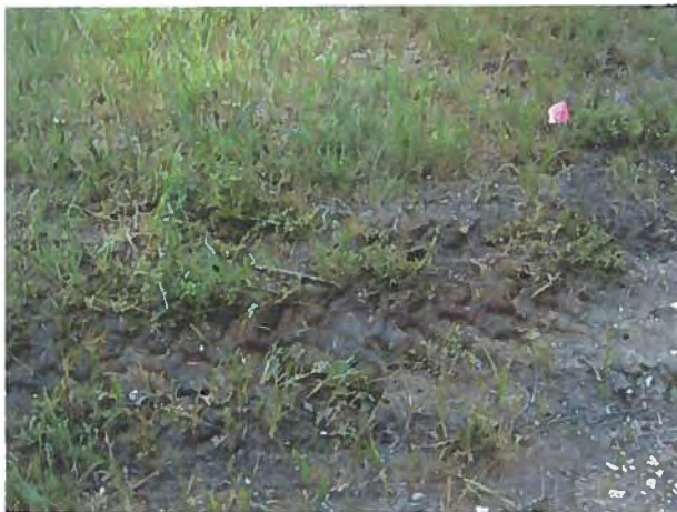
Photo 6 Rutting in soft, relatively damp area. TVA survey point #3006.
