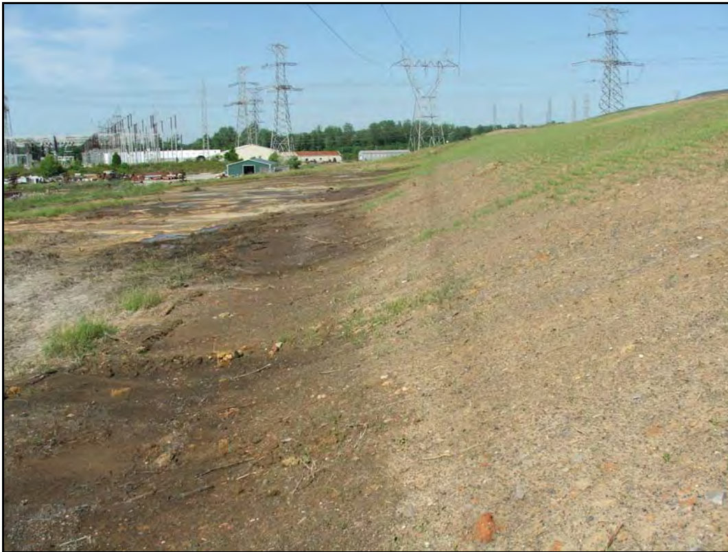
Figure 2. Example of Action Level 1 – Non-Flowing – Wet Area
