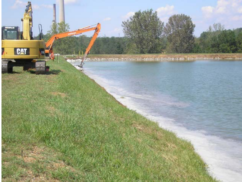
Photograph 5.3.2-2: Disposal Area 5 Drainage Basin South Embankment Inside Slope; Track Hoe Installing Riprap for Wave Erosion Protection.
