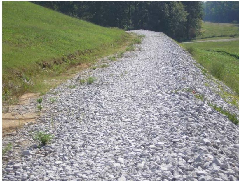
Photograph 5.2.4-1: Southeast Outside Groin with Inverted Filter Drain and Buttress
