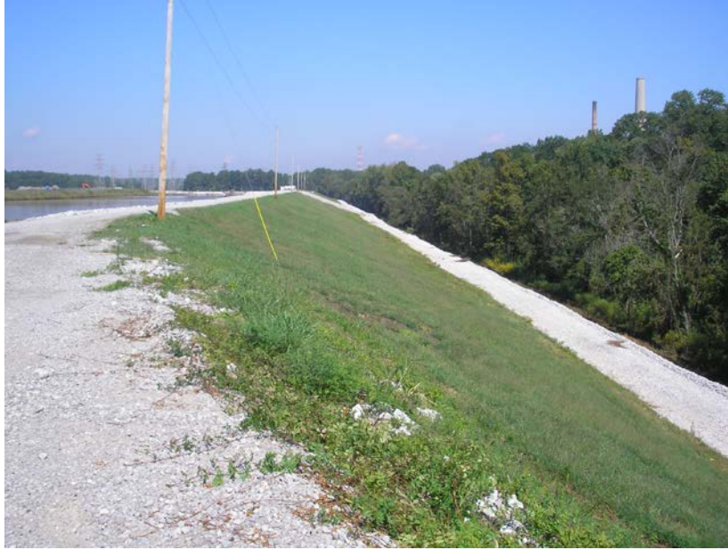
Photograph 5.2.3-1: Outside Slope of East Embankment with Inverted Filter Drain and Riprap Buttress
