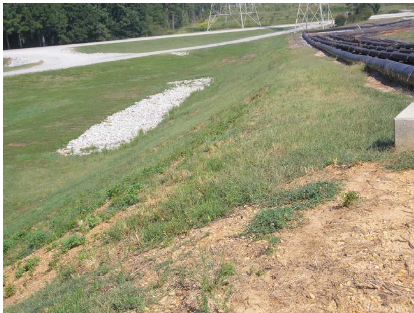
Photograph 5.2.3-2: Seepage Blanket at Toe of West Embankment North End
