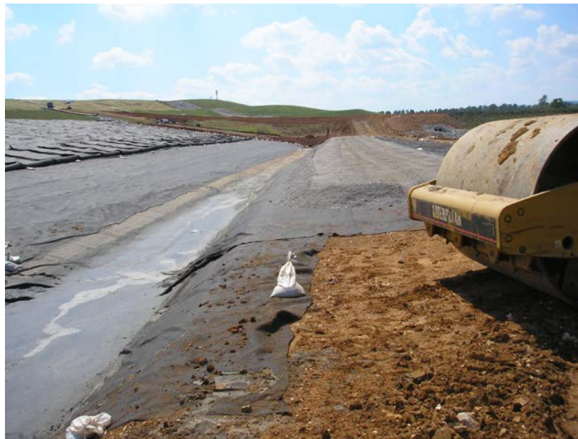
Photograph 5.3.2-1: Disposal Area 5 Ash Stack Perimeter Ditch Construction Along Inside of Impoundment Embankment Crest.
