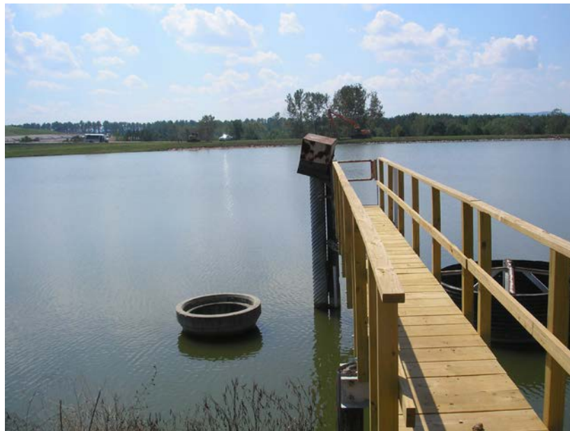
Photograph 5.4.1-4: Ash Pond 5 Drainage Basin Inactive Riser
