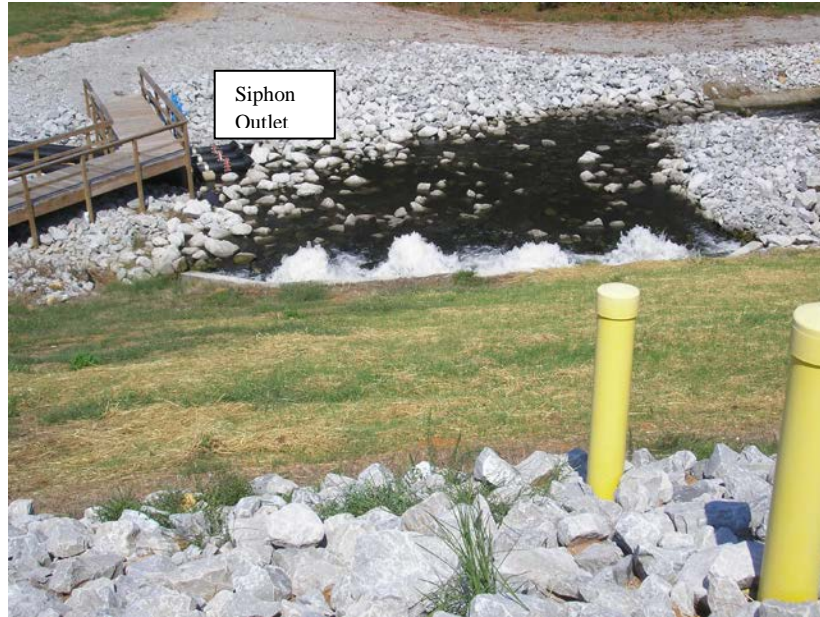
Photograph 5.4.2-2: Spillway Discharge Channel. Outlet End of Siphon Pipes to Right of Walkway in top Left Portion of Photograph.
