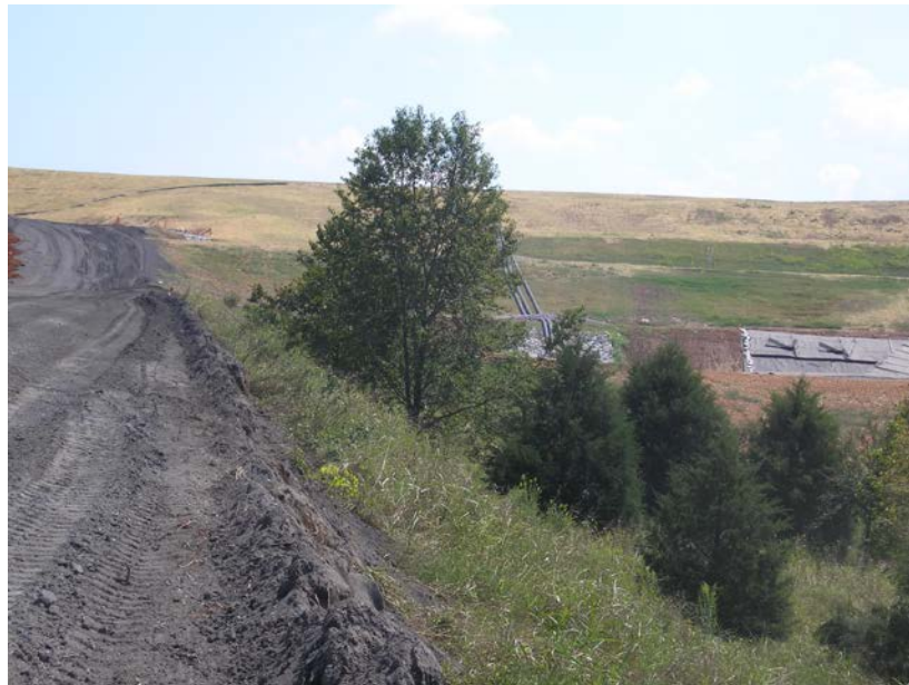
Photograph 5.3.3-3: Drainage Basin South Embankment Trees on Outside Slope
