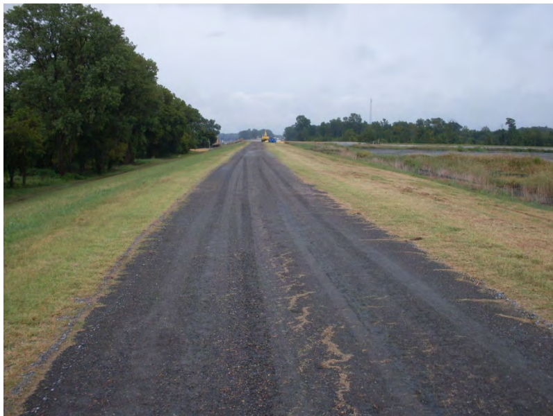
Photo 5.2: EAP Perimeter dike crest north side, looking east.
