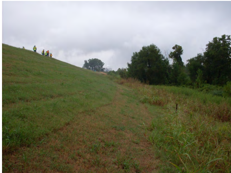
Photo 5.14: EAP Perimeter dike outside slope east side, looking north.
