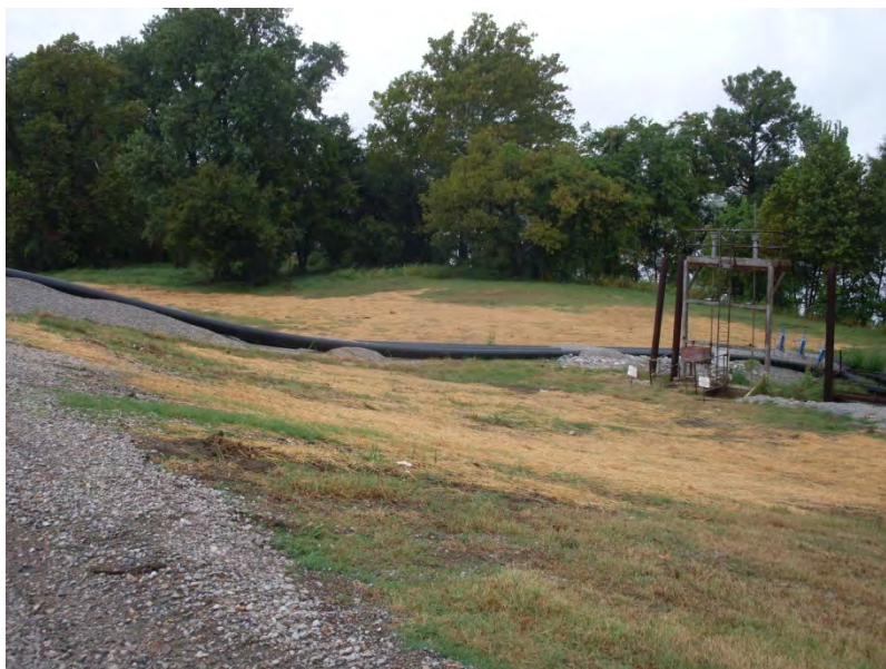
Photo 5.25: EAP Partial view of siphons, looking west.
