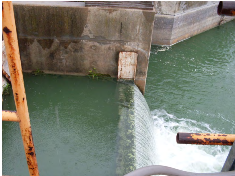
Photo 5.19: EAP South bay of concrete spillway in divider dike, discharging into stilling pond.
