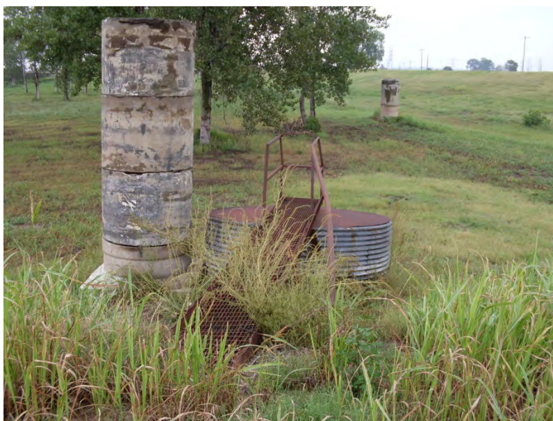
Photo 5.21: WAP View of old overflow riser in inactive pond, looking east. Note extra RCP section on top of riser.
