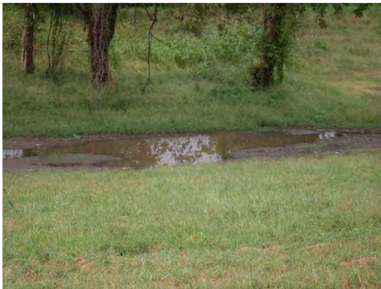
Photo 5.17: EAP Perimeter dike outside toe north side. Note ponded water.
