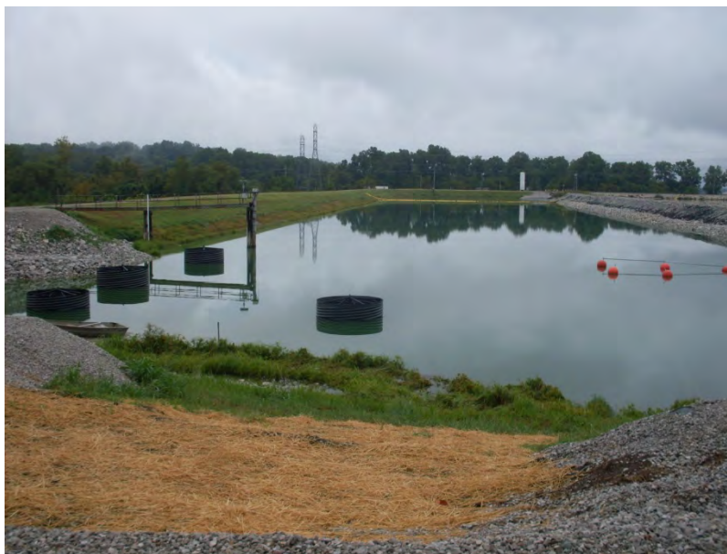
Photo 5.20: EAP View of skimmers atop overflow risers in stilling pond, looking south.
