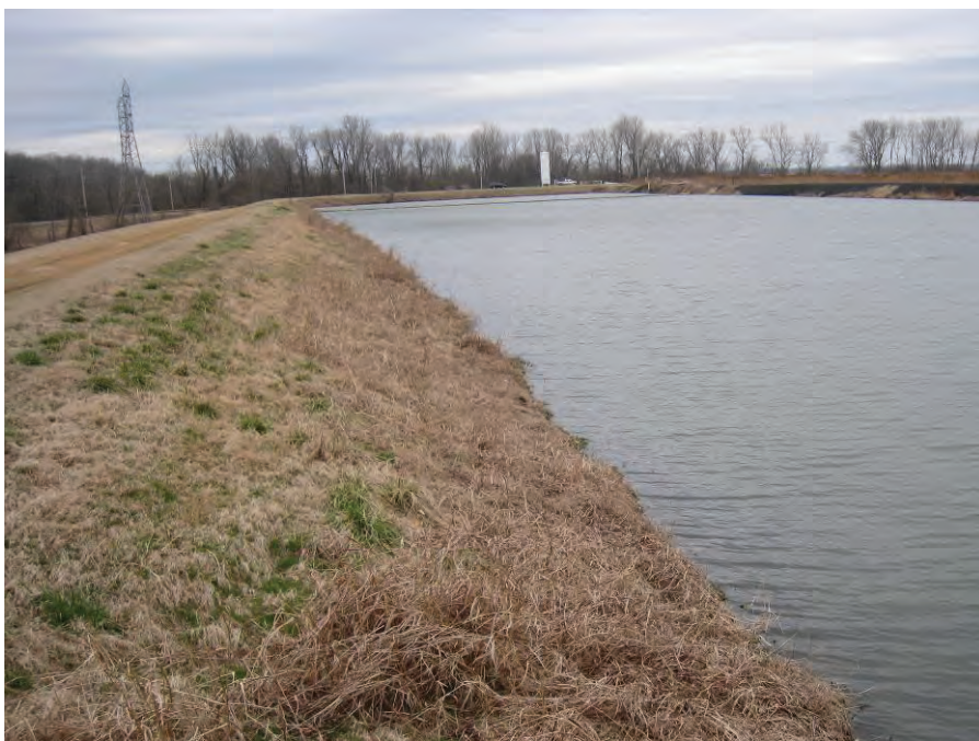
Drawing Mark EASP-10 Interior slope wave erosion.
