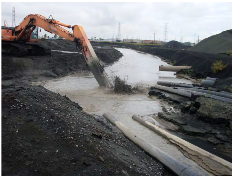
Photo 5.8: EAP Excavation of fly ash in dredge cell, looking south. Note greenish stockpile of boiler slag/bottom ash in background.
