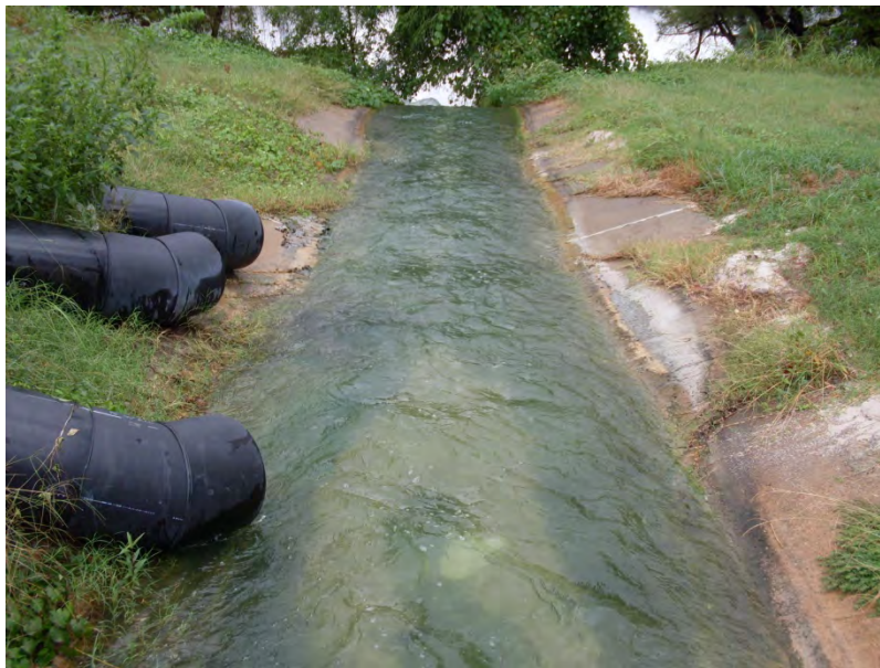
Photo 5.23: EAP View of flume to Lake McKellar, looking north. Note outlet ends of siphons.
