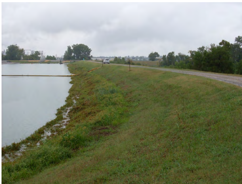
Photo 5.5: EAP Perimeter dike inside slope east side (stilling pond), looking north.
