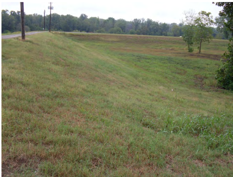
Photo 5.11: WAP Typical view perimeter inside slope west side, viewed north.
