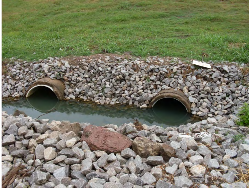
Photo 5.24: EAP View of outlet ends of emergency spillway conduits, looking west.
