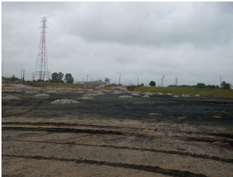
Photo 5.13: WAP View of apparent ash fill at east end of pond, viewed southeast. Note stone piles as deterrent for Least Tern nesting.
