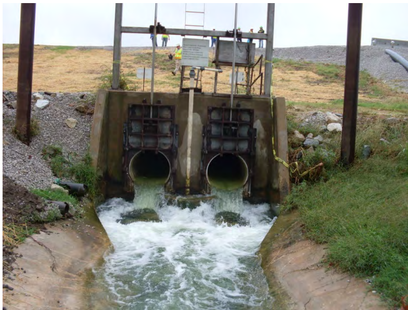
Photo 5.22: EAP View of outlet ends of primary spillway conduits, looking south.
