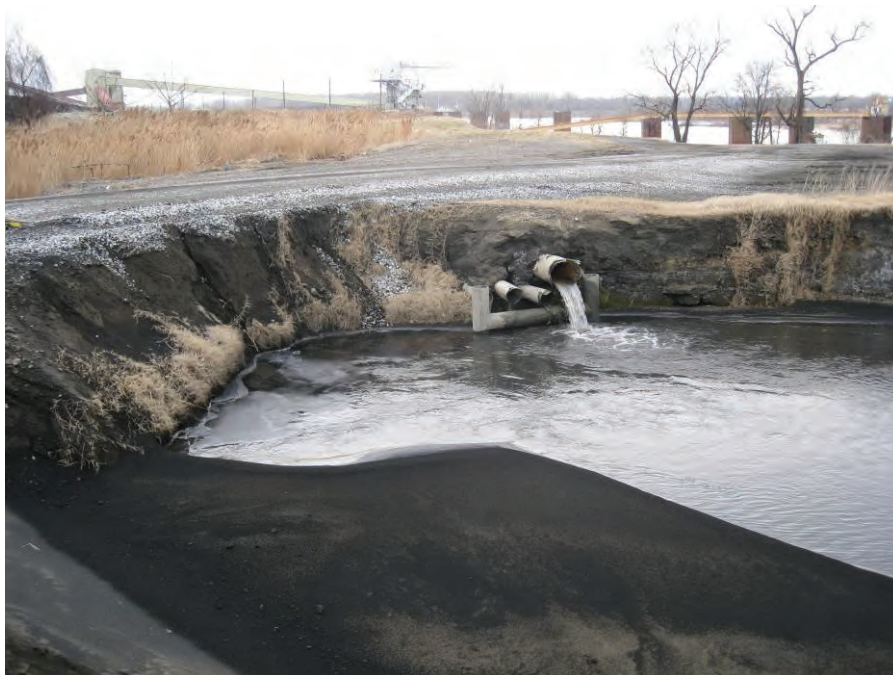
Drawing Mark EAP-3 Fly Ash influent pipes at northwest corner.
