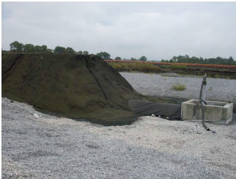
Photo 5.9: EAP South end of temporary bypass construction for active sanitary sewer under dredge cell.
