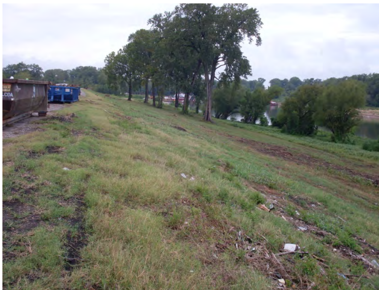
Photo 5.18: WAP Perimeter dike outside slope north side. Note dumpsters for cleanup of debris from spring flooding.
