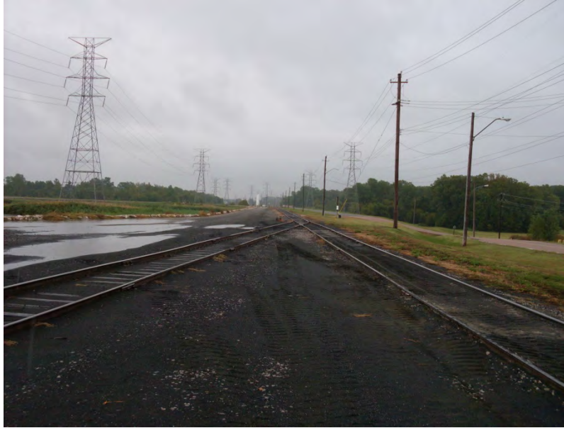
Photo 5.1: EAP Perimeter dike crest south side, looking east. Note ponded water.
