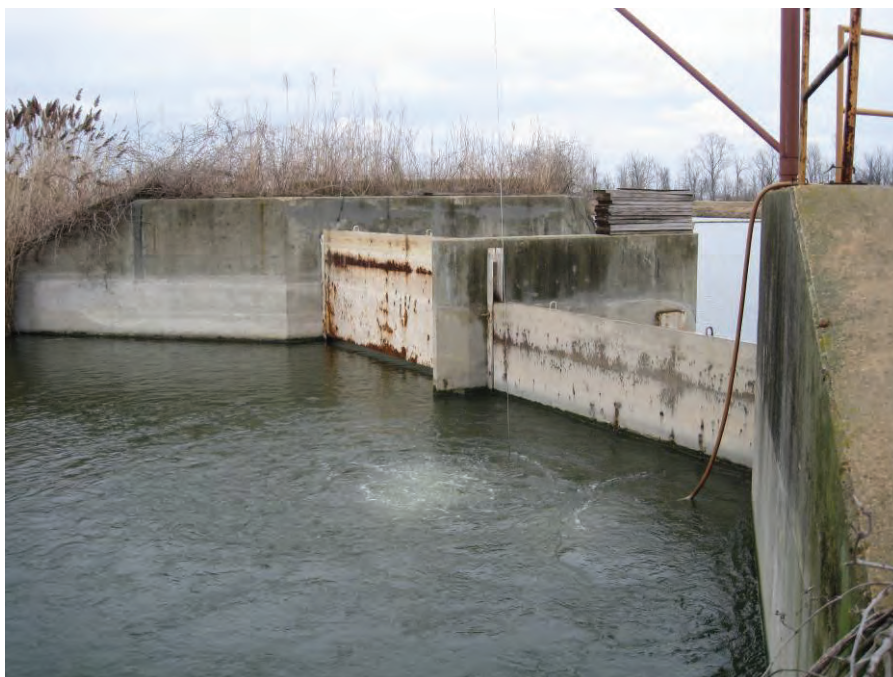
Drawing Mark EAP-2 Outlet Structure operated using stop logs.
