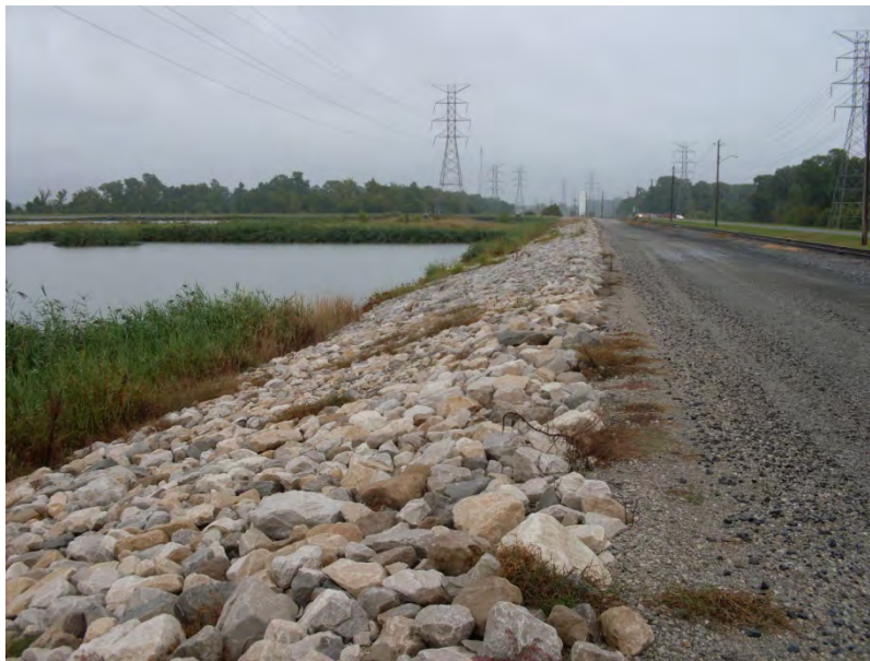
Photo 5.4: EAP Perimeter dike inside slope south side, looking east. Note riprap that was placed in 2010 to protect against wave erosion.
