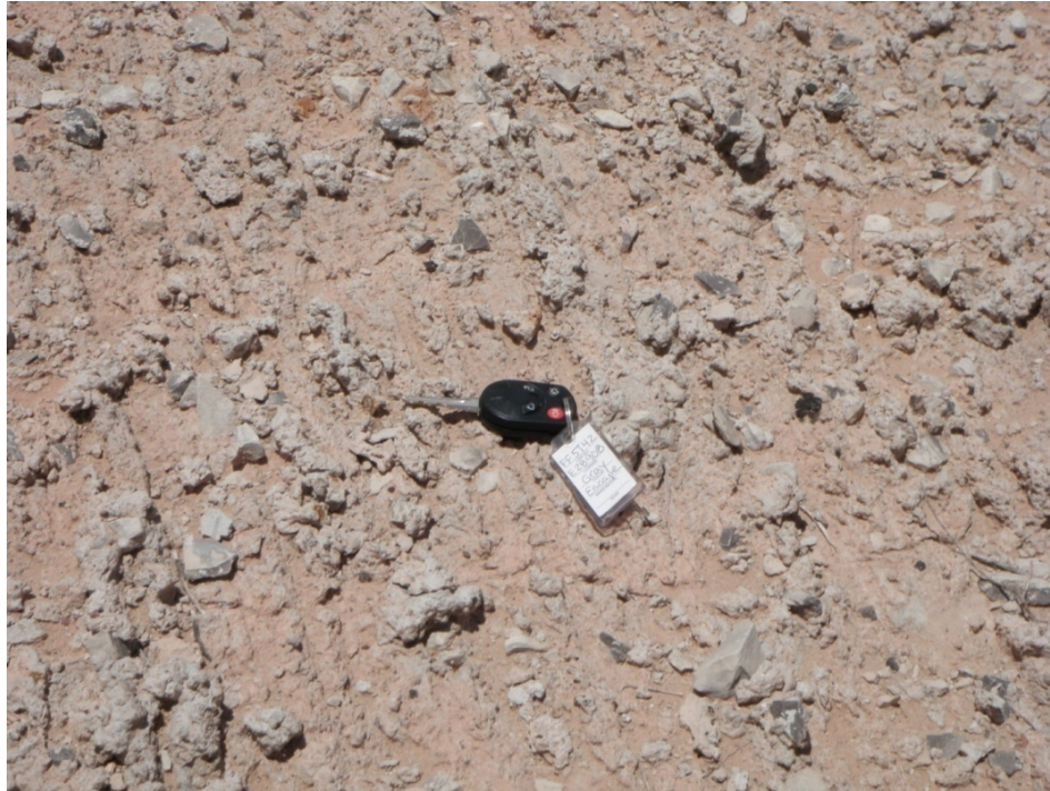
Photo 23: Evaporation Pond 5 : Raked liner finish
