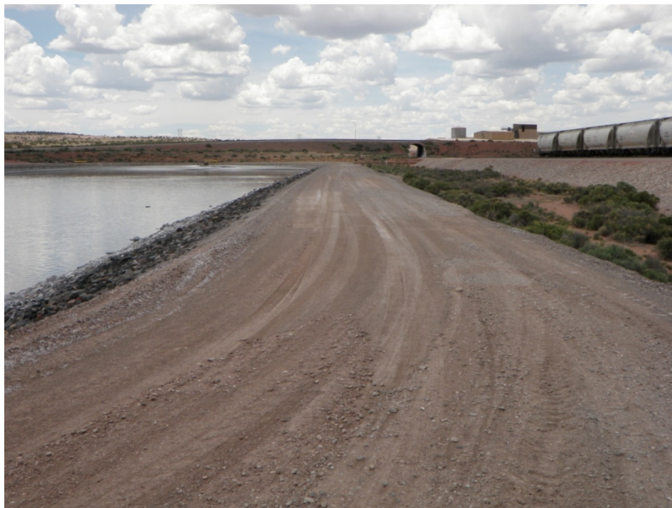
Photo 9: Bottom Ash Pond – North : Crest : Looking West along North Dike
