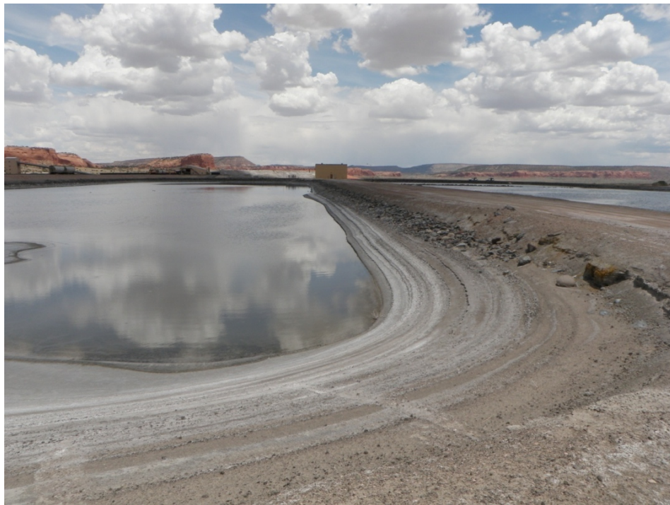
Photo 12: Bottom Ash Pond – North : Upstream Toe : Looking East along South Dike
