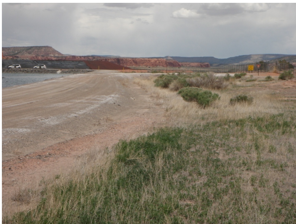
Photo 14: Bottom Ash Pond – South : Downstream Toe : Looking East along South Dike
