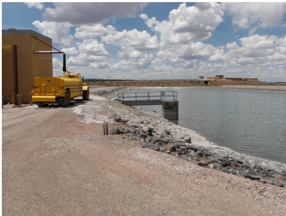
Photo 6: Bottom Ash Pond – North : Crest/Upstream Toe: Looking West along South Dike
