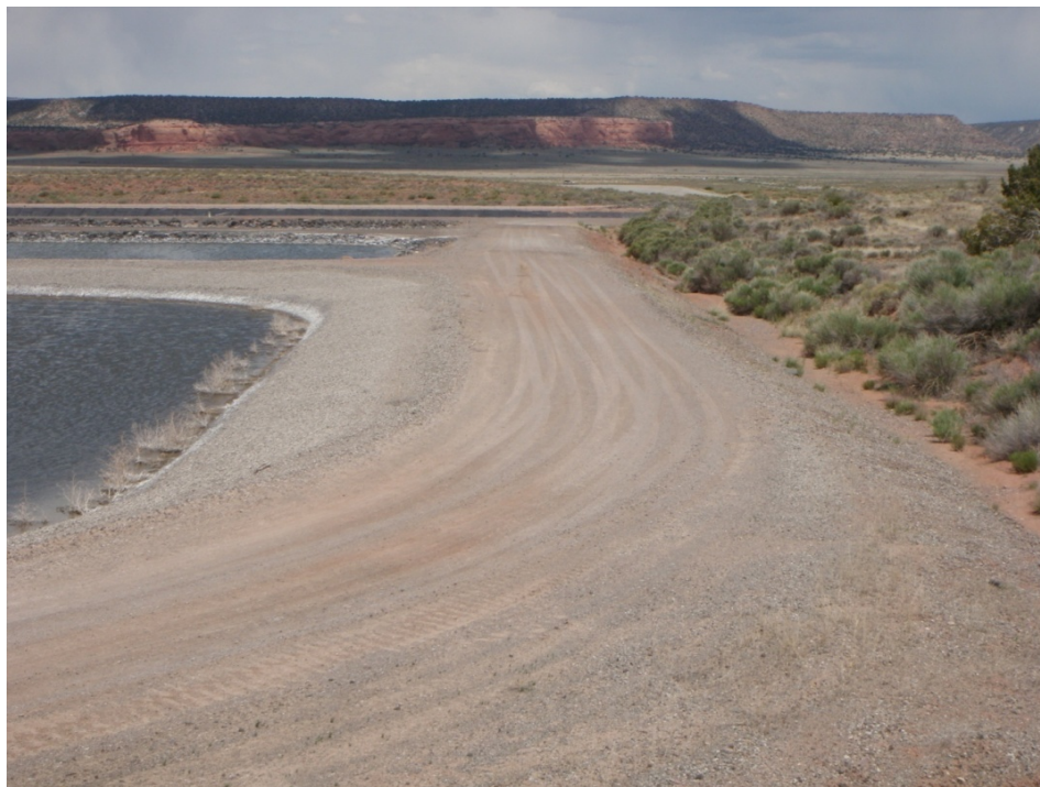
Photo 31: Evaporation Pond 1b : Crest : Looking East along south dike
