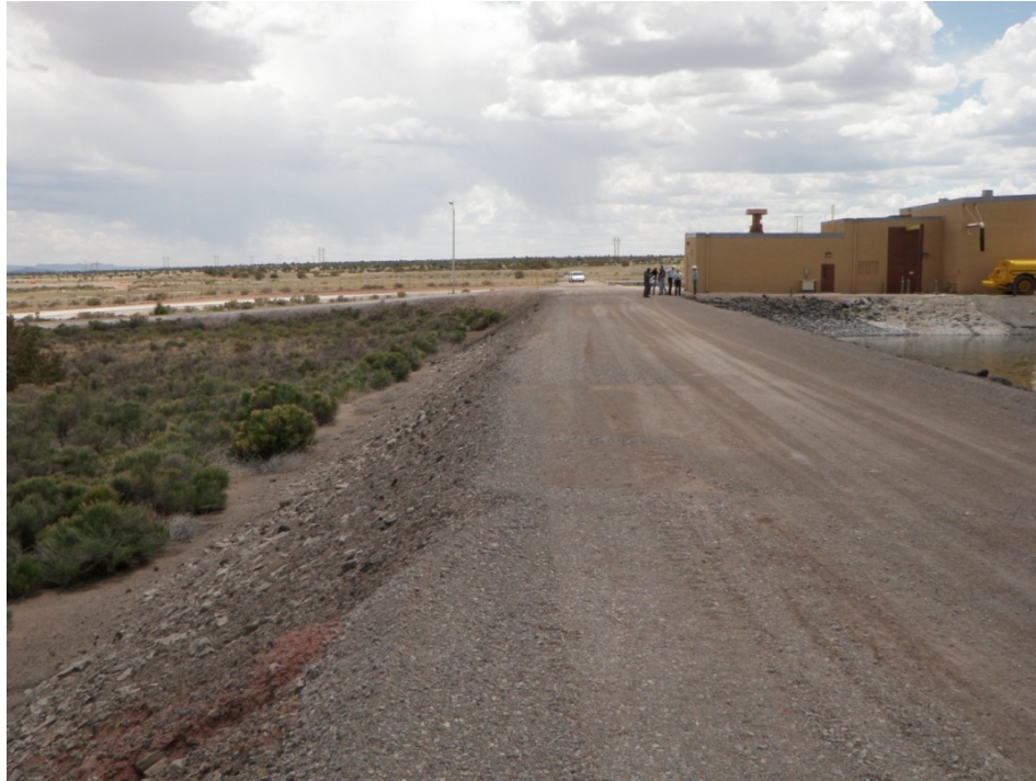
Photo 7: Bottom Ash Pond – North : Crest: Looking South along East Dike
