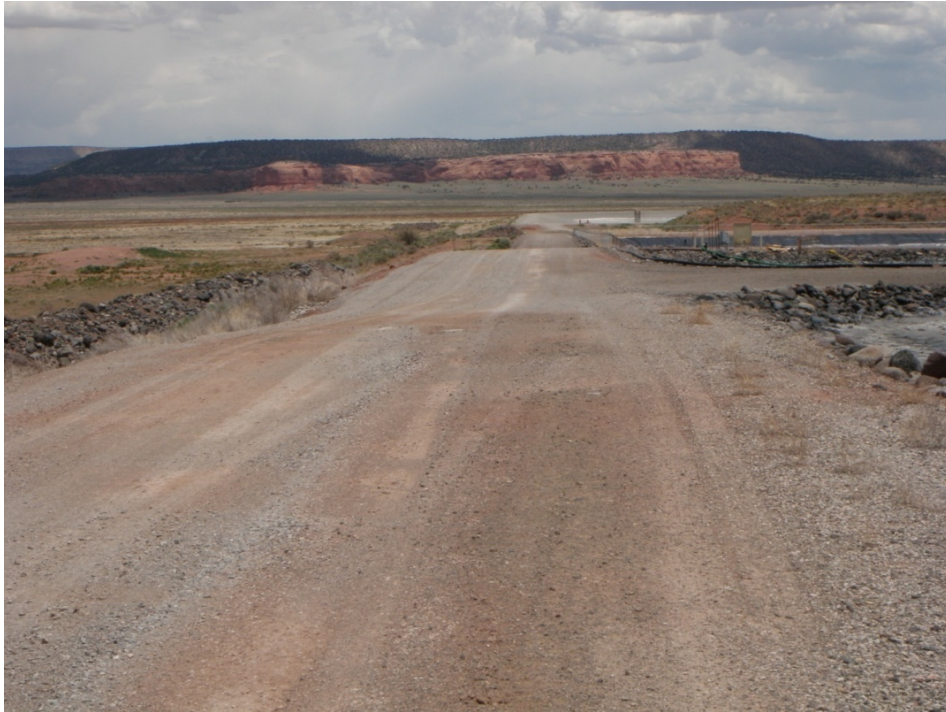
Photo 17: Evaporation Pond 2 : Crest : Looking East along North dike
