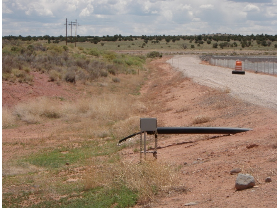
Photo 21: Evaporation Pond 4 : Downstream Toe : Looking South along east dike
