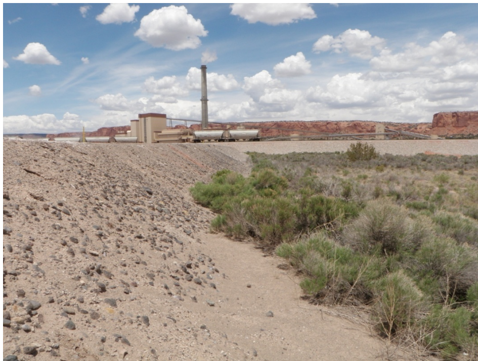
Photo 5: Bottom Ash Pond – North : Downstream Toe: Looking North along East Dike
