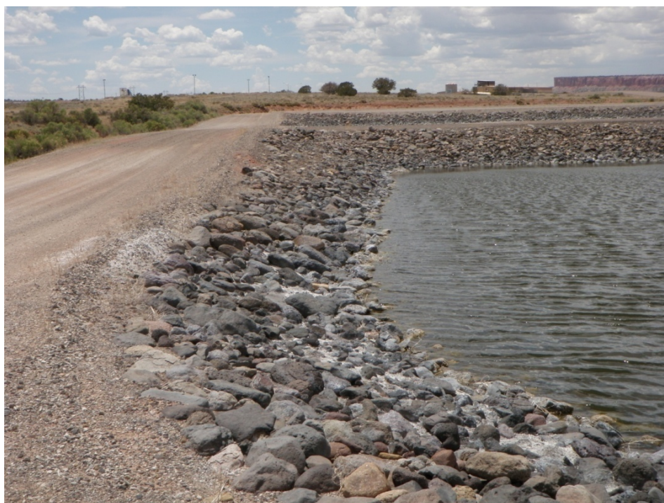
Photo 28: Evaporation Pond 3 : Upstream Toe : Looking West along south dike
