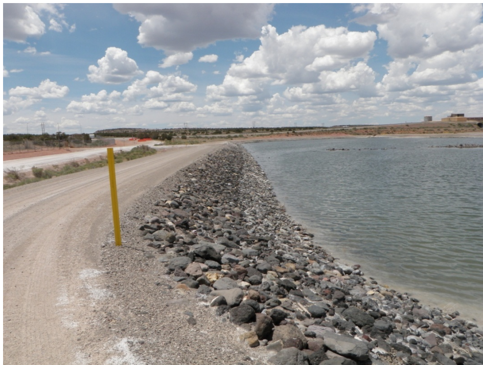
Photo 3: Bottom Ash Pond – South : Upstream Toe: Looking West along South Dike
