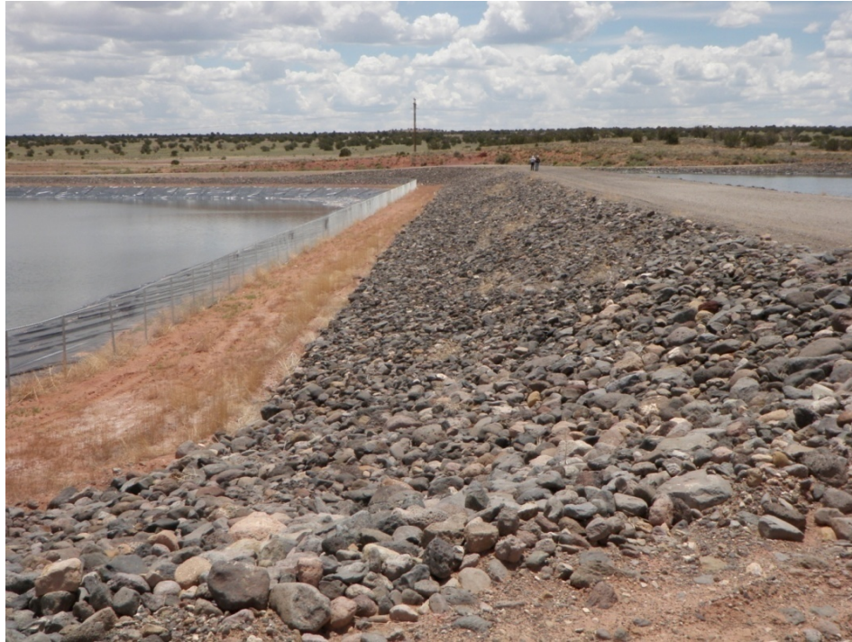
Photo 19: Evaporation Pond 4 : Upstream Toe : Looking South along West dike
