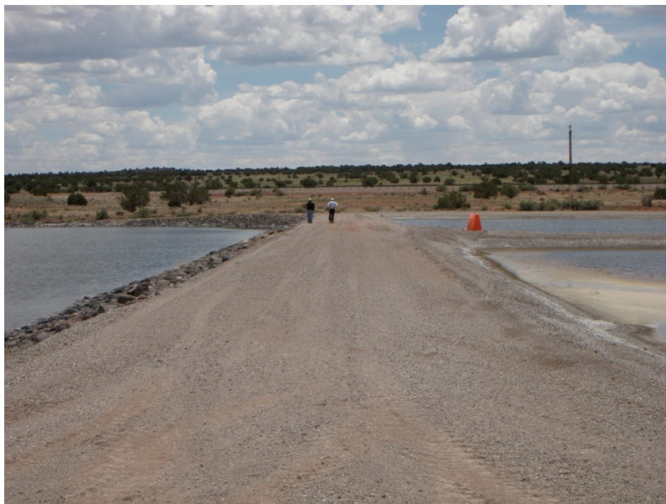
Photo 16: Evaporation Pond 2 (left) & 1a (right) & 1b (right background) : Crest : Looking South
