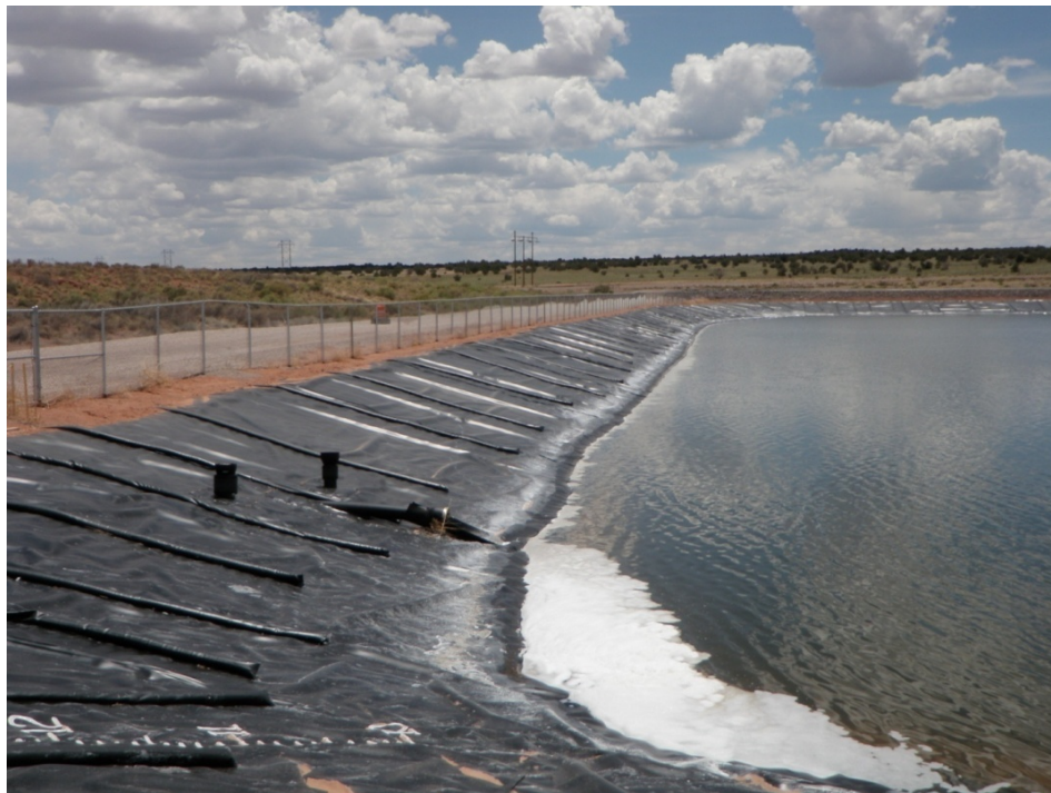
Photo 20: Evaporation Pond 4 : Upstream Toe : Looking South along east dike
