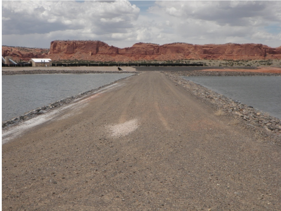
Photo 29: Evaporation Pond 2 (left) & Pond 3 (right) : Crest : Looking North
