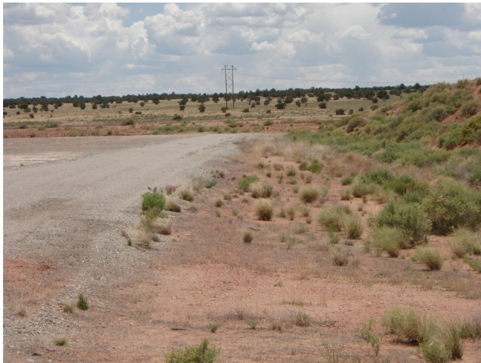
Photo 22: Evaporation Pond 5: Downstream Toe : Looking South along west dike
