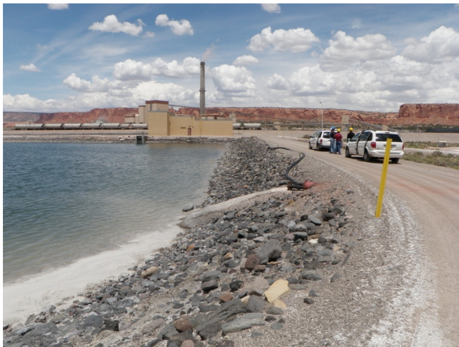
Photo 4: Bottom Ash Pond – South : Upstream Toe: Looking North along East Dike
