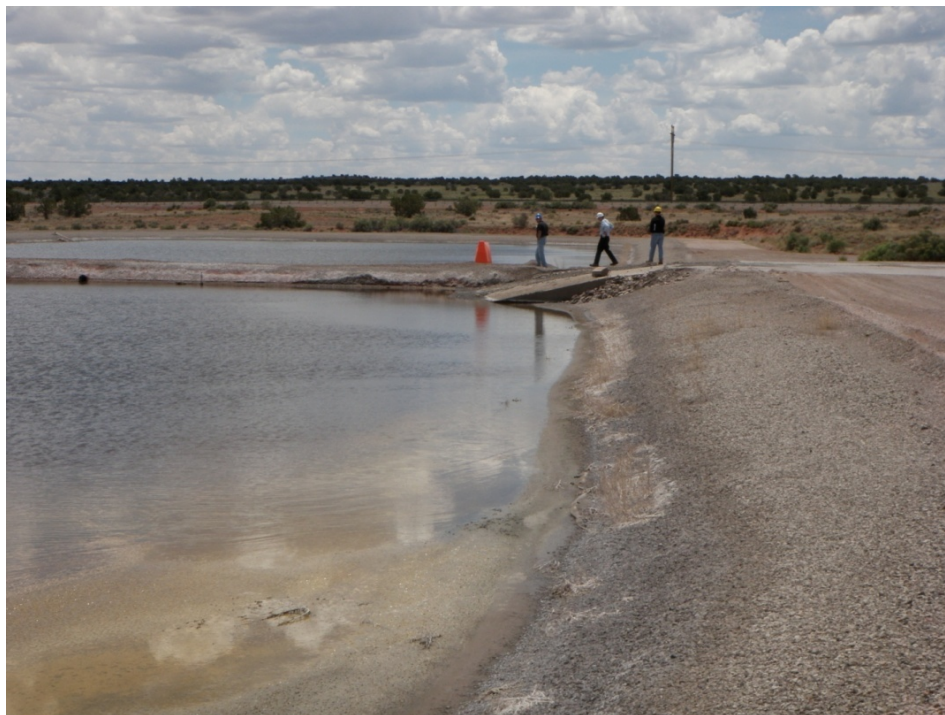
Photo 15: Evaporation Pond 1a : Upstream Toe : Looking South along West dike
