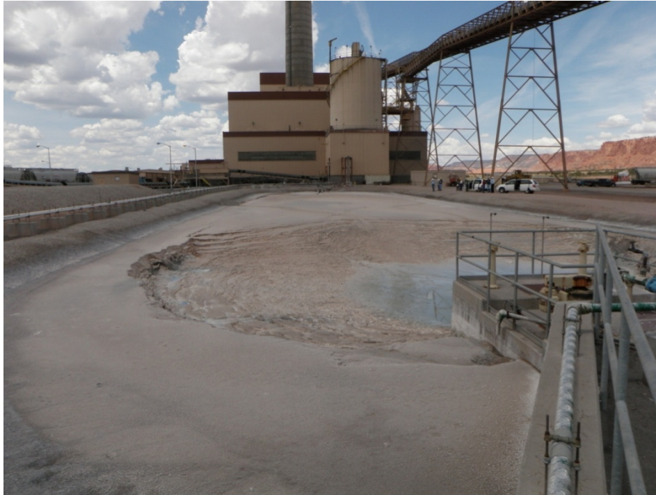
Photo 1: Emergency Scrubber Pond Looking West
