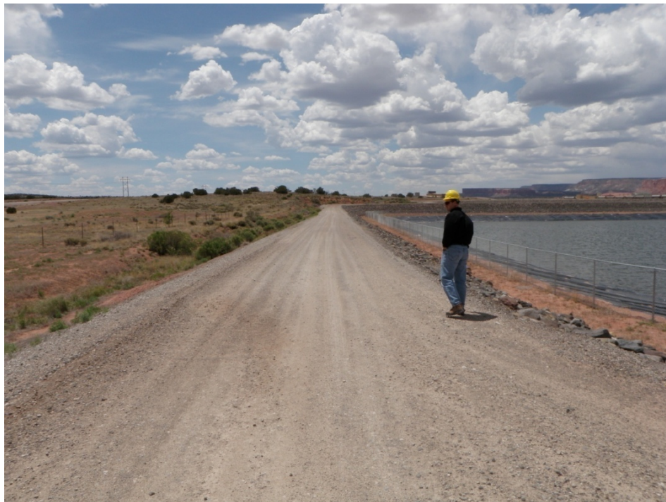
Photo 26: Evaporation Pond 4 : Crest : Looking East along south dike
