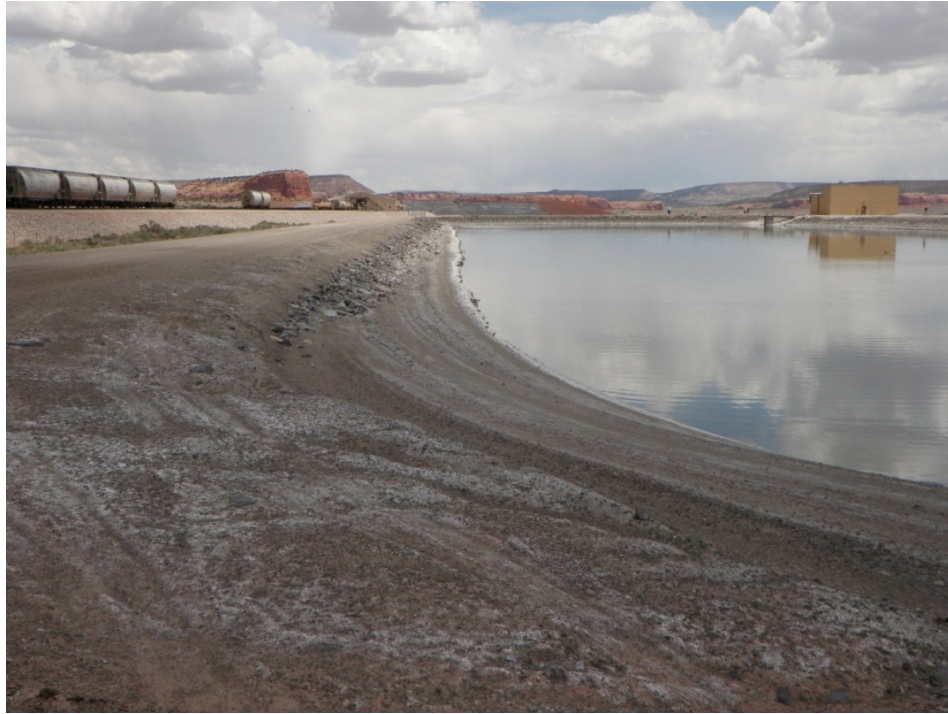
Photo 11: Bottom Ash Pond – North : Upstream Toe : Looking East along North Dike
