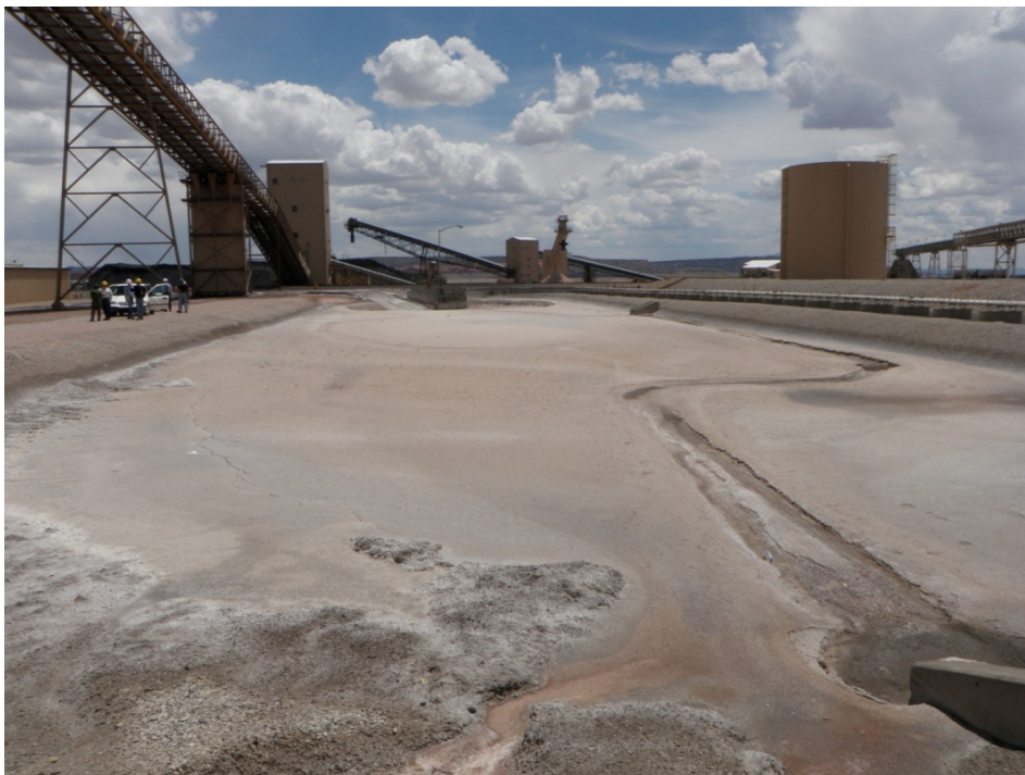
Photo 2: Emergency Scrubber Pond Looking East
