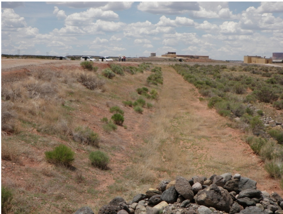
Photo 18: Evaporation Pond 2 : Downstream Toe : Looking West along north dike
