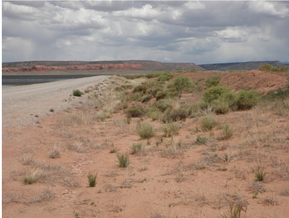
Photo 25: Evaporation Pond 5 : Downstream Toe : Looking East along south dike
