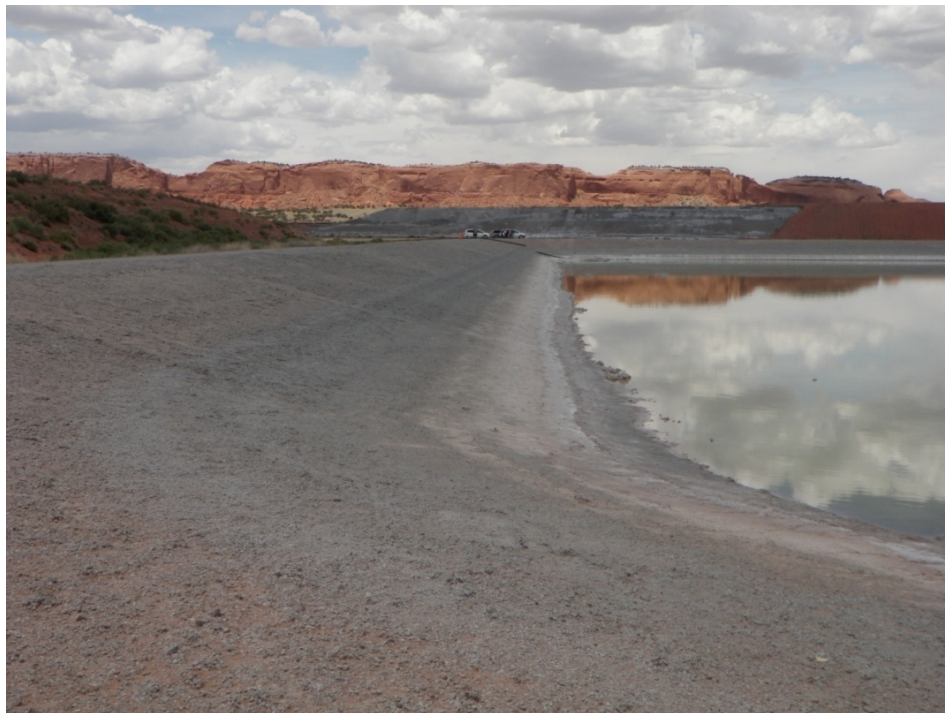
Photo 24: Evaporation Pond 5 : Upstream Toe : Looking North along west dike
