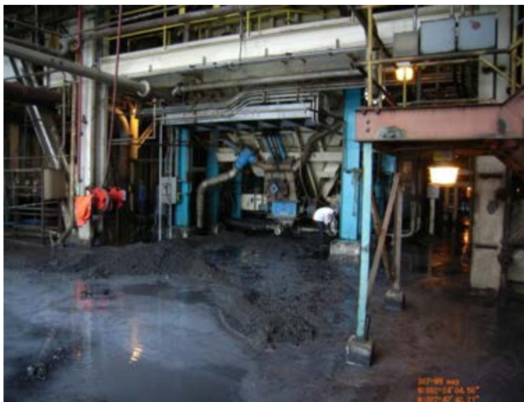
Boiler where boiler slag is collected
