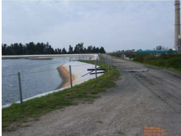
North Bottom Ash Pond Interior Lined Slope
