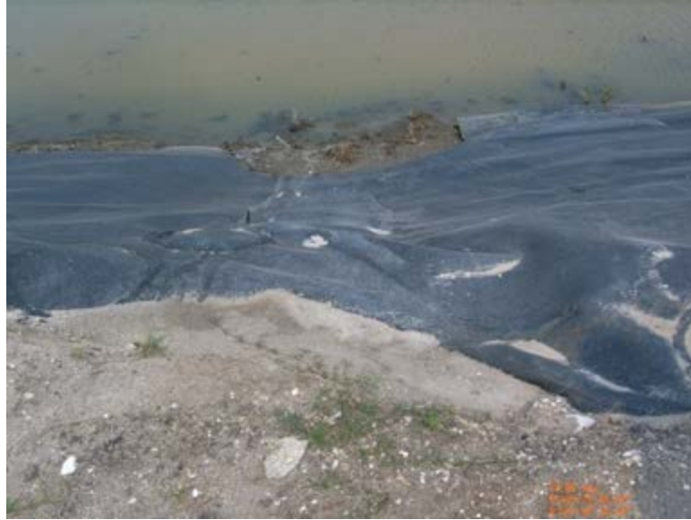
South Economizer Interior Lined Slope (Shear Failure In Liner)
