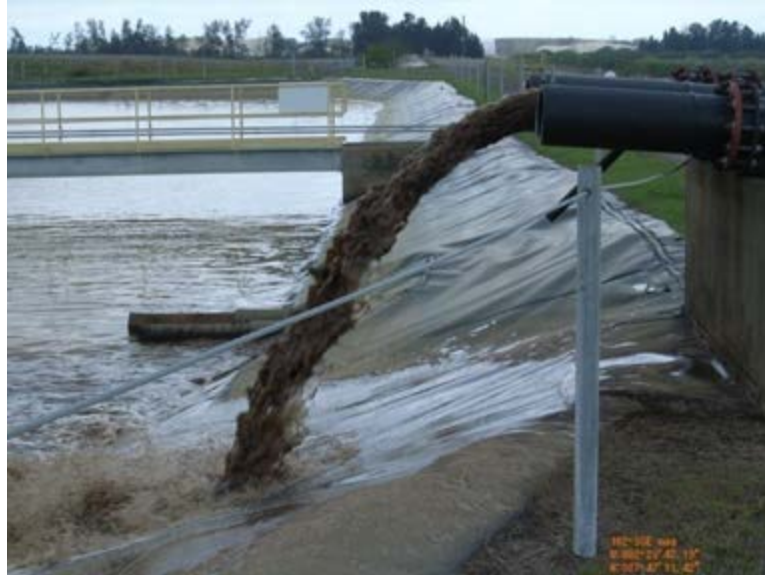
North Economizer Settling Pond Interior Slope and Influent Pipe
