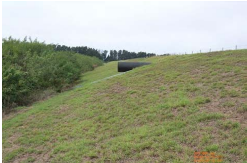
South Bottom Ash Pond Downstream Slope
