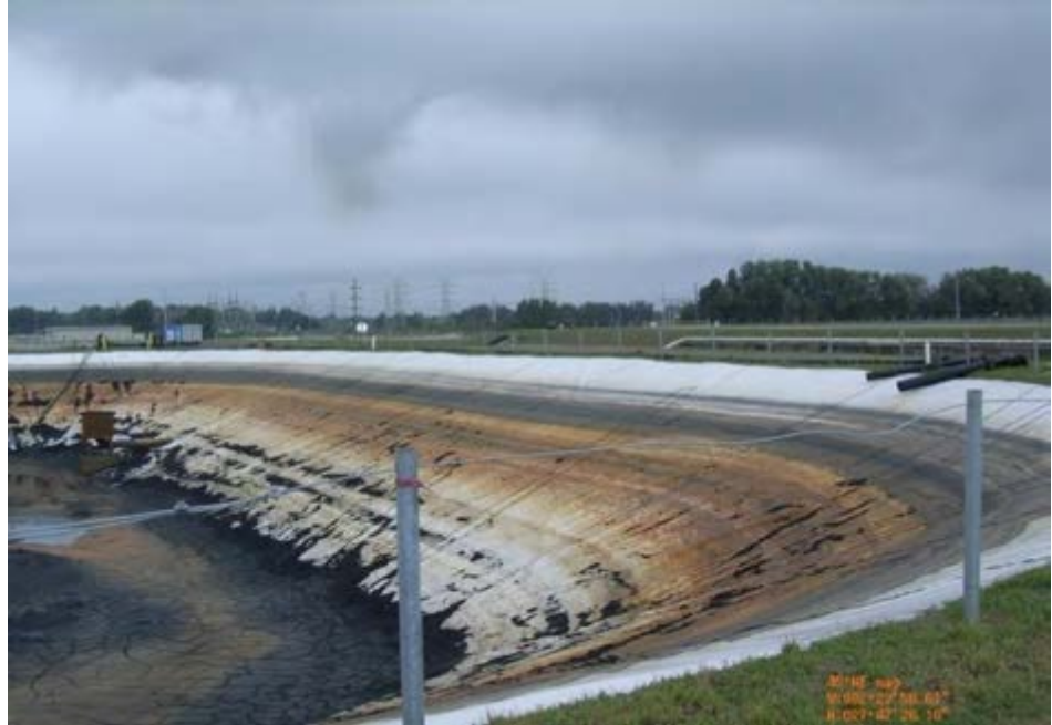
South Bottom Ash Pond Interior Lined Slope
