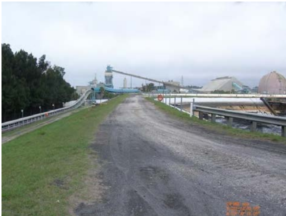
South Bottom Ash Pond Crest
