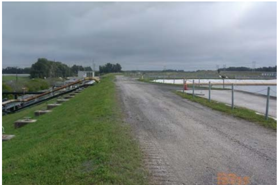
North Bottom Ash Pond Crest
