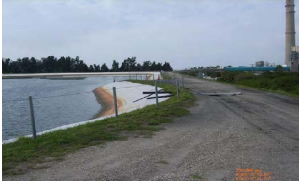
North Bottom Ash Pond Interior Lined Slope
