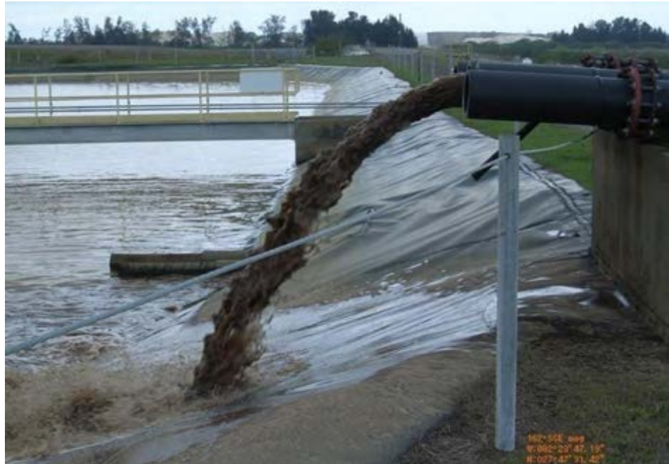
North Economizer Settling Pond Interior Slope and Influent Pipe
