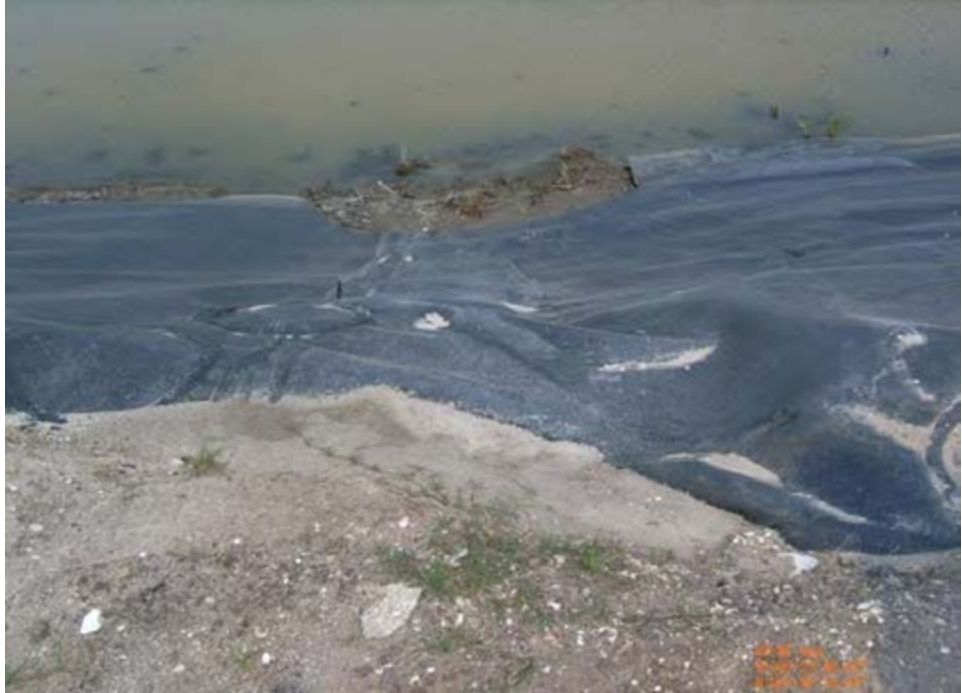
South Economizer Interior Lined Slope (Shear Failure in Liner)
