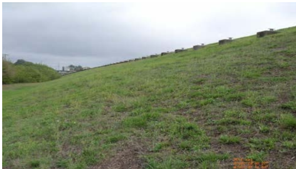
North Bottom Ash Pond Downstream Slope
