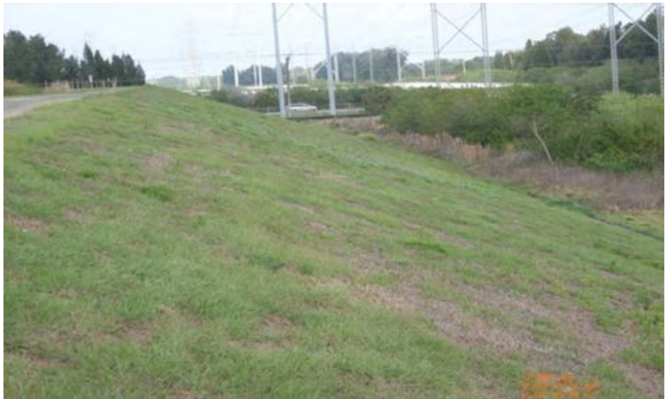
South Economizer Downstream Slope
