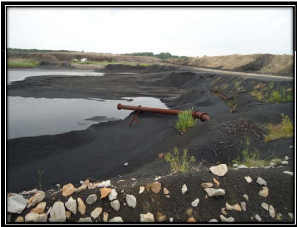
Photo 10 – Ash Pond 2 Inlet Sluice Pipe
