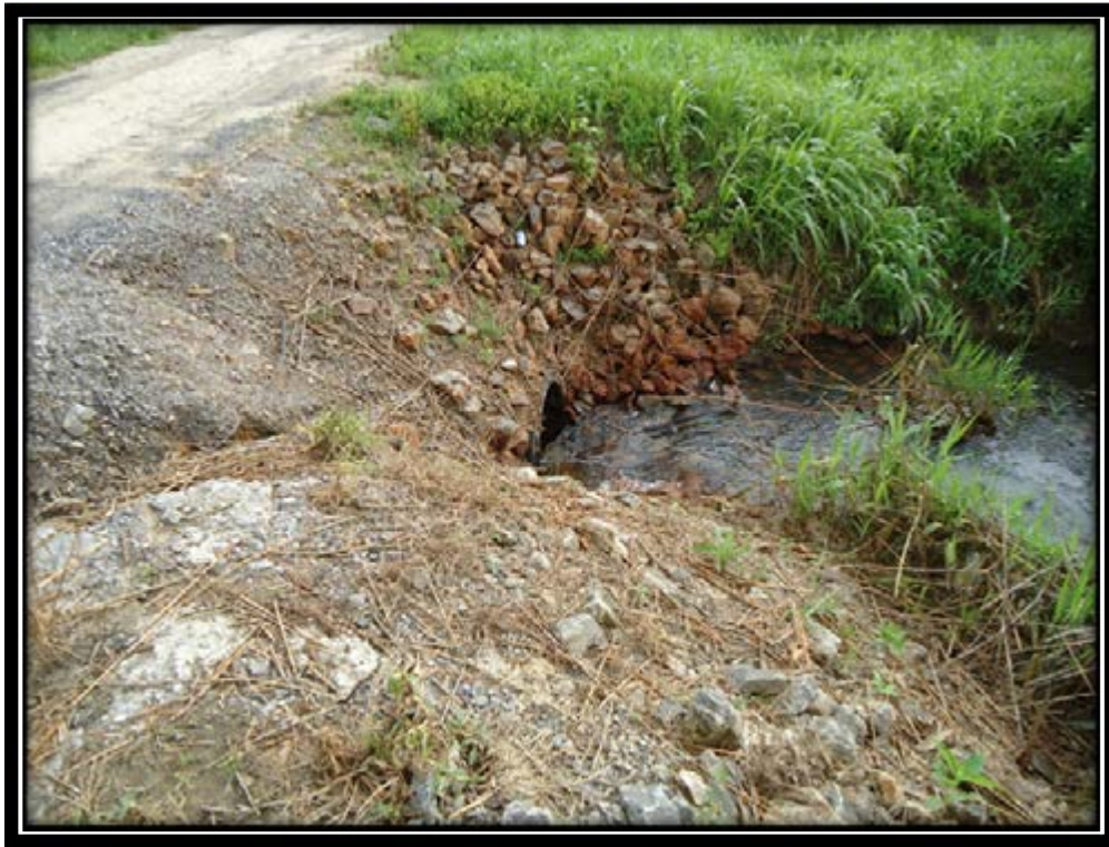
Photo 27 – Corrugated Metal Pipe under Access Road Leading to Outfall Downstream of Pond 4 May 25, 2011 IL50160
