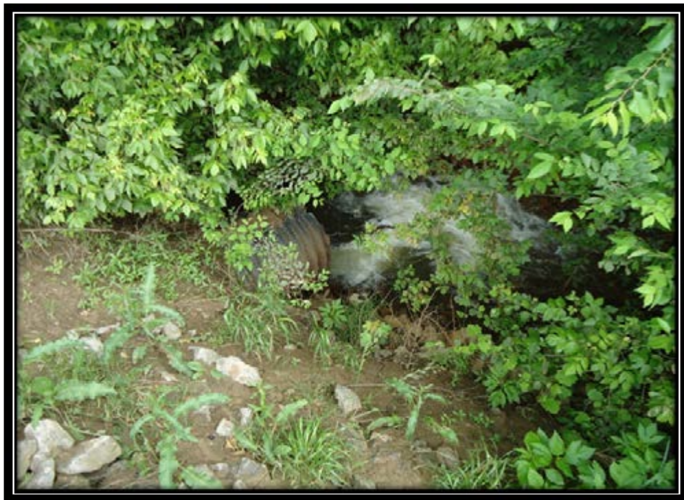
Photo 28 – Corrugated Metal Pipe Outfall from Ash Ponds to the South Fork of Little Saline Creek May 25, 2011 IL50160
