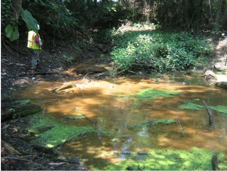
Figure 5.2.3a: Ash Pond 1 Downstream Seepage
