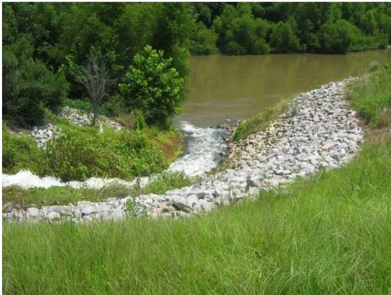
Figure 5.3.2: Ash Pond 2 Discharge into Wateree River
