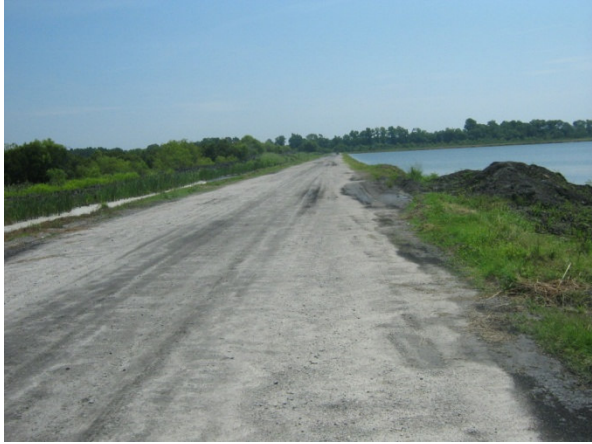
Photo 043: Internal Dike Crest
