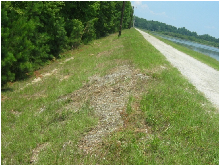
Figure 5.2.3b: Ash Pond 2 Downstream Slope
