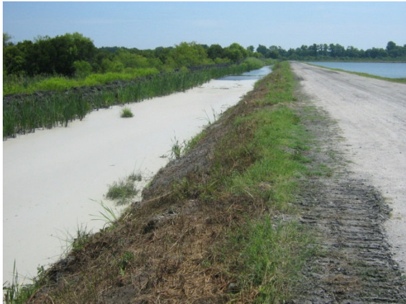
Photo 045: Internal Dike Upstream Slope
