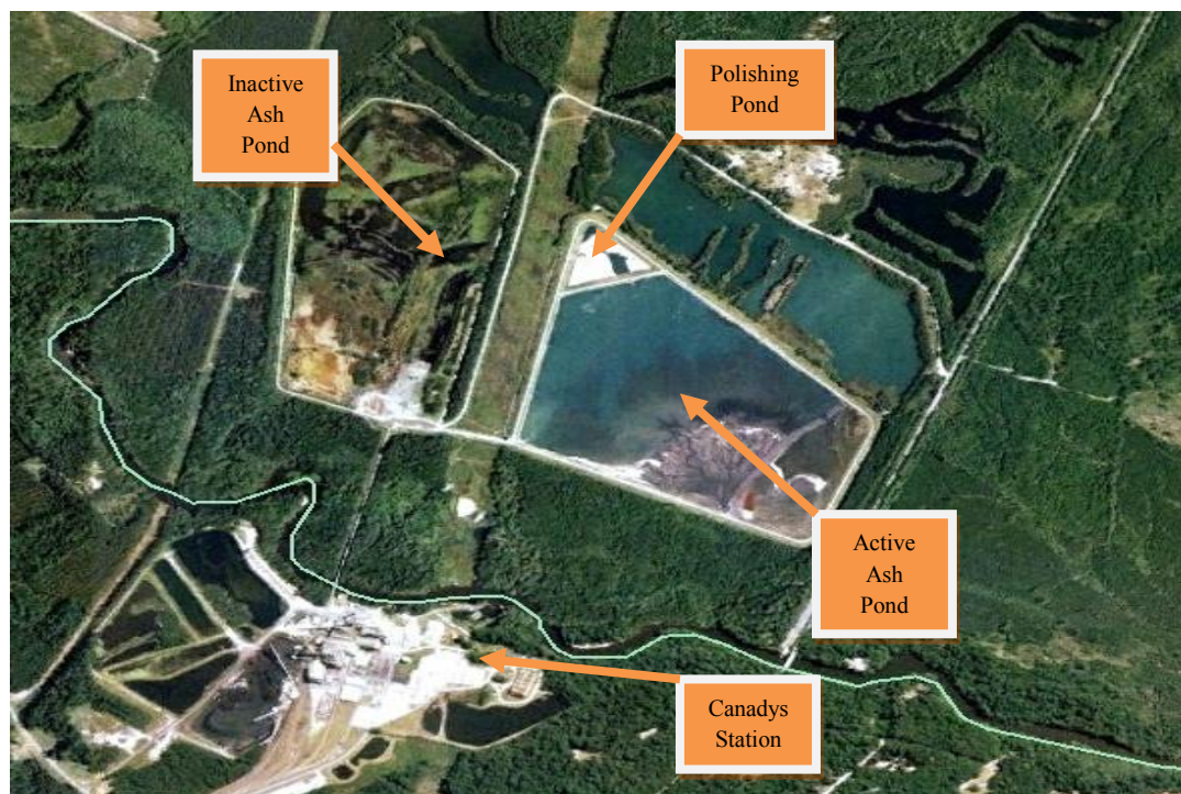
Figure 2.1b: Canadys Steam Power Station Aerial View
