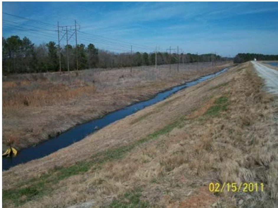
Photo 2. Channel along the downstream toe
