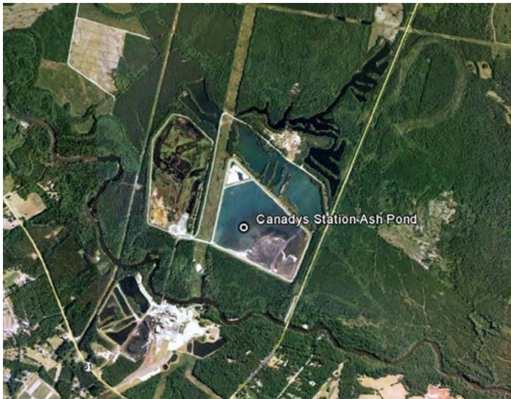
Figure 1. Aerial Image of Canadys Station Ash Storage Pond Site
