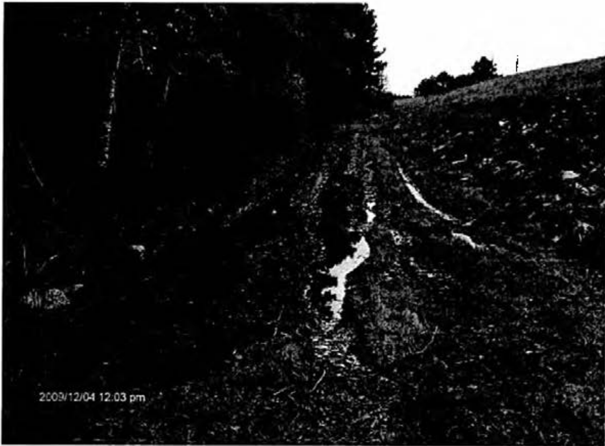
Figure 9: Example Damage from Driving Pick-Up Truck on Toe of Berm
