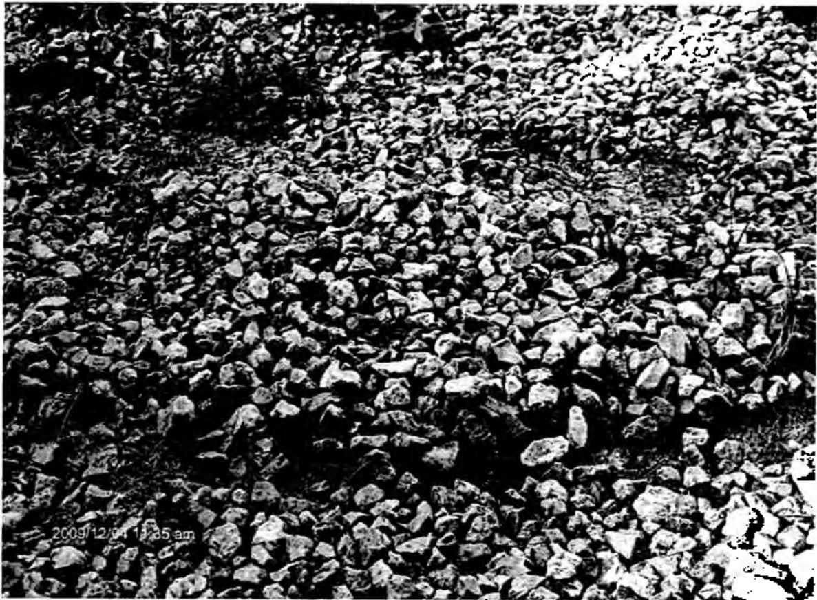
Figure 3: WA-1 at Time of Annual Inspection
