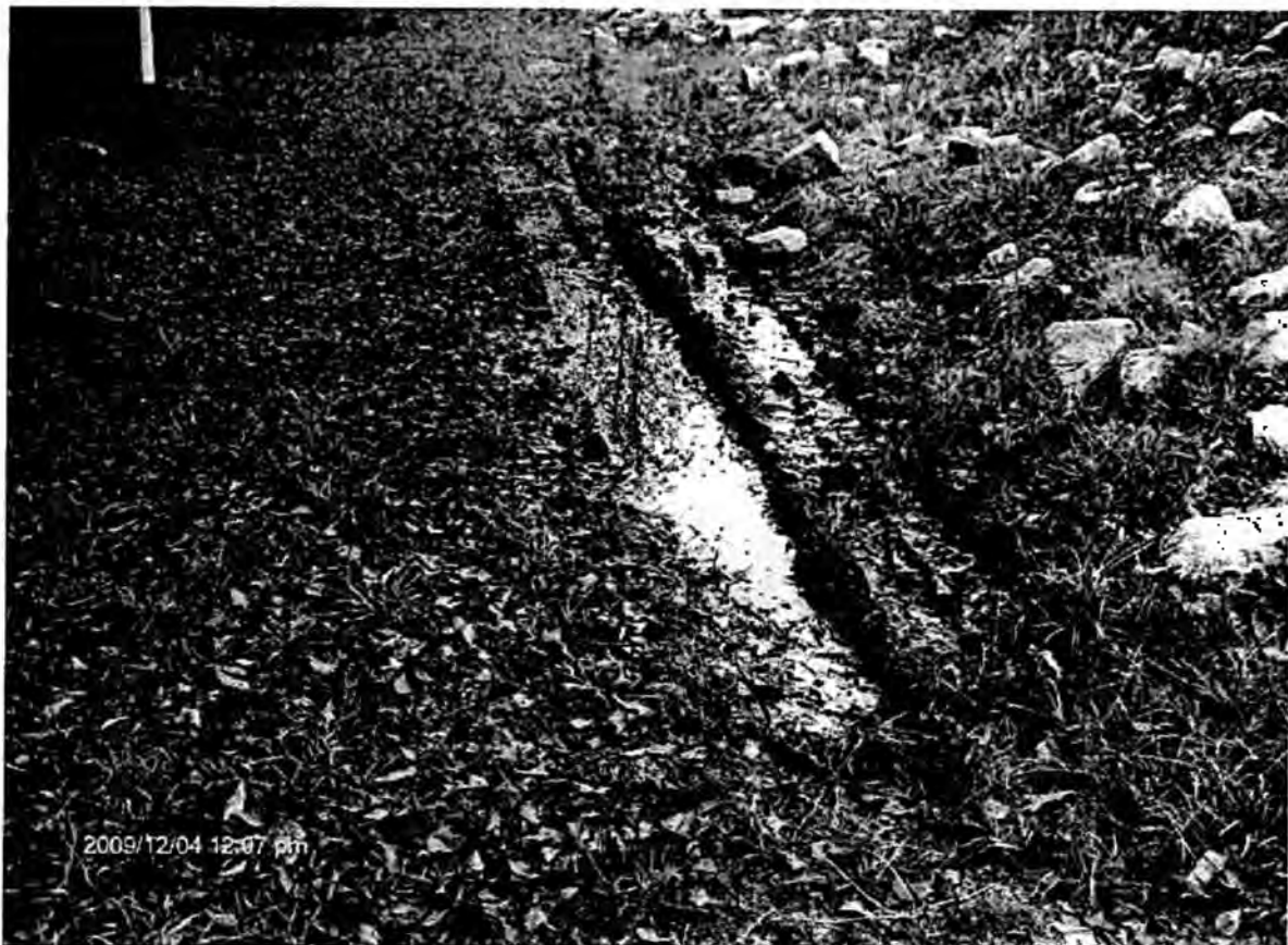
Figure 8: Example of Area of Standing Water Along Toe of Active Pond West Berm
