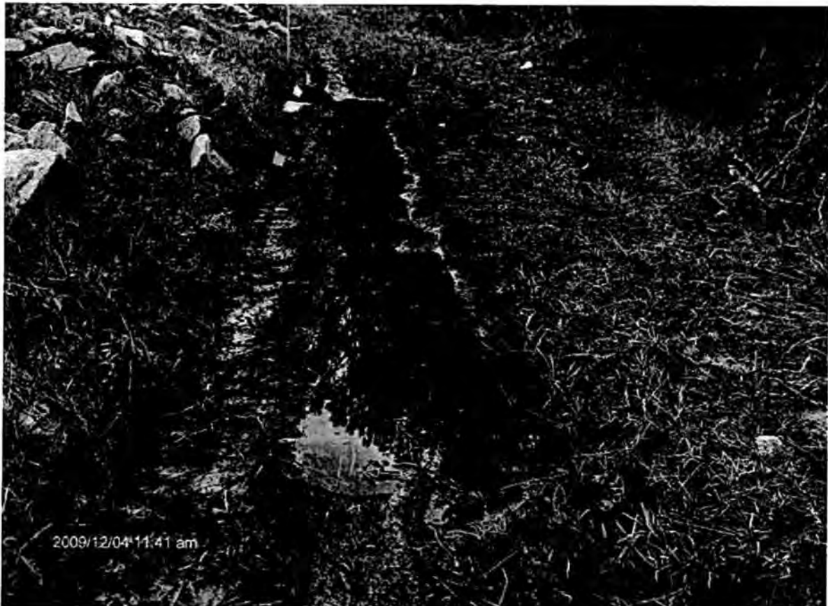
Figure 4: Standing Water Near Rip Rap Armoring at Southwestern Corner of Active Pond
