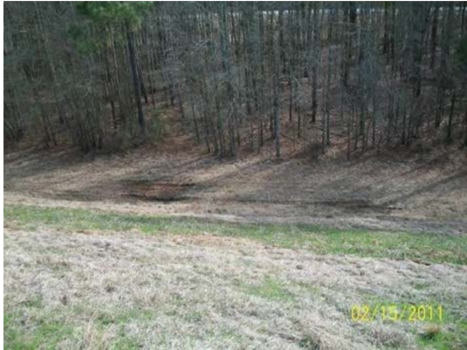
Photo 1. Standing water in vehicular traffic ruts
