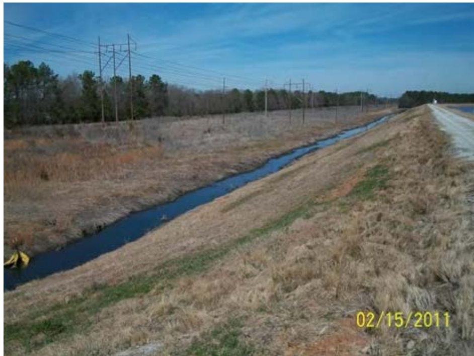
Photo 2. Channel along the downstream toe
