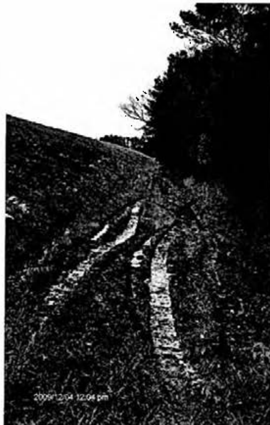
Figure 10: Example Damage from Driving Pick-Up Truck on Toe of Berm
