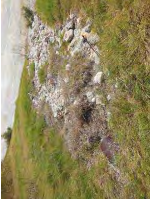
Photo 102: Approximately 3-ft-high area of erosion or settlement under stormwater inlet.
