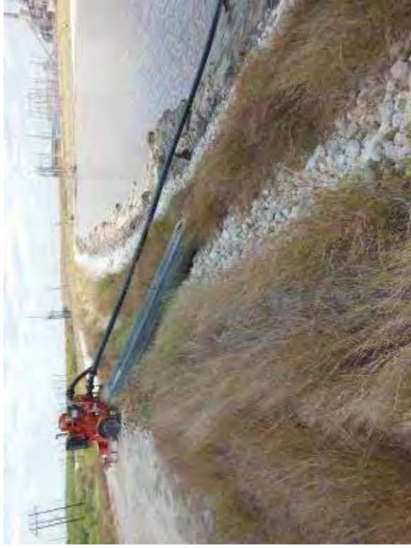
Photo 145: 6-inch-diameter outlet pipe and pump at south embankment interior slope, looking west.
