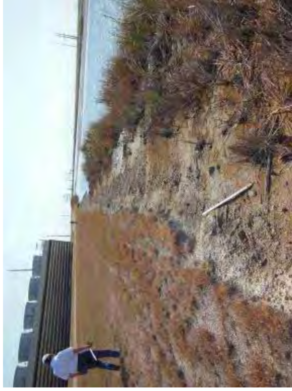
Photo 68: North embankment interior slope, looking east. Note vegetation growing on interior slope.
