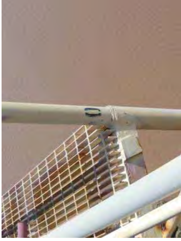
Photo 150: Reference mark for measuring water level in Sludge Basin. Zero corresponds to 18 inches of freeboard.
