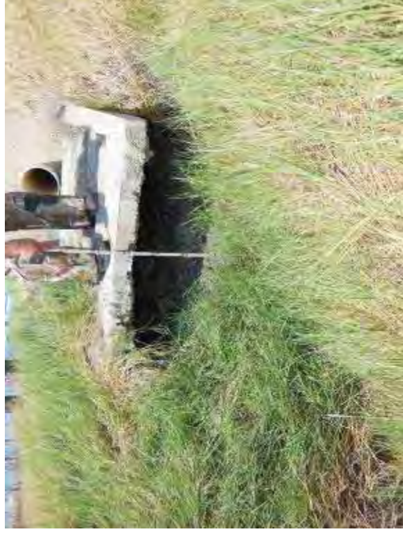
Photo 102: Approximately 3-ft-high area of erosion or settlement under stormwater inlet.
