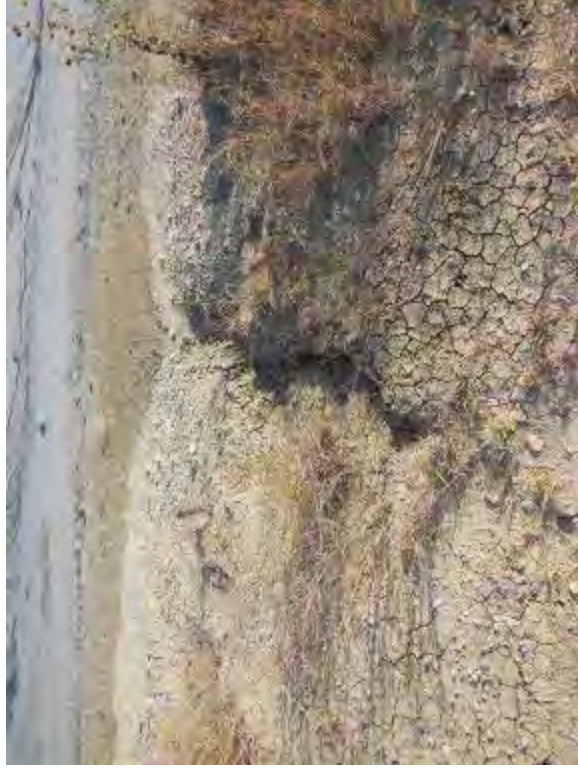
Photo 23: Erosion rills at south embankment interior slope.
