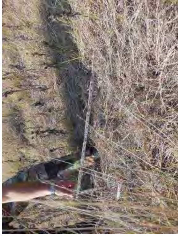
Photo 6: East embankment exterior slope approximately 2.5H:1V.
