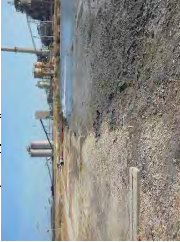
Photo 49: 24-inch-diameter steel outlet pipe at west embankment interior slope. PVC pipe along center embankment.
