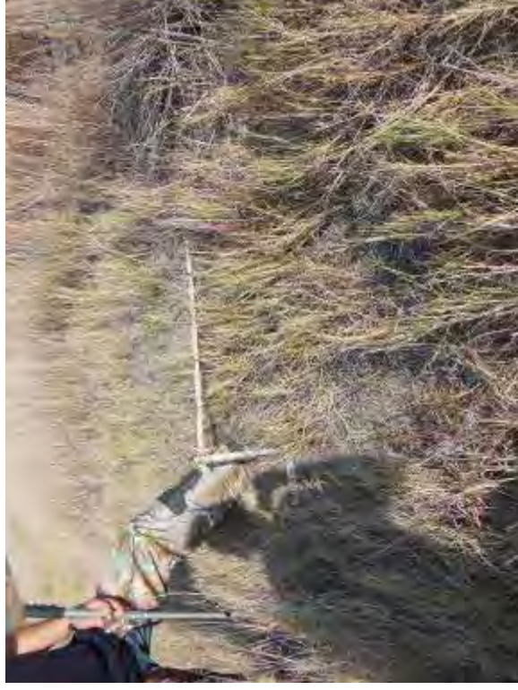
Photo 20: South embankment exterior slope approximately 2.5H:1V.
