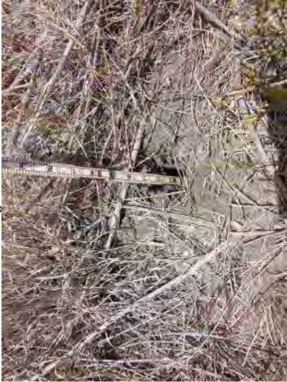
Photo 143: Approximately 3-foot-deep animal burrow at south embankment exterior slope.
