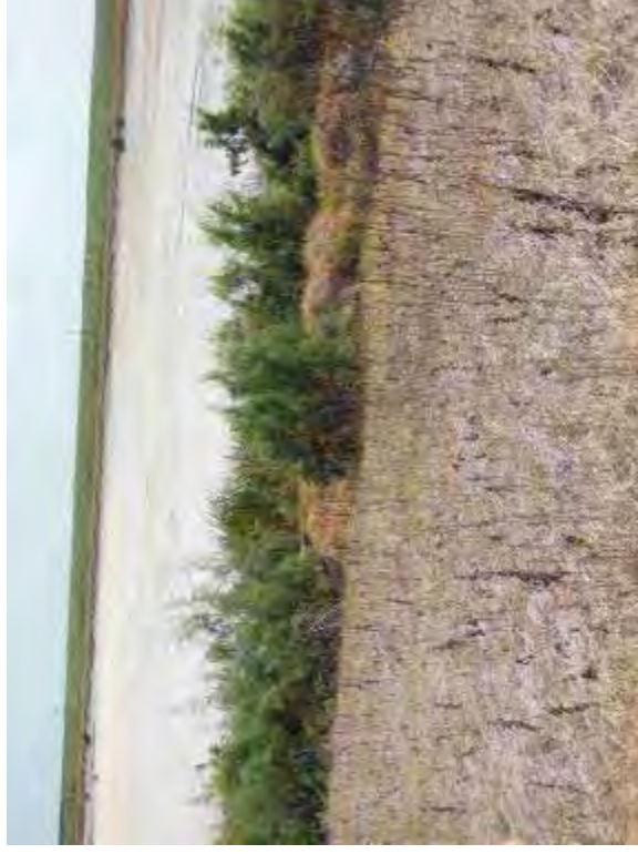
Photo 112: Mounded earth at west embankment interior slope, looking east. Note vegetation on slope.
