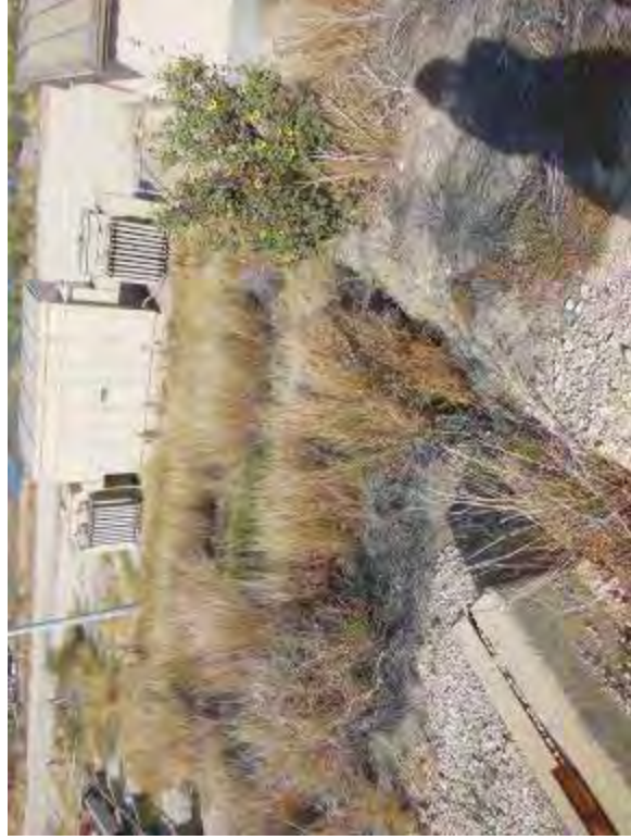
Photo 61: Erosion rill at west embankment exterior slope, looking west.
