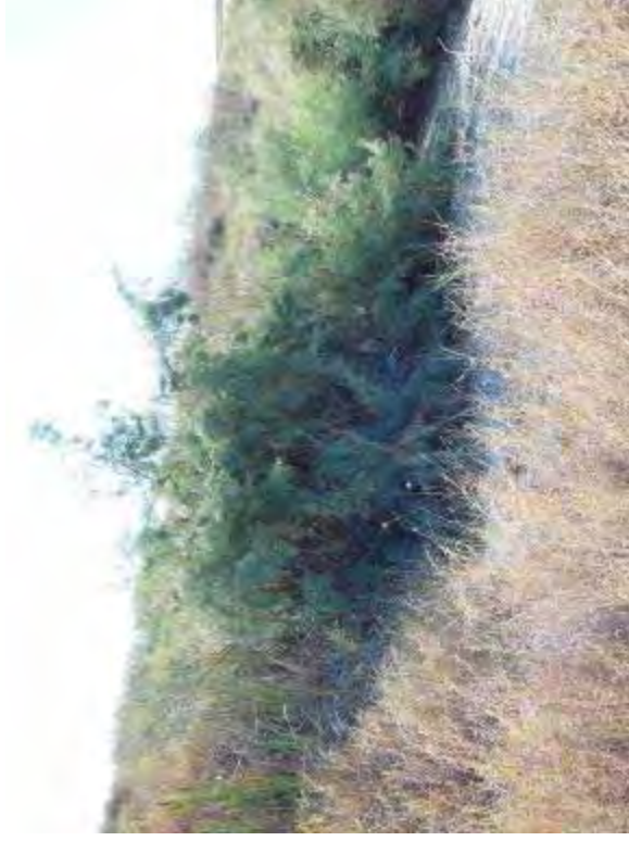
Photo 58: Cattails and vegetation growing near wet area at west embankment exterior slope.
