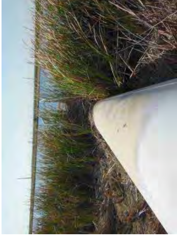
Photo 50: 24-inch-diameter steel outlet pipe at west embankment interior slope.
