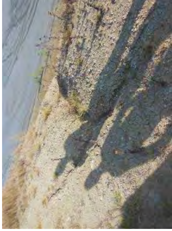
Photo 25: Erosion rills at south embankment interior slope.
