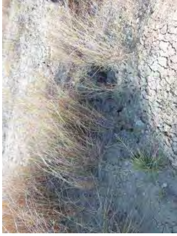
Photo 26: Erosion rills at south embankment interior slope.
