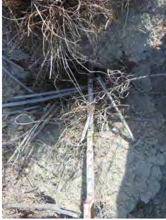
Photo 17: Approximately 12-inch-deep animal burrow hole at west embankment exterior slope.
