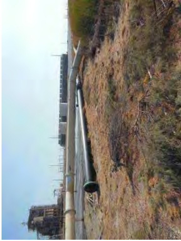
Photo 49: 24-inch-diameter steel outlet pipe at west embankment interior slope. PVC pipe along center embankment.
