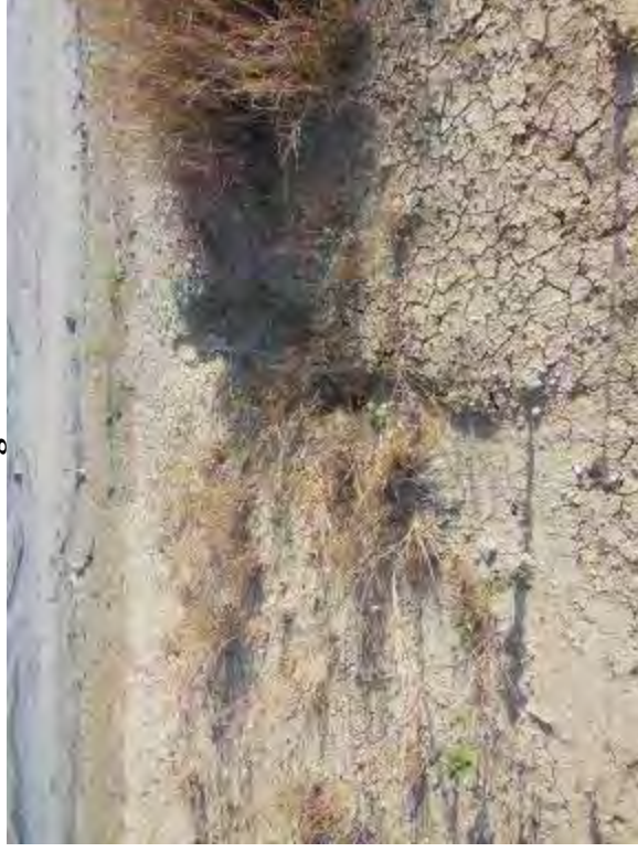
Photo 24: Erosion rills at south embankment interior slope.
