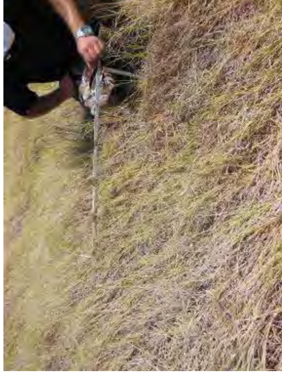
Photo 98: West embankment interior slope approximately 3.5H:1V.
