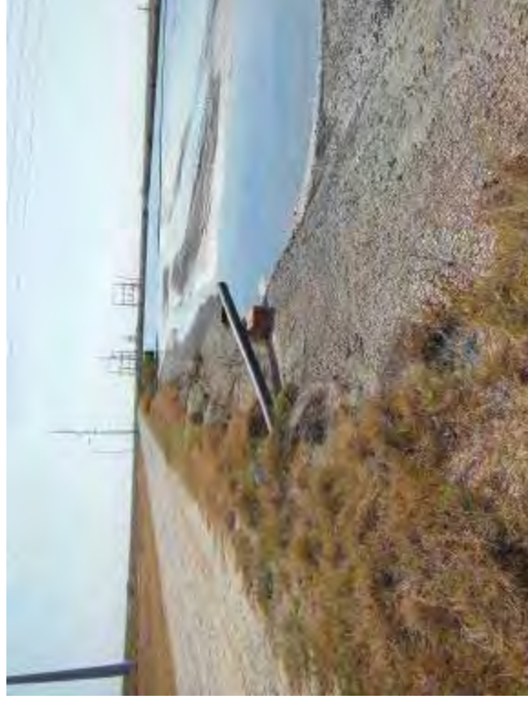
Photo 74: 6-inch-diameter inlet pipe from waste treatment sump at north embankment interior slope.
