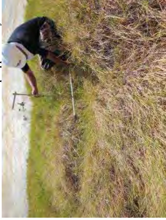
Photo 98: West embankment interior slope approximately 3.5H:1V.
