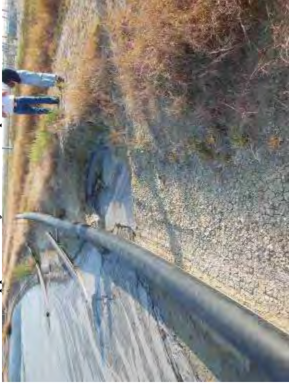
Photo 13: East embankment crest tension or desiccation cracks approximately 15 inches deep.
