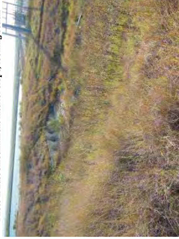
Photo 4: East embankment exterior slope, looking northeast. Note culvert at northeast corner toe.
