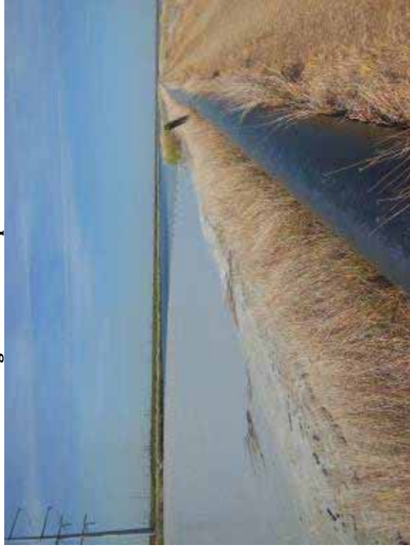
Photo 81: Center embankment north slope, looking west. Note vegetation on slope.
