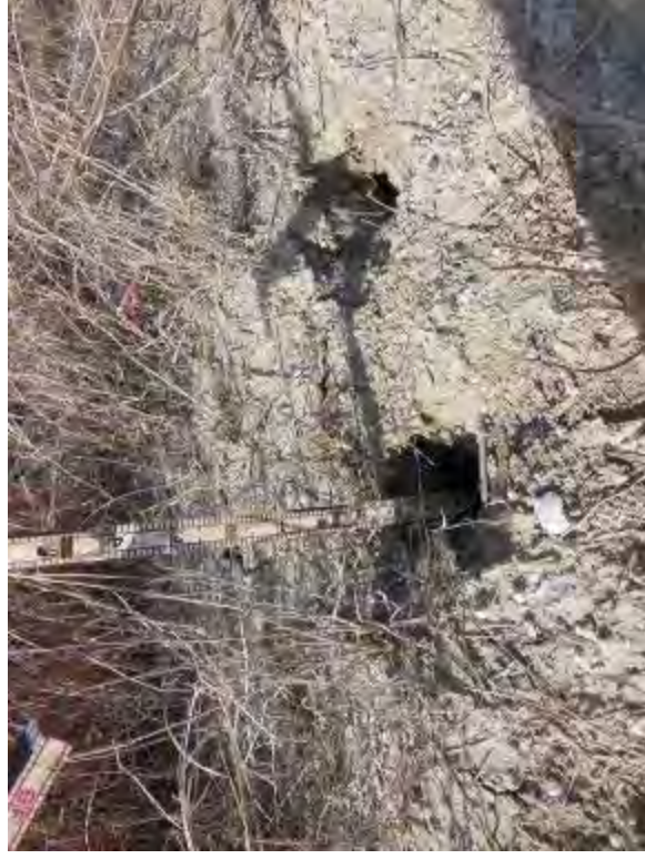
Photo 42: Approximately 6-inch-deep animal burrows on crest near south west corner.
