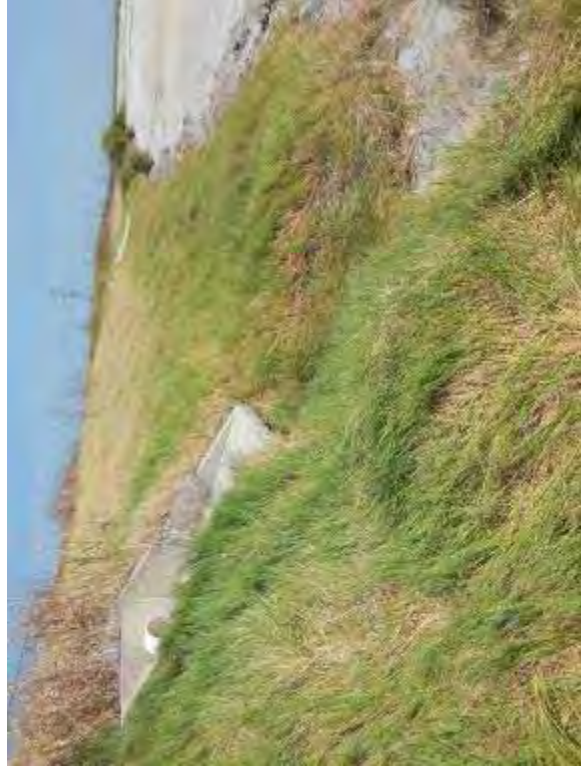
Photo 101: 12-inch-diameter substation stormwater drain inlet at west embankment interior slope.
