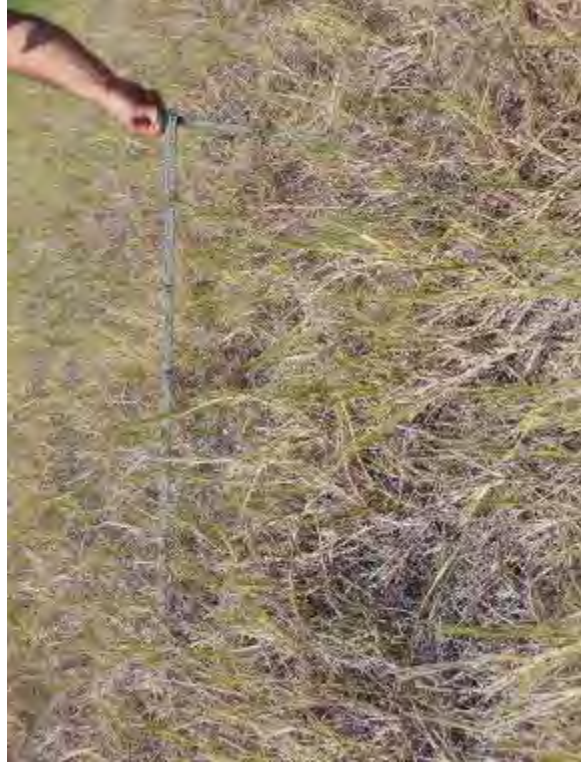
Photo 126: North embankment exterior slope approximately 3H:1V.
