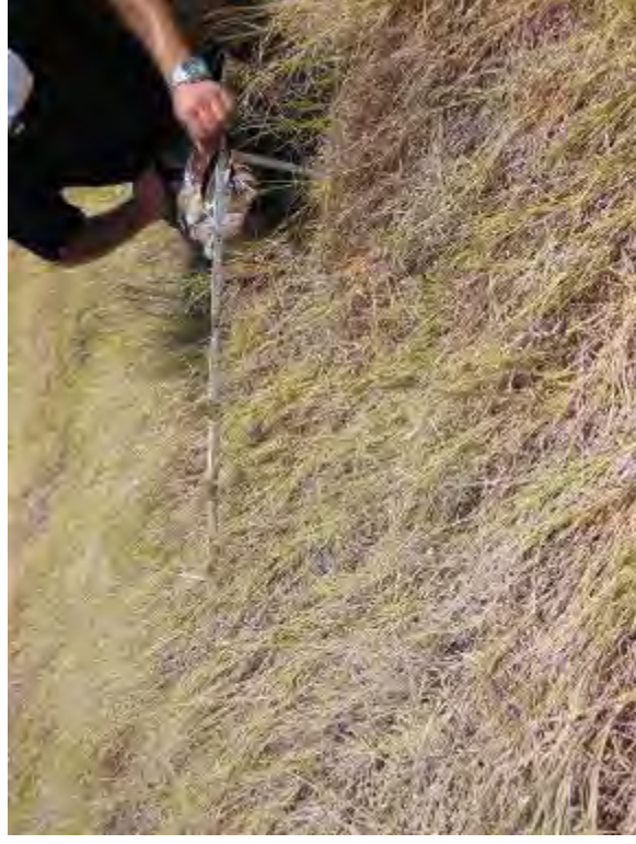
Photo 98: West embankment interior slope approximately 3.5H:1V.
