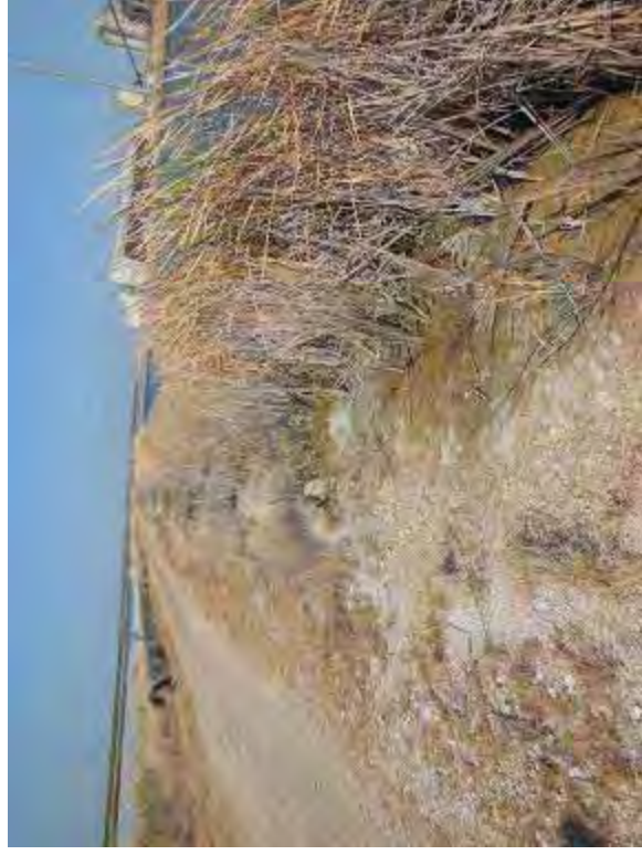
Photo 81: Center embankment north slope, looking west. Note vegetation on slope.
