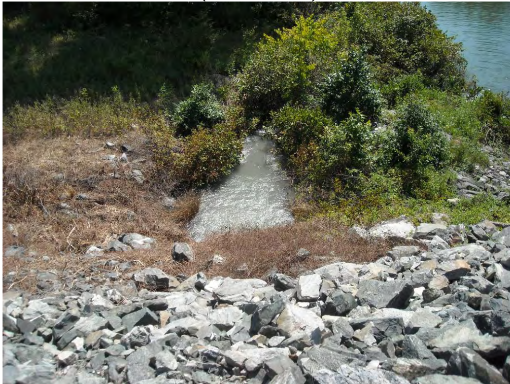
PHOTO 21: DIKE 1 DOWNSTREAM EMBANKMENT AND DISCHARGE (FILTER DIKE)
