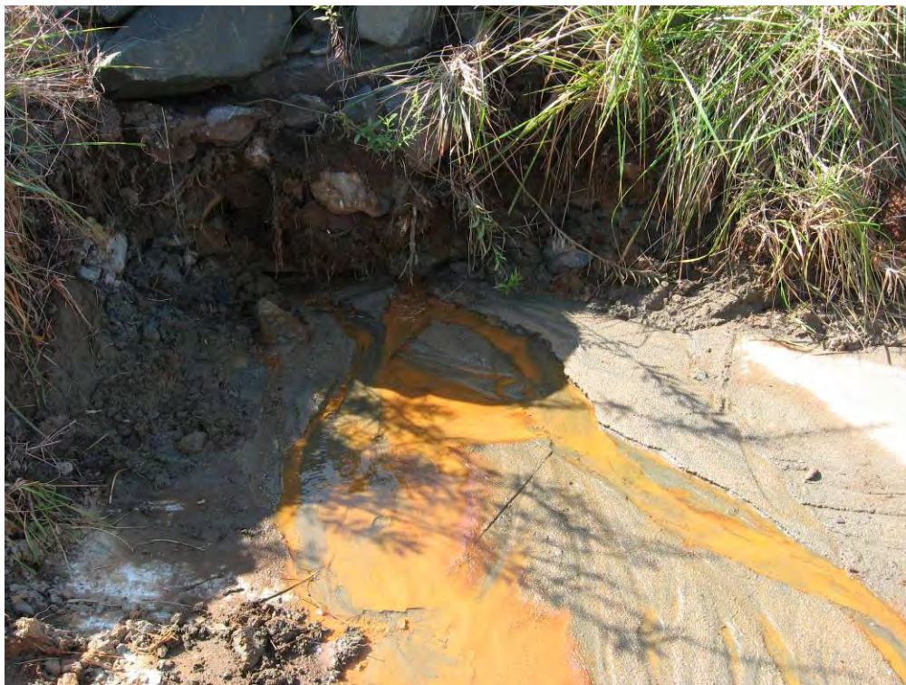
PHOTO 3: CHIMNEY DRAIN AT TOE OF WEST ASH POND DAM
