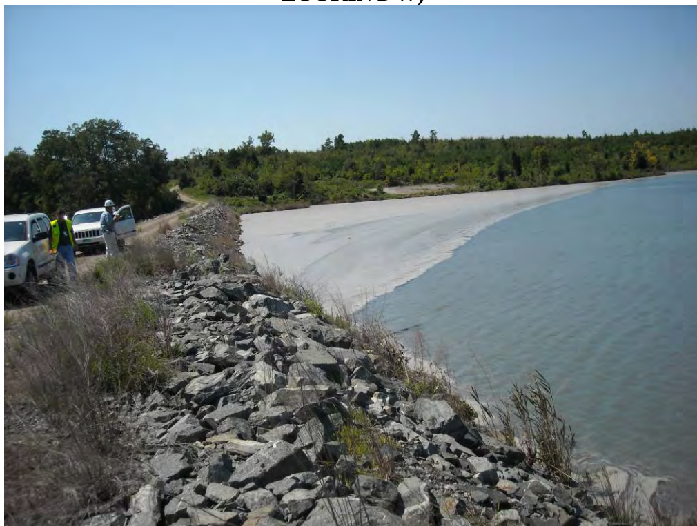
PHOTO 20: UPSTREAM EMBANKMENT OF DIKE 1 (FILTER DIKE, LOOKING W)
