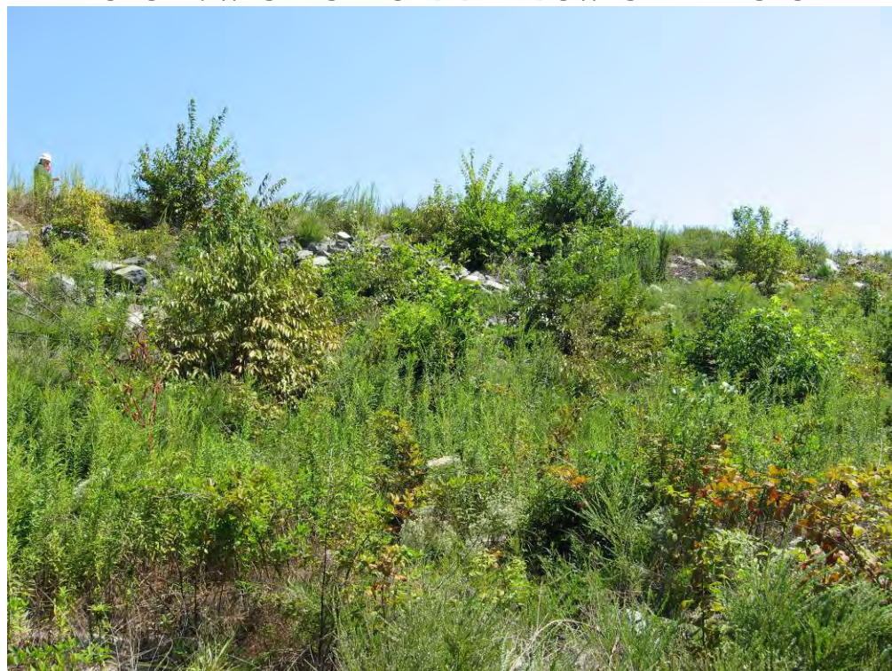
PHOTO 24: WEST ASH POND DAM DOWNSTREAM SLOPE
