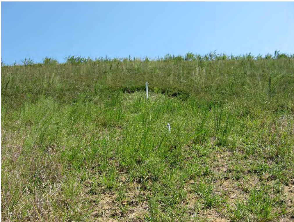
PHOTO 13: DOWNSTREAM EMBANKMENT OF FGD SETTLING POND
