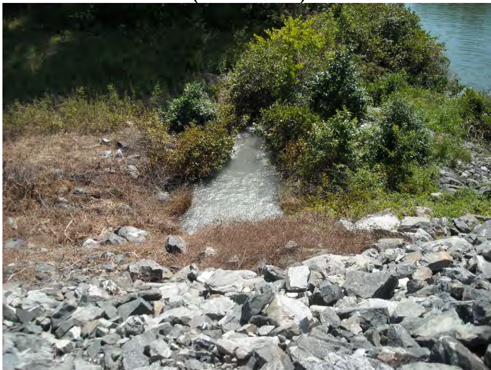
PHOTO 21: DIKE 1 DOWNSTREAM EMBANKMENT AND DISCHARGE (FILTER DIKE)
