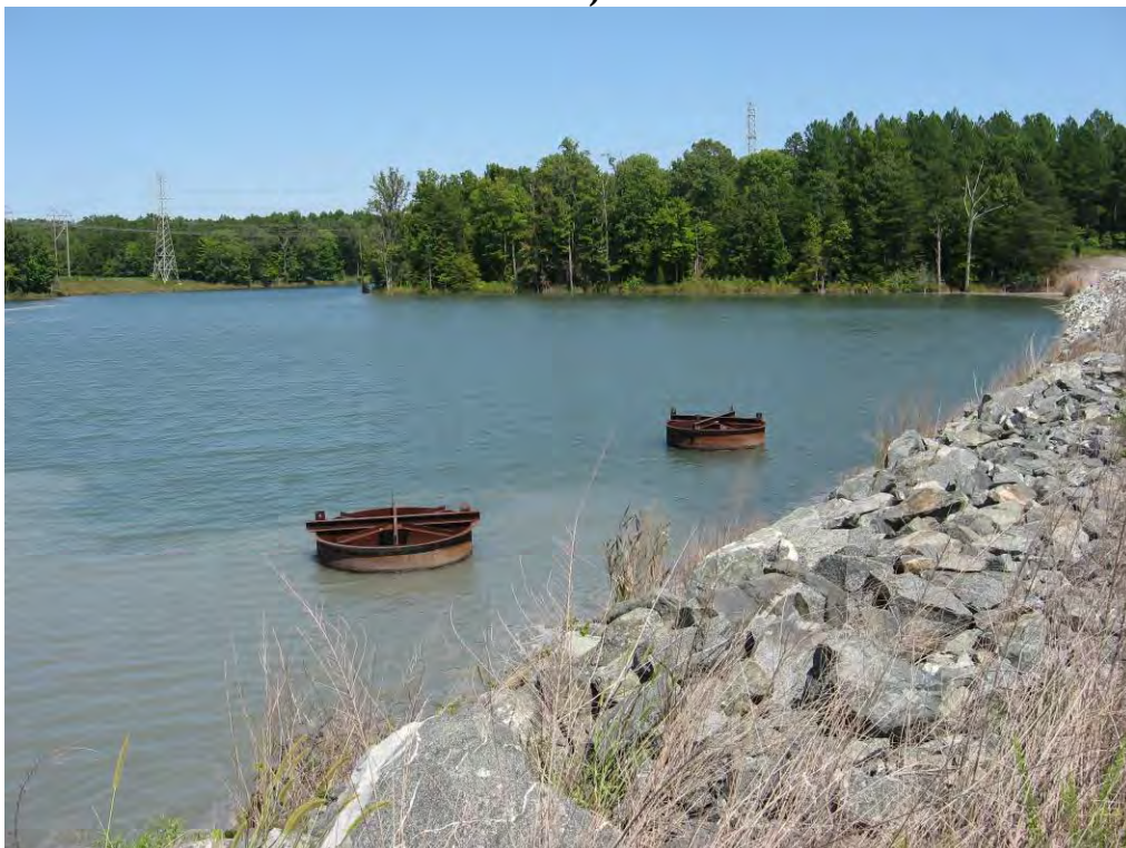
PHOTO 18: DISCHARGE RISER PIPES AT DIKE 1 (FILTER DIKE, LOOKING NE)
