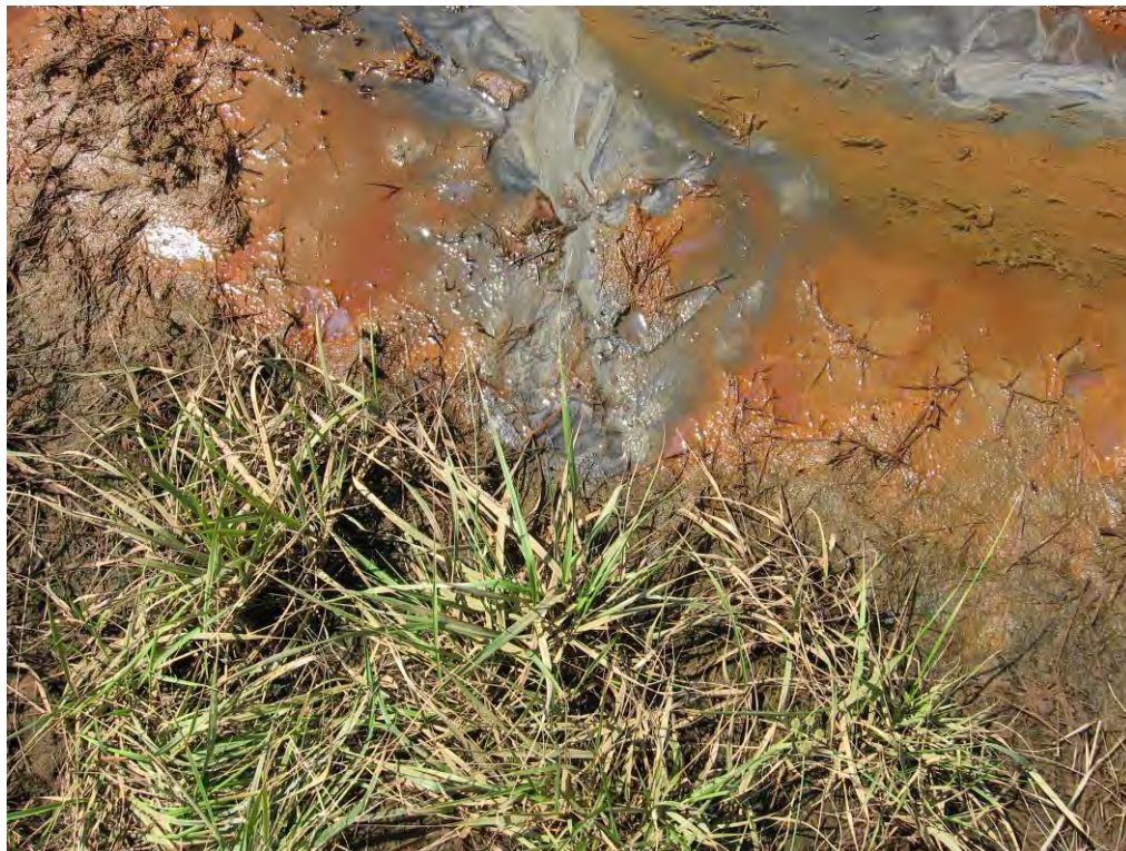
PHOTO 14: TOE OF FGD SETTLING POND
