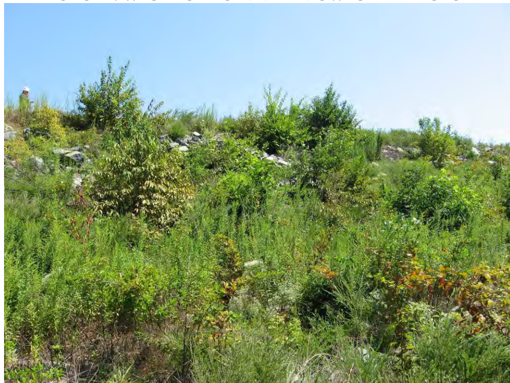
PHOTO 24: WEST ASH POND DAM DOWNSTREAM SLOPE
