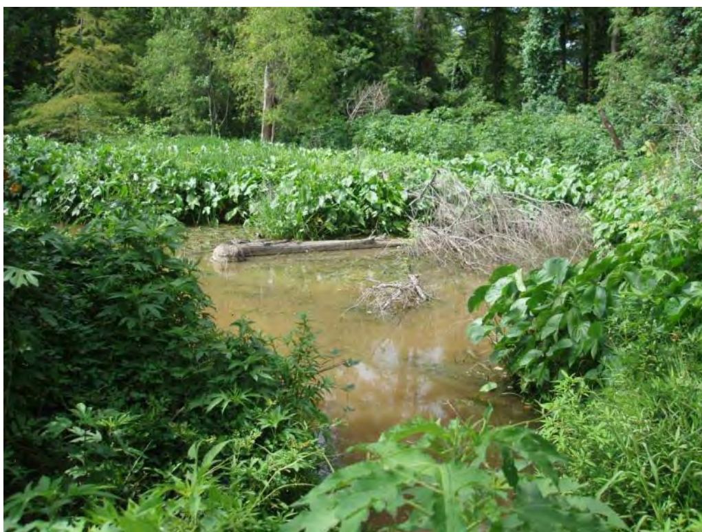
Photo No. 28: Bottom Ash Pond – North embankment exterior toe, looking north. Standing water near toe. Note beaver activity on downed tree.
