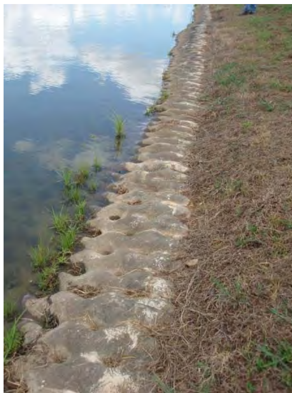
Photo No. 4: Bottom Ash Pond - East embankment interior slope, looking at typical concrete armor.
