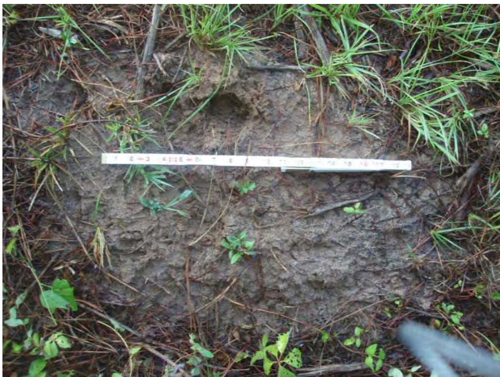
Photo No. 37: Bottom Ash Pond – North embankment exterior slope. Looking at 2'x1.5' area of damp, bare soil excavated from animal rooting/burrowing.
