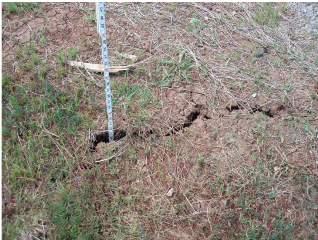
Photo No. 113: Fly Ash Pond – South embankment exterior slope. Looking at cracks in soil (approximately 2 inches wide and 21 inches deep).
