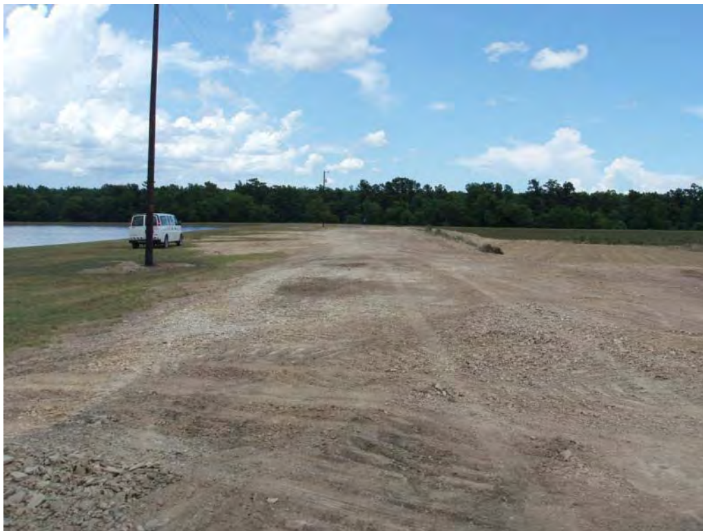
Photo No. 3: Fly Ash Pond - West embankment interior slope, looking northeast. Fill material covering slope.
