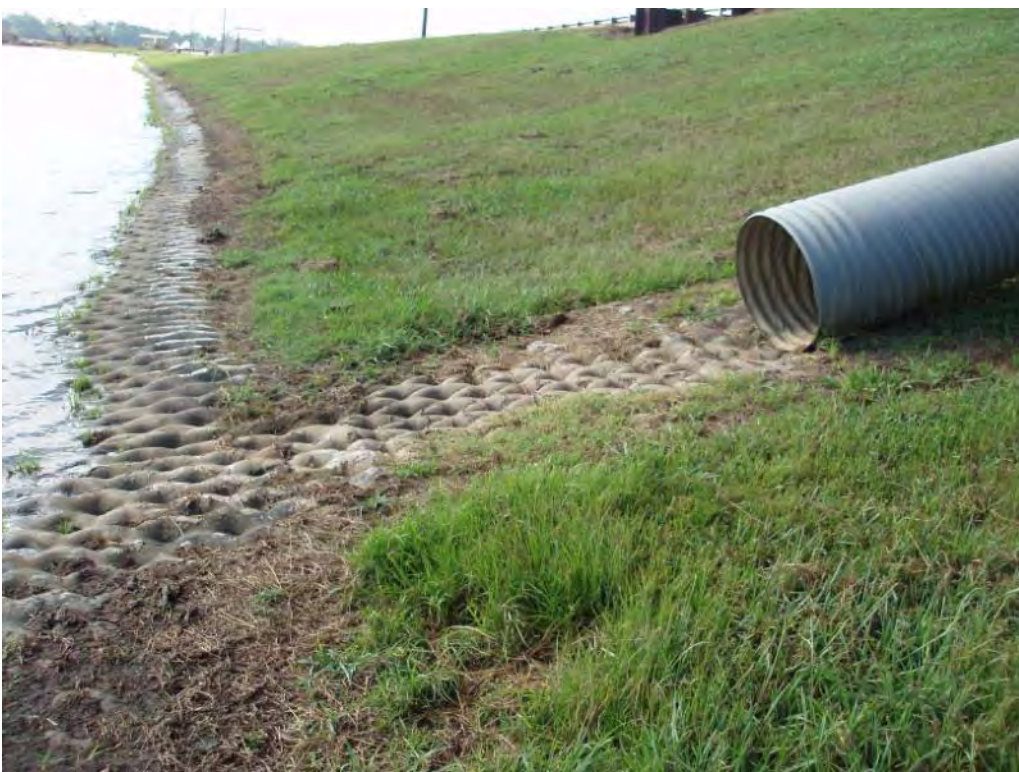
Photo No. 58: Bottom Ash Pond – South embankment interior slope, looking southeast. Looking at concrete armor on pond slope and at pipe discharge.
