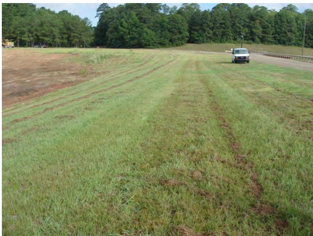
Photo No. 66: Bottom Ash Pond - South embankment exterior slope, looking northwest. Note exterior slope has been backfilled up to crest elevation.
