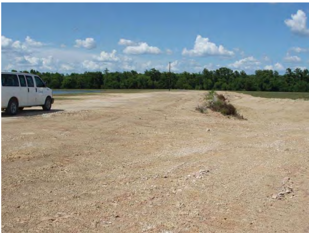
Photo No. 128: Fly Ash Pond - Near southwest corner of pond. Note ash material has been placed up to the crest elevation.
