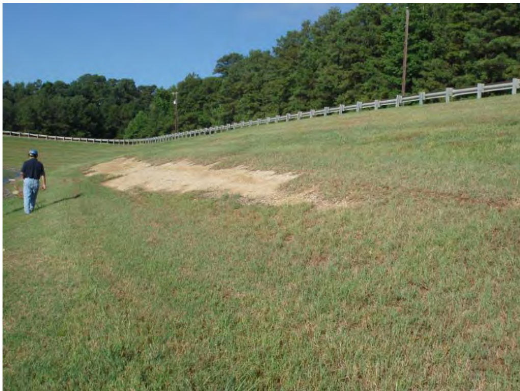
Photo No. 51: Bottom Ash Pond - West embankment interior slope, looking southwest. Looking at patch of bare soils.
