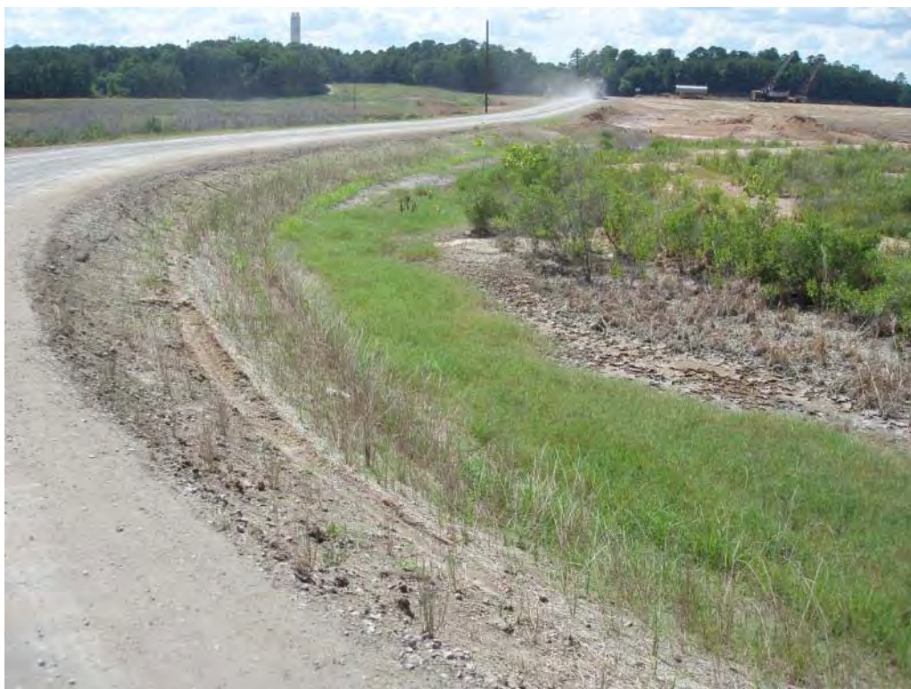
Photo No. 122: Fly Ash Pond - South embankment interior slope, looking northwest. Note ash material placed on slope.
