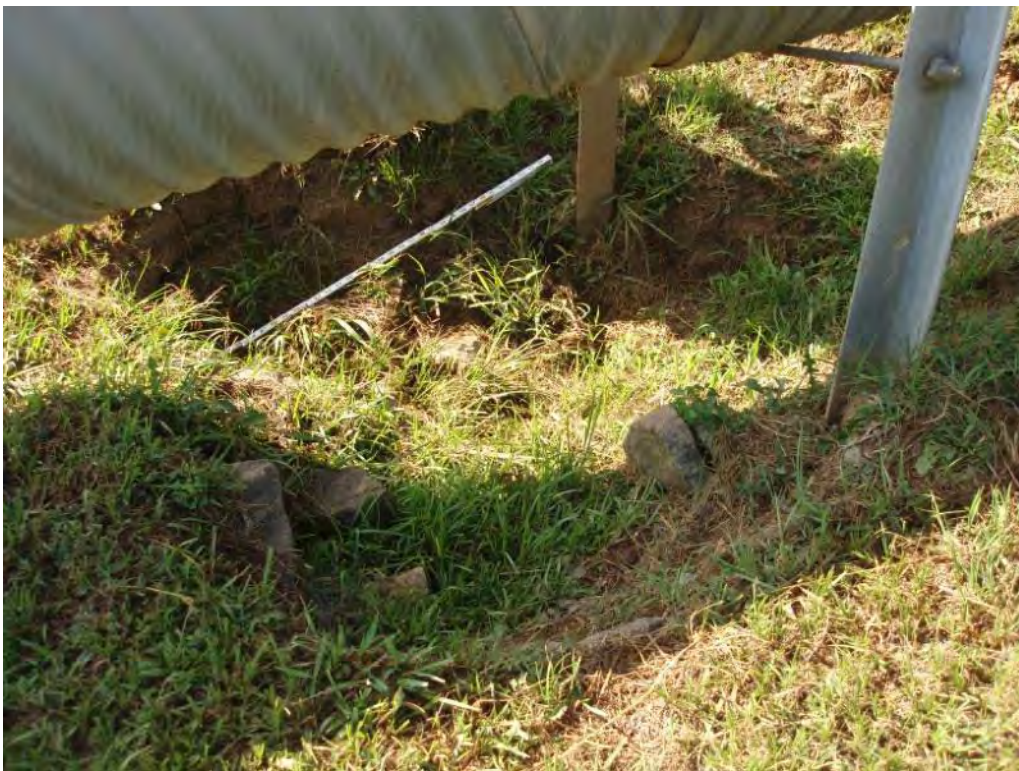
Photo No. 57: Bottom Ash Pond – South embankment interior slope. Looking at depression (approximately 3 feet wide and 2 feet deep) beneath pipe supports.
