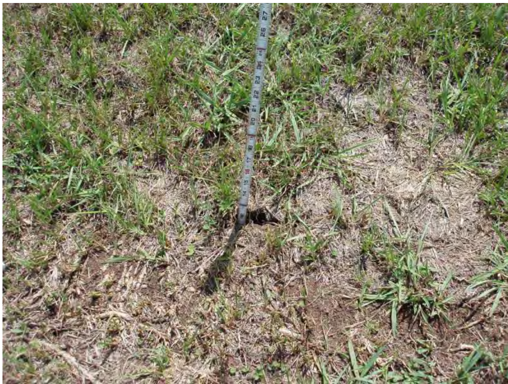
Photo No. 101: Fly Ash Pond - East embankment interior slope. Looking at crack in soils (approximately 2 inches wide and 11 inches deep).
