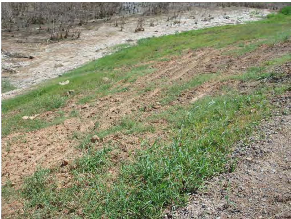
Photo No. 121: Fly Ash Pond - South embankment exterior slope, looking southwest. Note ruts and missing vegetation.
