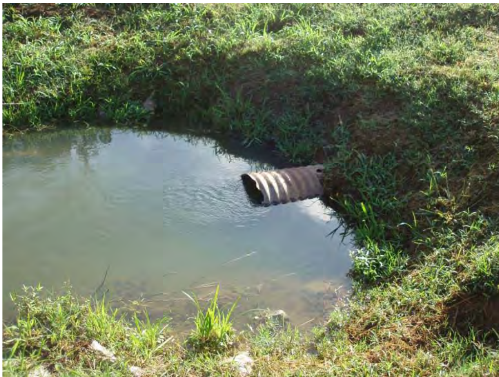
Photo No. 47: Discharge channel located at west embankment exterior toe. Water discharged into channel from Bottom Ash Pond.
