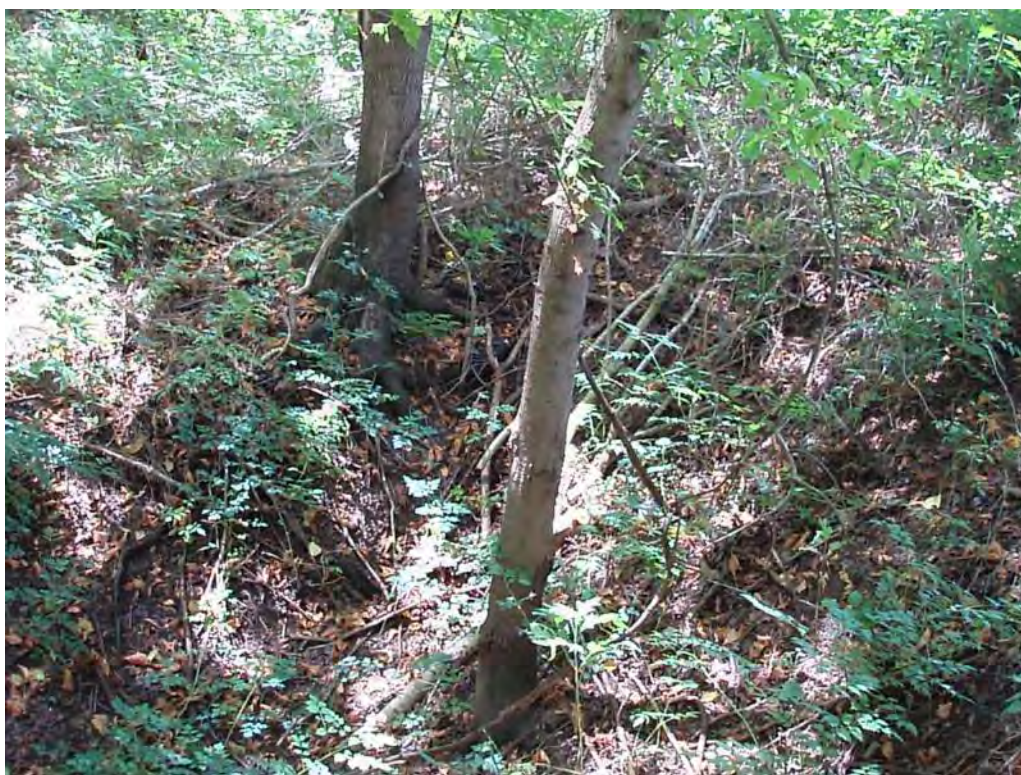
Photo No. 88: Fly Ash Pond - North embankment exterior slope. Looking at area of surface erosion located outside the slope toe.
