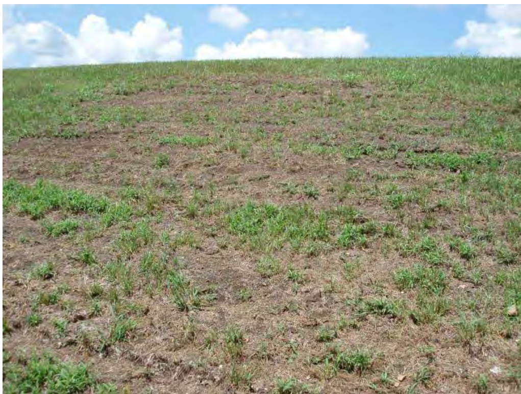
Photo No. 98: Fly Ash Pond – North embankment exterior slope. Looking at minor rutting and loss of grass cover.
