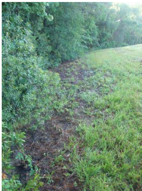
Photo No. 36: Bottom Ash Pond - North embankment exterior slope, looking southeast. Note change in vegetation near toe.
