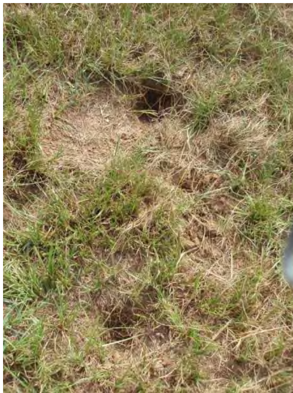
Photo No. 23: Bottom Ash Pond - North embankment exterior slope. Looking at two areas of animal burrowing/rooting.
