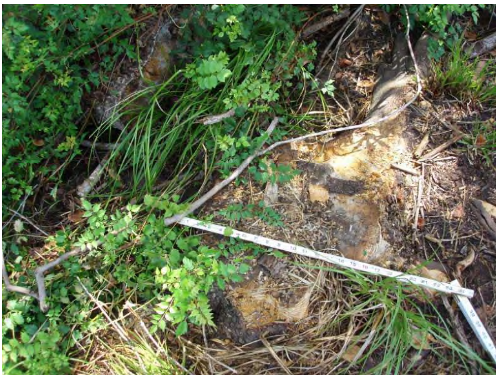
Photo No. 80: Fly Ash Pond - North embankment exterior slope. Tree stump (approximately 18 inches in diameter).
