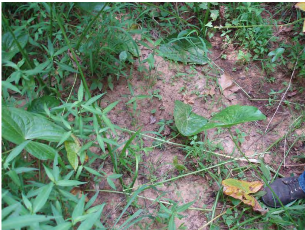
Photo No. 33: Bottom Ash Pond – North of north embankment toe, looking at damp area of soil approximately 4'x3'.
