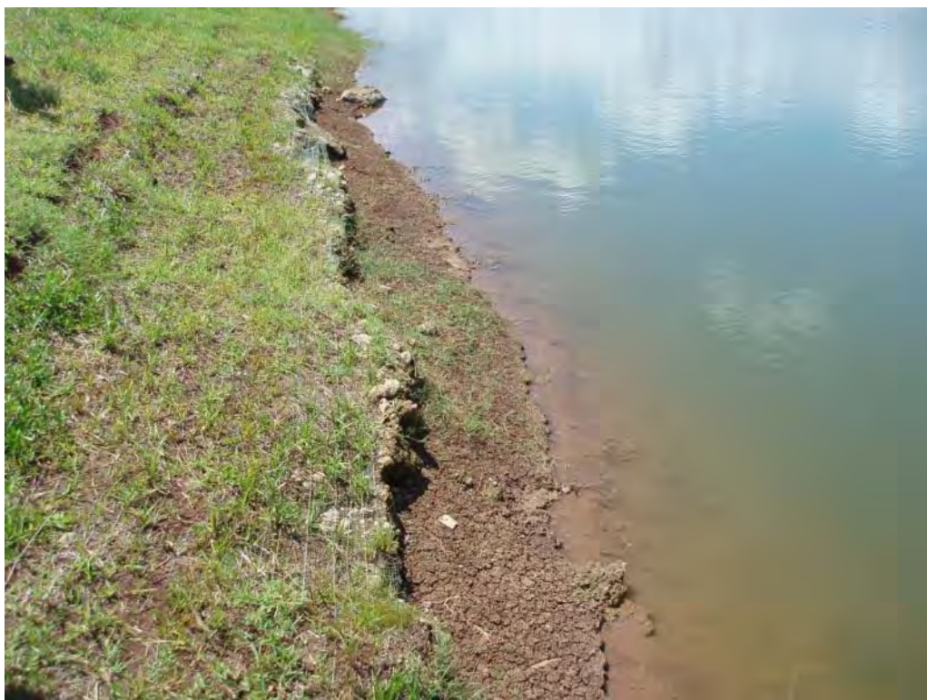
Photo No. 111: Fly Ash Pond - South embankment interior slope. Looking at erosion near water line. Note TRM on slope where recently re-seeded.
