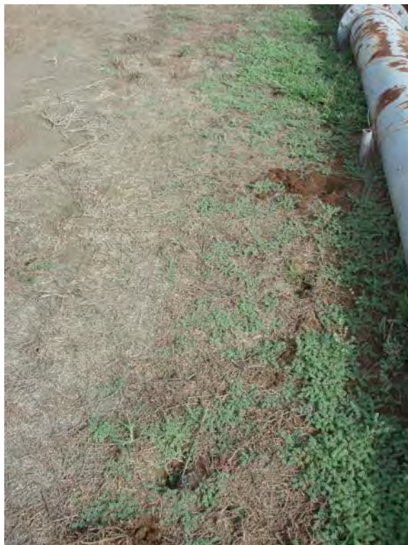
Photo No. 65: Bottom Ash Pond - South embankment interior slope. Looking at surface erosion near sluice lines.
