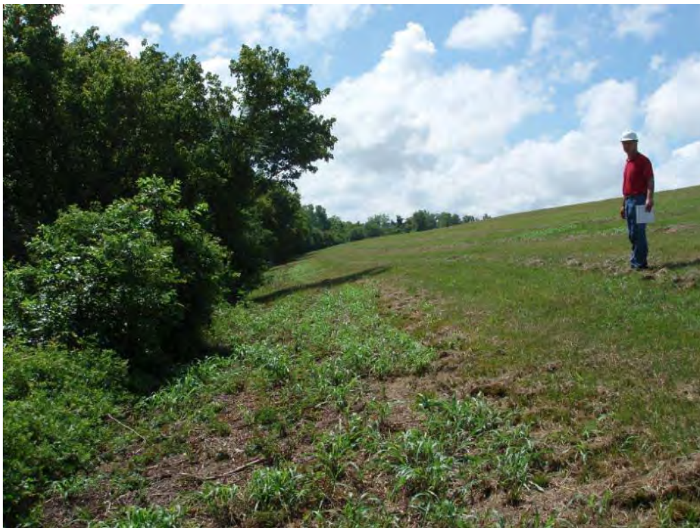
Photo No. 79: Fly Ash Pond - North embankment exterior slope, looking southeast. Note vegetation growing on bottom third of slope.
