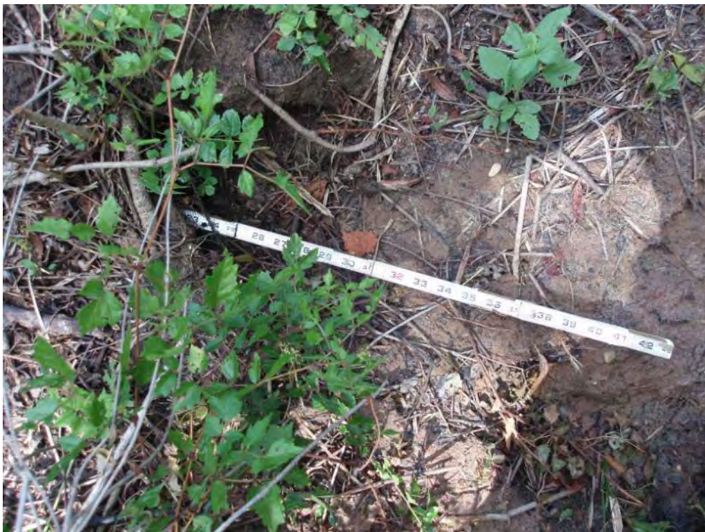
Photo No. 75: Fly Ash Pond – North embankment exterior slope. Rodent burrow (approximately 4 inches in diameter and 24 inches deep).
