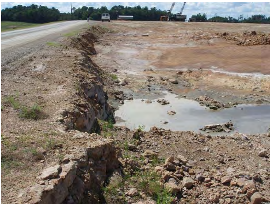
Photo No. 124: Fly Ash Pond - South embankment interior slope, looking northwest. Note slope has been excavated into during removal of ash material.
