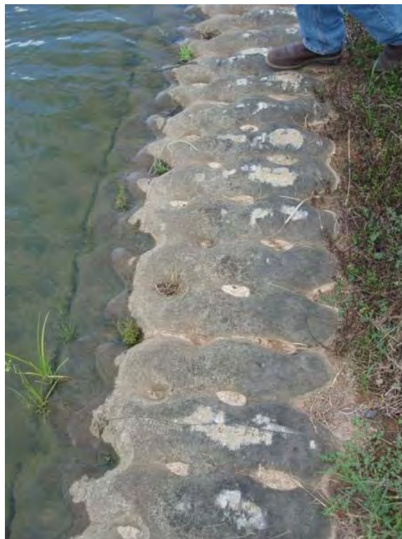
Photo No. 7: Bottom Ash Pond - East embankment interior slope, concrete armor.
