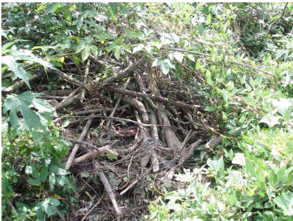
Photo No. 27: Bottom Ash Pond – North embankment exterior toe, looking southwest. Possible beaver dam activity.
