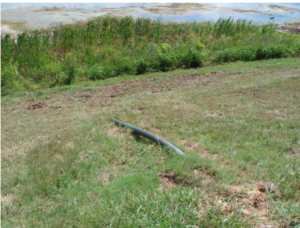
Photo No. 126: Fly Ash Pond – South embankment exterior slope, looking south. Unknown pipe discharging into ash storage area.
