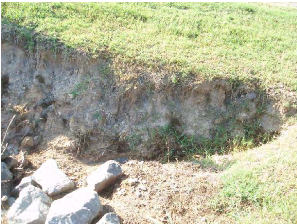
Photo No. 49: Bottom Ash Pond - West embankment exterior slope. Looking at erosion around edges of riprap.
