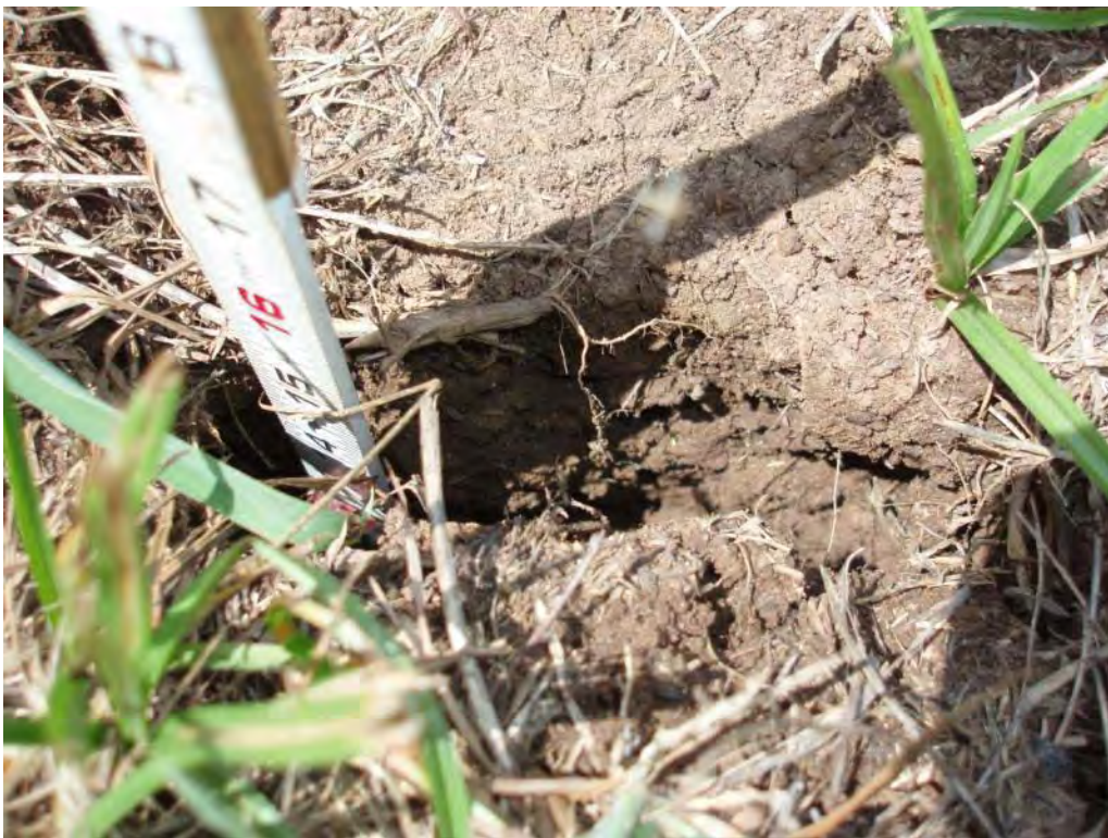
Photo No. 91: Fly Ash Pond – North embankment interior slope. Looking at crack in soils (approximately 2 inches wide and 15 inches deep).
