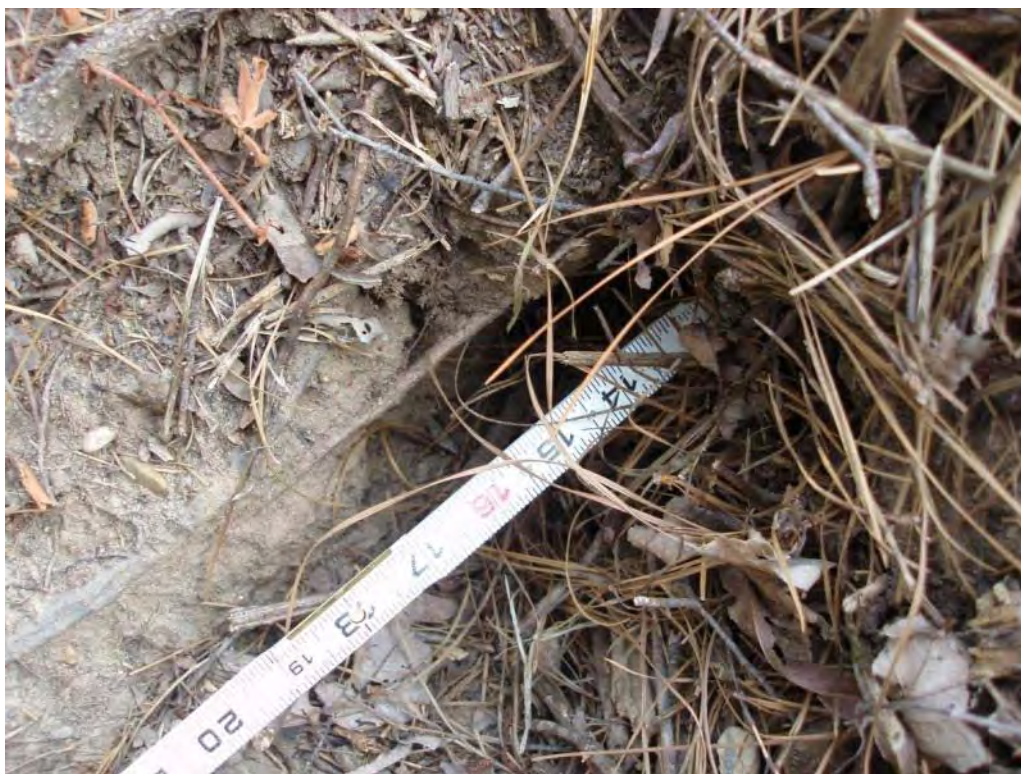
Photo No. 34: Bottom Ash Pond – North embankment exterior slope. 2-inch-diameter, 16-inch-deep rodent burrow.
