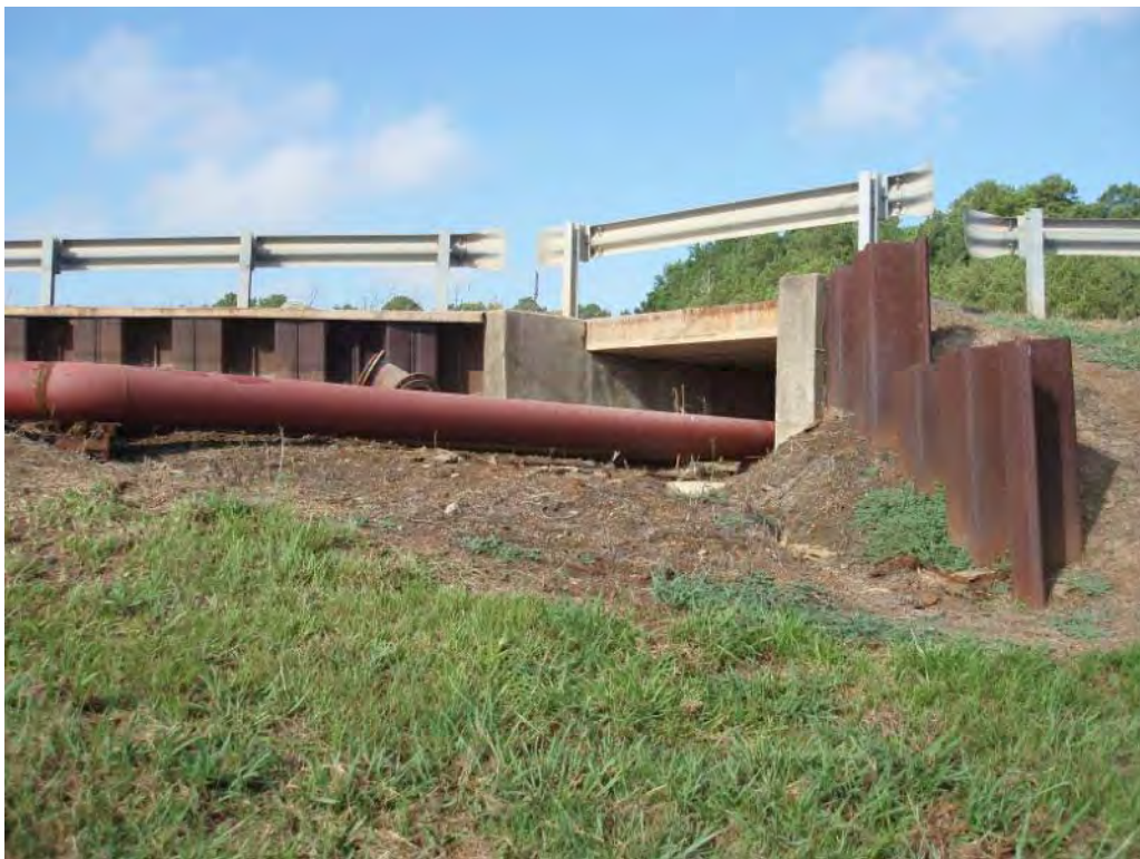
Photo No. 59: Bottom Ash Pond - South embankment interior slope, looking southwest. Looking at surface erosion near sluice piping.
