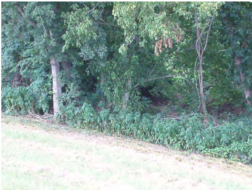
Photo No. 19: Bottom Ash Pond - North embankment exterior slope, looking north. Note vegetation growing on bottom of slope.
