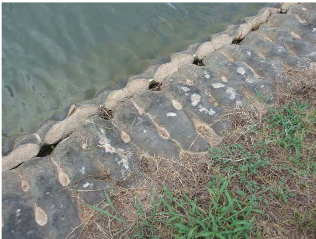
Photo No. 6: Bottom Ash Pond – East embankment interior slope, fracture of concrete armor.
