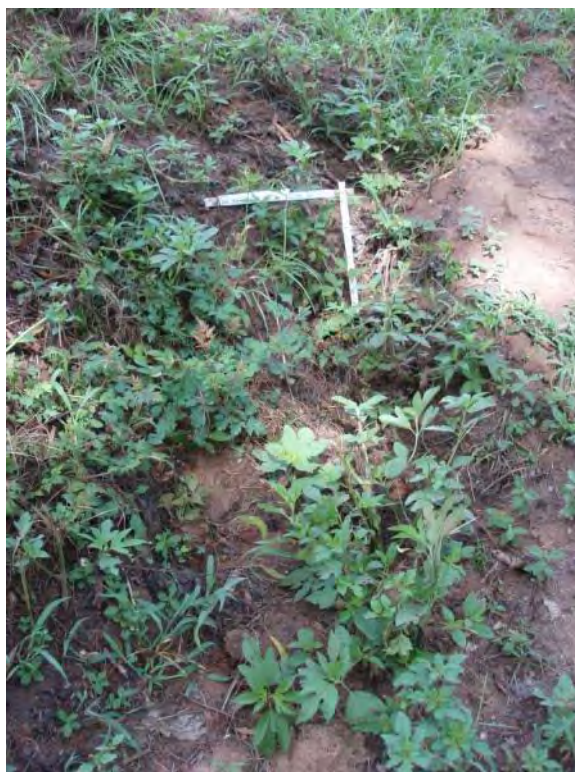
Photo No. 74: Fly Ash Pond – North embankment exterior slope. Looking at erosion rill.
