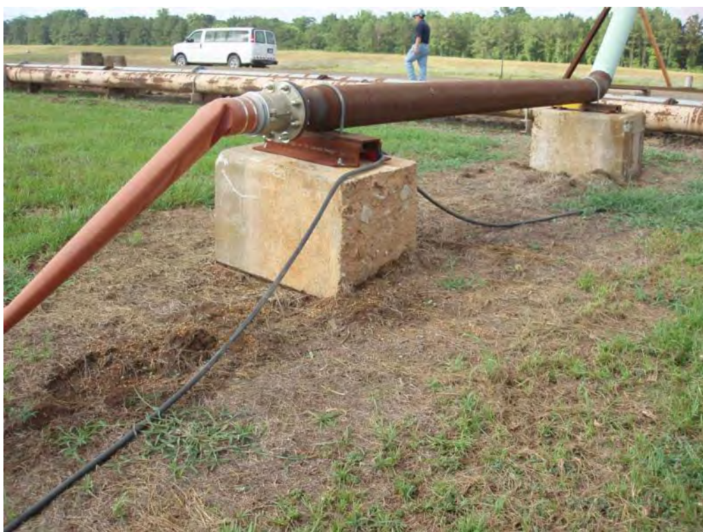
Photo No. 68: Bottom Ash Pond - South embankment interior slope, looking at minor surface erosion at piping for water truck filling.
