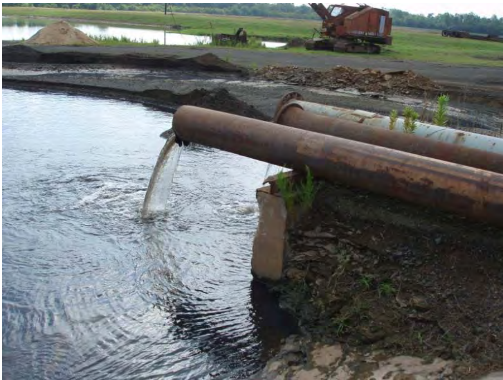
Photo No. 71: Bottom Ash Pond - Discharge sluice lines near southeast corner.
