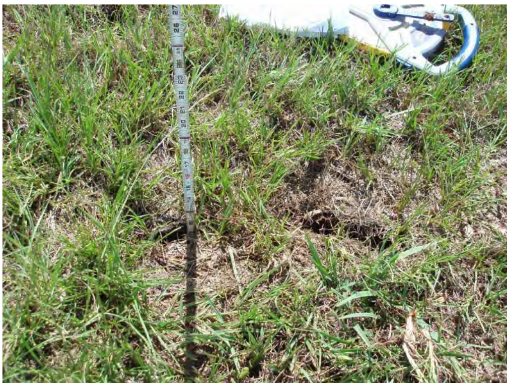
Photo No. 96: Fly Ash Pond - North embankment interior slope. Looking at crack in soils (approximately 2 inches wide and 12 inches deep).
