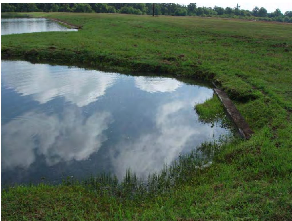
Photo No. 72: Bottom Ash Pond - East embankment interior slope, looking northeast. Note concrete armoring missing from the slope.
