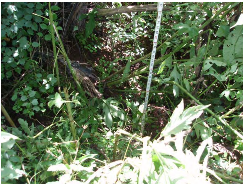
Photo No. 100: Fly Ash Pond - East embankment exterior slope, downed tree near toe created depression and erodible soils.
