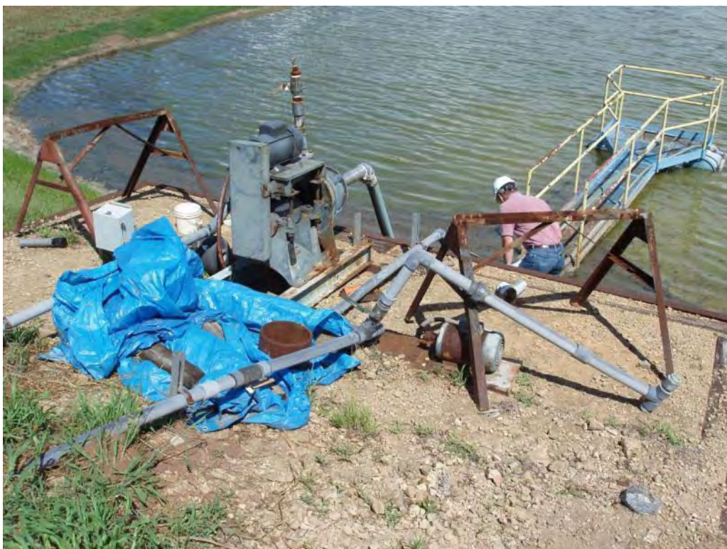
Photo No. 130: Fly Ash Pond - West embankment interior slope, looking east. Outlet pump and piping.
