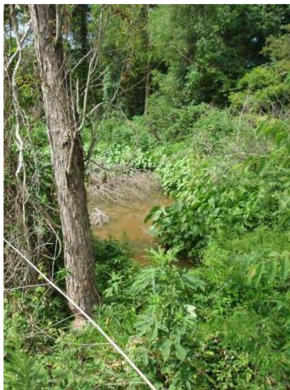
Photo No. 26: Bottom Ash Pond - North embankment exterior toe, looking north. Standing water at toe. Note beaver activity on tree in foreground.
