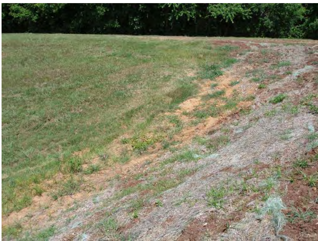
Photo No. 106: Fly Ash Pond - Southeast corner interior slope, looking southeast. Note surface erosion.
