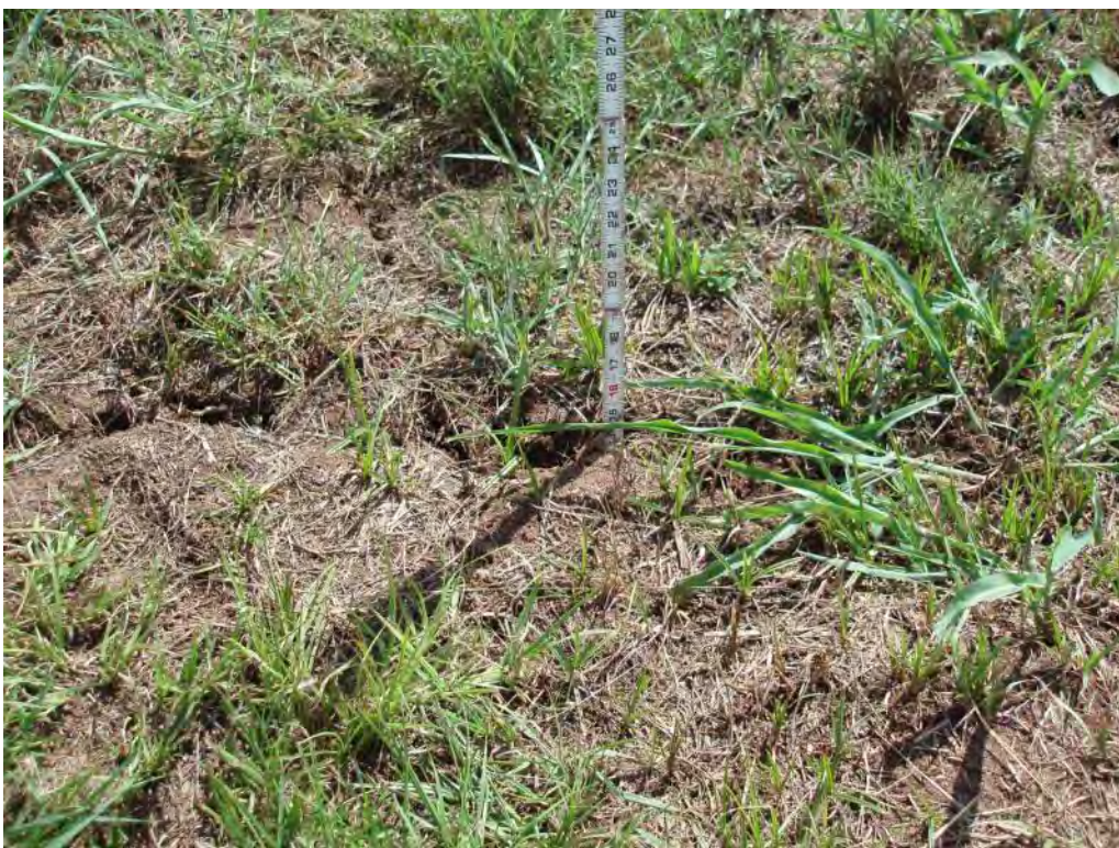
Photo No. 92: Fly Ash Pond – North embankment interior slope. Looking at crack in soils (also shown in Photo No. 91).
