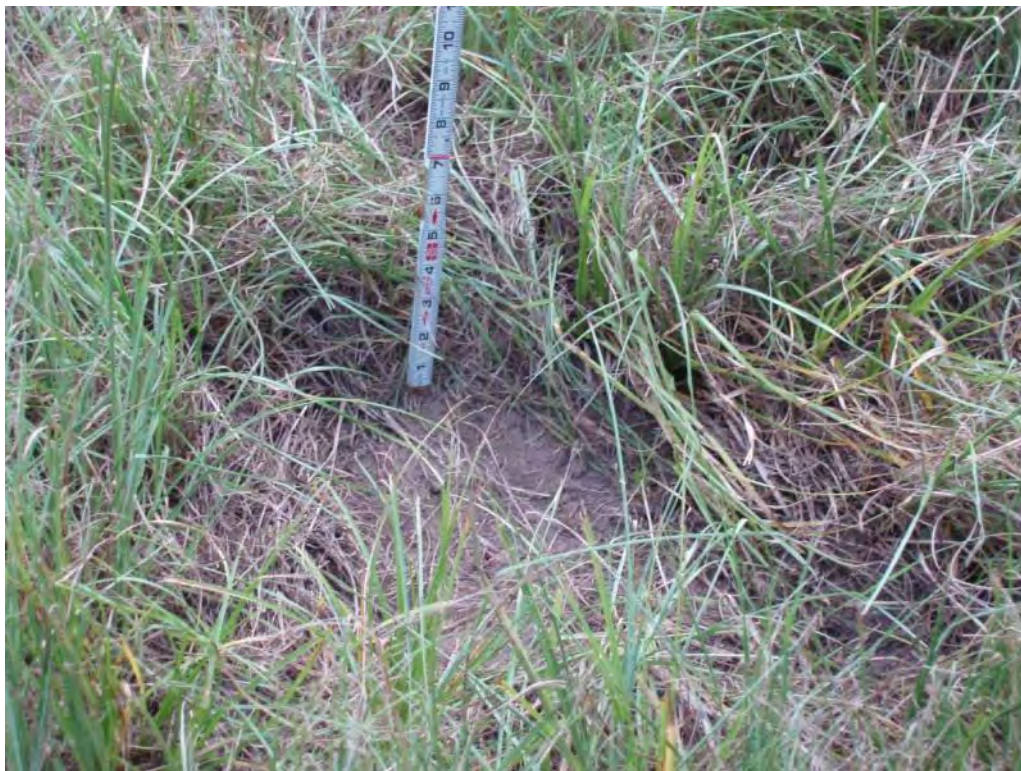
Photo No. 15: Bottom Ash Pond - North embankment exterior slope. 6"x6" area of bare soil.
