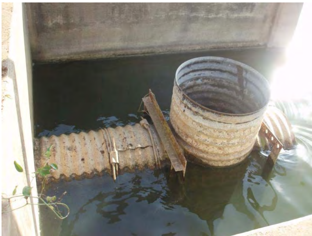
Photo No. 45: Bottom Ash Pond – 24-inch-diameter corrugated metal pipe outlet on west embankment. Outlet discharges to channel on exterior slope of west embankment.
