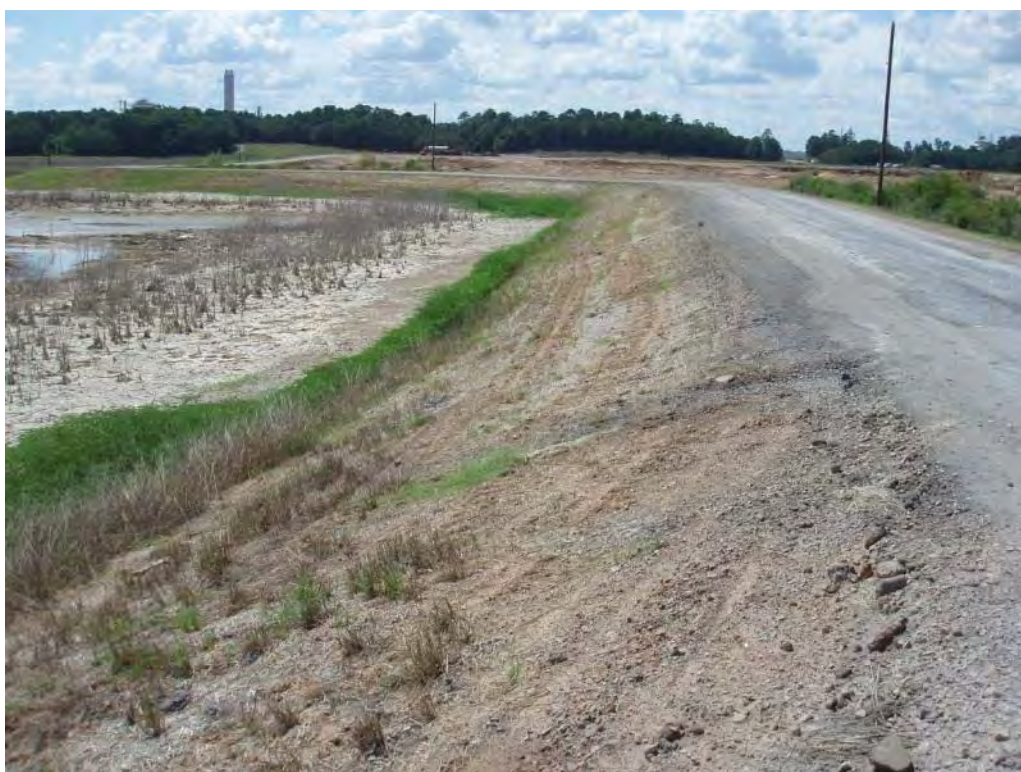
Photo No. 118: Fly Ash Pond - South embankment exterior slope, looking northwest. Note missing vegetation.
