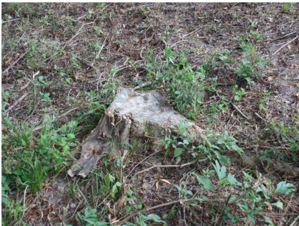
Photo No. 20: Bottom Ash Pond - North embankment exterior slope. Tree stump located on slope.
