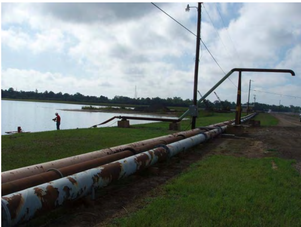
Photo No. 67: Bottom Ash Pond - South embankment interior slope, looking southeast. Sluice lines in foreground, piping to fill water trucks in background.
