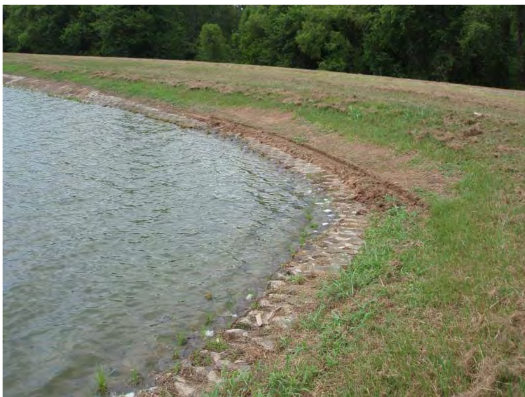
Photo No. 12: Bottom Ash Pond - Northeast corner interior slope. Note ruts and areas void of vegetation/protective cover.
