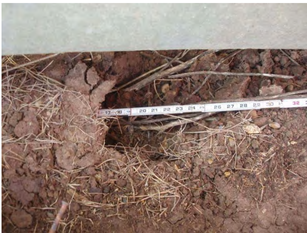
Photo No. 44: Bottom Ash Pond – Outlet structure, looking at erosion hole 24 inches deep on northwest side of outlet structure.
