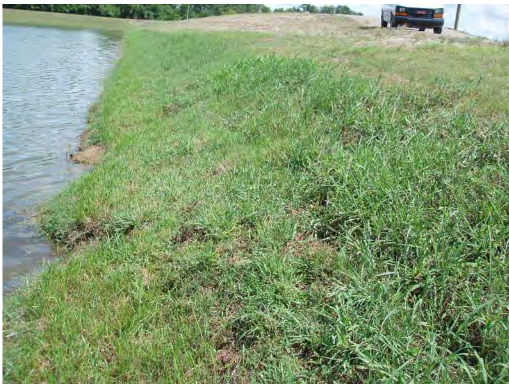
Photo No. 117: Fly Ash Pond - South embankment interior slope, looking southeast. Note erosion near water line.
