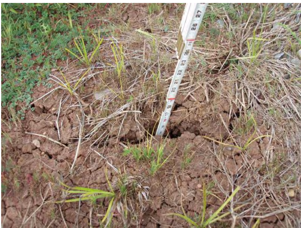
Photo No. 142: Leachate Pond - West embankment exterior slope. Note cracks in soil (approximately 2 inches wide and 14 inches deep).
