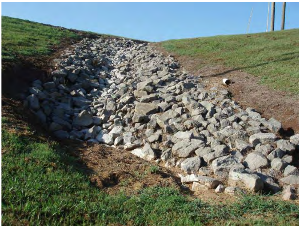
Photo No. 48: Bottom Ash Pond - West embankment exterior slope, looking at riprap protection and outlet pipes discharging into channel.
