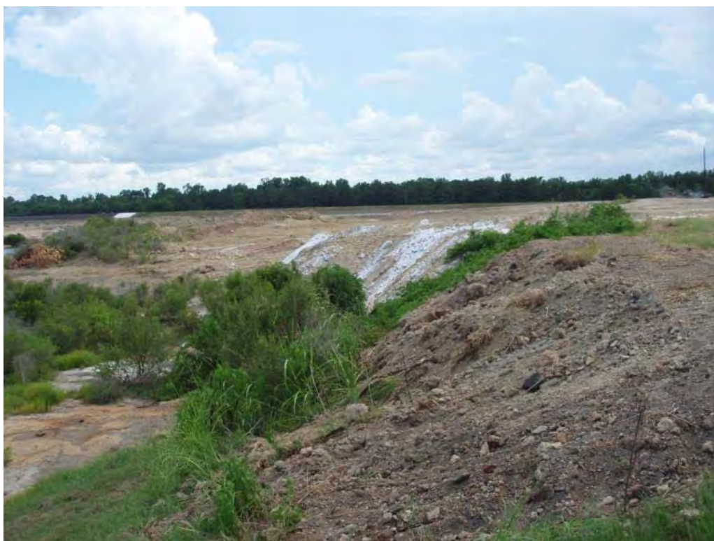
Photo No. 10: Fly Ash Pond - West embankment interior slope, looking southwest. Fill material covering slope.
