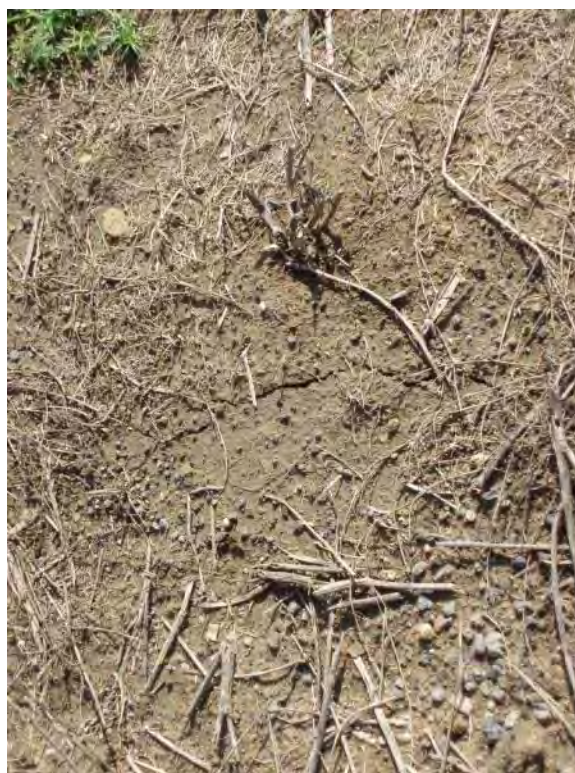
Photo No. 56: Bottom Ash Pond - South embankment interior slope. Looking at small crack (less than 1/2 inch wide).
