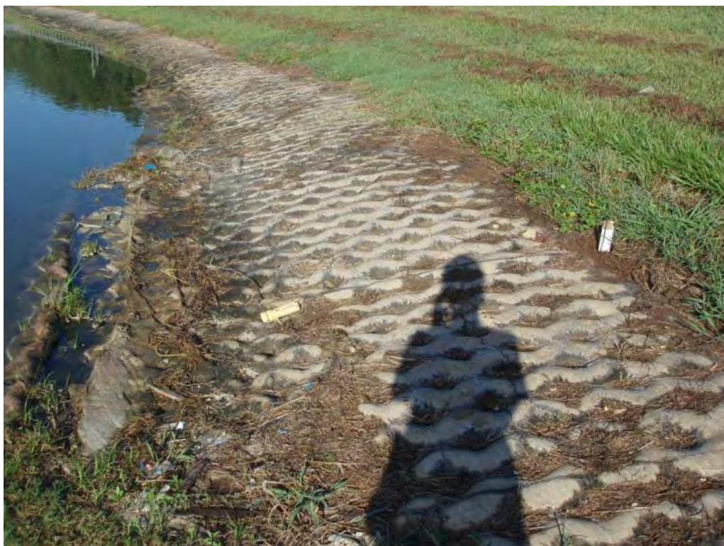
Photo No. 39: Bottom Ash Pond - West embankment interior slope. Typical concrete armor.
