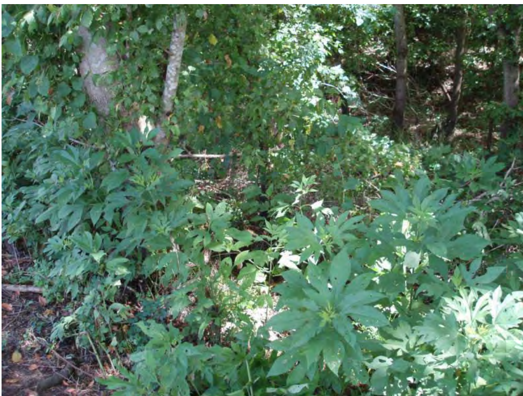
Photo No. 84: Fly Ash Pond – North embankment exterior slope. Looking at vegetation on bottom third of slope.
