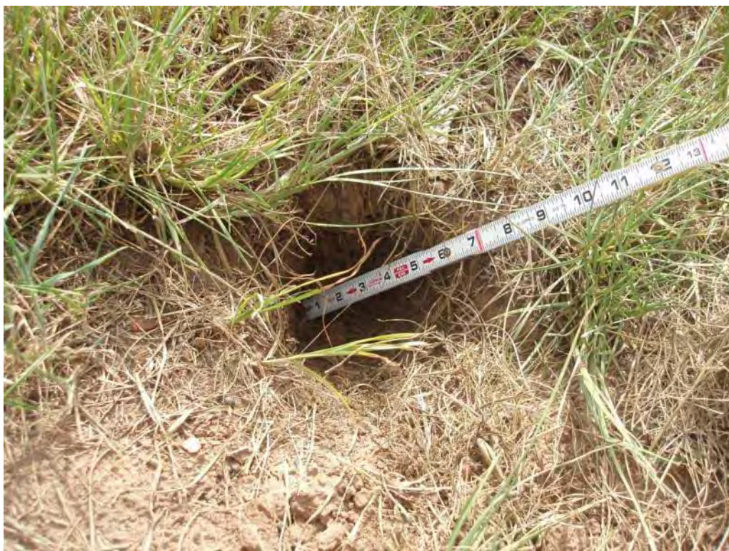
Photo No. 24: Bottom Ash Pond - North embankment exterior slope. Looking at 3-inch-diameter, 6-inch-deep animal burrow hole.
