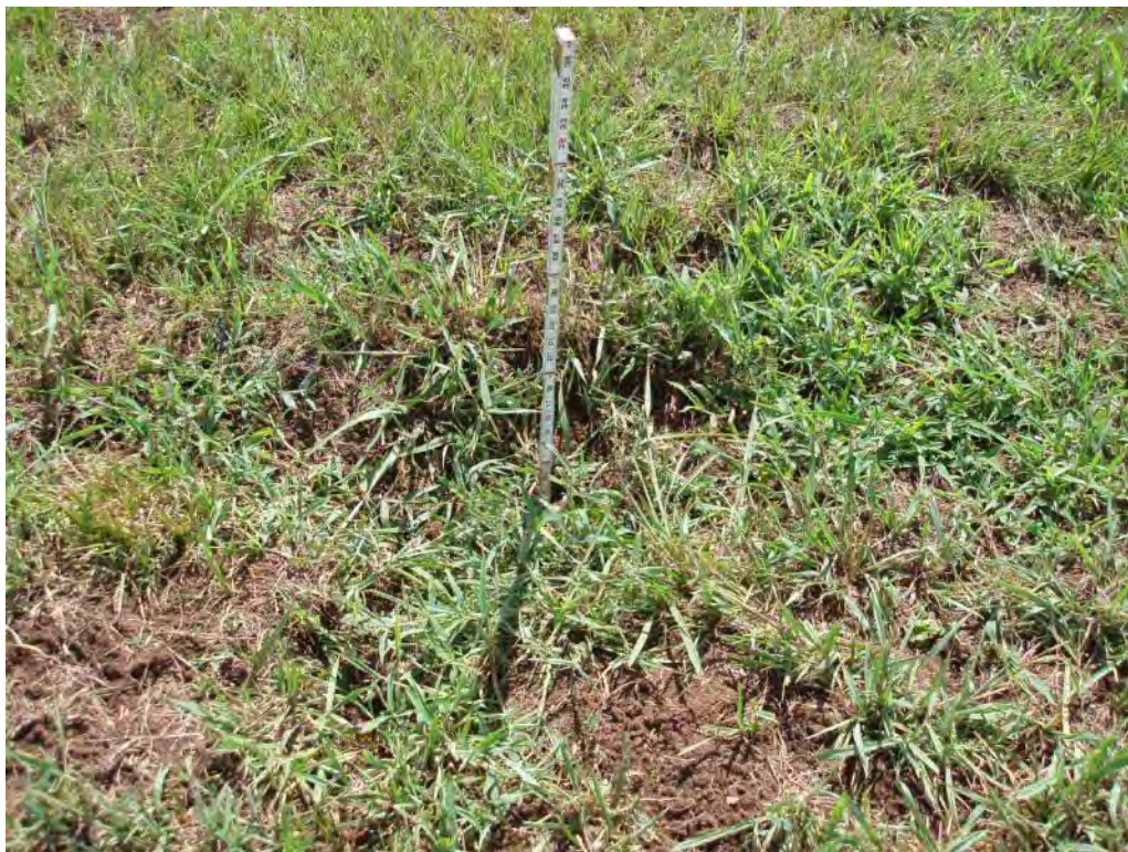
Photo No. 97: Fly Ash Pond – North embankment interior slope. Looking at crack in soils (approximately 2 inches wide and 11 inches deep).
