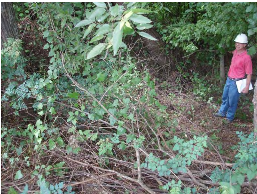
Photo No. 22: Bottom Ash Pond - North embankment exterior slope. Vegetation growing on bottom of slope.
