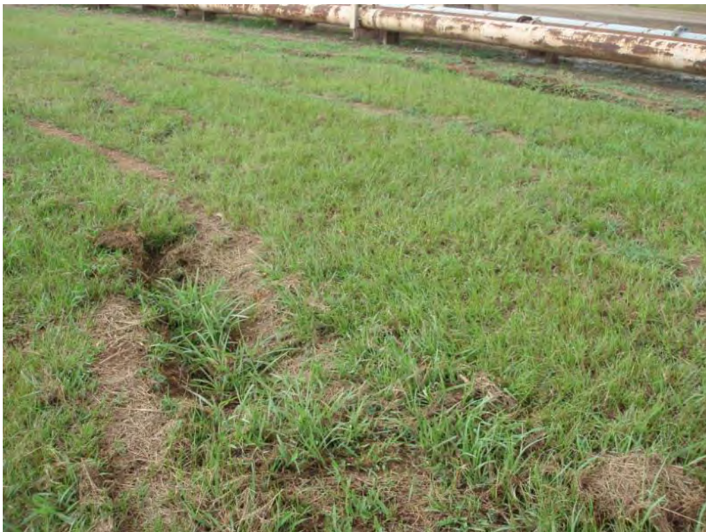
Photo No. 69: Bottom Ash Pond – South embankment interior slope. Looking at rut on slope.
