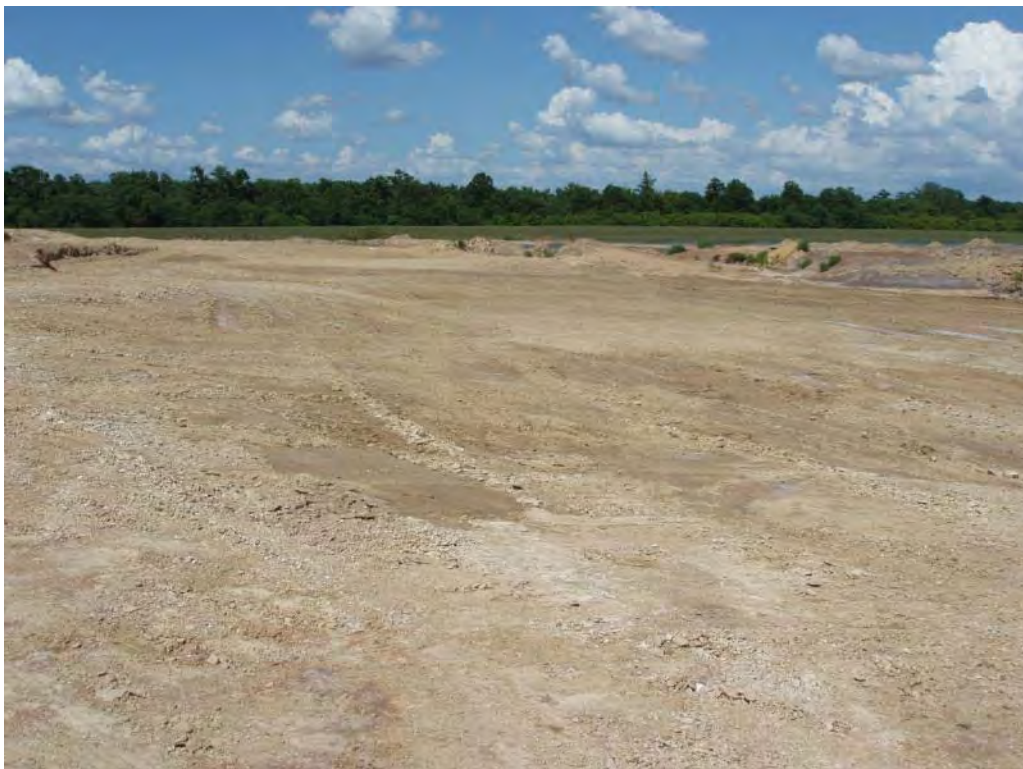
Photo No. 127: Fly Ash Pond - Near southwest corner of pond. Note ash material has been placed up to the crest elevation.
