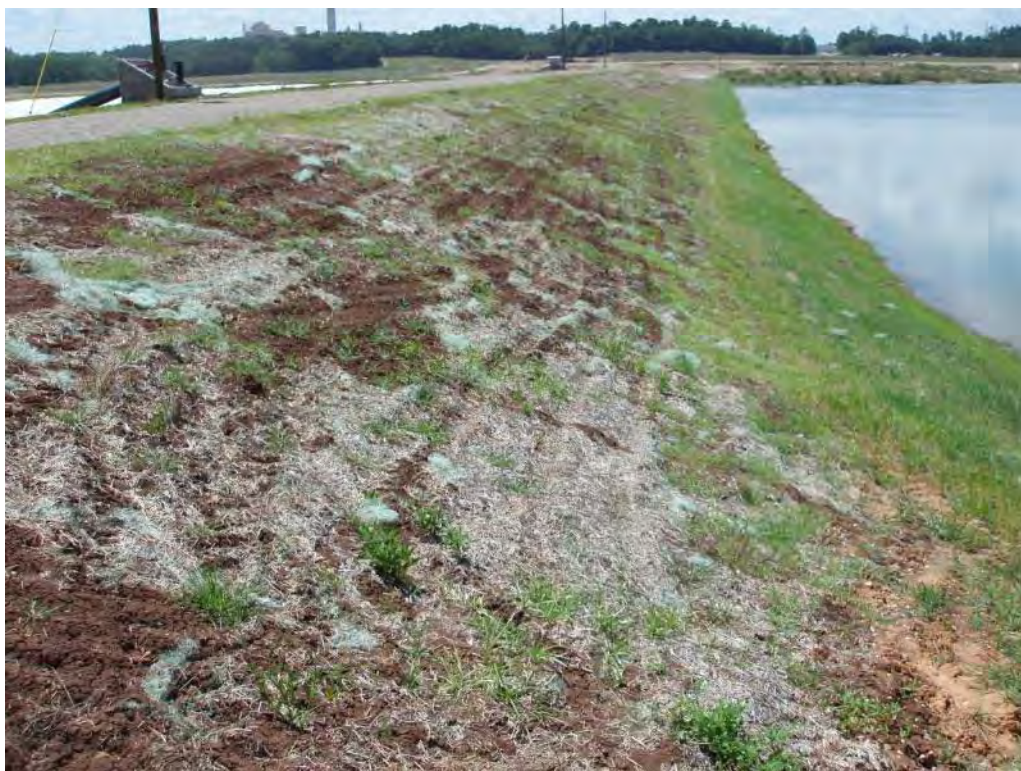
Photo No. 105: Fly Ash Pond - South embankment interior slope, looking northwest. Looking at TRM at location recently re-seeded.
