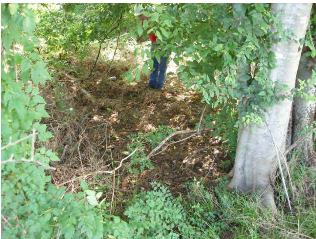
Photo No. 78: Fly Ash Pond - North embankment exterior slope. Vegetation located on bottom third of slope.
