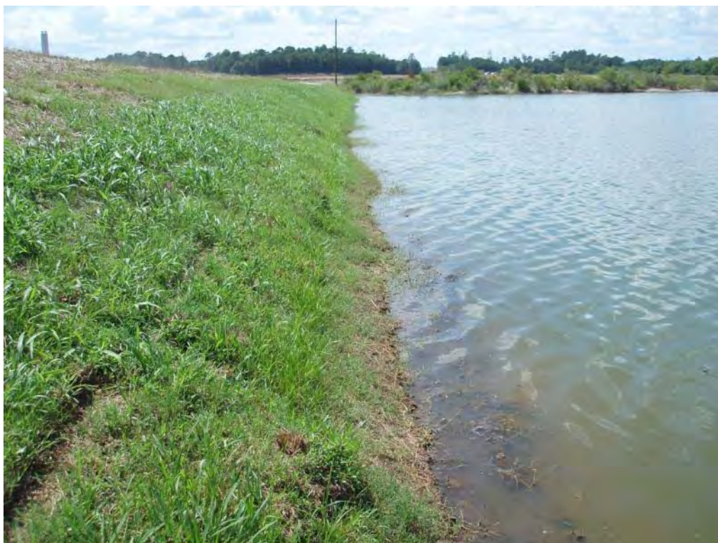
Photo No. 114: Fly Ash Pond – South embankment interior slope, looking northwest. Note erosion near water line and ruts on slope.
