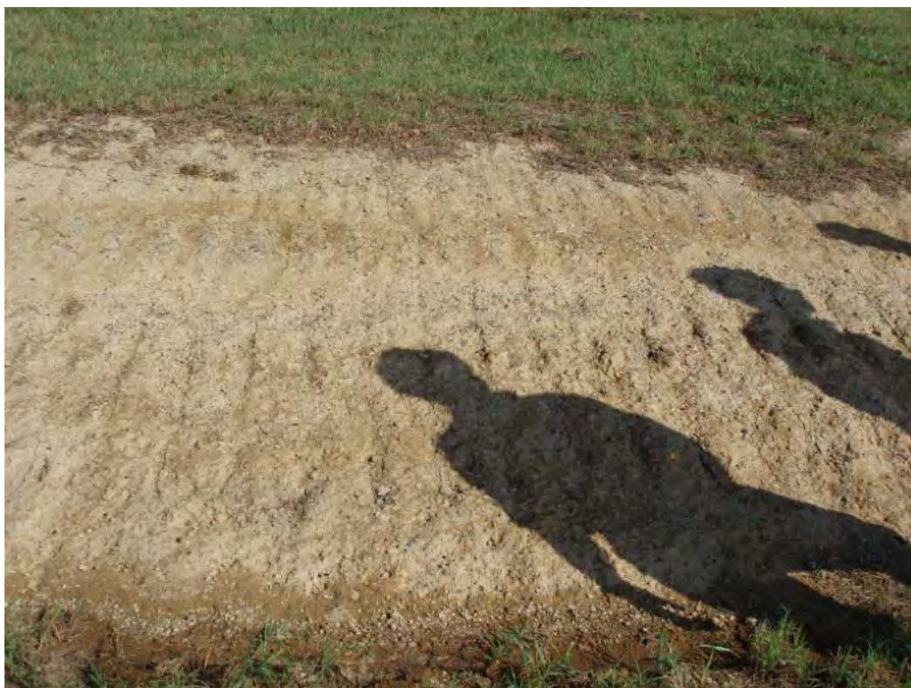
Photo No. 53: Bottom Ash Pond – West embankment interior slope. Looking at close-up of bare patch of soils (also shown in Photo No. 51)
