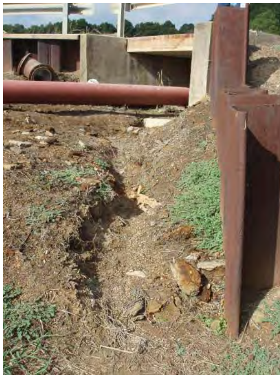
Photo No. 63: Bottom Ash Pond – South embankment interior slope. Looking at erosion rill (approximately 20 inches wide and 10 inches deep) near sluice lines.
