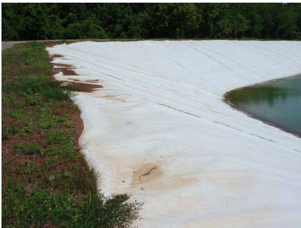
Photo No. 108: Fly Ash Pond - South (divider) embankment exterior slope. Leachate Pond lined with 60-mil-thick HDPE liner.
