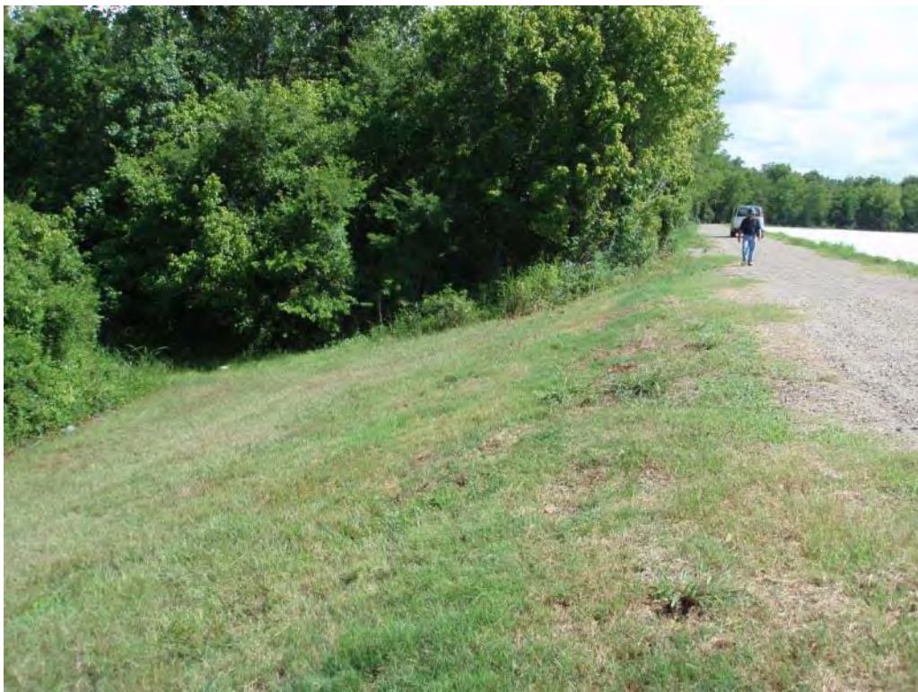
Photo No. 133: Leachate Pond - East embankment exterior slope, looking southeast. Note dense vegetation covering slope.
