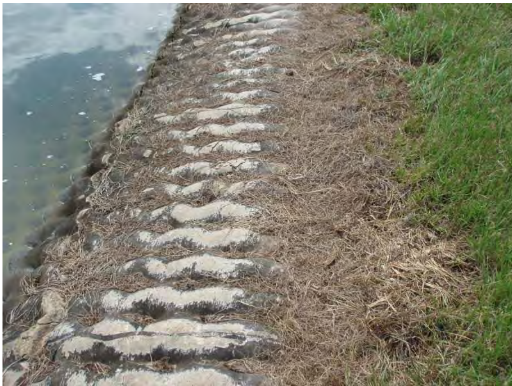
Photo No. 29: Bottom Ash Pond - North embankment interior slope, looking northwest. Looking at concrete armor.
