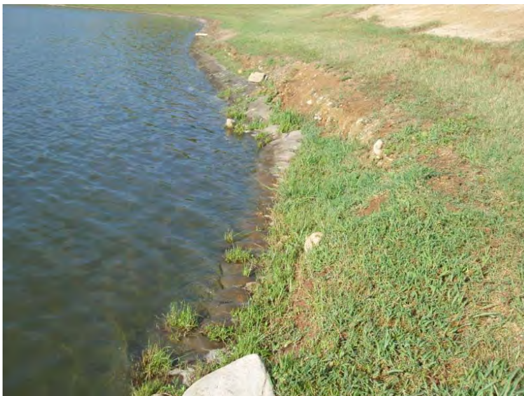
Photo No. 52: Bottom Ash Pond - West embankment interior slope, looking southwest. Looking at surface erosion above concrete armor.
