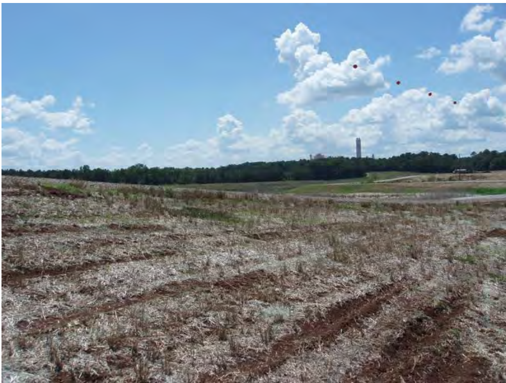
Photo No. 115: Fly Ash Pond - South embankment interior slope, looking northwest. Note area recently re-seeded and covered with TRM.
