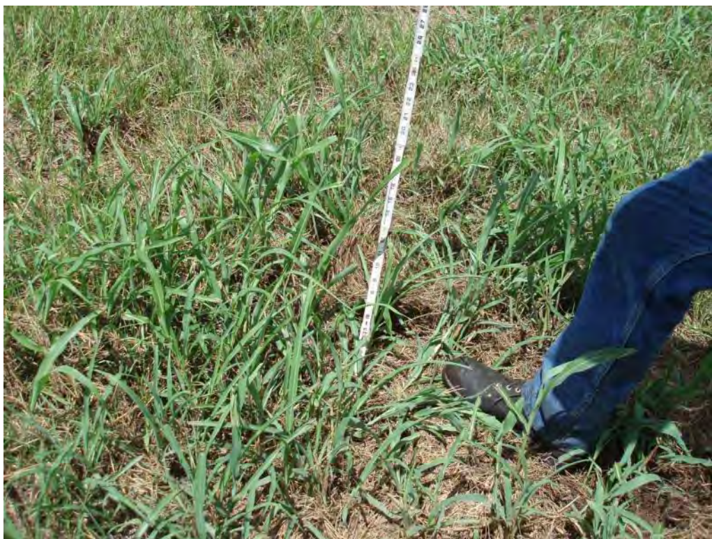
Photo No. 86: Fly Ash Pond - North embankment interior slope. Looking at area of animal rooting/burrowing.
