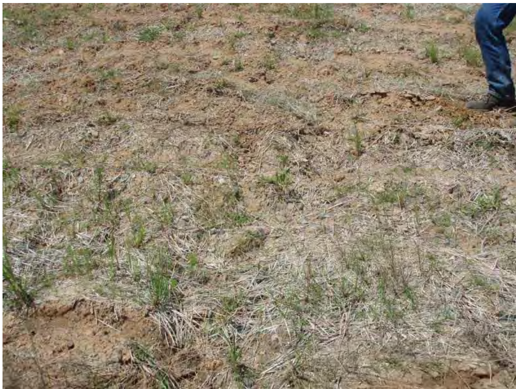
Photo No. 119: Fly Ash Pond - South embankment exterior slope, looking northeast. Note missing vegetation and ruts.
