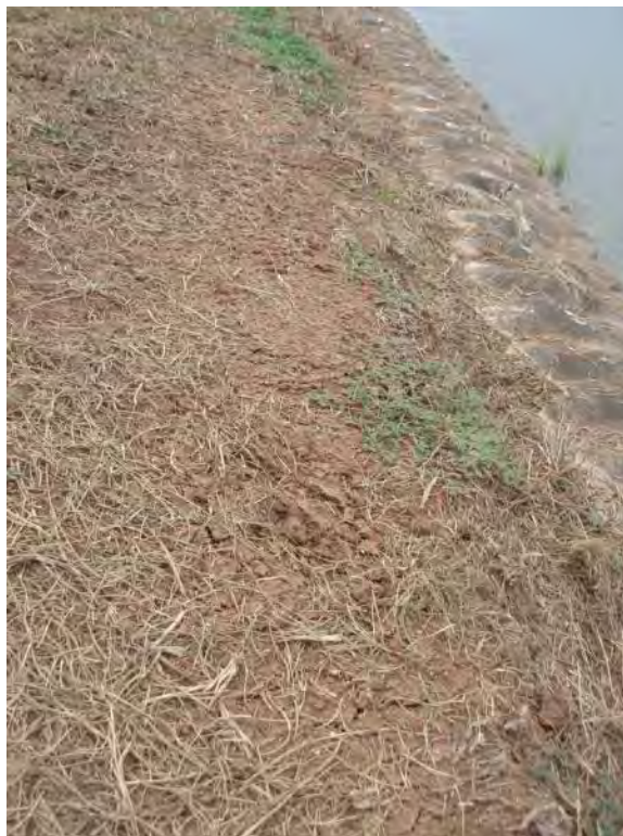
Photo No. 5: Bottom Ash Pond – East embankment interior slope, looking at sparse vegetation and surface cracks.
