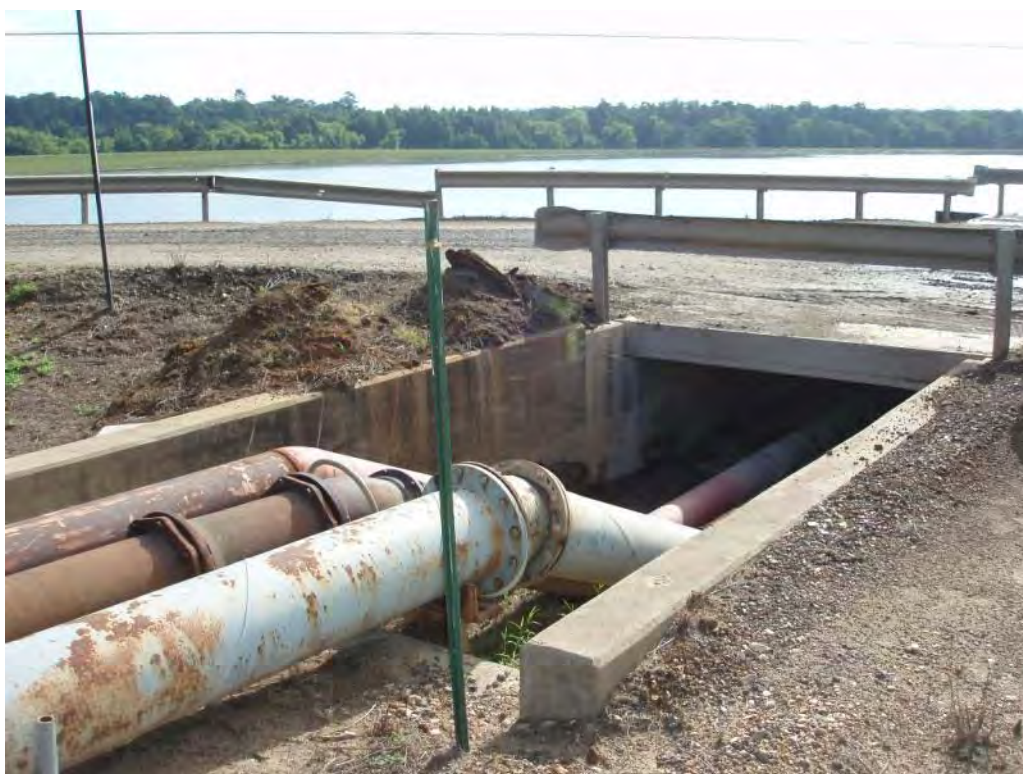
Photo No. 60: Bottom Ash Pond - South embankment exterior slope. Looking at sluice lines passing under haul road at embankment crest.
