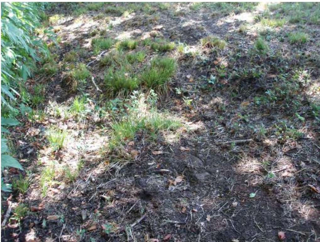
Photo No. 89: Fly Ash Pond - North embankment exterior slope. Looking at small depression in area of spongy, damp soils.
