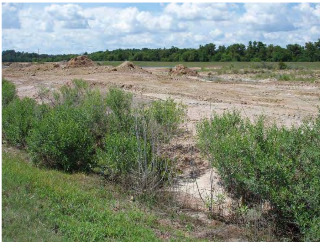
Photo No. 120: Fly Ash Pond - South embankment interior slope, looking northwest. Note ash material placed on slope.
