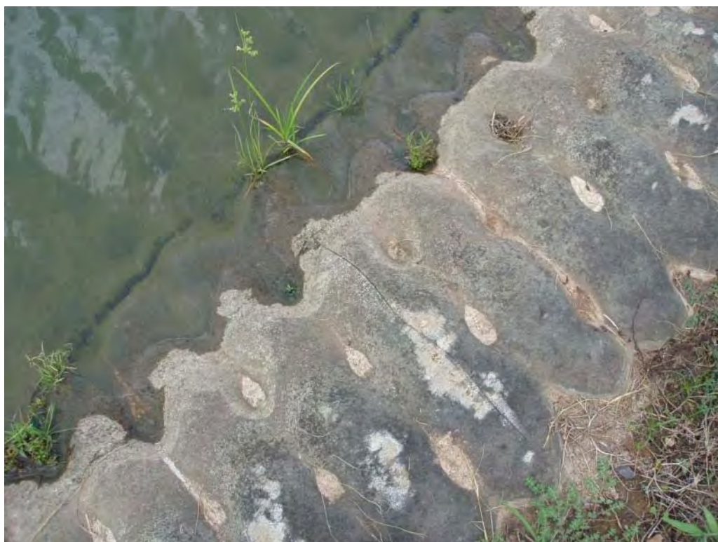
Photo No. 8: Close-up of fracture in concrete armor below waterline, at east embankment interior slope.
