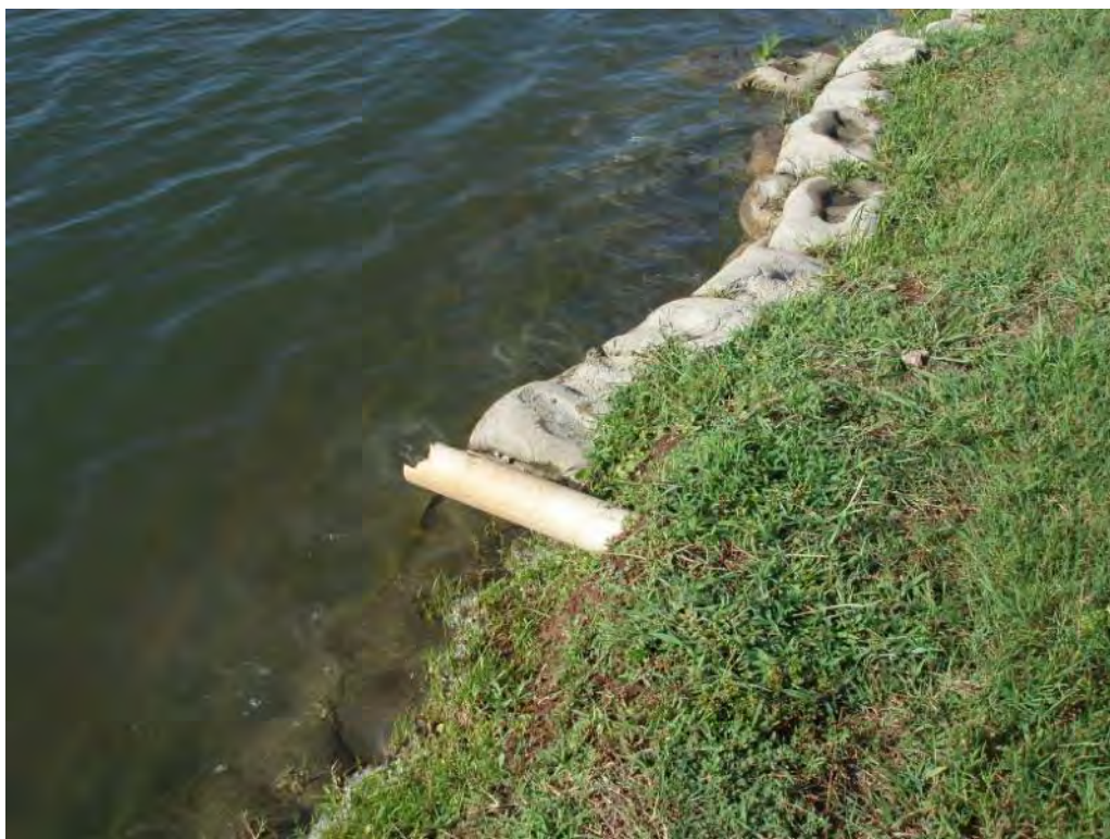
Photo No. 50: Bottom Ash Pond - West embankment interior slope. Looking at discharge pipe (unknown origin) and discontinuation of concrete armor.
