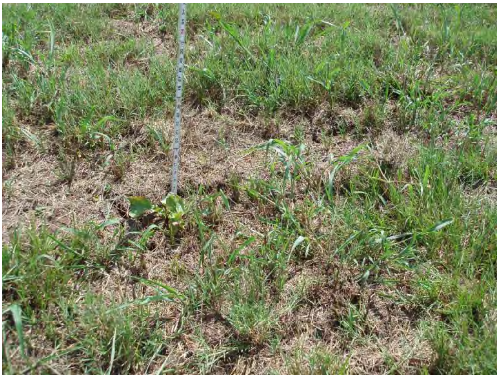
Photo No. 93: Fly Ash Pond - North embankment interior slope. Second location of cracks in soil (approximately 2 inches wide and 14 inches deep).
