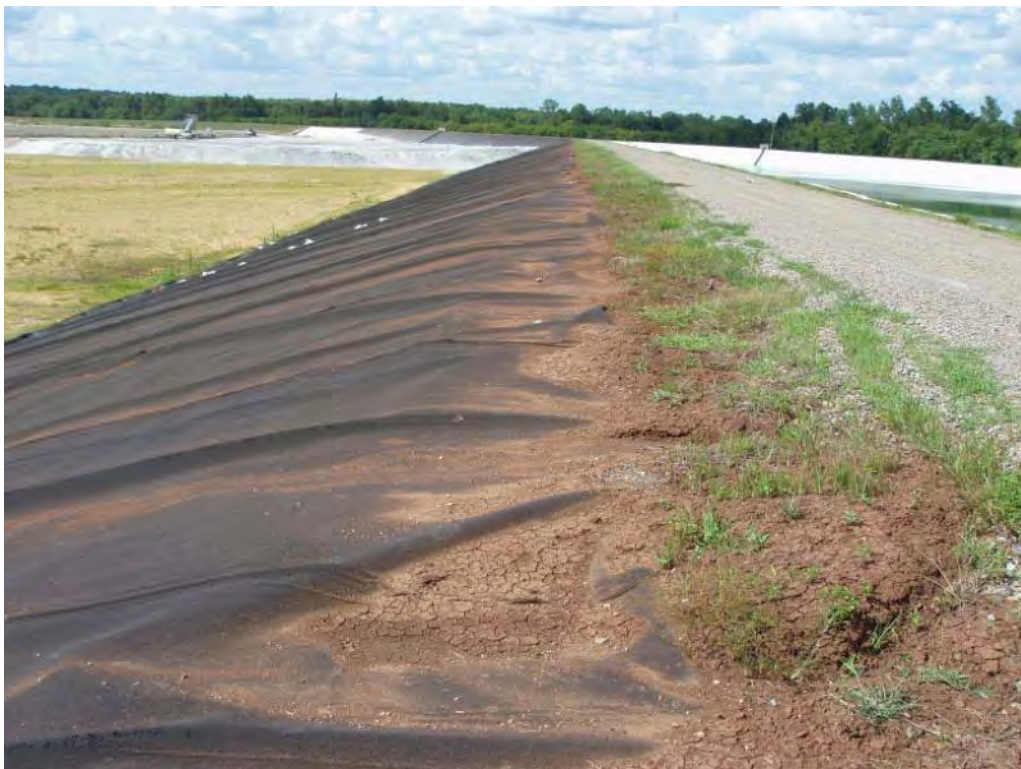
Photo No. 141: Leachate Pond - West embankment exterior slope, looking north. Divider embankment with coal ash landfill covered with geotextile fabric.
