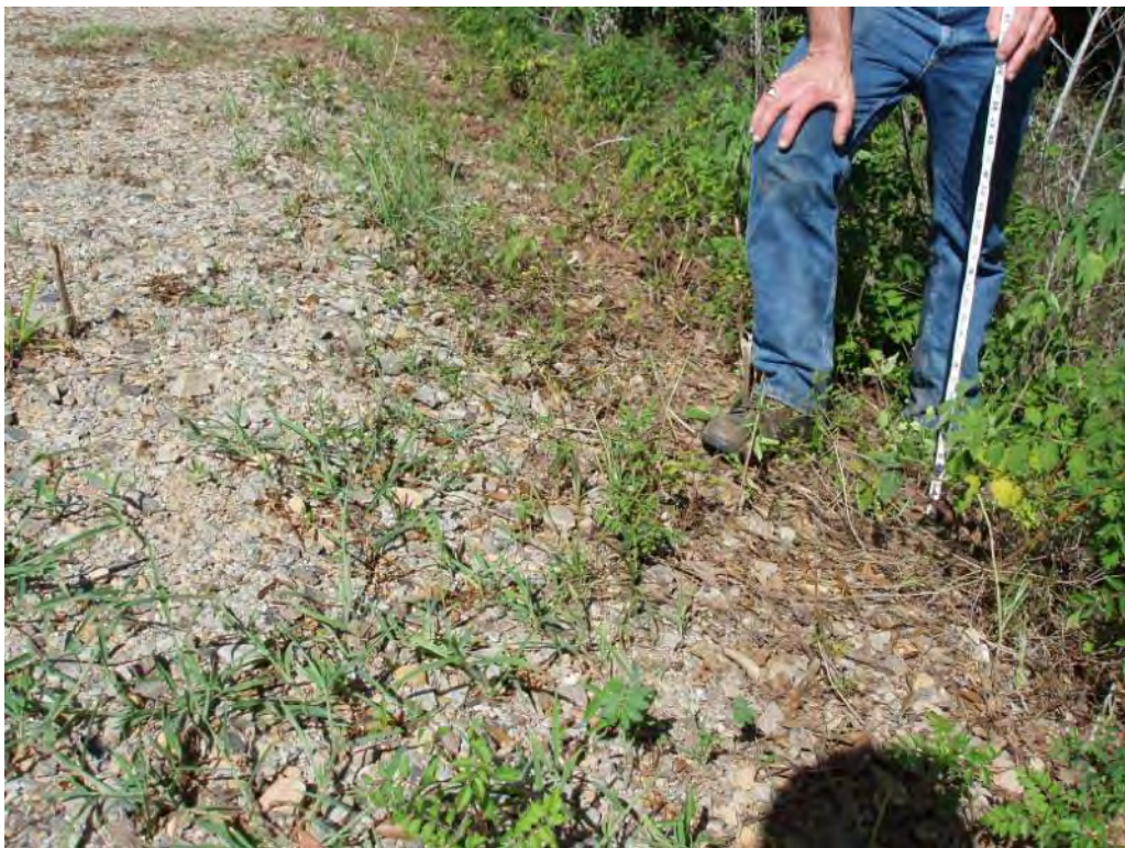
Photo No. 139: Leachate Pond – South embankment exterior slope. Looking at extent of granular surfacing on crest.
