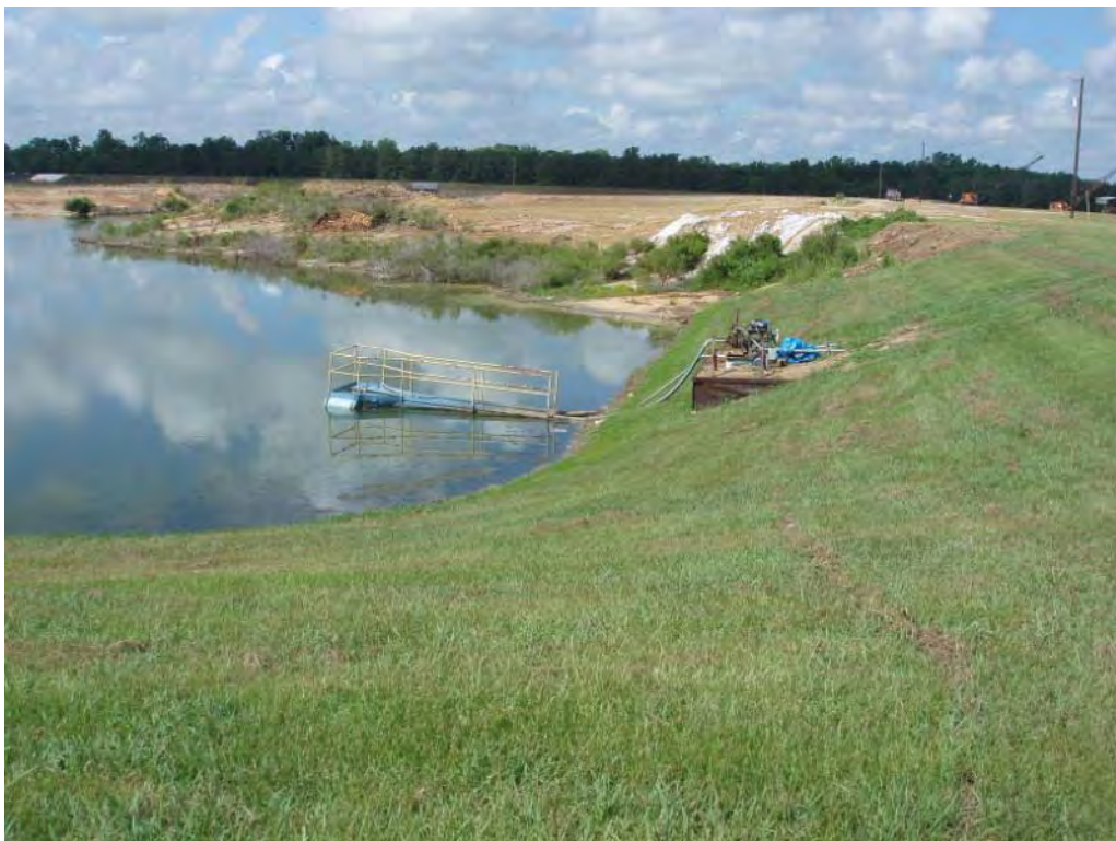
Photo No. 73: Fly Ash Pond – West embankment interior slope, looking southwest. Looking at outlet pump and piping.
