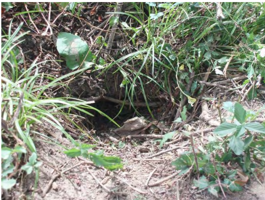
Photo No. 21: Bottom Ash Pond - North embankment exterior slope. Looking at rodent burrow.
