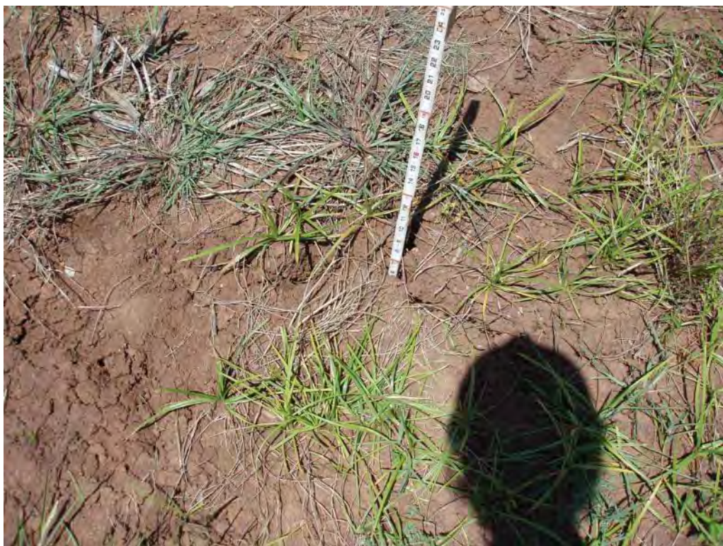
Photo No. 109: Fly Ash Pond – South embankment exterior slope. Looking at cracks in soils (approximately 1 inch wide and 6 inches deep).
