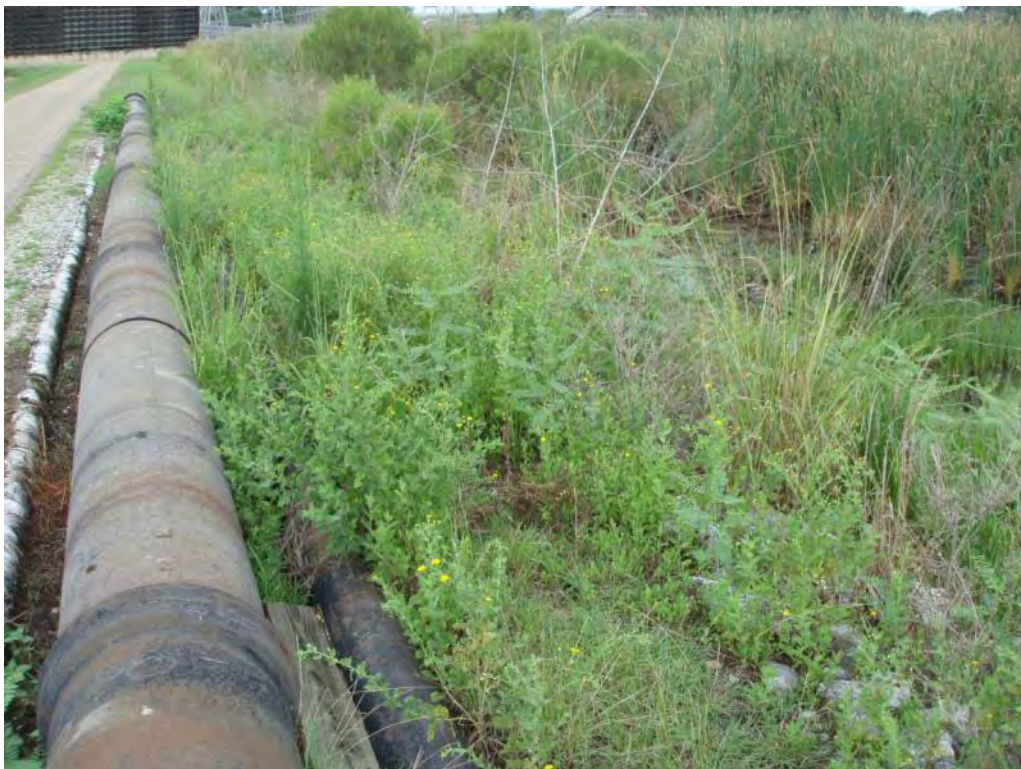
Photo No. 131: #2/#3 Bottom Ash Pond – North embankment interior slope, looking east. Note vegetation growing on slope and cattails within pond.
