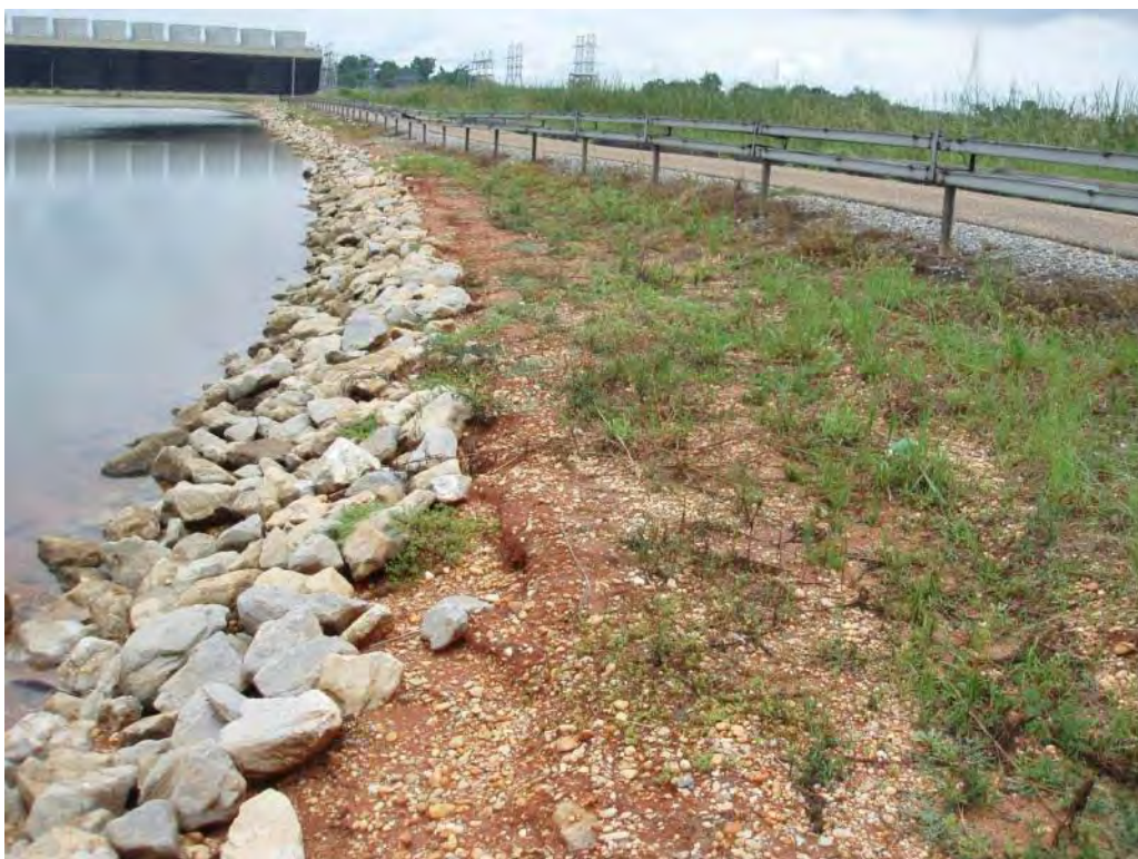
Photo No. 76: Scrubber Waste Pond – South (divider) embankment interior slope, looking east. Note surface erosion and settlement above riprap.
