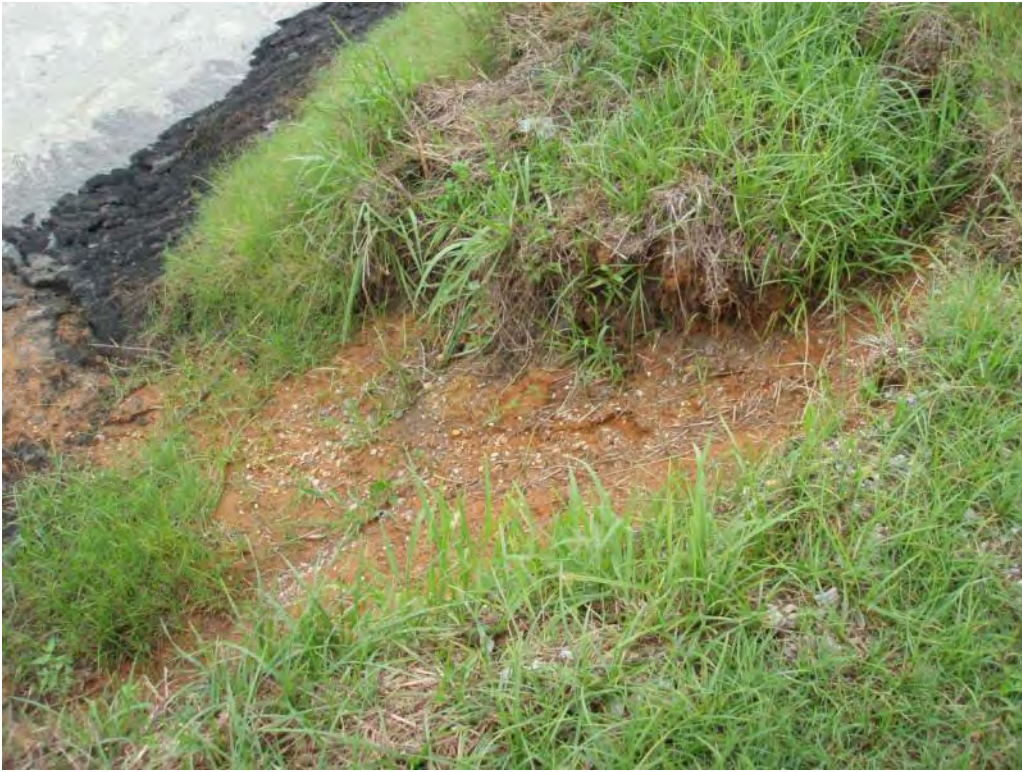
Photo No. 41: #1 Bottom Ash Pond – North embankment interior slope. Looking at erosion rill.
