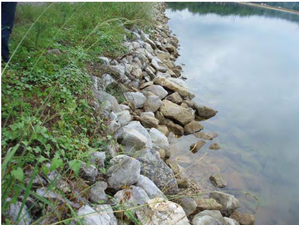
Photo No. 73: Scrubber Waste Pond – West embankment interior slope, looking north. Note erosion of riprap.
