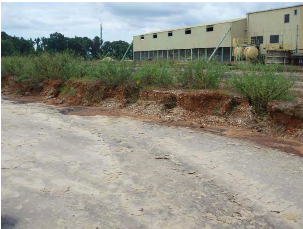
Photo No. 98: Scrubber Waste Pond – North embankment interior slope, looking northwest. Looking at erosion rills in fill material.
