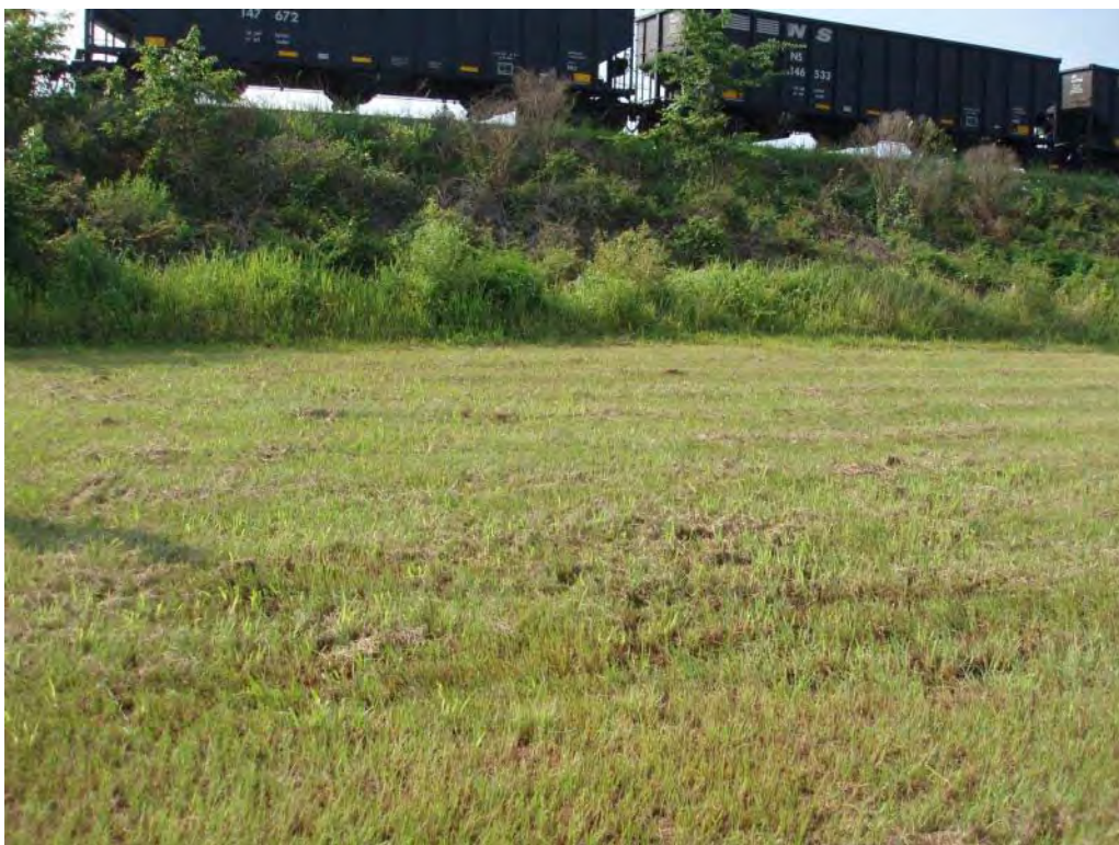
Photo No. 141: #2/#3 Bottom Ash Pond – West embankment exterior slope, looking east. Looking at extent of spongy material in area of possible seepage.
