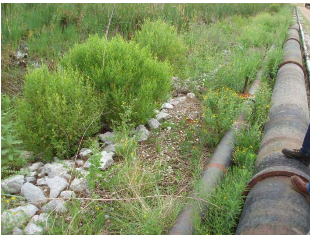
Photo No. 132: #2/#3 Bottom Ash Pond – North embankment interior slope, looking west. Note vegetation growing within riprap.
