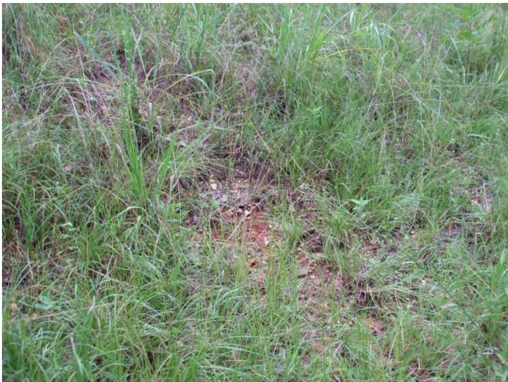
Photo No. 35: #1 Bottom Ash Pond – East embankment exterior slope. Looking at minor surface erosion.
