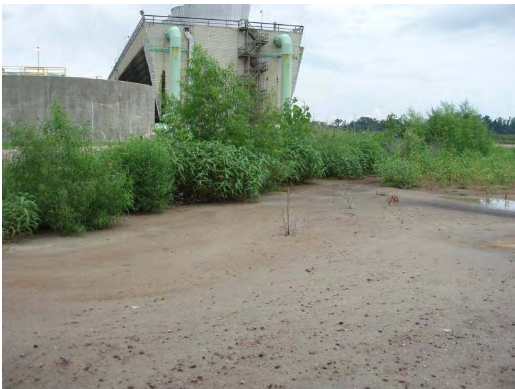
Photo No. 90: Scrubber Waste Pond – East embankment interior slope, looking southeast. Looking at ash product and vegetation on slope.
