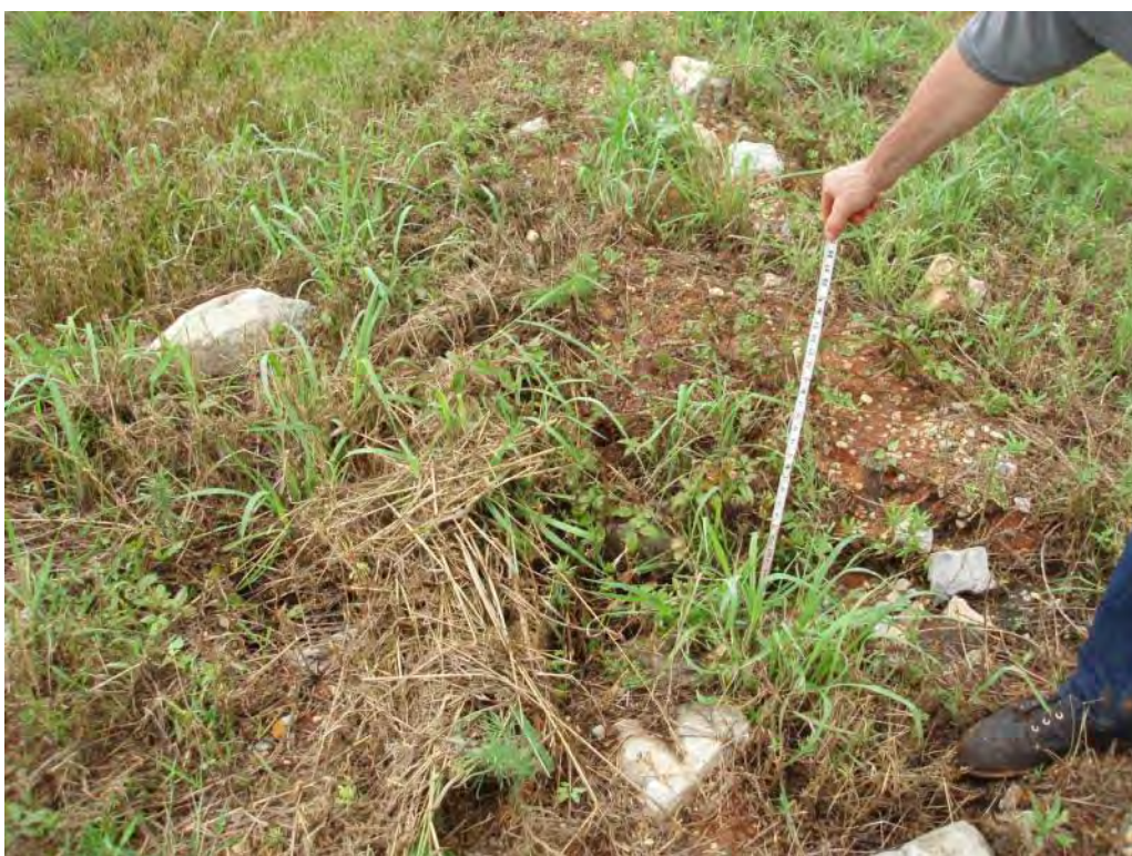
Photo No. 84: Scrubber Waste Pond – East embankment interior slope. Looking at surface erosion and sparse riprap.
