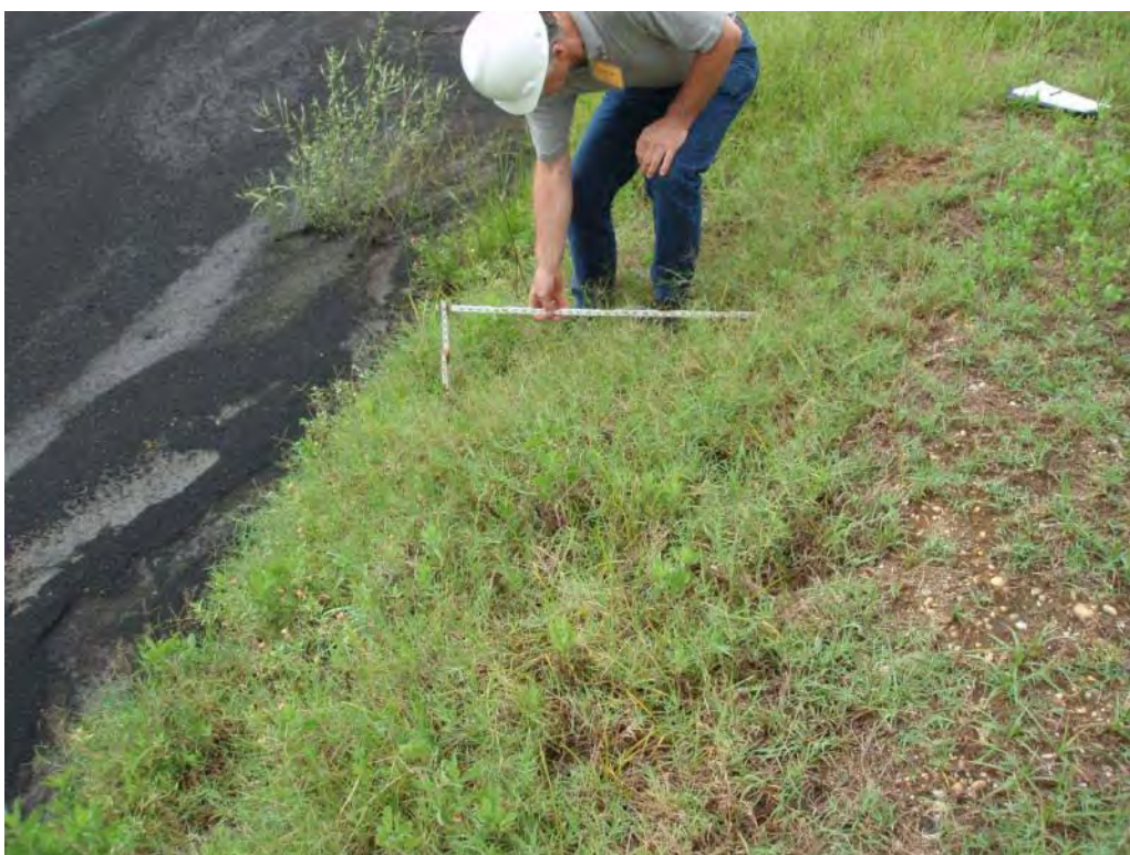
Photo No. 6: #1 Bottom Ash Pond – West embankment interior slope. 3H:1V slope measured toward bottom of slope, 2H:1V measured on upper 8 to 10 feet.
