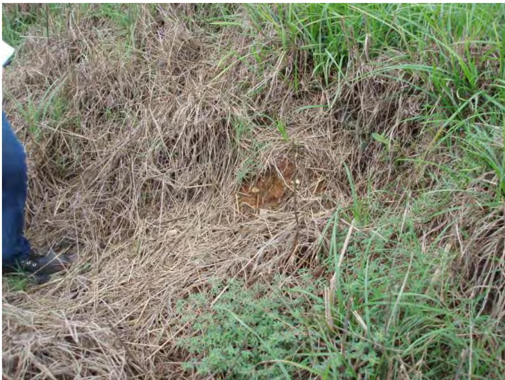
Photo No. 43: #1 Bottom Ash Pond - North embankment interior slope. Looking at surface erosion.
