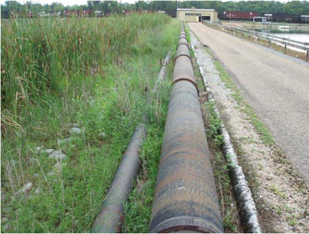
Photo No. 133: #2/#3 Bottom Ash Pond – North (divider) embankment interior slope and crest, looking west. Note dense vegetation covering slope.
