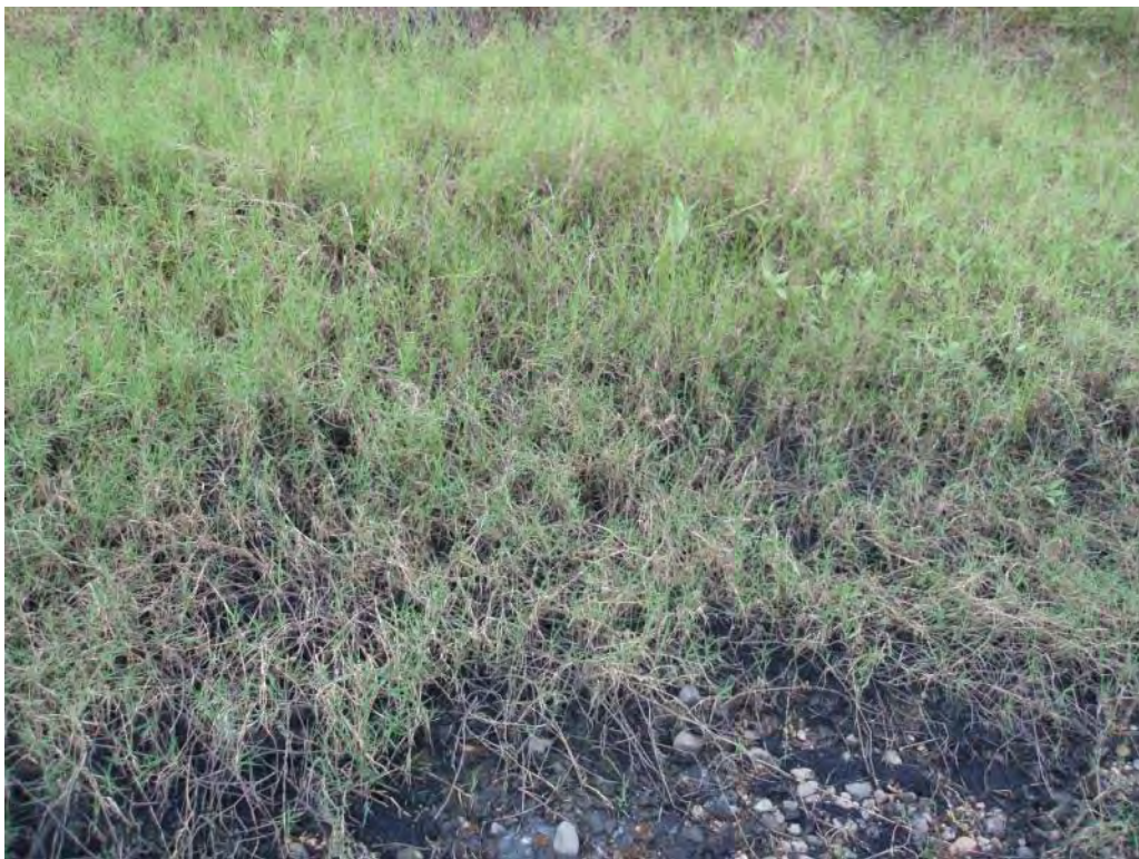
Photo No. 31: #1 Bottom Ash Pond – East embankment interior slope. Note vegetation and surface erosion.
