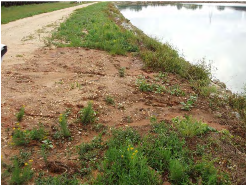
Photo No. 55: Process Waste Pond – West embankment interior slope, looking north. Note surface erosion.
