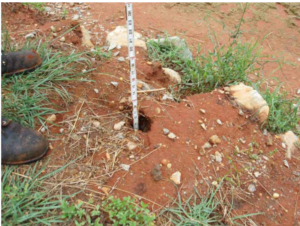
Photo No. 80: Scrubber Waste Pond – South embankment exterior slope. Looking at 10-inch-deep void in soils.
