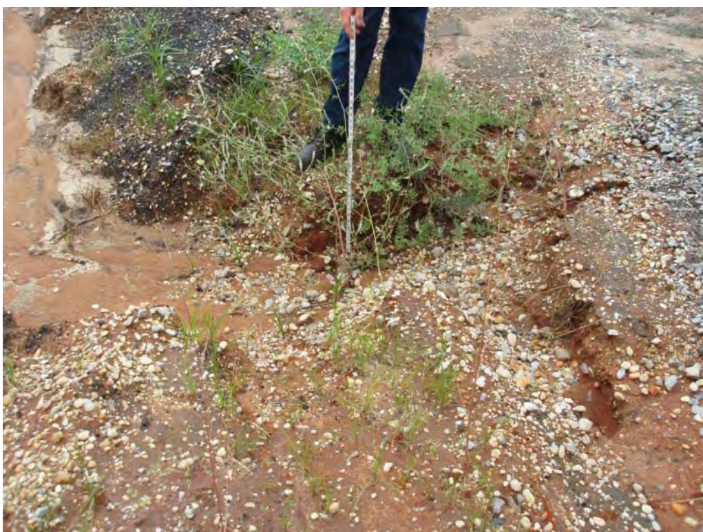
Photo No. 96: Scrubber Waste Pond – North (divider) embankment interior slope. Looking at erosion rills in fill material.
