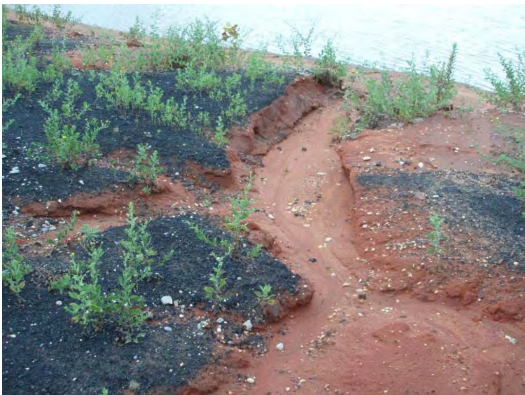
Photo No. 59: Process Waste Pond – South (divider) embankment exterior slope. Looking at erosion rills in fill material.
