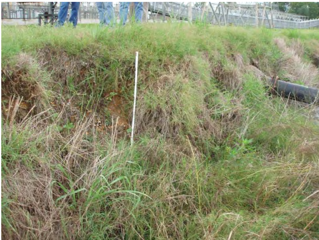
Photo No. 47: North embankment interior slope, looking northeast. Looking at erosion rill. Sluice line from Unit 1 to the right.
