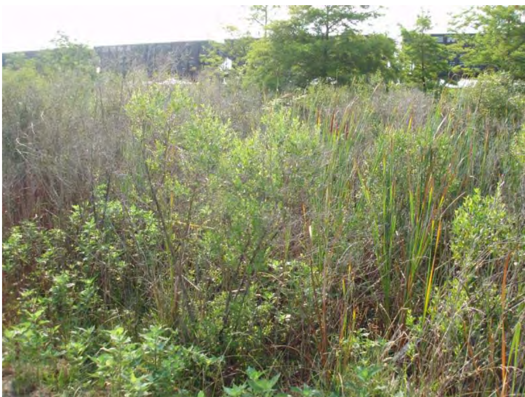
Photo No. 142: Scrubber Waste Pond – West embankment exterior slope. Note dense vegetation on slope.
