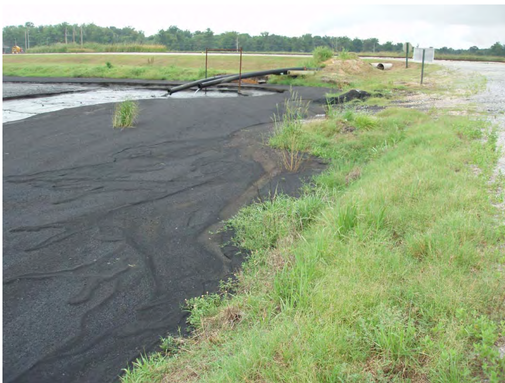
Photo No. 2: #1 Bottom Ash Pond – North embankment interior slope, looking west. Looking at sluice line discharge from Units 2 & 3.
