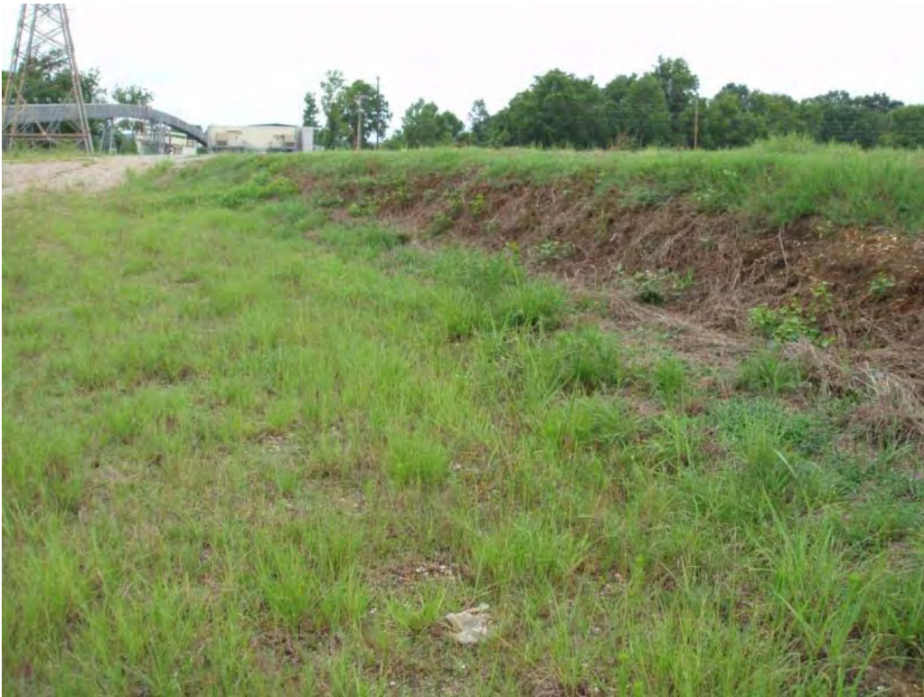
Photo No. 45: #1 Bottom Ash Pond - North embankment exterior slope, looking east. Note surface erosion on upper slope.
