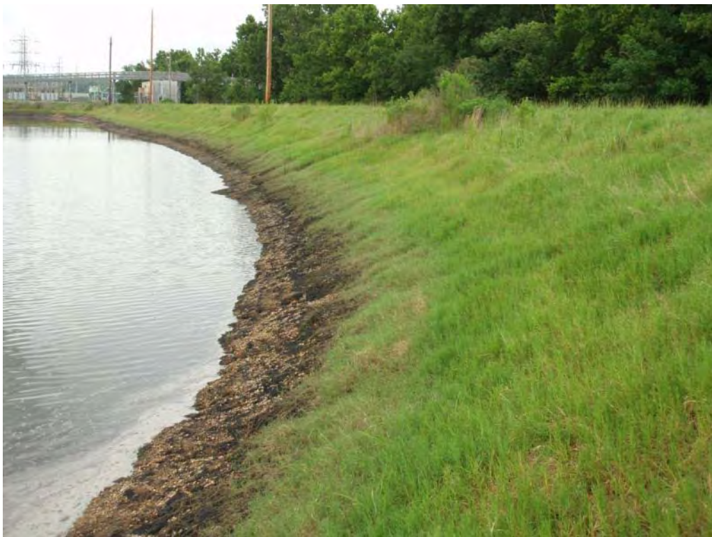
Photo No. 25: #1 Bottom Ash Pond – East embankment interior slope, looking north. Note surface erosion near water line.
