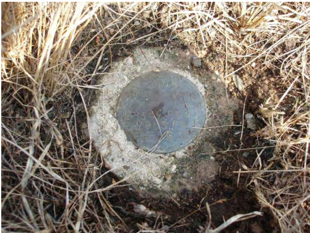
Photo No. 145: #2/#3 Bottom Ash Pond – South embankment exterior slope. Looking at plant survey monument.
