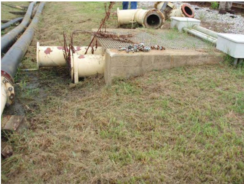
Photo No. 123: #2/#3 Bottom Ash Pond - East embankment exterior slope, looking south. Looking at piping used to divert Units 1, 2, & 3 CCW from the #1 Bottom Ash Pond into the #2/#3 Bottom Ash Pond.
