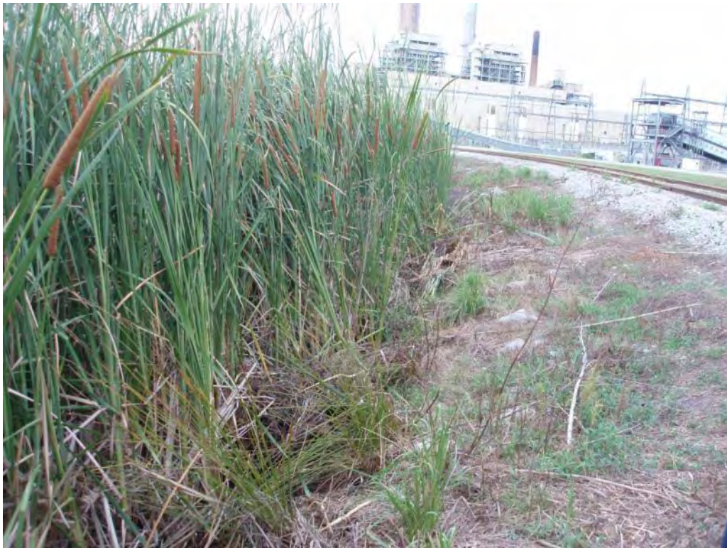
Photo No. 117: #2/#3 Bottom Ash Pond – East embankment interior slope, looking north. Note sparse riprap and cattails growing on slope.
