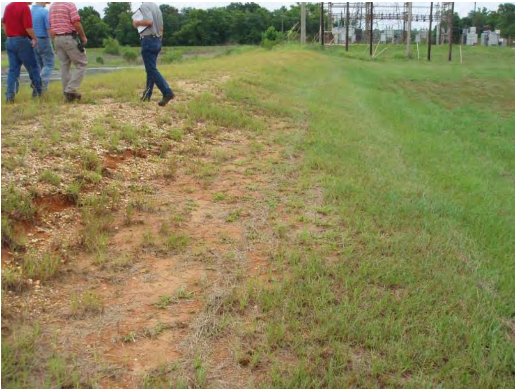
Photo No. 17: #1 Bottom Ash Pond – South embankment exterior slope, looking east. Note surface erosion.
