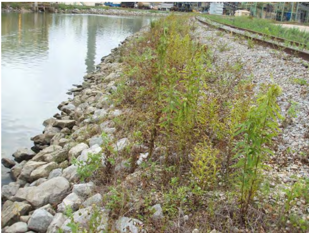
Photo No. 61: Process Waste Pond – South embankment interior slope, looking east. Note vegetation growing within riprap
