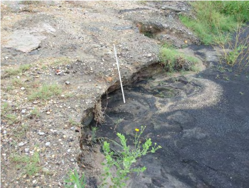
Photo No. 3: #1 Bottom Ash Pond – North embankment interior slope, looking east. Ash product covering slope.
