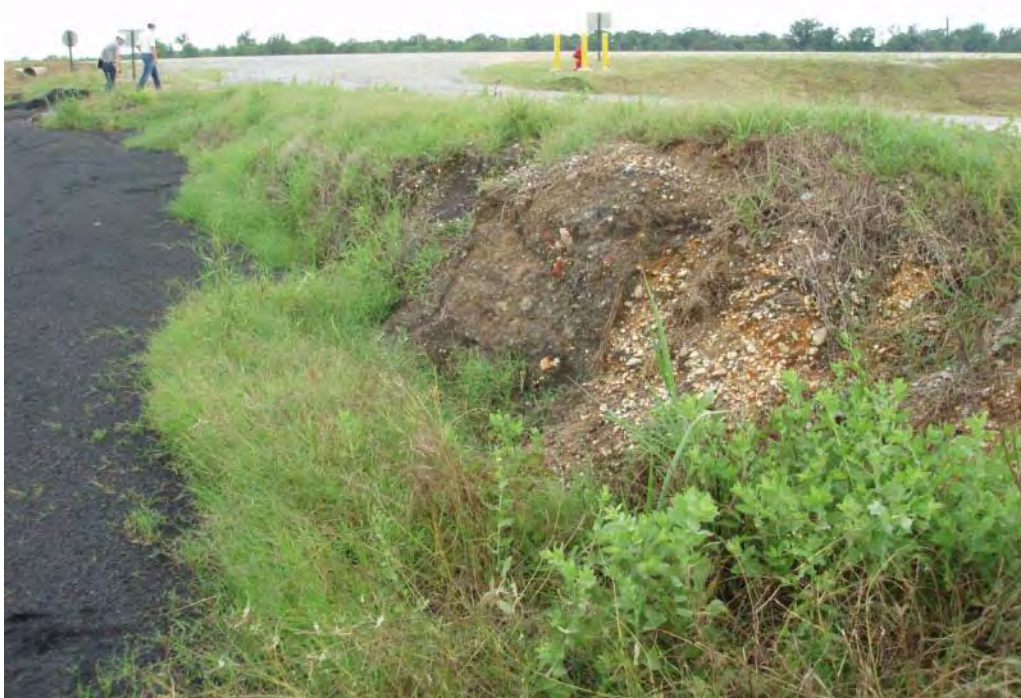
Photo No. 48: #1 Bottom Ash Pond – North embankment interior slope, looking northwest. Looking at surface erosion.
