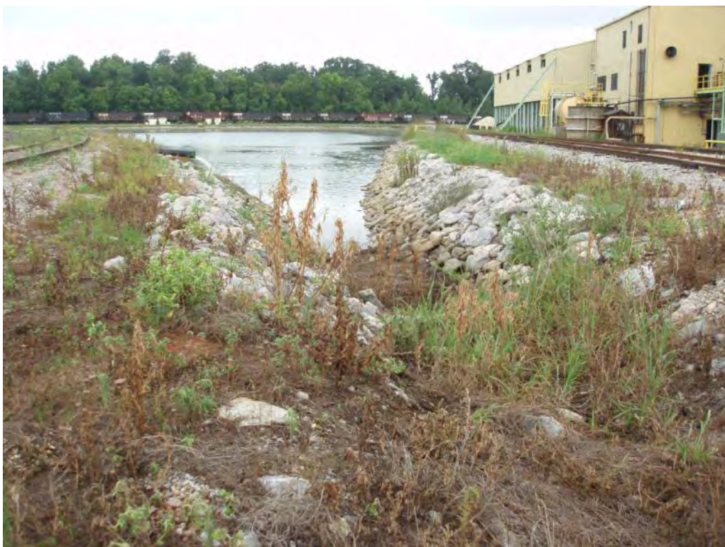
Photo No. 63: Process Waste Pond – South and north embankment interior slopes, looking northwest. Note vegetation growing within riprap.
