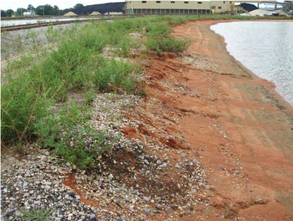
Photo No. 57: Process Waste Pond – South (divider) embankment exterior slope, looking east. Note erosion rills in fill material, placed in the past for construction access road.
