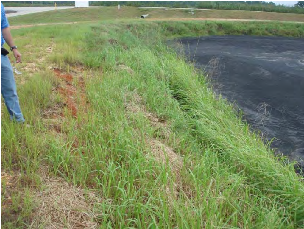
Photo No. 15: #1 Bottom Ash Pond – South embankment interior slope, looking west. Note minor surface erosion.
