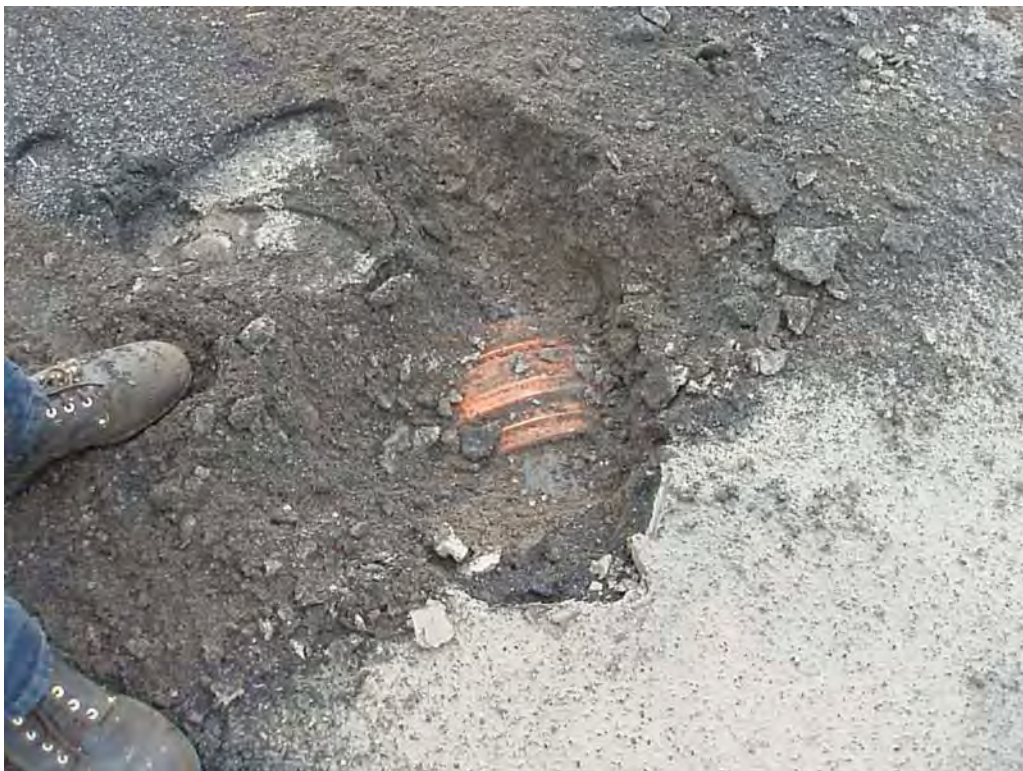
Photo No. 125: #2/#3 Bottom Ash Pond – East embankment interior slope. Looking at buried piping within ash product.
