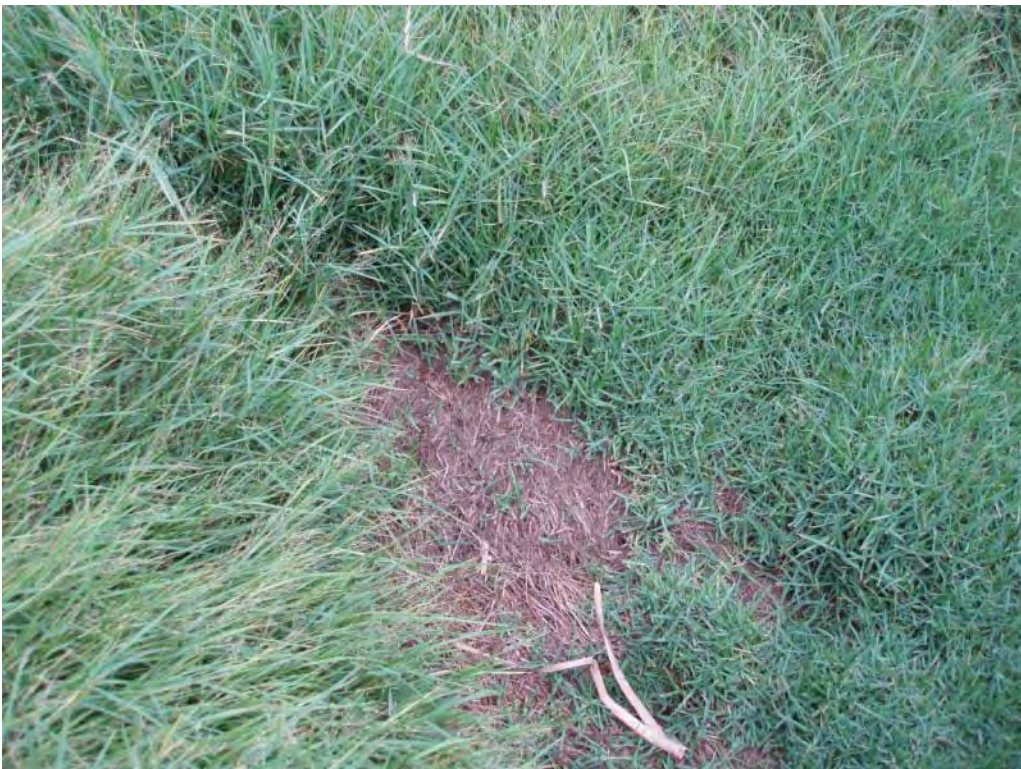
Photo No. 128: #2/#3 Bottom Ash Pond – North embankment interior slope. Looking at rut or inactive erosion rill.
