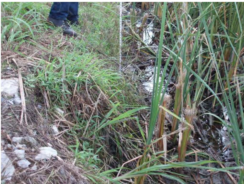
Photo No. 114: #2/#3 Bottom Ash Pond – South embankment interior slope, looking southwest. Looking at erosion and missing riprap.
