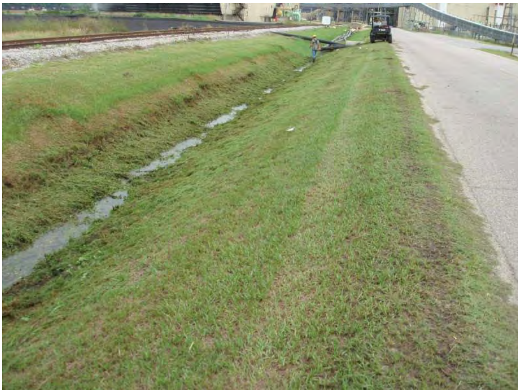
Photo No. 7: #1 Bottom Ash Pond – West embankment exterior slope, looking north. Note standing water in drainage ditch at toe.
