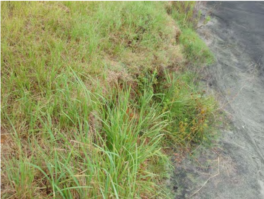
Photo No. 18: #1 Bottom Ash Pond – South embankment interior slope, looking west. Note erosion and undercut of slope.
