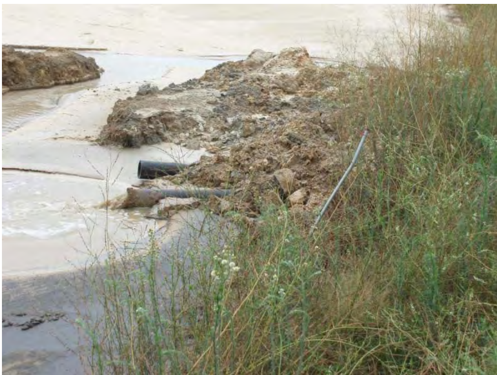
Photo No. 95: Scrubber Waste Pond – North embankment interior slope. Looking at discharge pipes from gypsum plant.
