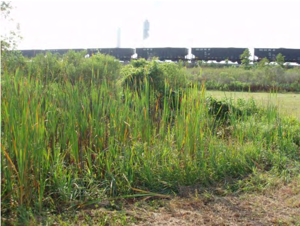
Photo No. 143: Scrubber Waste Pond – Outside west embankment toe. Looking at cattails in area of possible seepage.
