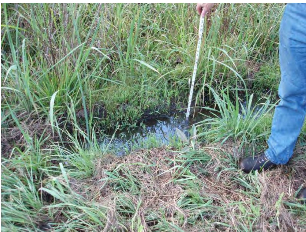
Photo No. 138: #2/#3 Bottom Ash Pond – West embankment exterior slope. Looking at area of possible seepage.
