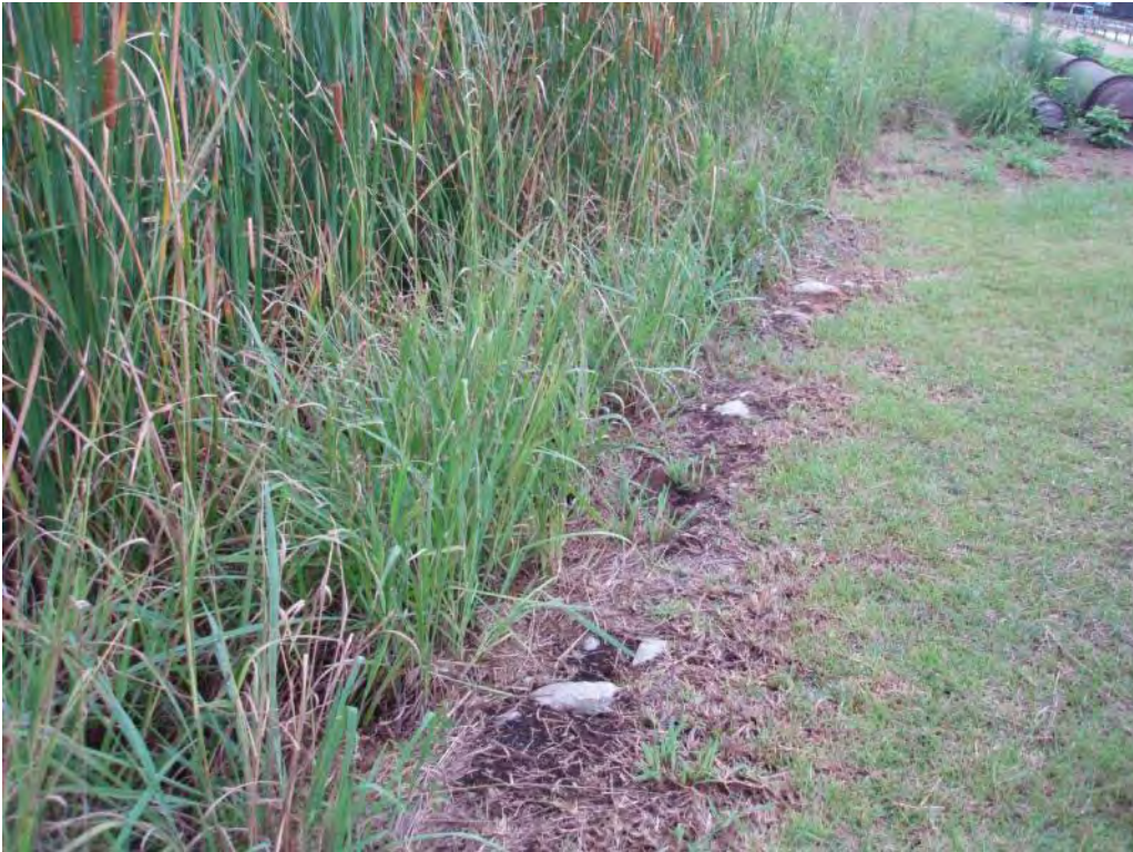
Photo No. 129: #2/#3 Bottom Ash Pond – North embankment interior slope. Looking at vegetation and sparse riprap.
