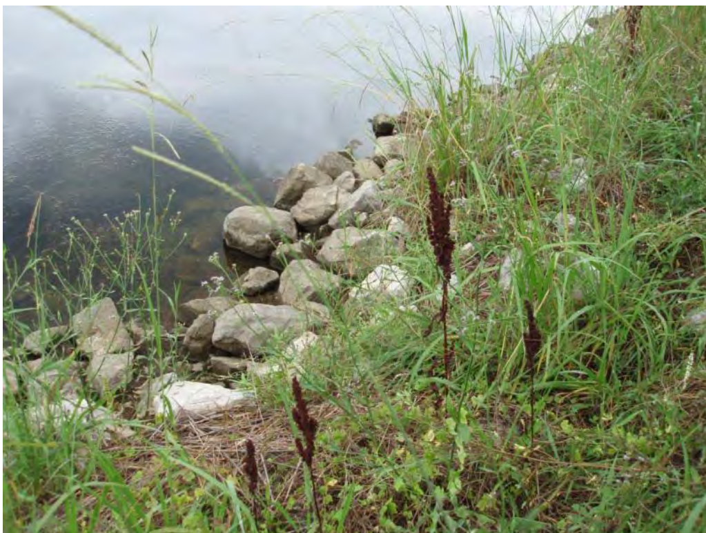
Photo No. 106: #2/#3 Bottom Ash Pond – West embankment interior slope. Looking at erosion of riprap.
