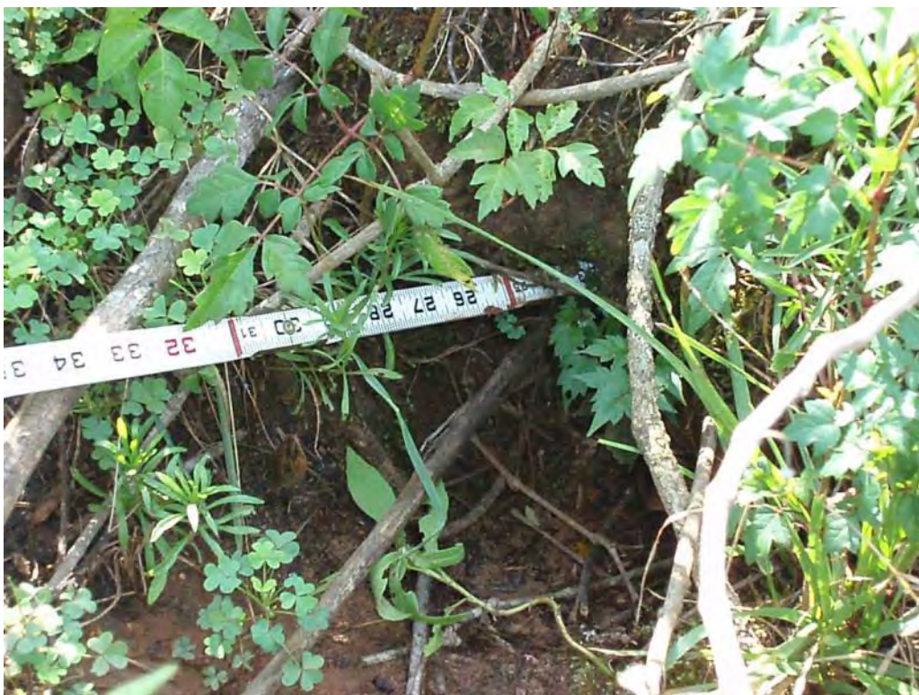
Photo No. 150: Scrubber Waste Pond – West embankment exterior slope. Looking at rodent burrow (4 inches in diameter, 26 inches deep).
