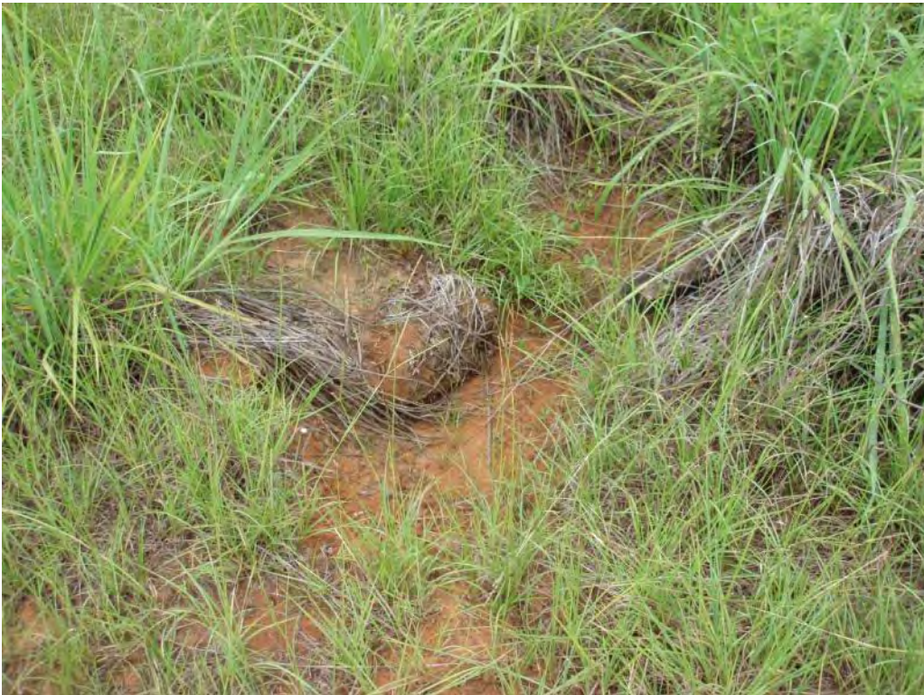
Photo No. 22: #1 Bottom Ash Pond – South embankment exterior slope. Looking at minor erosion rill.
