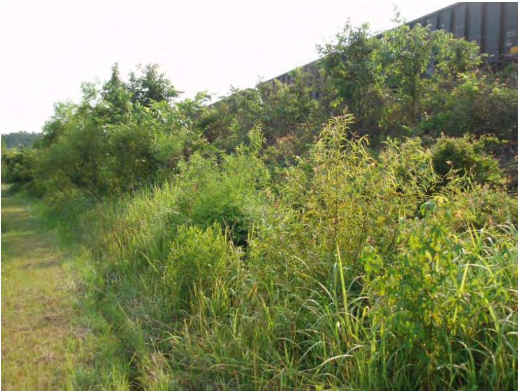
Photo No. 139: #2/#3 Bottom Ash Pond – West embankment exterior slope, looking north. Note dense vegetation on slope.
