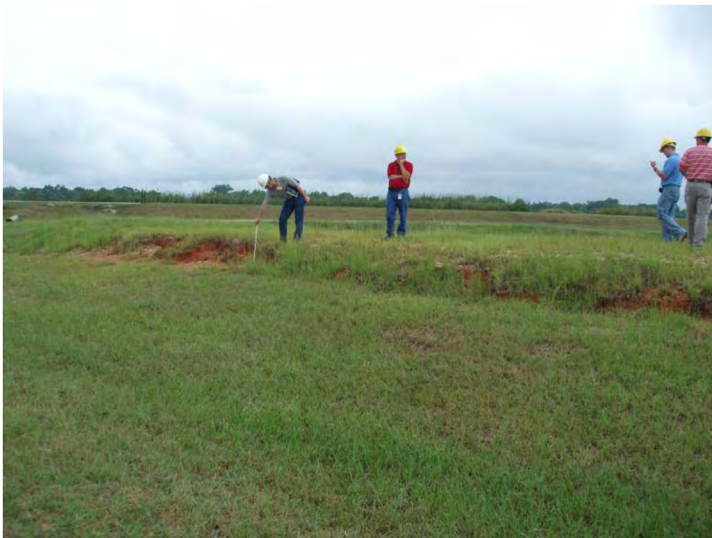
Photo No. 14: #1 Bottom Ash Pond – South embankment exterior slope, looking north. Note surface erosion.
