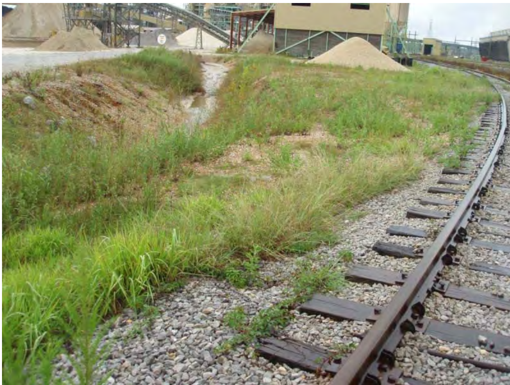
Photo No. 69: Process Waste Pond – North embankment crest, incised into finished yard grade.
