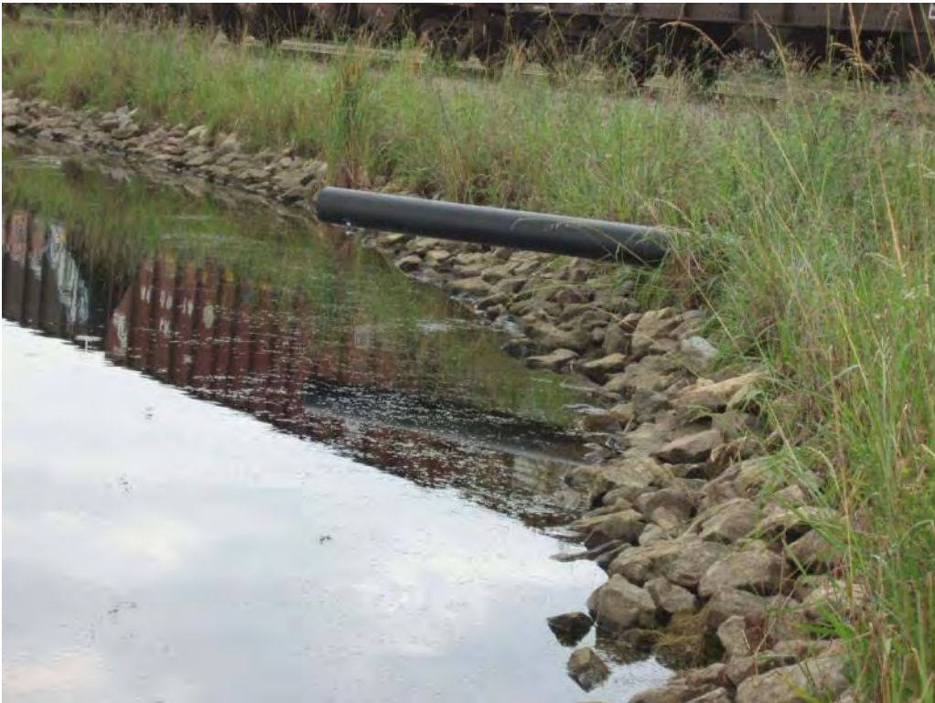
Photo No. 104: #2/#3 Bottom Ash Pond – West embankment interior slope, looking southwest. Looking at discharge pipe from pump station.
