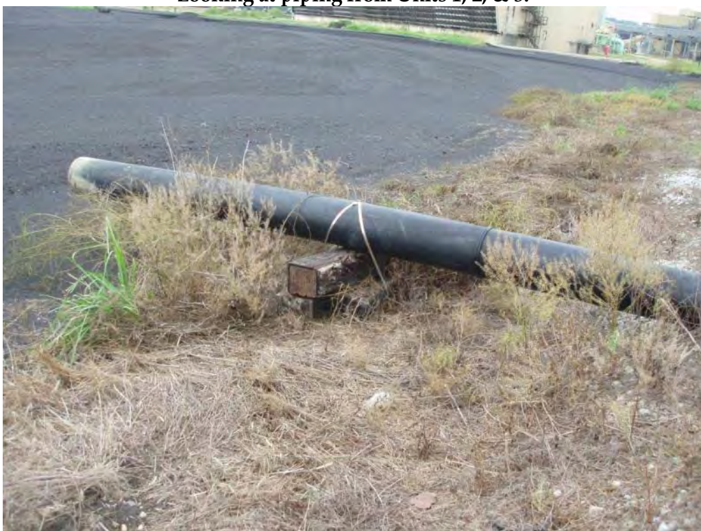
Photo No. 120: #2/#3 Bottom Ash Pond – East embankment interior slope. Looking at inactive discharge pipe from Units 1, 2, & 3. Note sluice lines were configured for discharge of Units 1, 2 & 3 CCW to #1 Bottom Ash Pond.
