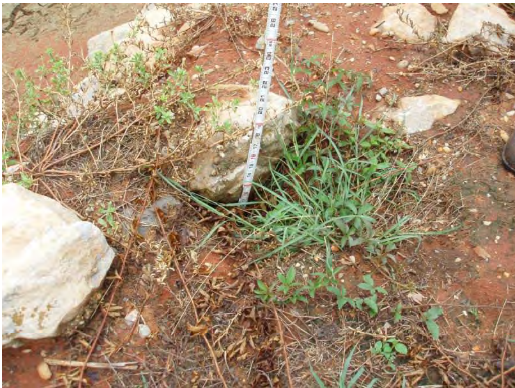
Photo No. 79: Scrubber Waste Pond – South embankment exterior slope. Looking at 10-inch-deep void beneath riprap.
