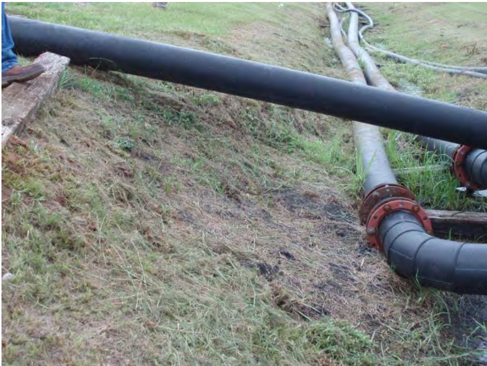
Photo No. 122: #2/#3 Bottom Ash Pond – East embankment exterior slope. Looking at piping used to divert Units 1, 2, & 3 CCW from the #1 Bottom Ash Pond into the #2/#3 Bottom Ash Pond.
