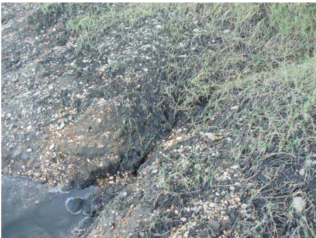
Photo No. 28: #1 Bottom Ash Pond – East embankment interior slope. Looking at erosion rills.
