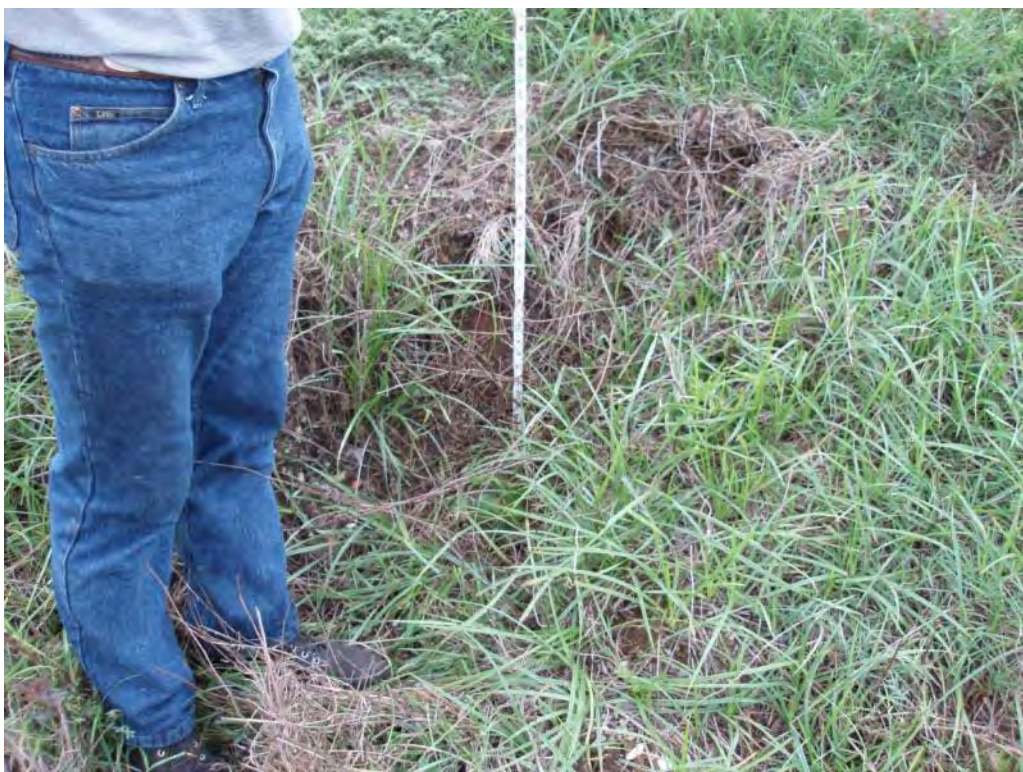
Photo No. 44: #1 Bottom Ash Pond - North embankment interior slope. Looking at surface erosion/erosion rill.
