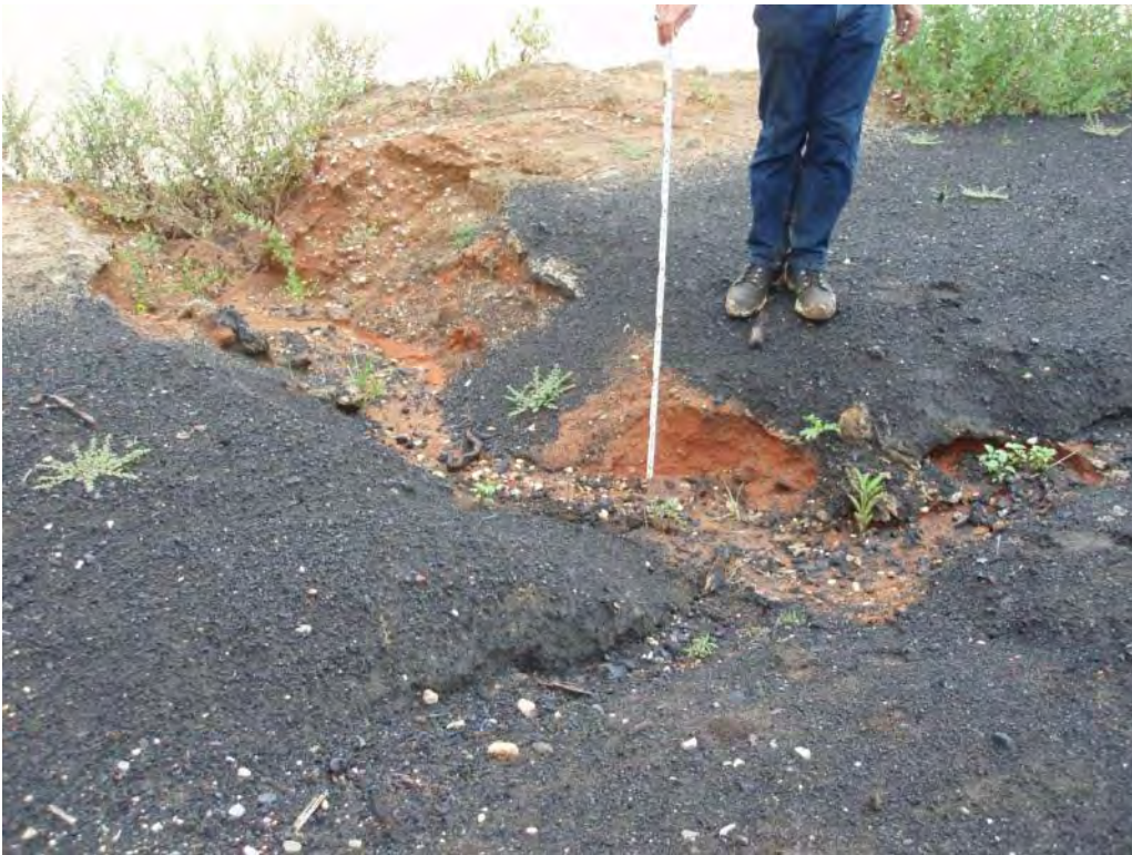
Photo No. 99: Scrubber Waste Pond – North embankment interior slope. Looking at erosion rill in fill material.
