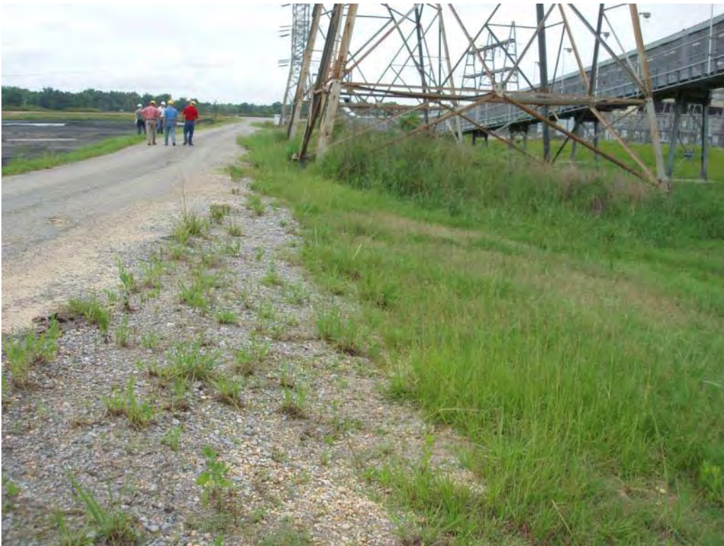
Photo No. 40: #1 Bottom Ash Pond – North embankment crest and exterior slope, looking west. Note transmission towers on slope.
