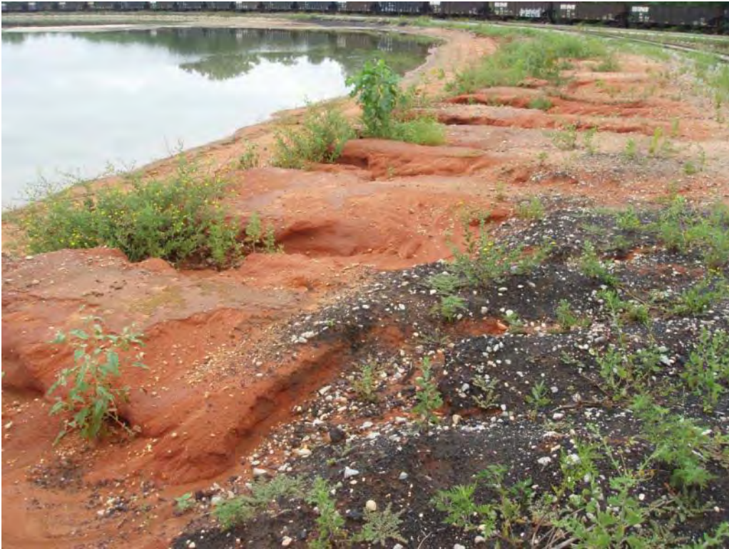
Photo No. 101: Scrubber Waste Pond – North embankment interior slope. Looking at erosion rills in fill material.
