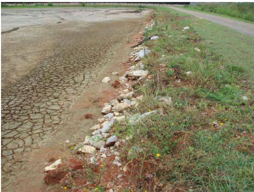
Photo No. 78: Scrubber Waste Pond – South embankment interior slope, looking east. Note surface erosion and sparse riprap.
