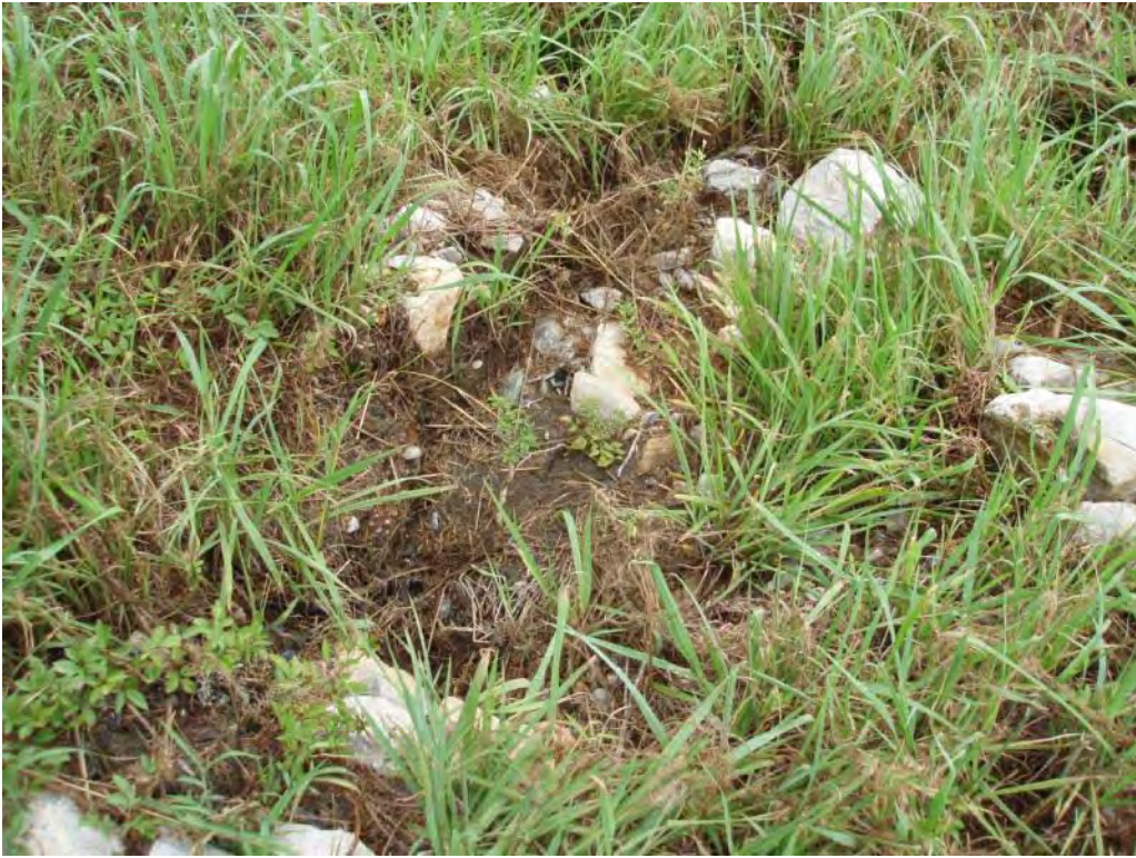
Photo No. 87: Scrubber Waste Pond – East embankment interior slope. Looking at surface erosion, sparse riprap and vegetation within riprap.
