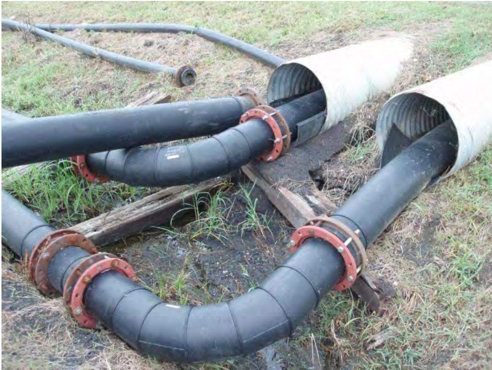
Photo No. 121: #2/#3 Bottom Ash Pond – East embankment exterior slope. Looking at piping used to divert Units 1, 2, & 3 CCW from the #1 Bottom Ash Pond into the #2/#3 Bottom Ash Pond.
