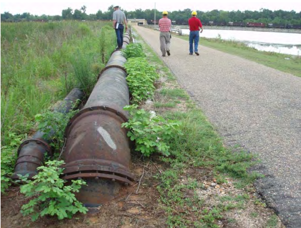
Photo No. 130: #2/#3 Bottom Ash Pond – North (divider) embankment interior slope and crest, looking west. Note vegetation around sluice lines.
