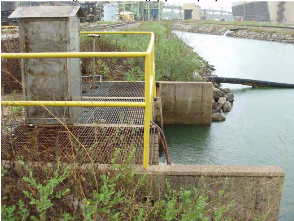
Photo No. 66: Process Waste Pond – South embankment interior slope, looking south. Looking at discharge from FGD (concrete structure) and second discharge pipe from pump station (HDPE pipe).
