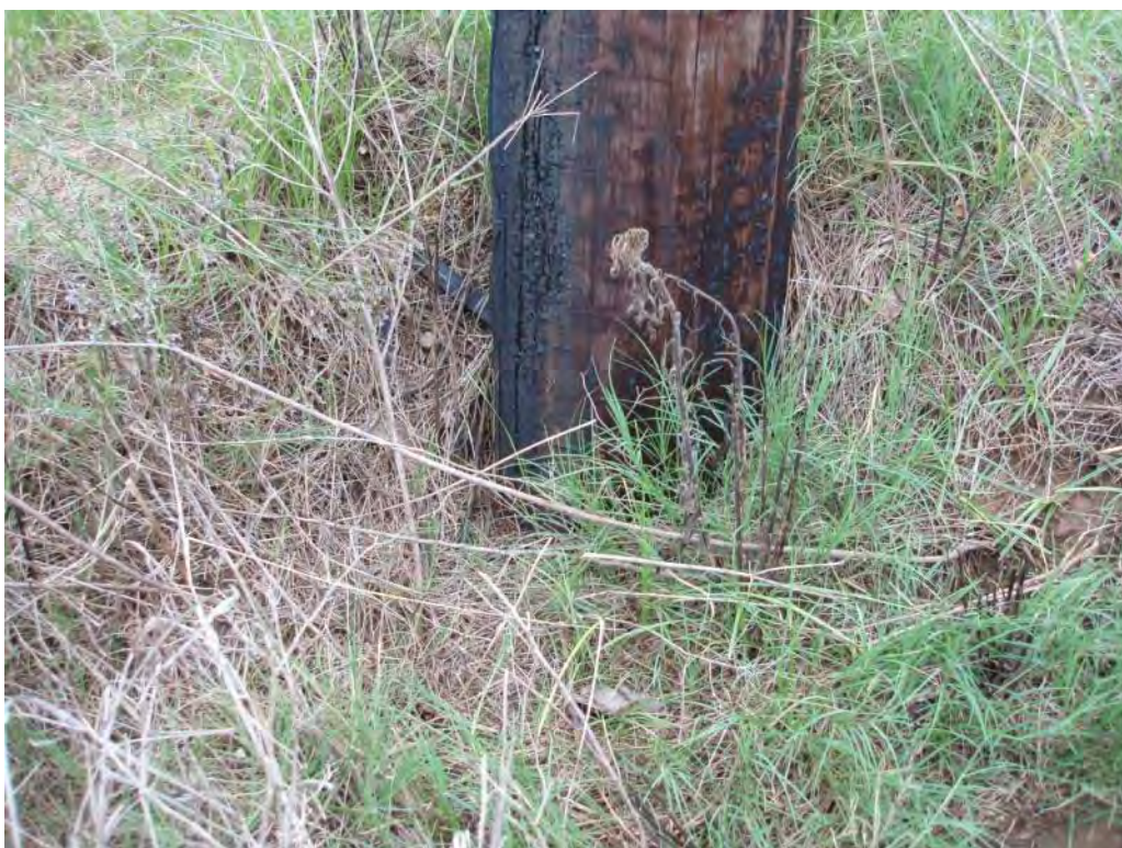
Photo No. 38: #1 Bottom Ash Pond – East embankment interior slope. Looking at eroded or missing soils near utility pole.
