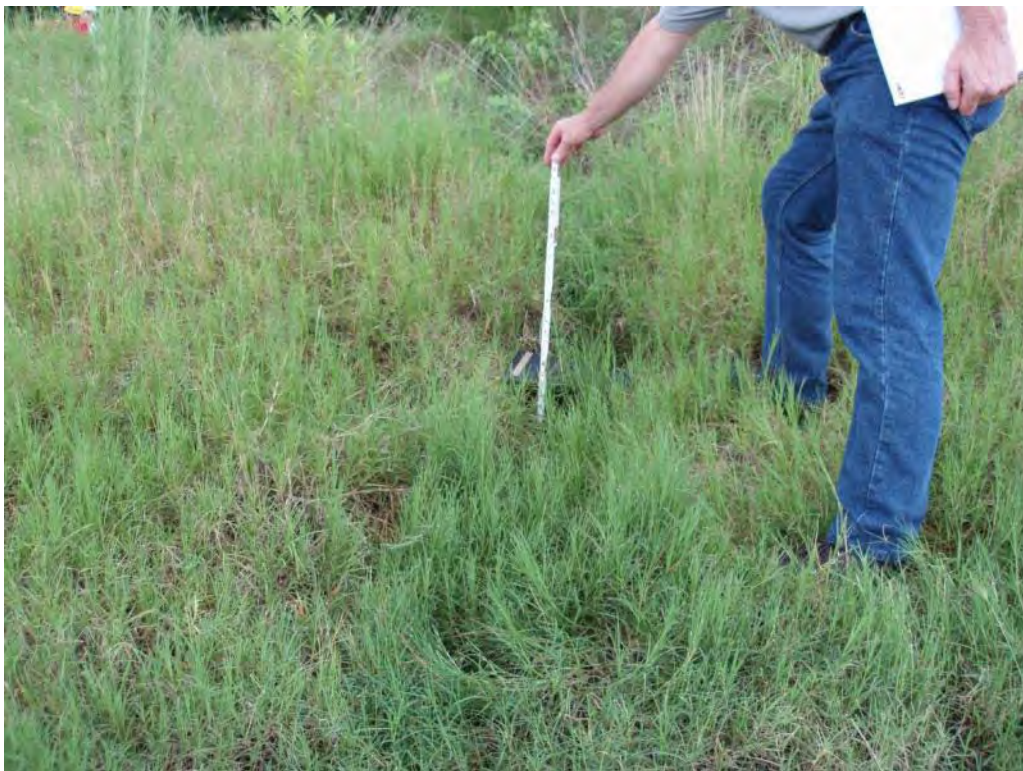
Photo No. 27: #1 Bottom Ash Pond – East embankment interior slope. Looking at minor erosion rills.
