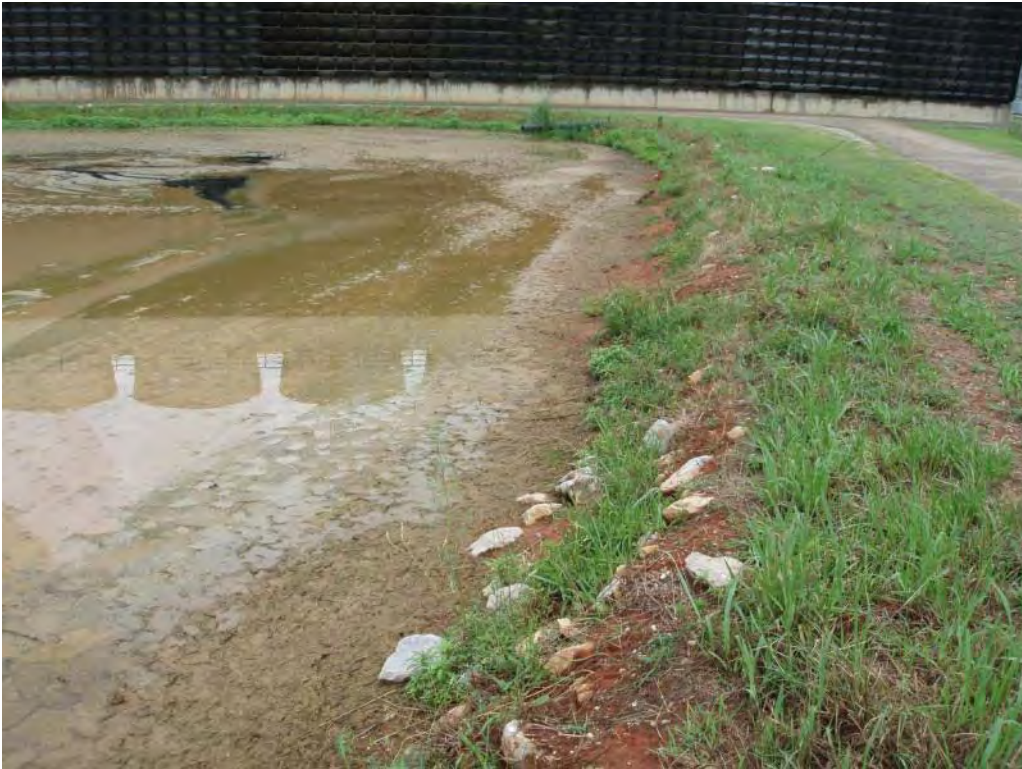
Photo No. 81: Scrubber Waste Pond – South embankment interior slope, looking east. Note sparse riprap and surface erosion.
