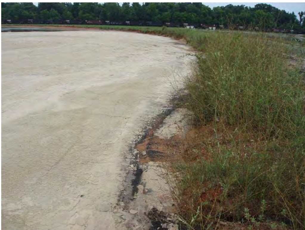
Photo No. 97: Scrubber Waste Pond – North (divider) embankment interior slope, looking west. Note ash product and vegetation on slope.
