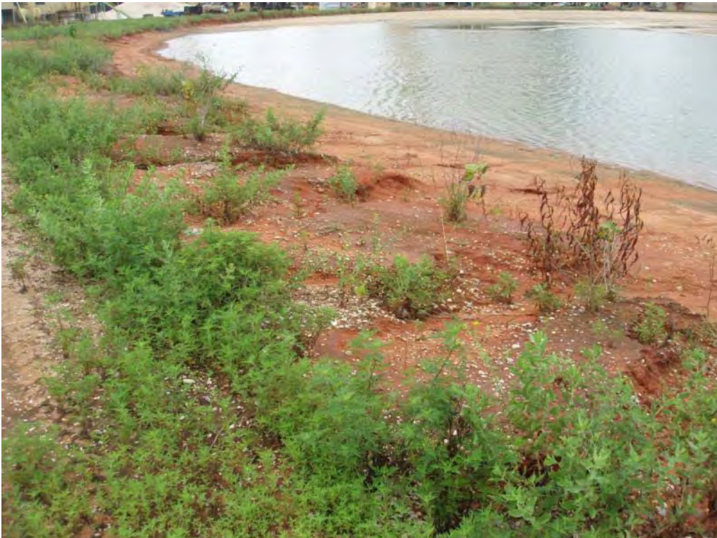
Photo No. 58: Process Waste Pond – South (divider) embankment exterior slope, looking southeast. Looking at erosion rills in fill material.
