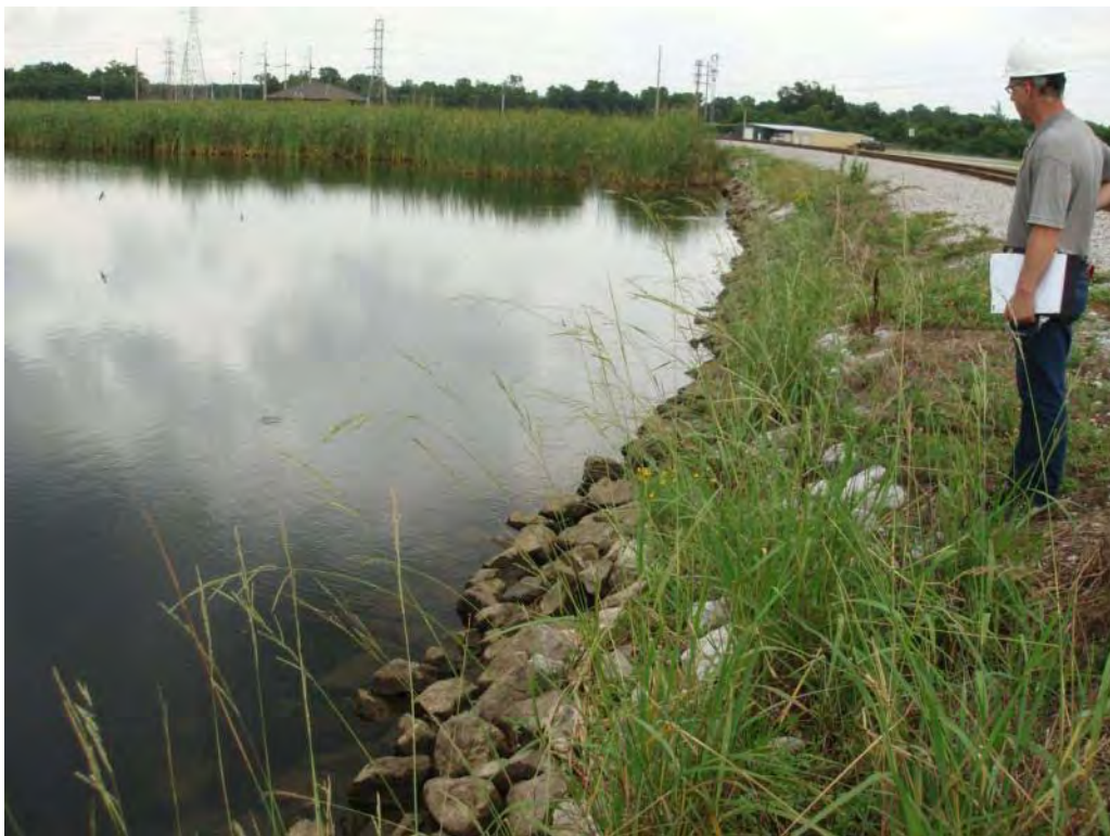
Photo No. 109: #2/#3 Bottom Ash Pond – South embankment interior slope, looking southeast. Note cattails growing within impoundment in background.
