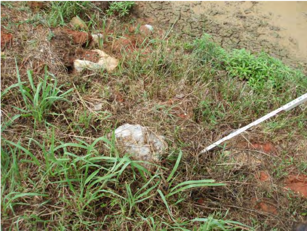
Photo No. 82: Scrubber Waste Pond – South embankment interior slope. Looking at 8-inch-deep void.
