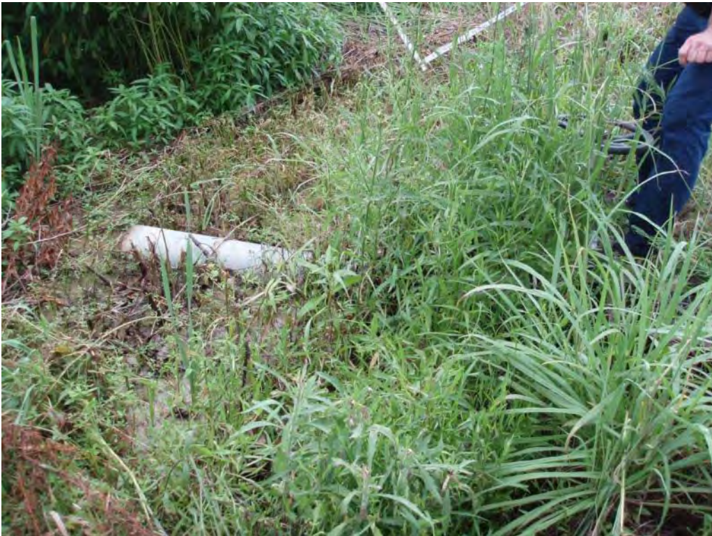
Photo No. 86: Scrubber Waste Pond – East embankment interior slope. Looking discharge pipe from cooling tower blowdown.
