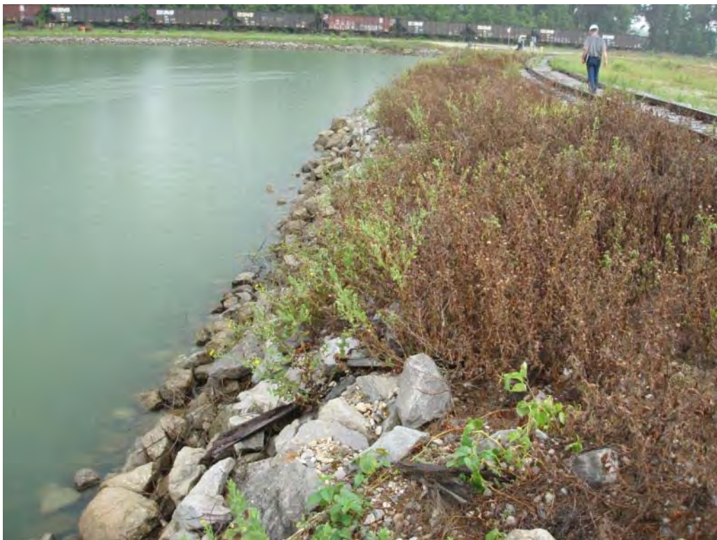
Photo No. 67: Process Waste Pond – North embankment interior slope, looking north. Note vegetation growing in riprap.
