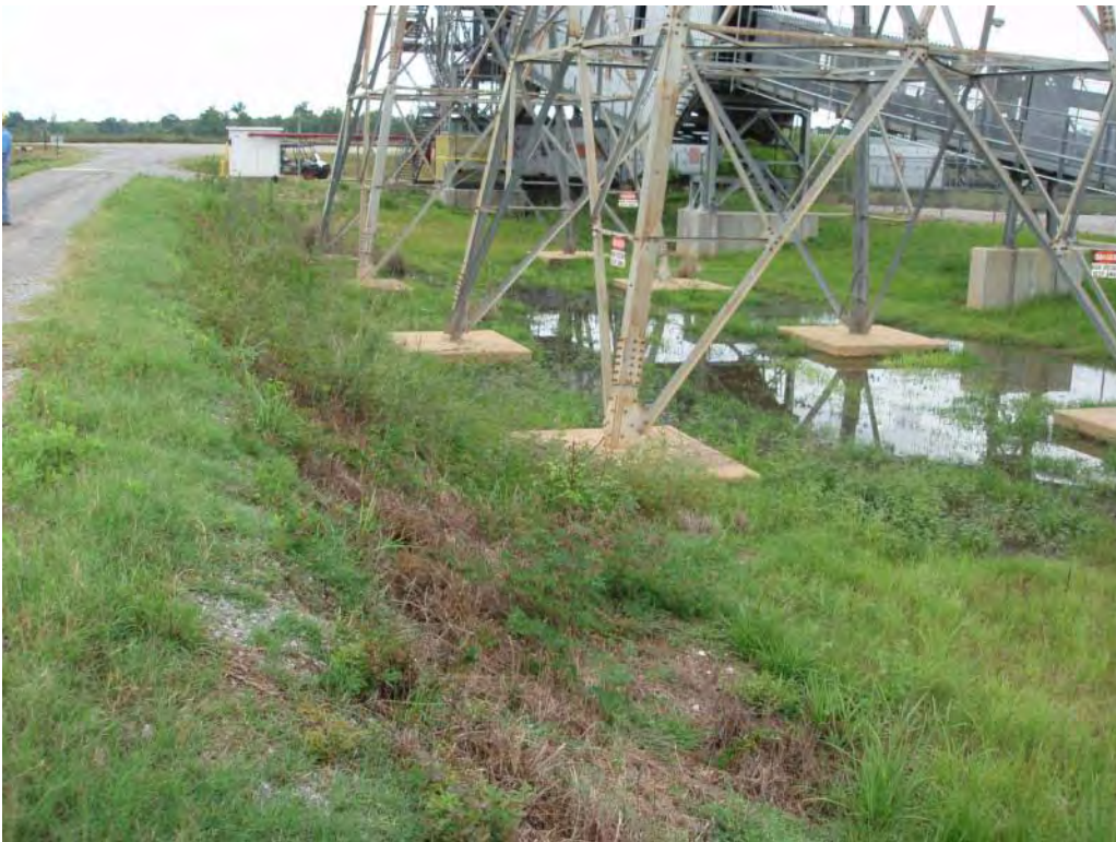
Photo No. 46: #1 Bottom Ash Pond - North embankment exterior slope, looking west. Note standing water near transmission tower base.
