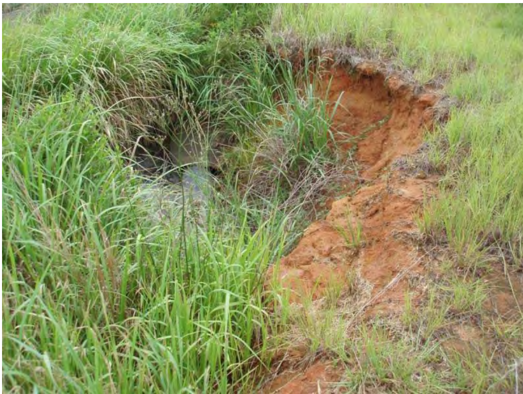
Photo No. 19: #1 Bottom Ash Pond – South embankment interior slope. Location of excavation into slope/crest and subsequent erosion.
