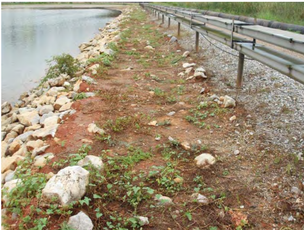
Photo No. 77: Scrubber Waste Pond – South embankment interior slope, looking east. Looking at location of spongy soils in area of buried pipeline.
