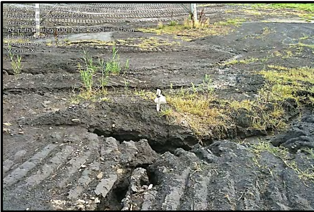
Photograph 5.9- Erosion Rills on Exterior Slope at Southeast Corner of Pond
