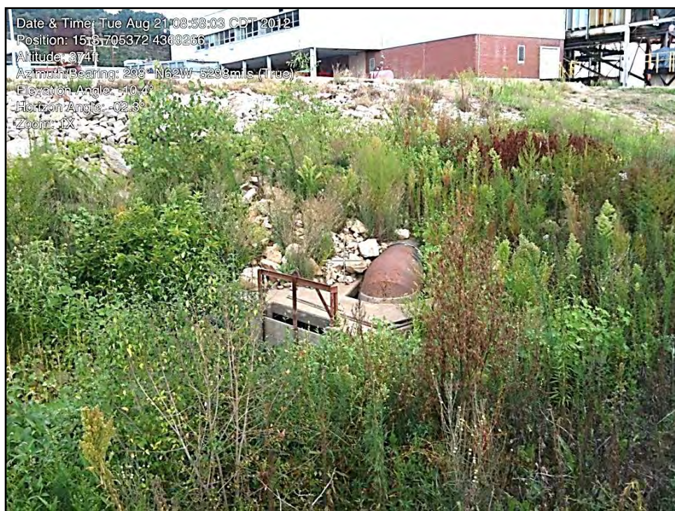
Photograph D.3. Plant Discharge into River
