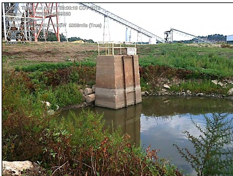
Photograph D.4. Intake to Plant from River
