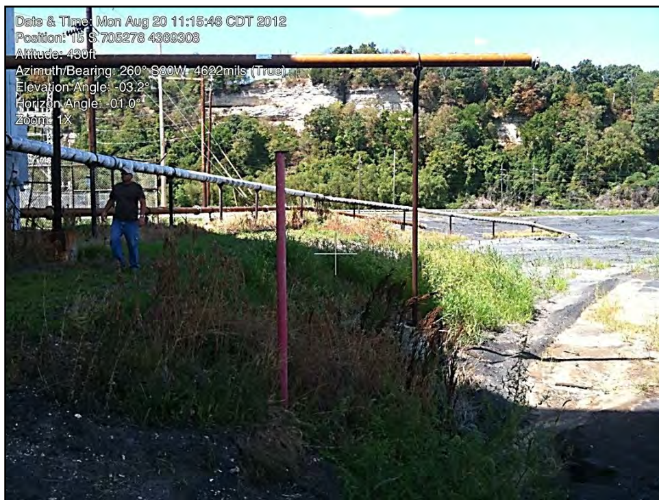
Photograph D.1. Interior Slope of South Embankment Showing Inlet Piping Looking West
