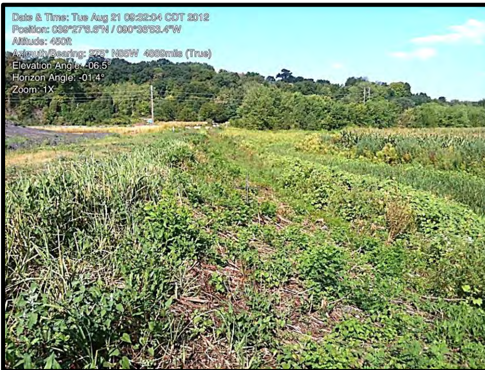
Photograph 5.8- Vegetation on Exterior Slope at Southeast Corner of Pond
