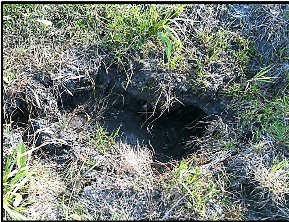
Photograph 5.6 - Erosion Feature on Interior Slope of South Embankment
