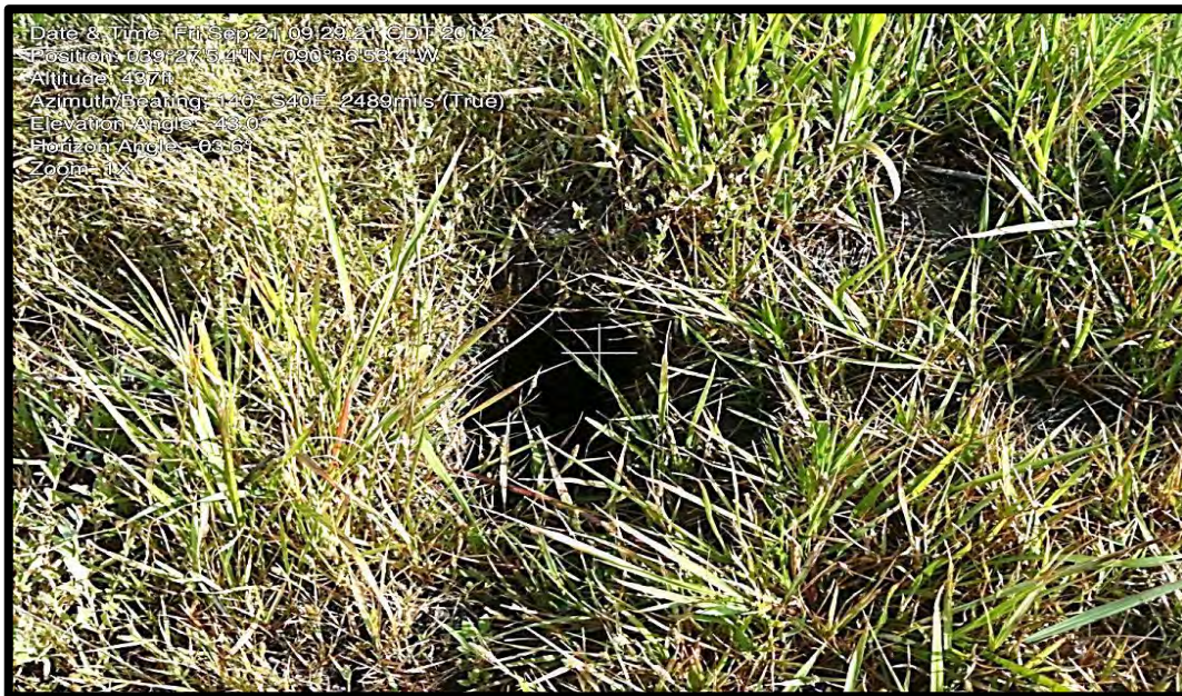
Photograph 5.5 - Animal Burrow on Interior Slope of East Embankment
