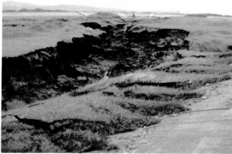
Photo 23 - A drainage ditch cut through the impoundment ash near the west embankment.
