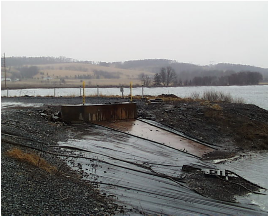
D48-149 New Concrete Pad & Headwall Structure – Ash Unloading Area on Right Side of 03/23/05 Upstream Face
