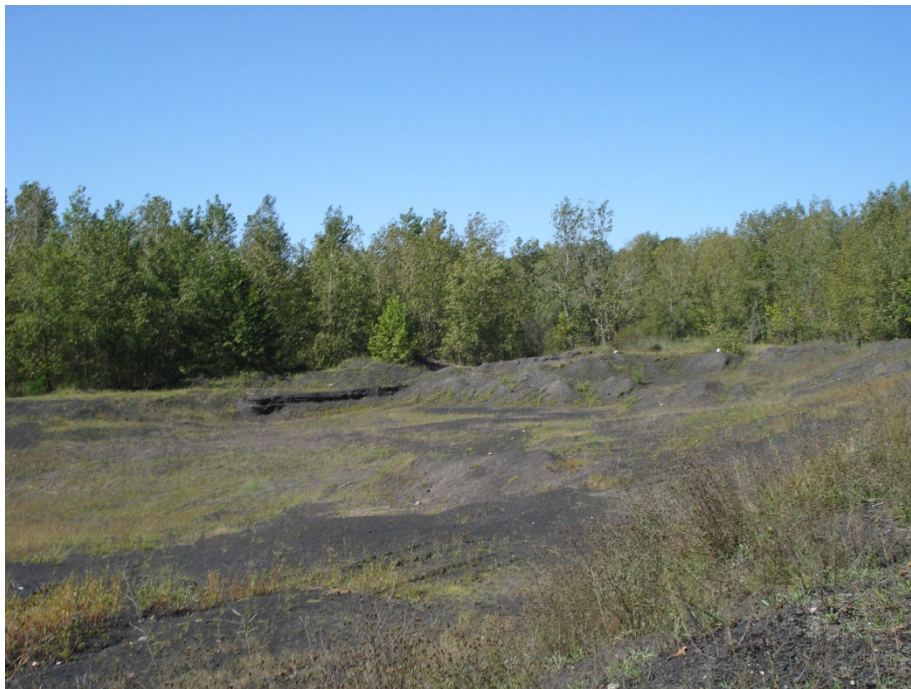
(Basin I) Berms to be Flattened Before Closure (black gravel=bottom ash; white objects are buckets), Martins Creek Power Plant, Bangor, PA, 09.01.09.
