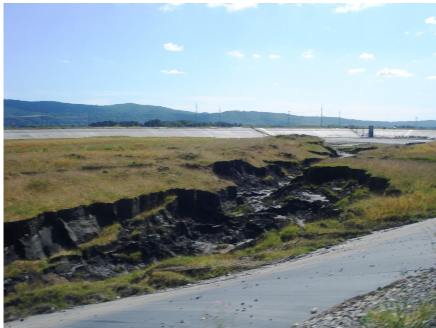
(Basin 4) Grass On Top of Coal Ash (nothing holding ash together, so subject to sloughing), Martins Creek Power Plant, Bangor, PA, 09.01.09.
