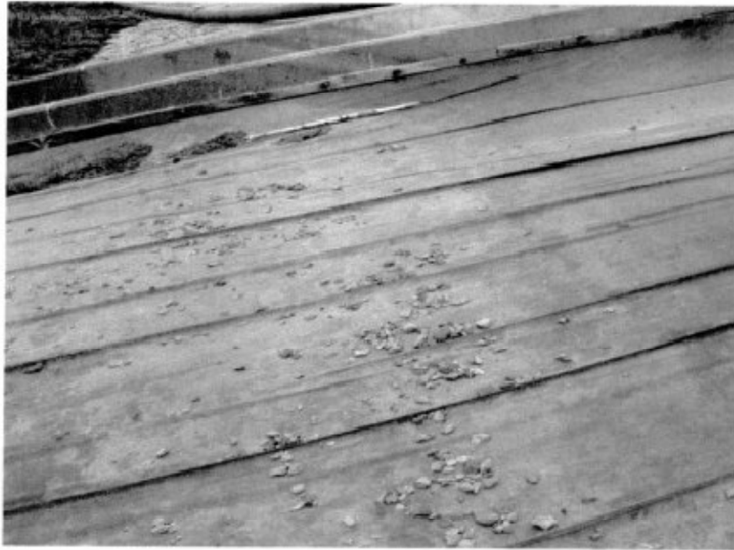
Photo 9 - Wrinkling of the upstream liner near the concrete loading ramp, Sta 13+50.
