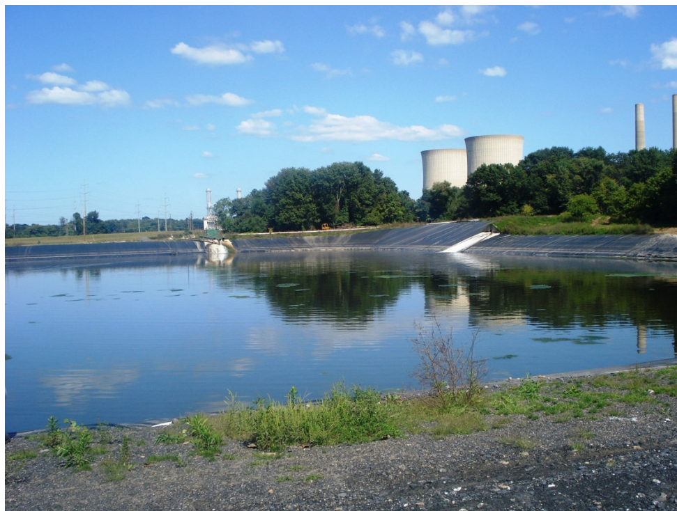
(IWTB) Inlets to Basin (far side is from cooling tower blowdown), Martins Creek Power Plant, Bangor, PA, 09.01.09.
