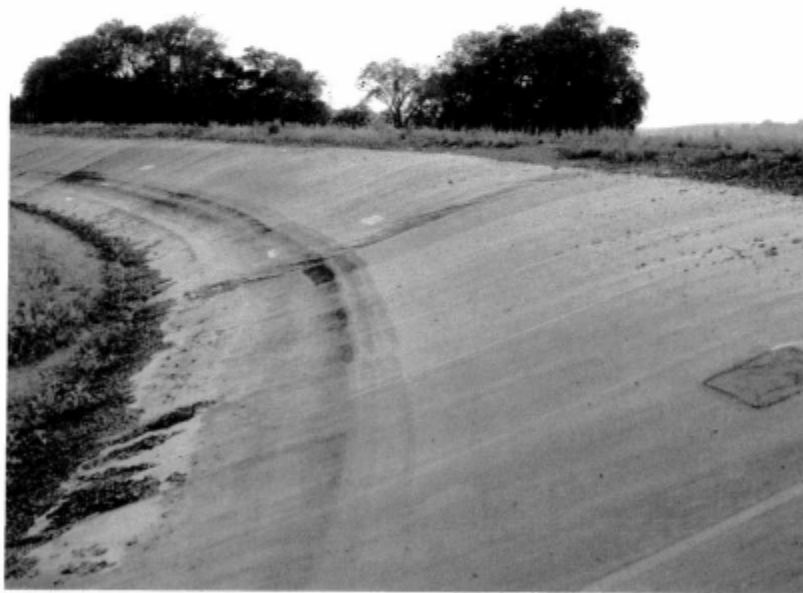
Photo 14 - Fabric wrinkle at northwest end of northeast embankment Sta 27+00.
