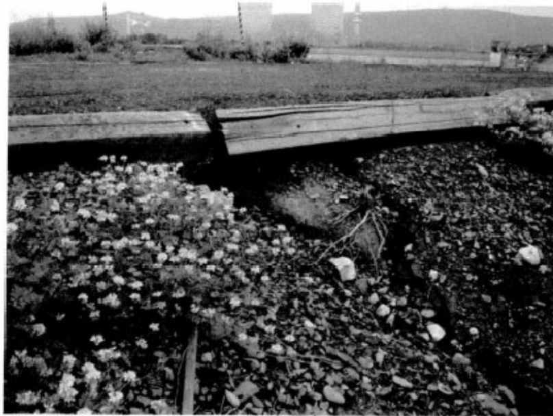
Photo 20 - Crest erosion near truck turnaround area on the southwest embankment.
