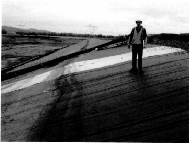
Photo 5 - Bulge in liner along upstream slope of east embankment, looking north from Sta 4+30.
