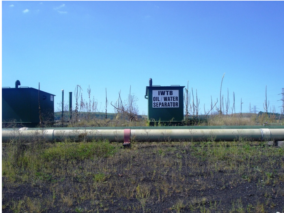
(IWTB) Oil Water Separator, Martins Creek Power Plant, Bangor, PA, 09.01.09.
