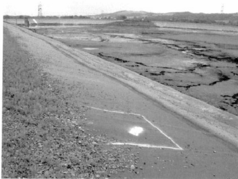
Photo 10 - Roadway gravel on top of liner.
