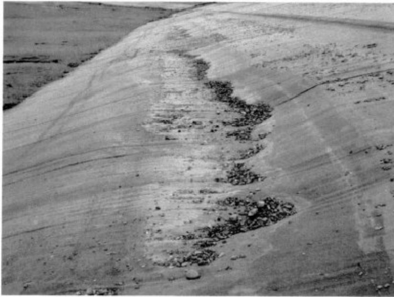
Photo 7 - Bulge in liner at Sta 9+75, looking north.
