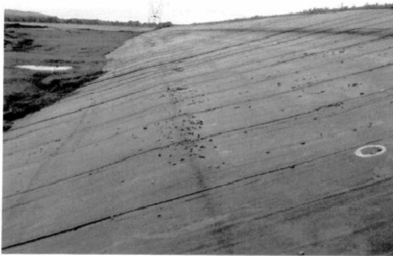
Photo 6 - Bulge in liner north of Station 8+00, looking north.
