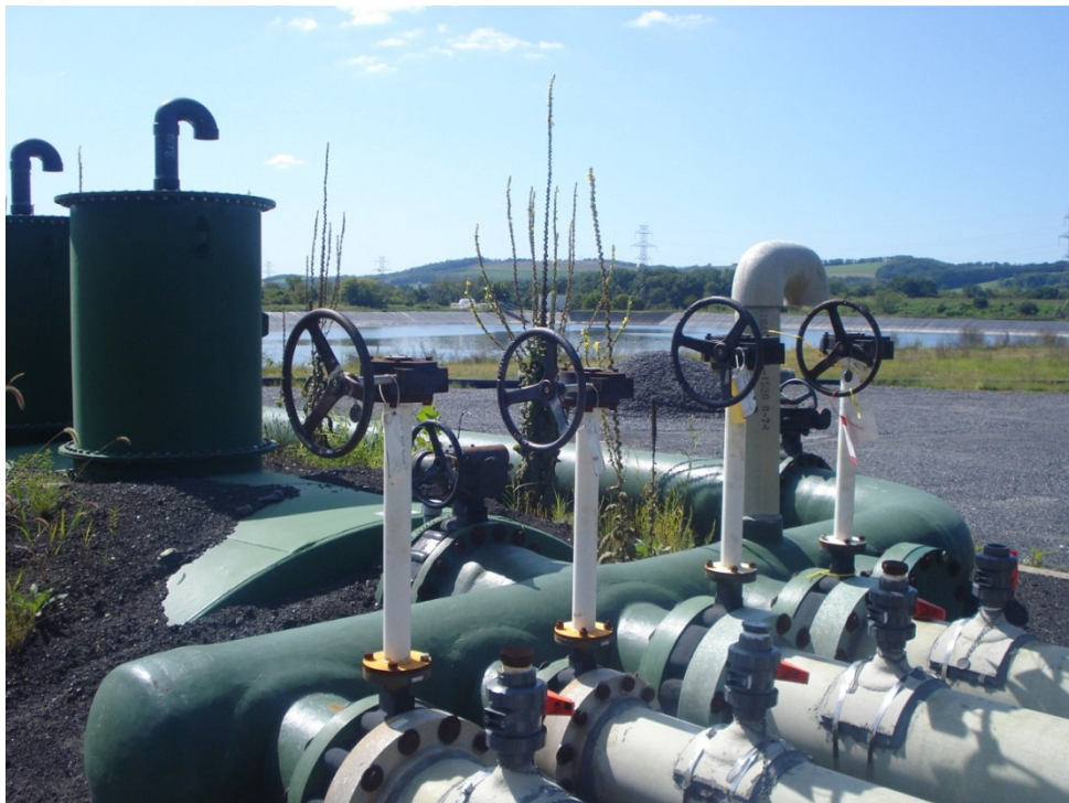
(IWTB) Oil Water Separator (with IWTB in background), Martins Creek Power Plant, Bangor, PA, 09.01.09.
