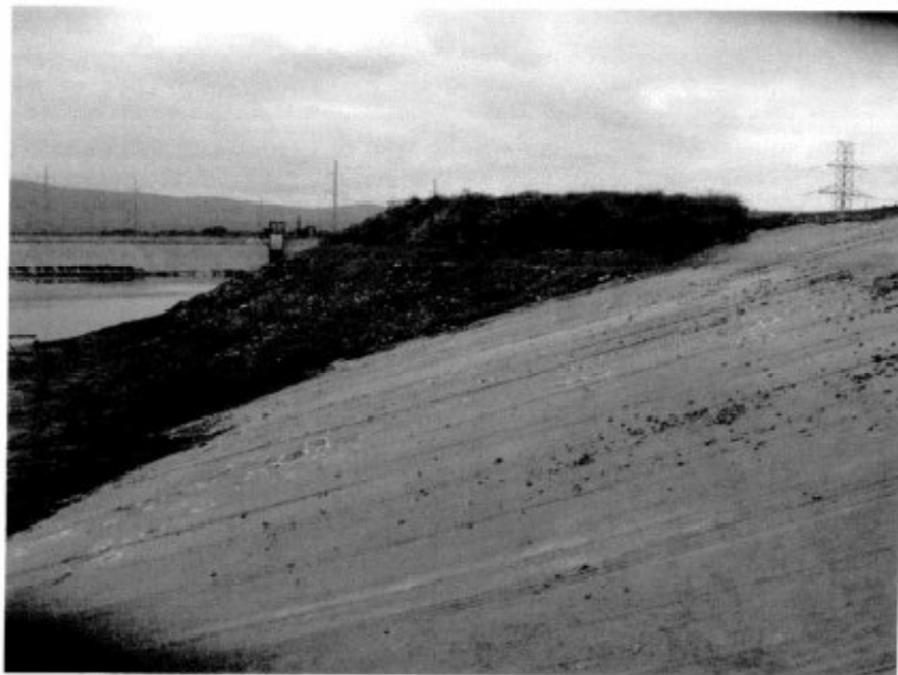
Photo 22 - Weathering and concentrated holes in liner north of truck turnaround on southwest embankment.
