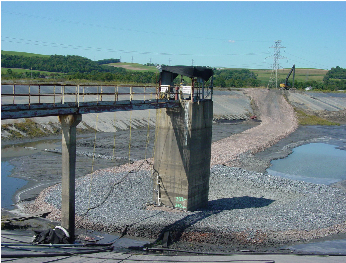
Photo B4-17: Ash Basin No. 4 View of East and North Sides of Decant Tower – Viewed Southwest Note Crushed Brick Access Causeway to Filter Around Base of Tower (Brick from Demolition of Smoke Stacks).
