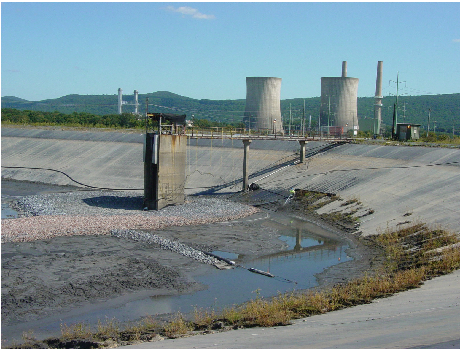
Photo B4-16: Ash Basin No. 4 View of South and West Sides of Decant Tower – Viewed Northeast Note Crushed Stone Filter Around Base of Tower.
