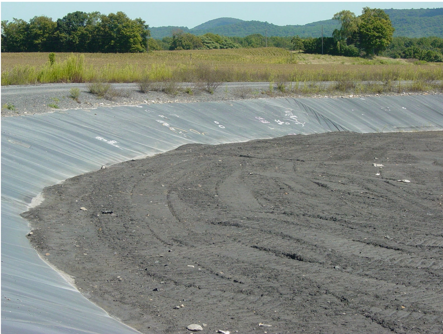
Photo B4-12: Ash Basin No. 4 Inside Slope of North Embankment at Northwest Corner – Note Highest Point of Ash in the Basin Spread in Place by Dozer in Preparation for Closure; White Marks on Liner from PPL Inspection Indicating Holes and Defects to be Patched.
