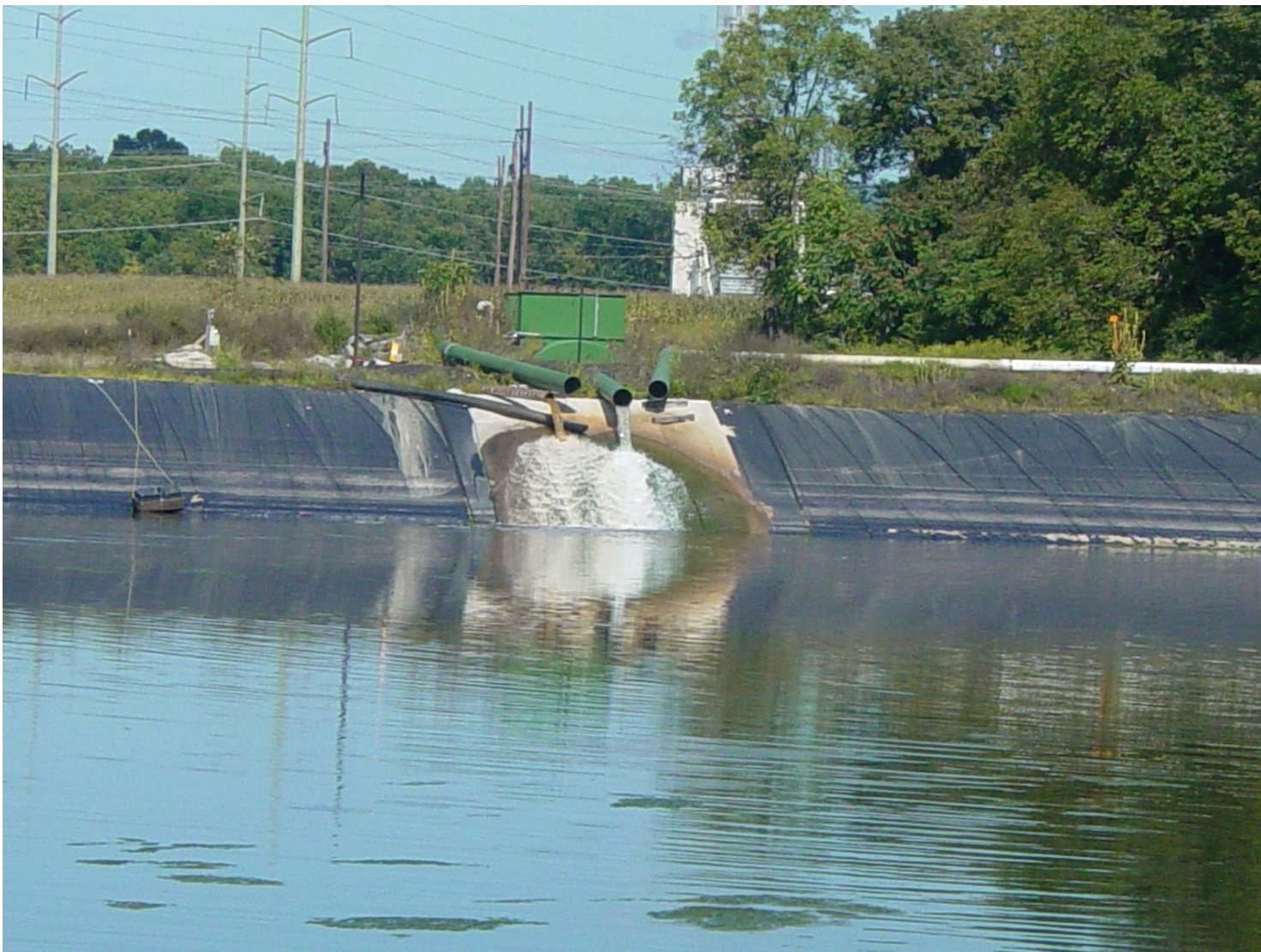
Photo I-4: IWTB North Incised Slope and Plant Drainage Discharge into Basin- Viewed North - Drainage Comes from both Martins Creek Power Plant via Oil/Water Separator (Green Fiberglass Pipes) and Lower Mt. Bethel Power Plant (Brown Fiberglass Pipe); Drainage also Comes from Ash Basin No. 4 (Black HDPE Pipe).
