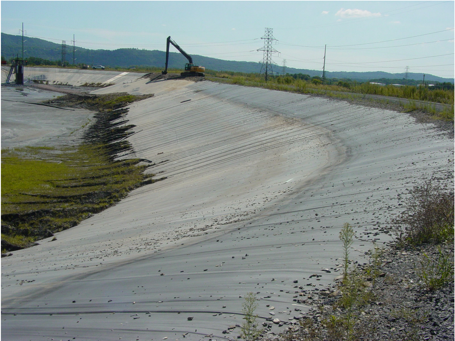
Photo B4-15: Ash Basin No. 4 Inside Slope of South Embankment – Viewed Southeast – Note Vertical Wrinkles.
