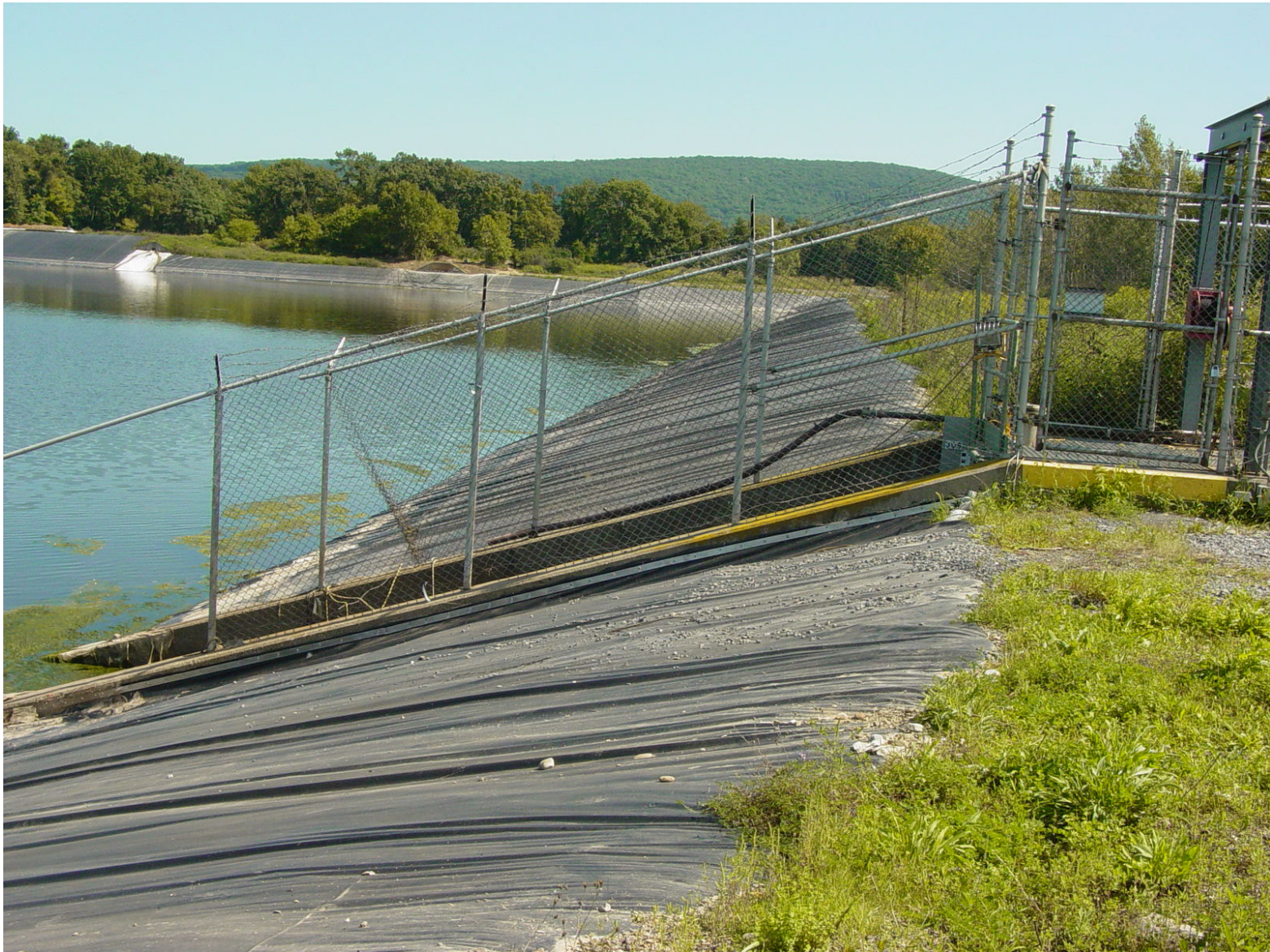
Photo I-2: IWTB South Incised Slope with Outlet Structure in Foreground – Viewed East – Note Vertical Wrinkles in Liner.
