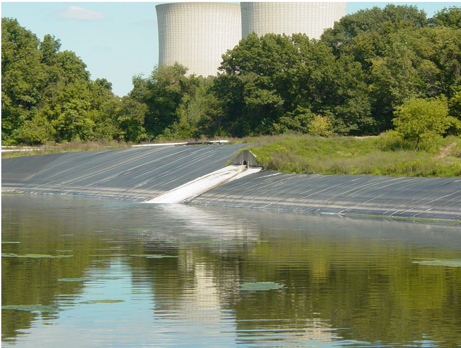
Photo I-3: IWTB East Incised Slope and Cooling Tower Blow-down Discharge into Basin - Viewed Northeast- Note Liner Extends Higher on North Half to Cover former Sinkhole Area in Shallow Rock.
