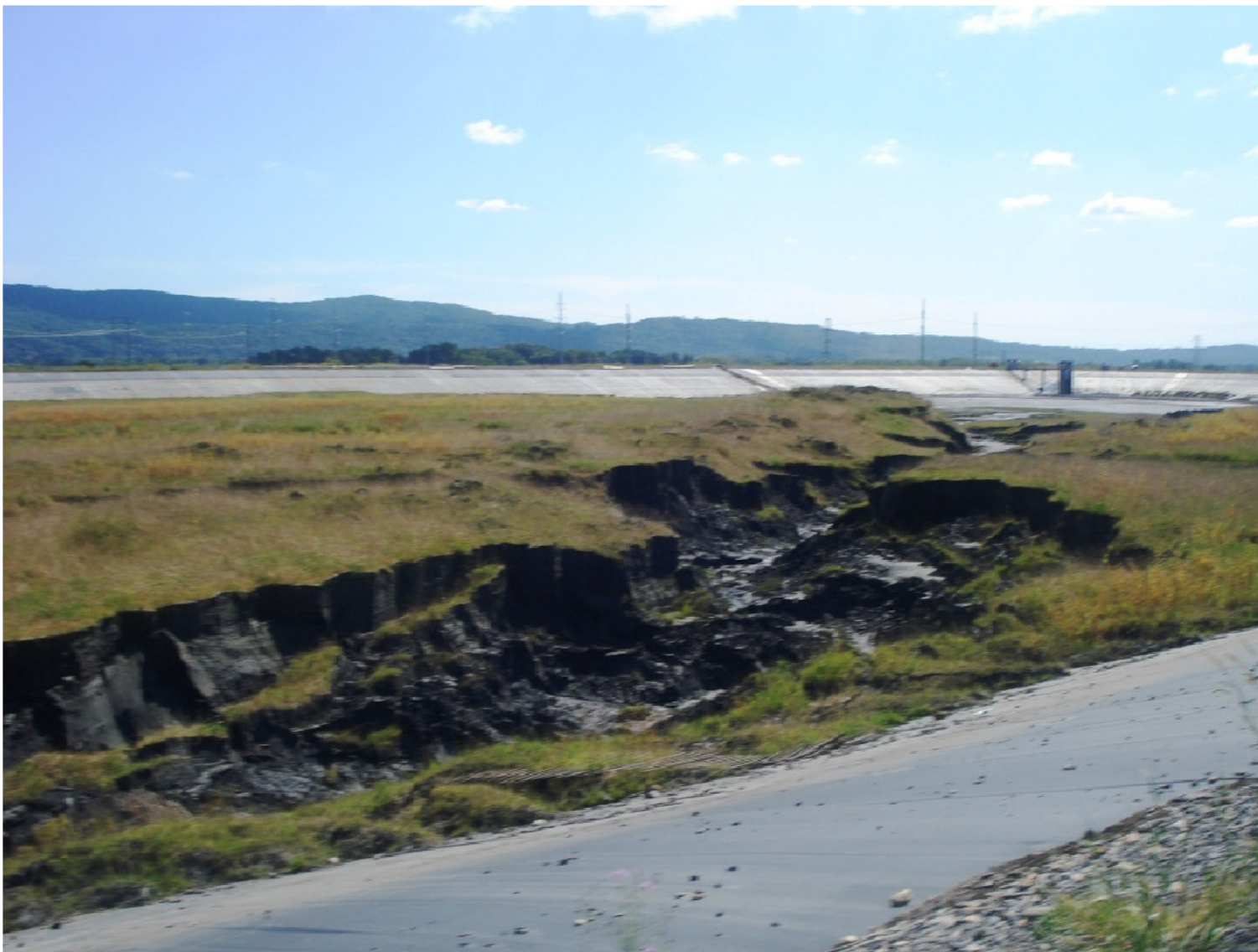
Photo B4-14: Ash Basin No. 4 View of Swale Cut Through Ash to Allow Drainage from West Part of Basin – Note Sloughing and Erosion of the Side Slopes of the Swale.
