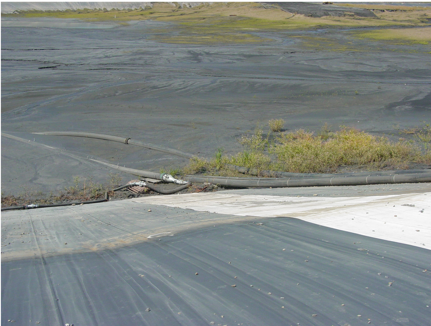
Photo B4-10: Ash Basin No. 4 View of Slight Linear Bulge Under Liner along Former Operating Water Level on Inside Slope of East Embankment Approximately 430' North of Decant Tower Footbridge.
