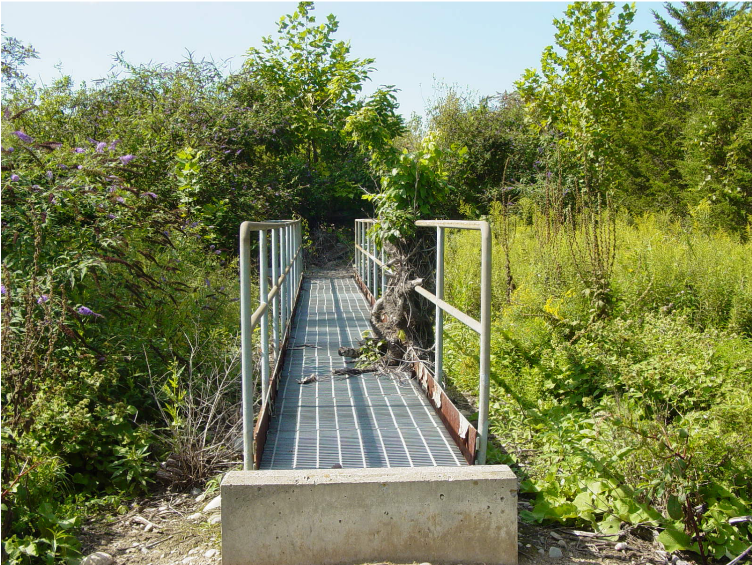
Photo B2-1: View of former Footbridge to North Decant Tower at Ash Basin No. 2 – Viewed West – Note Dense Vegetation on the Soil Cover over the Closed Basin.
