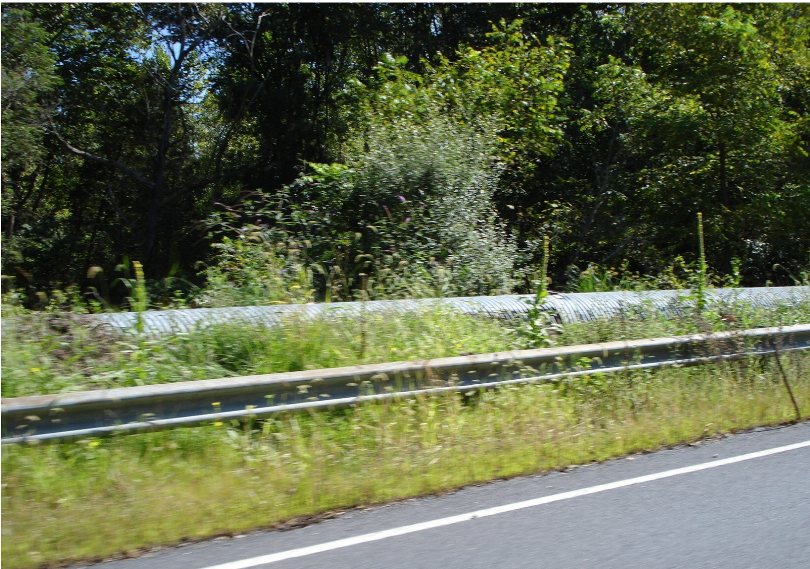
Photo B2-5: View of Above Ground 42" CMP Discharge Line from Combining Structure to Outfall Near the Delaware River.
