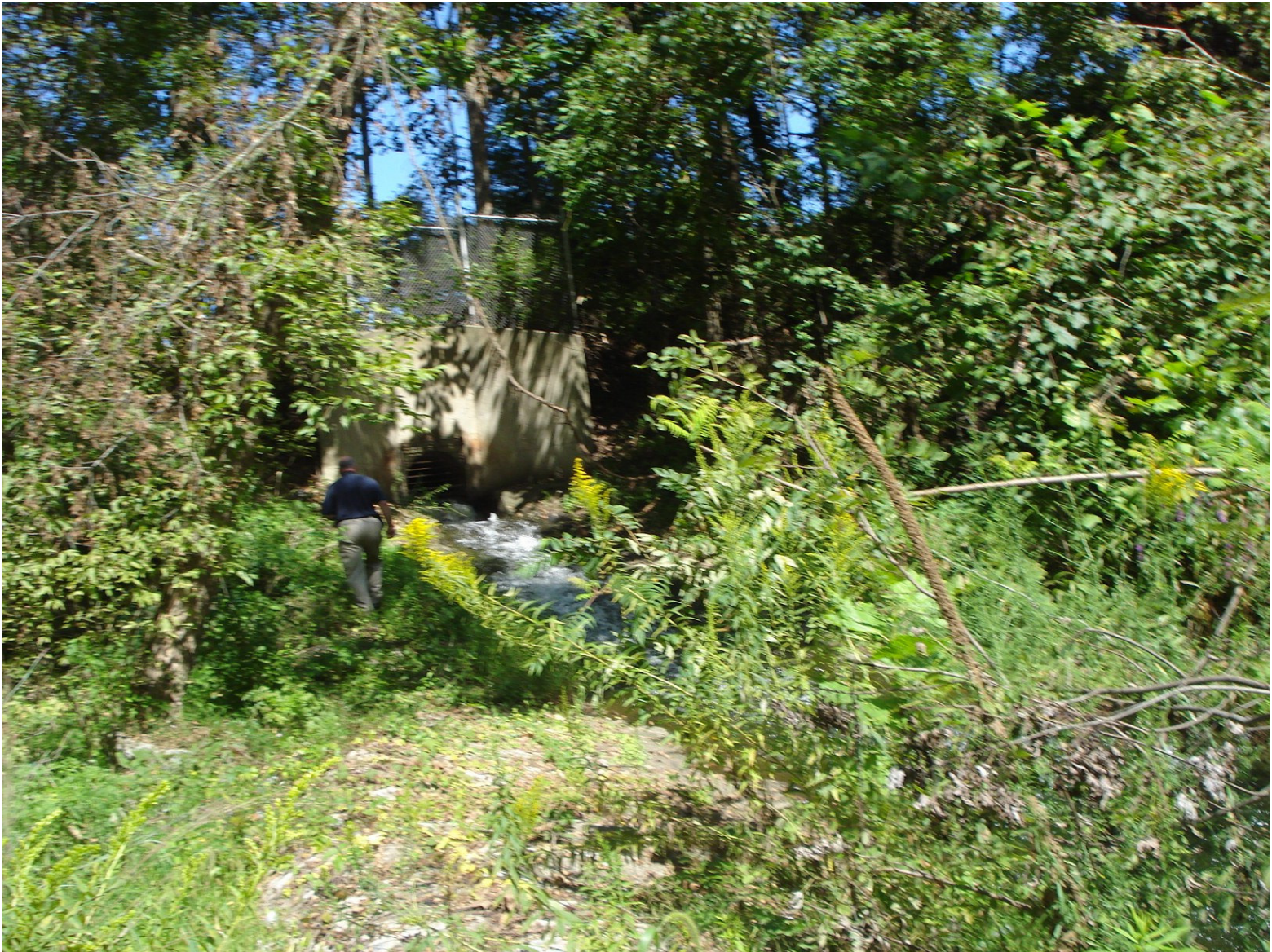
Photo B2-6: View of Outfall of 42" CMP Discharge Line into Grouted Riprap Channel to the Delaware River.
