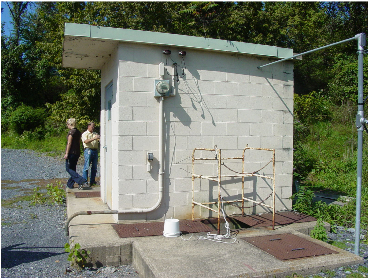
Photo B2-3: View of NPDES Monitoring Control Building at Combining Structure, which is a Below-grade Concrete Basin with Outflow Weir for Measuring Total Discharge from the Plant; Steel Plates Cover Top of the Basin for Safety- Note Bucket for Grabbing Water
