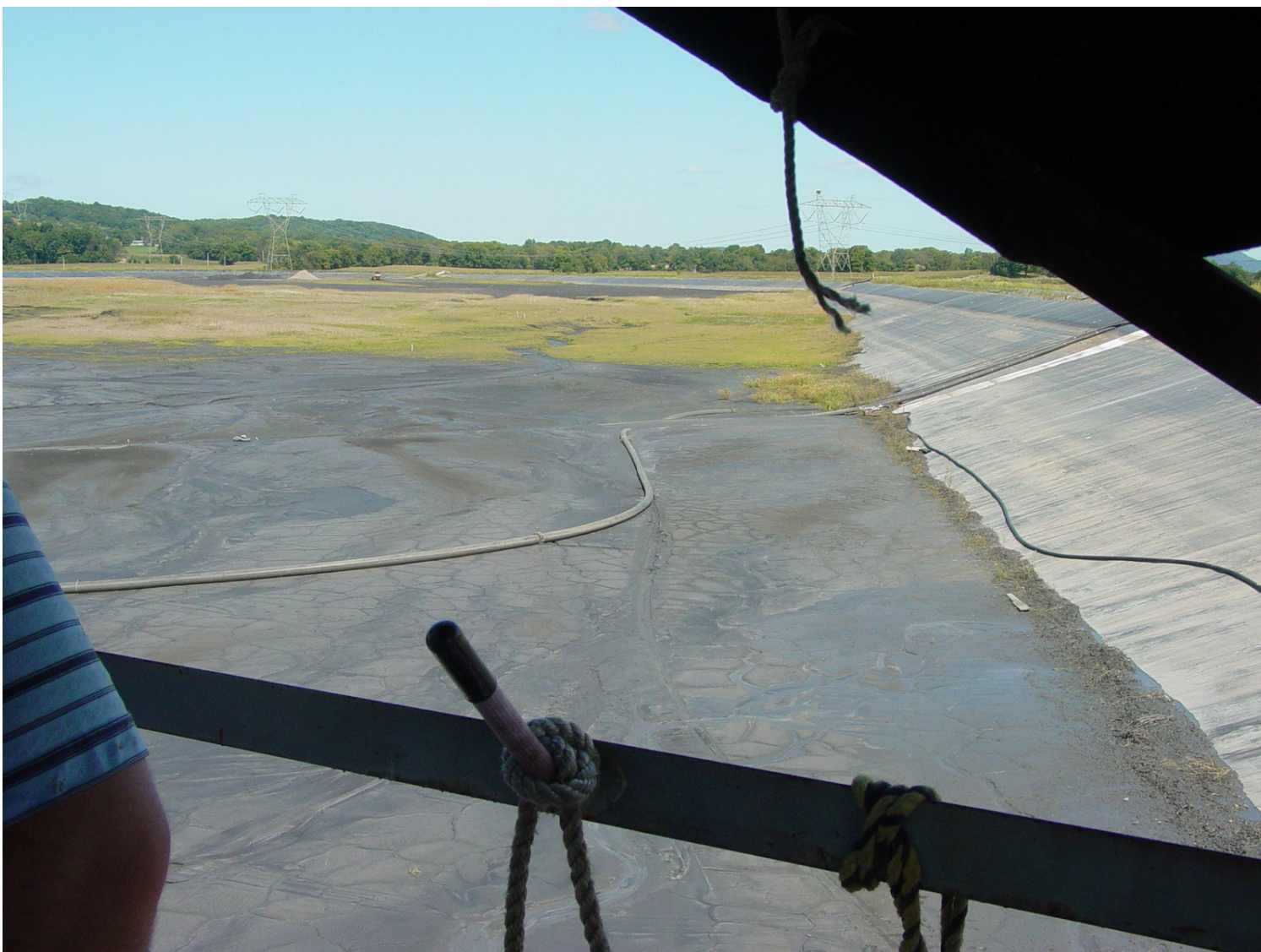
Photo B4-9: Ash Basin No. 4 Inside Slope of East Embankment and View of Ash Surface in Basin- Viewed North from Top of Decant Tower - Note Vertical Wrinkles in Liner (Commonly Occurs Throughout).
