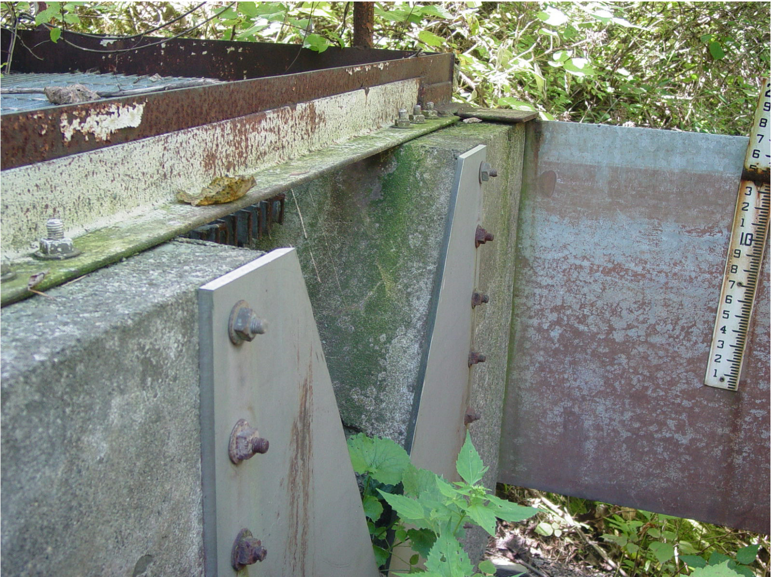
Photo BI-12: Ash Basin No. 1 V-Notch Weir at Top West Side of 4-foot Diameter RCP Outlet Standpipe.
