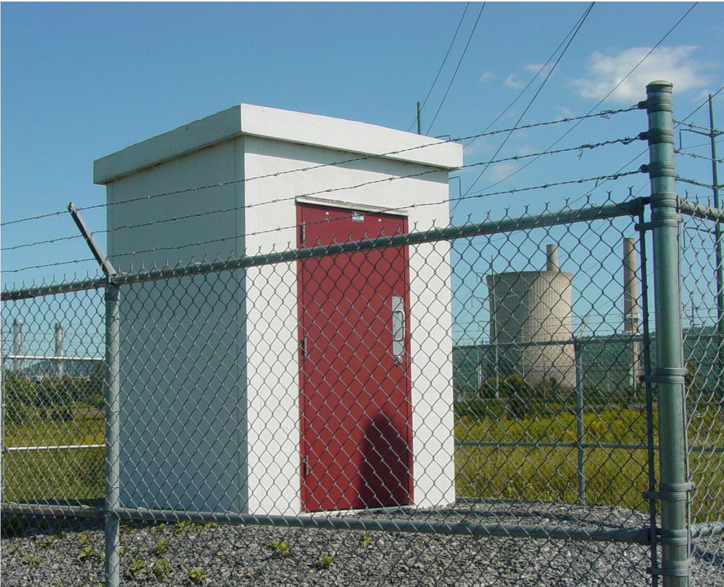
Photo B4-20: Ash Basin No. 4 View of Building Housing Operator for New Gate Valve in Underlying Concrete Vault.
