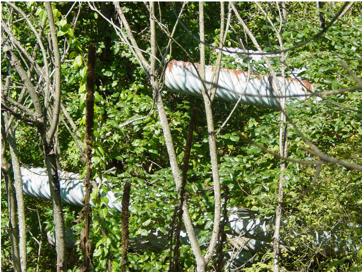
Photo BI-7: Ash Basin No. 1 View of Discharge End of 12" CMP Drains through Main Cross Dike that Divides the Higher Northern Two-Thirds of the Basin from the Lower Southern One-Third.
