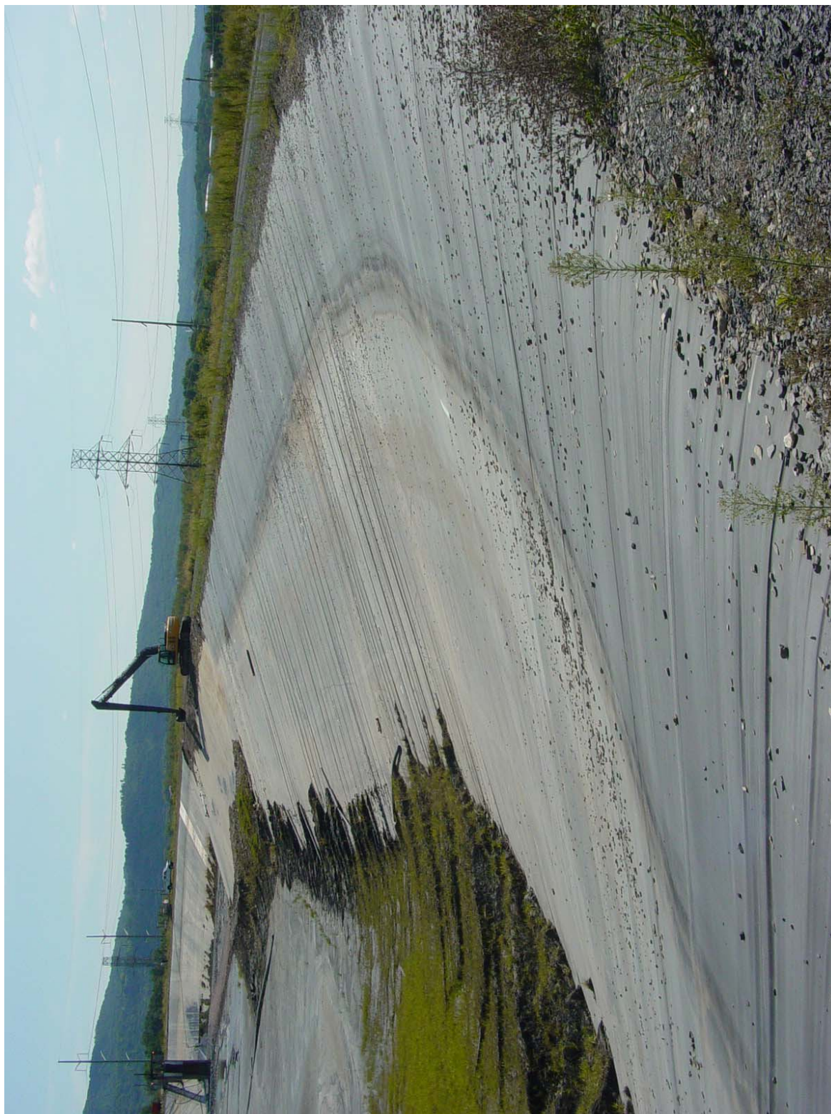
Photo B4-15: Ash Basin No. 4 Inside Slope of South Embankment – Viewed Southeast – Note Vertical Wrinkles.
