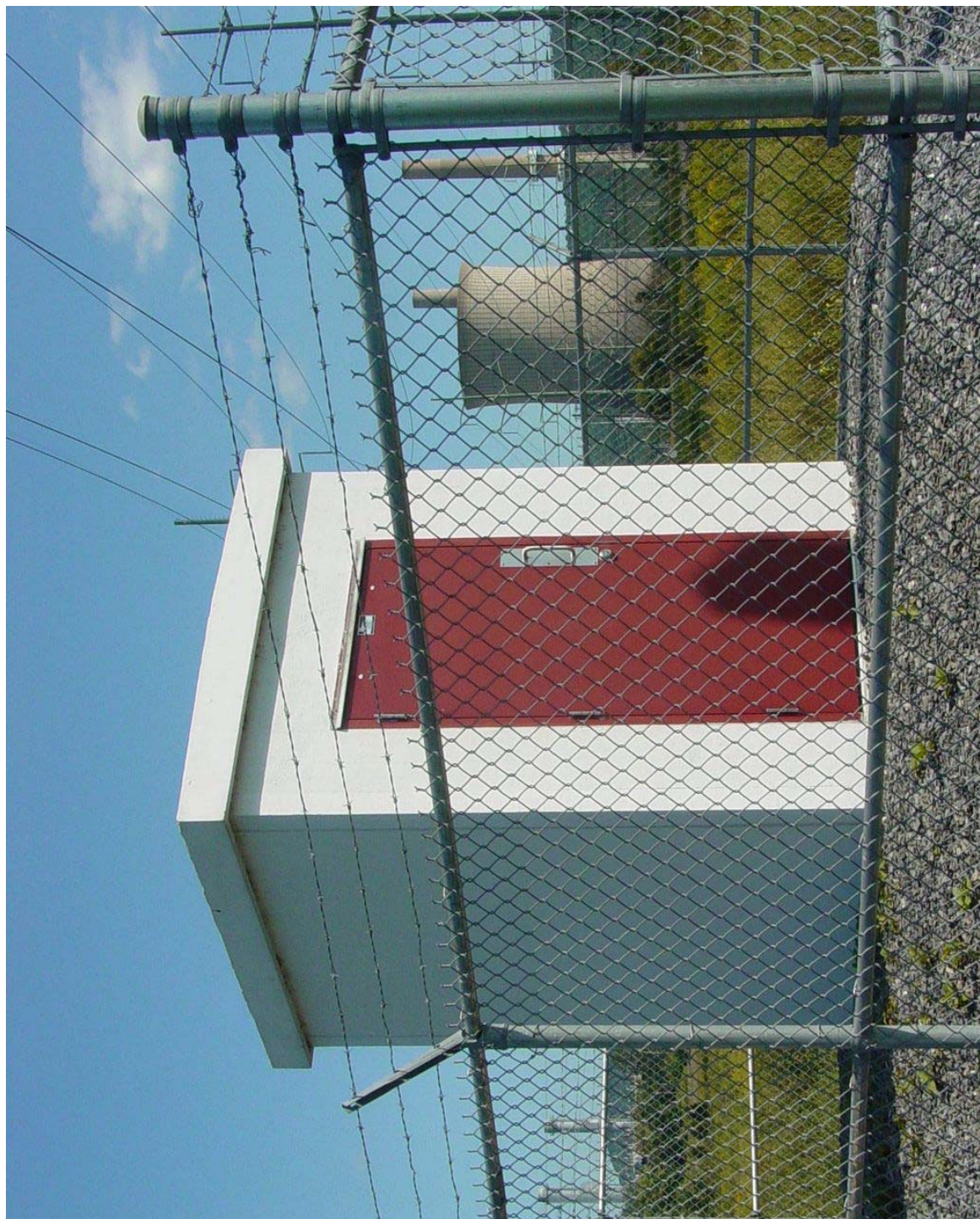
Photo B4-20: Ash Basin No. 4 View of Building Housing Operator for New Gate Valve in Underlying Concrete Vault.
