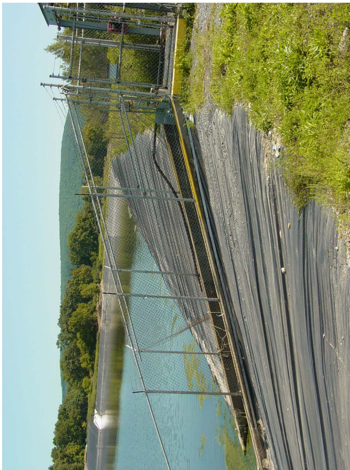
Photo I-2: IWTB South Incised Slope with Outlet Structure in Foreground – Viewed East – Note Vertical Wrinkles in Liner.
