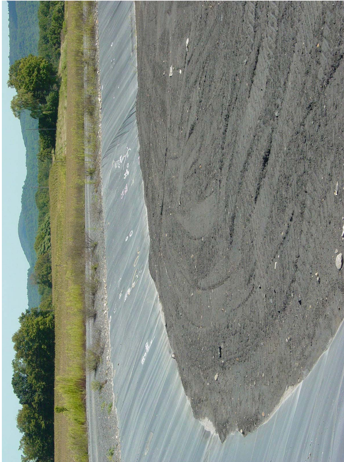
Photo B4-12: Ash Basin No. 4 Inside Slope of North Embankment at Northwest Corner – Note Highest Point of Ash in the Basin Spread in Place by Dozer in Preparation for Closure; White Marks on Liner from PPL Inspection Indicating Holes and Defects to be Patched.
