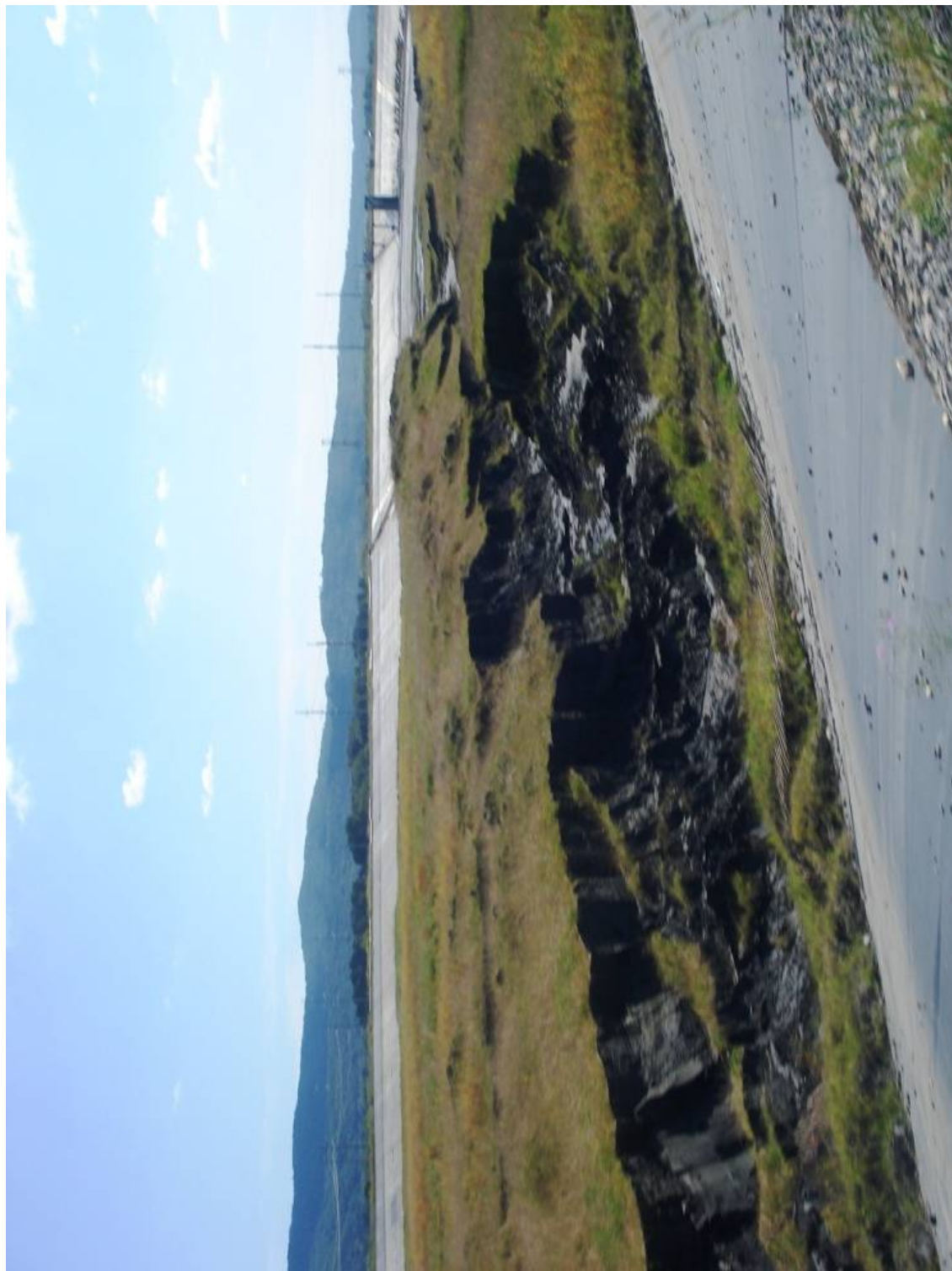
Photo B4-14: Ash Basin No. 4 View of Swale Cut Through Ash to Allow Drainage from West Part of Basin – Note Sloughing and Erosion of the Side Slopes of the Swale.
