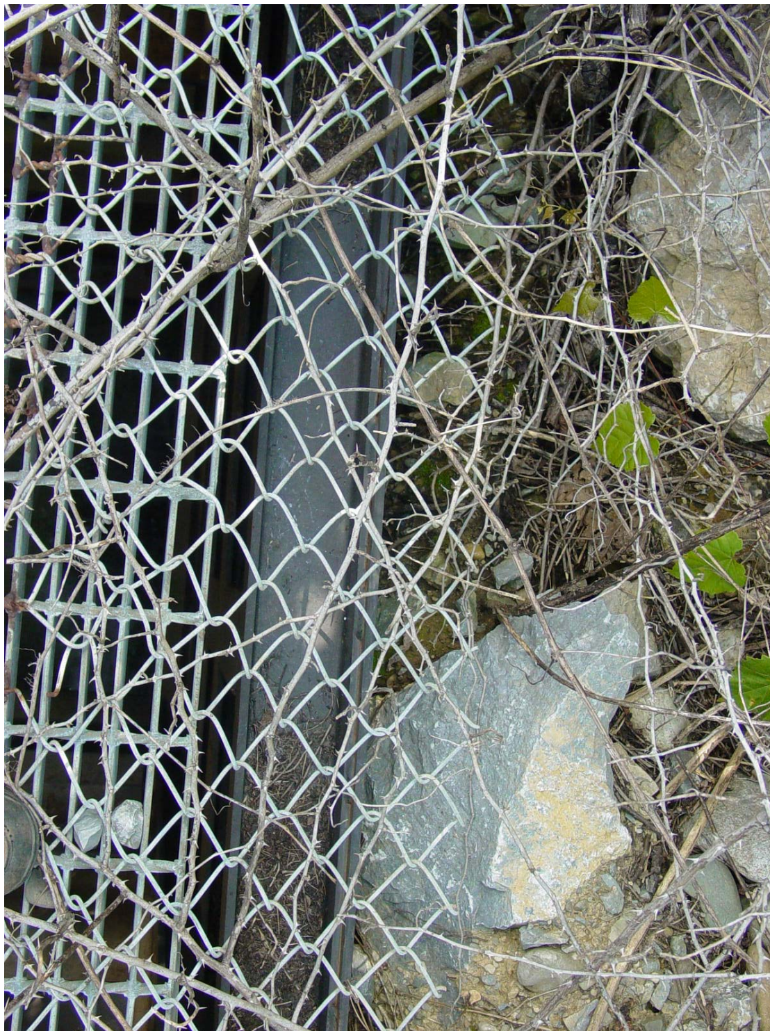
Photo B2-2: View of Top of Reinforced Steel Plate Bulkhead that Seals off the Wood Stop Log Side of the North Decant Tower at Ash Basin No. 2 – This and Two other Drainage Towers at the Closed Basin No. 2 are used for Drainage from the IWTB to the
