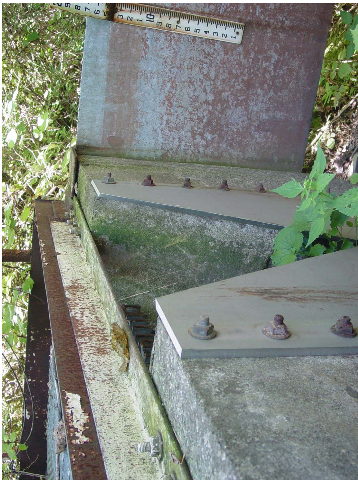
Photo BL-12: Ash Basin No. 1 V-Notch Weir at Top West Side of 4-foot Diameter RCP Outlet Standpipe.
