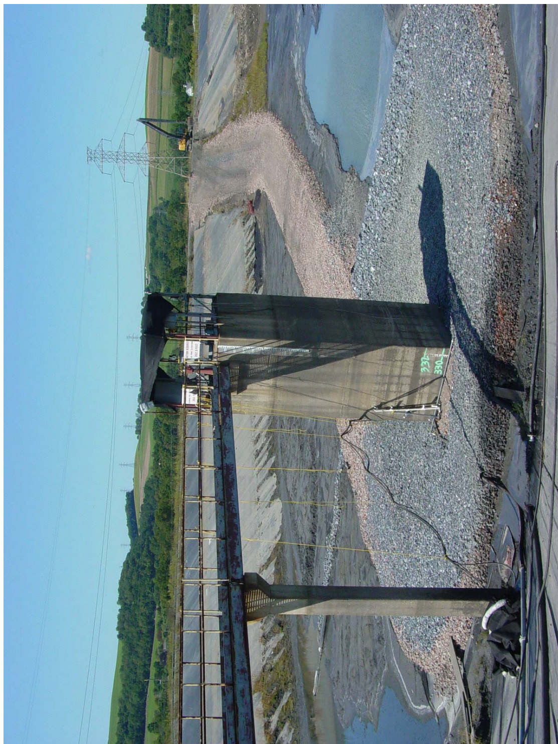
Photo B4-17: Ash Basin No. 4 View of East and North Sides of Decant Tower – Viewed Southwest Note Crushed Brick Access Causeway to Filter Around Base of Tower (Brick from Demolition of Smoke Stacks).
