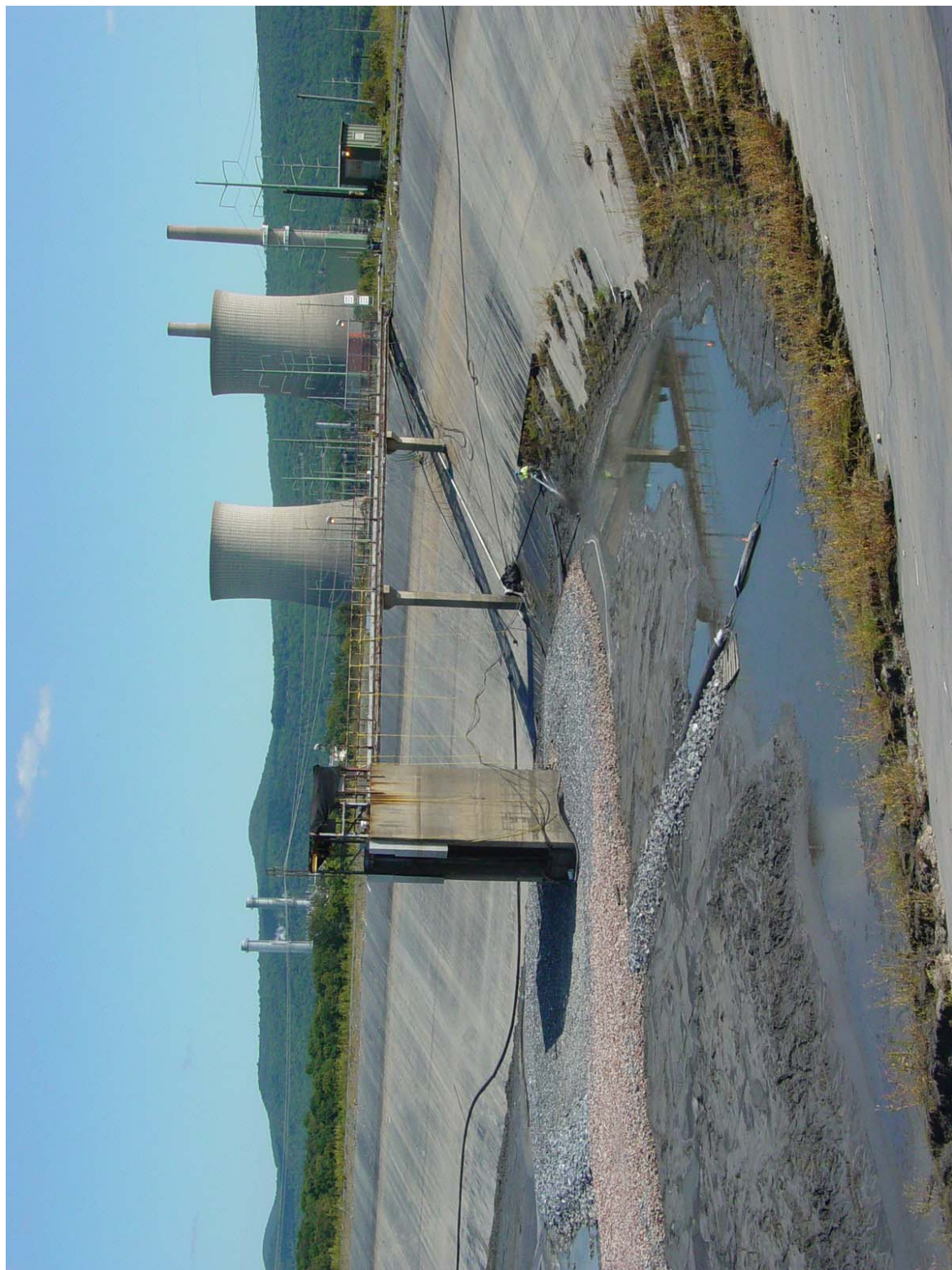
Photo B4-16: Ash Basin No. 4 View of South and West Sides of Decant Tower – Viewed Northeast Note Crushed Stone Filter Around Base of Tower.
