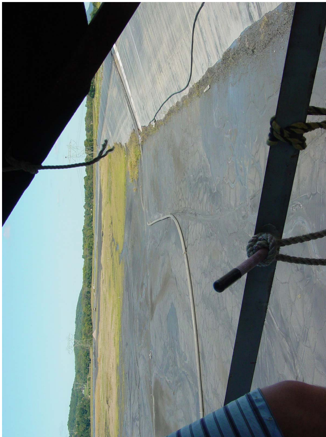
Photo B4-9: Ash Basin No. 4 Inside Slope of East Embankment and View of Ash Surface in Basin– Viewed North from Top of Decant Tower – Note Vertical Wrinkles in Liner (Commonly Occurs Throughout).
