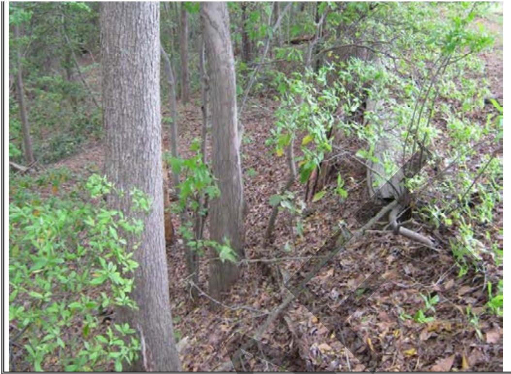
Photograph 11: Local timber restraint at crest level – Northern Ash Area, north dike.
