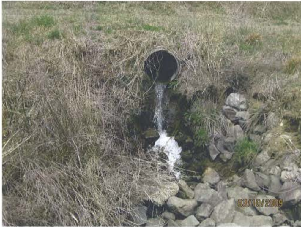
17. Ash Pond – Discharge from secondary settling basin
