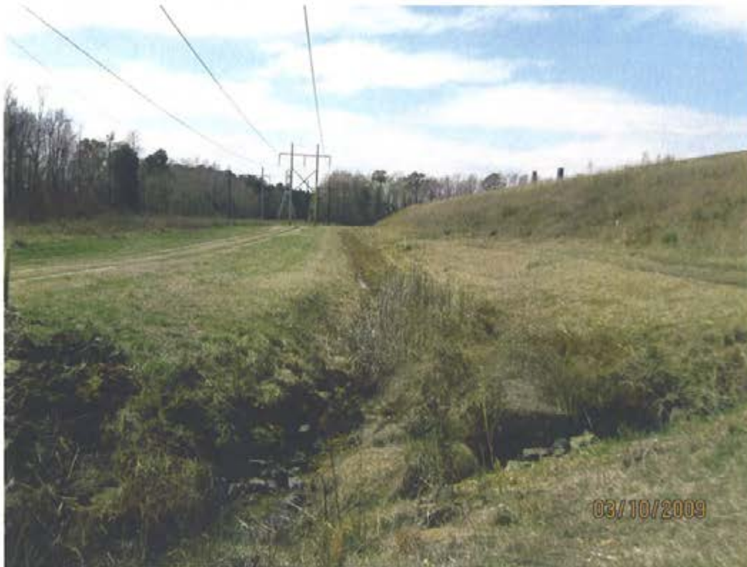
6. Ash Pond – Exterior slope, berm and drainage ditch – South Dike
