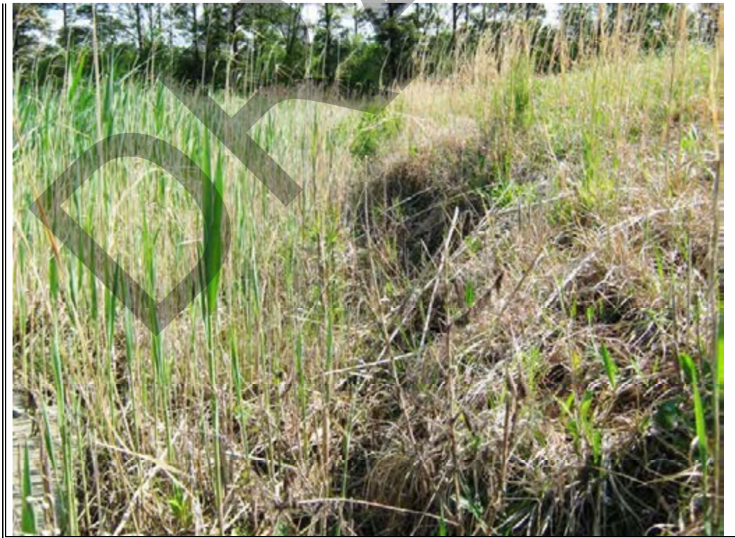
Photograph 18: Old beaching erosion on south dike – Southern Ash Area.
