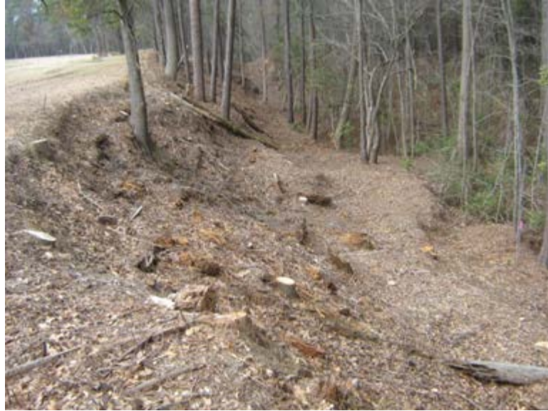
Downstream slope – Northern Ash Area
