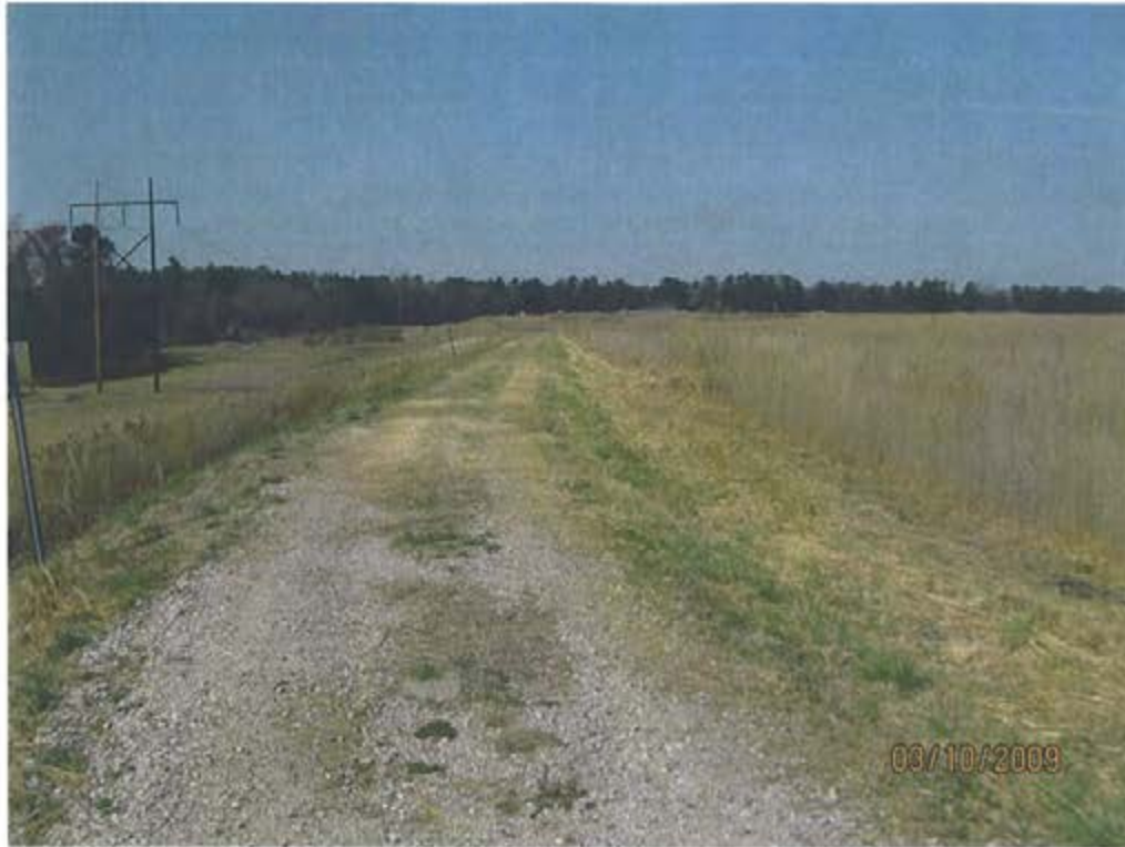
1. Ash Pond – Crest-West Dike looking North
