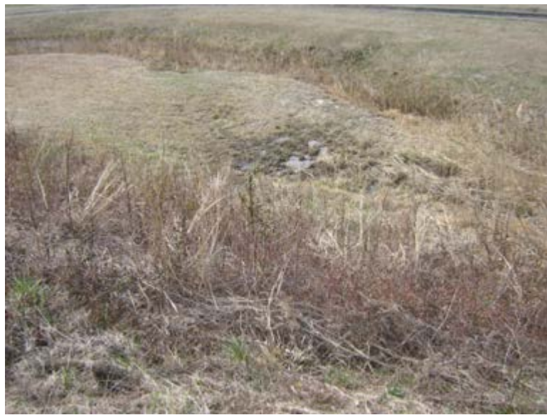
Potential seepage along downstream toe – Southern Ash Area
