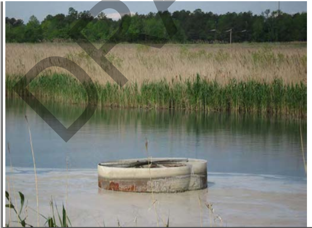
Photograph 28: Skimmer structure for Southern Ash Area.
