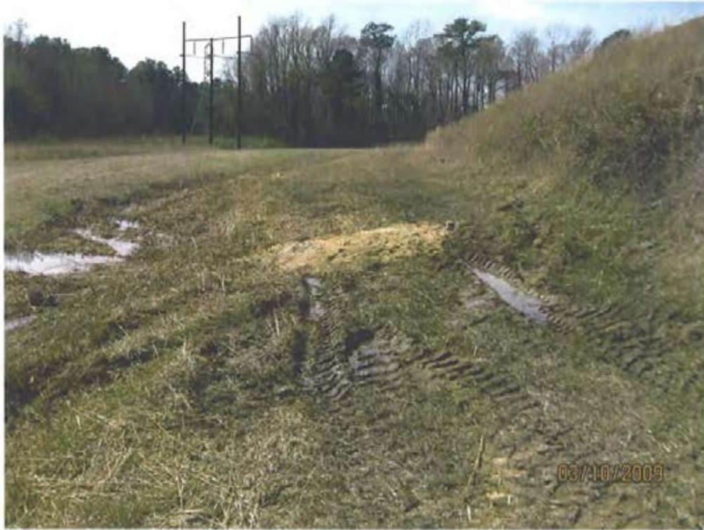
11. Ash Pond – South Dike-West end with ruts from mowing
