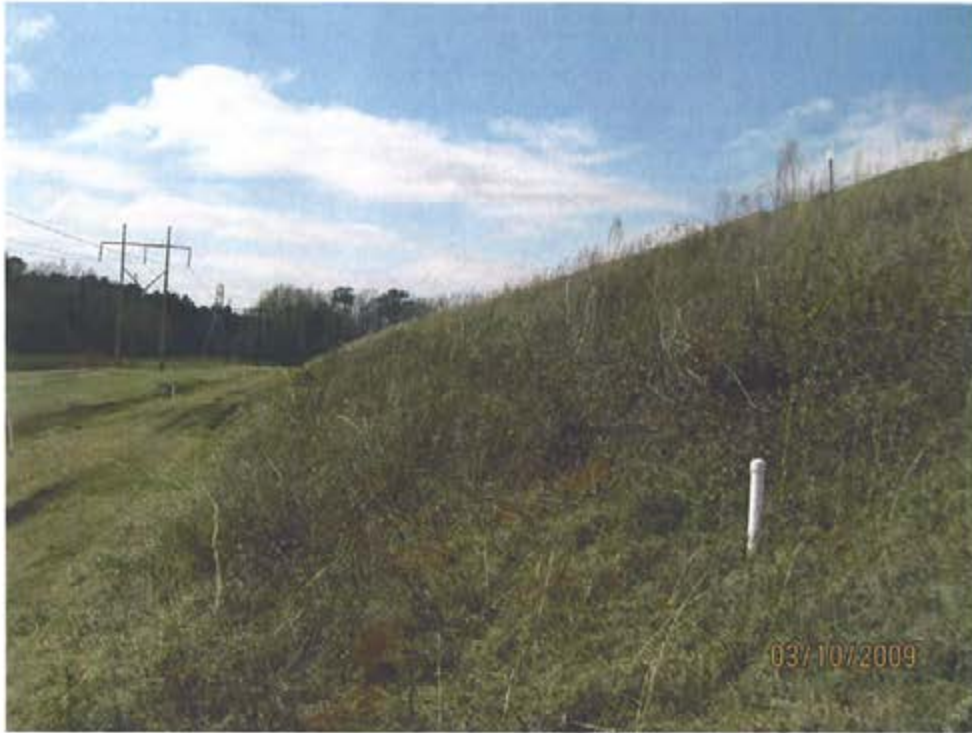
7. Ash Pond – South Dike-Exterior slope looking West
