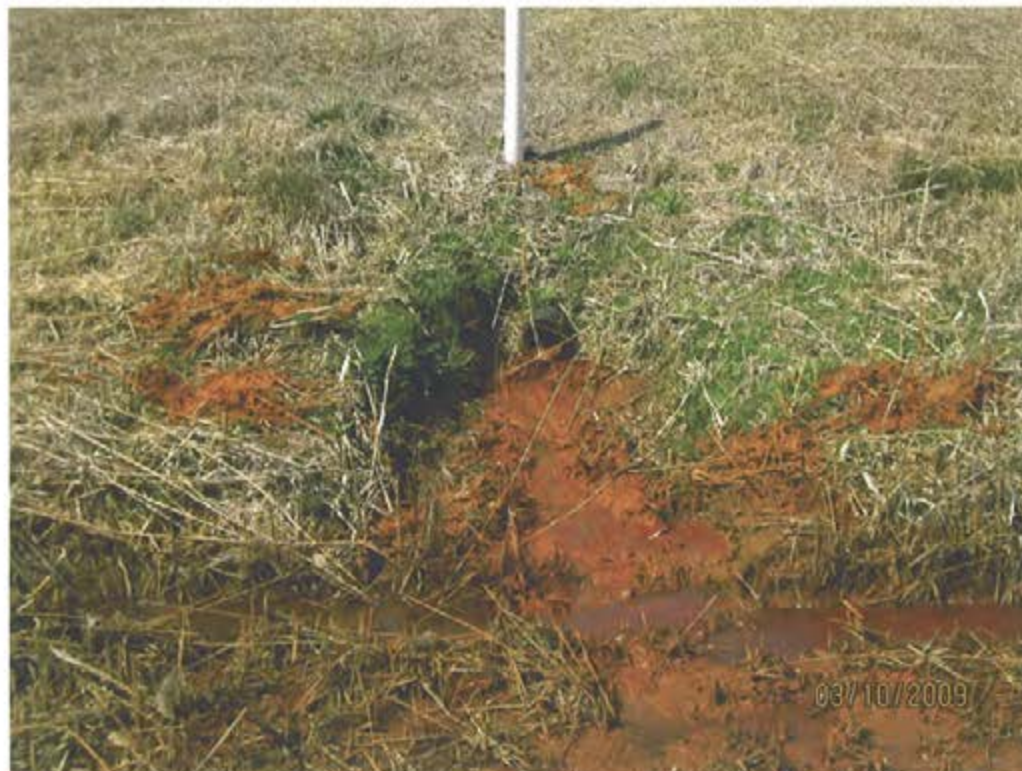
13. Ash Pond – Localized seep on south slope dike
