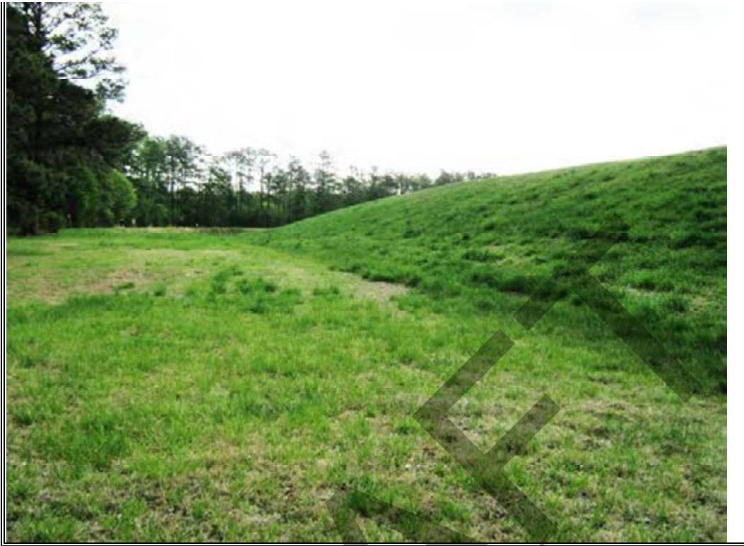
Photograph 3: Interior drainage swale – Northern Ash Area, north dike.
