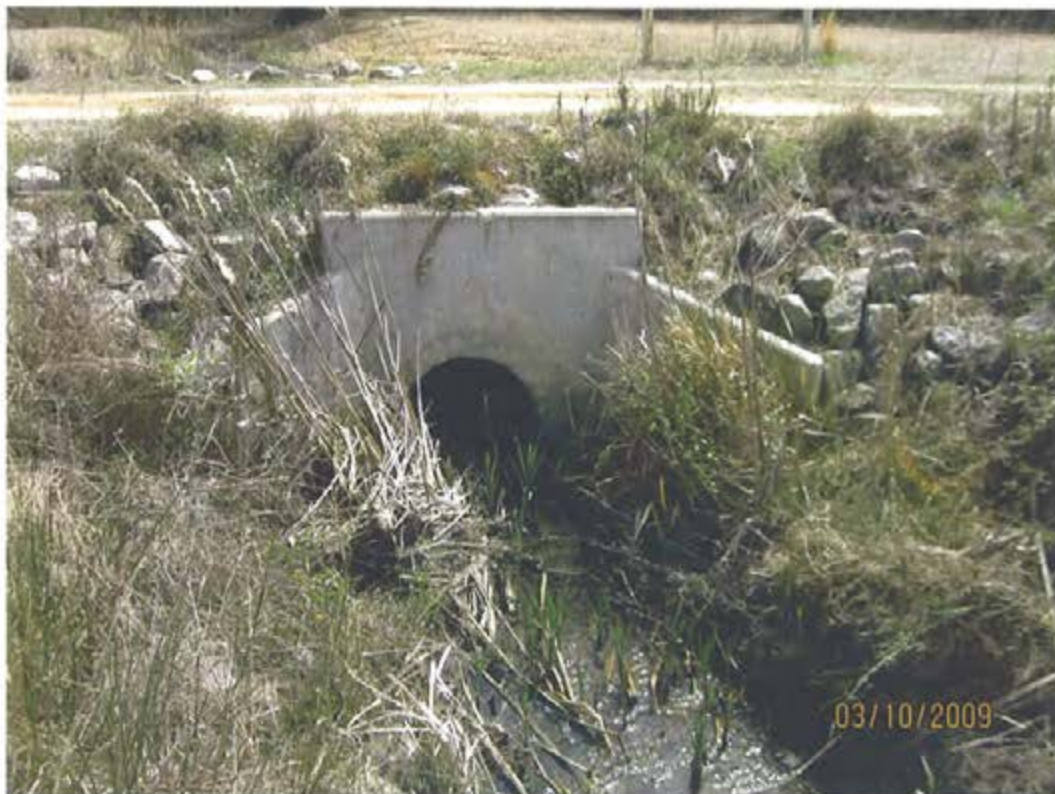
18. Ash Pond – Headwall for drainage pipe leading to cooling pond.
