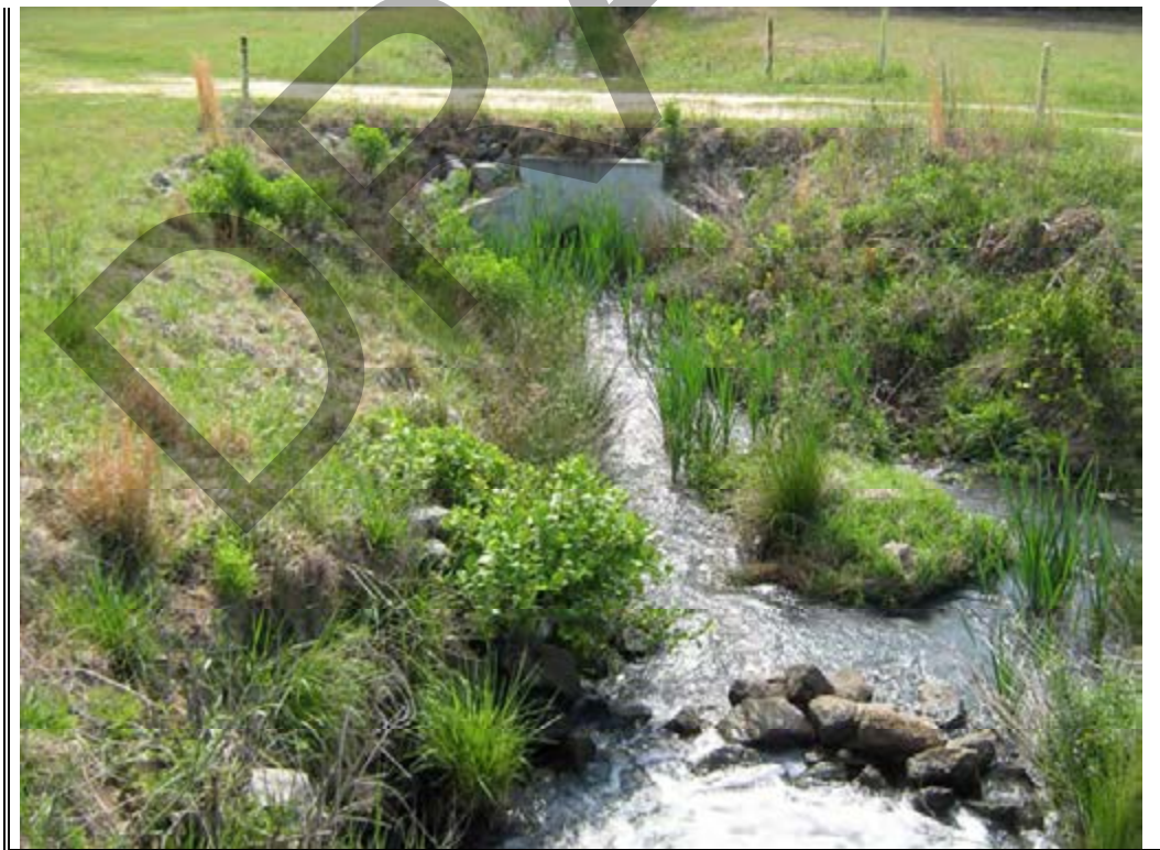
Photograph 30: Outflow channel toward Cooling Lake – Southern Ash Area.
