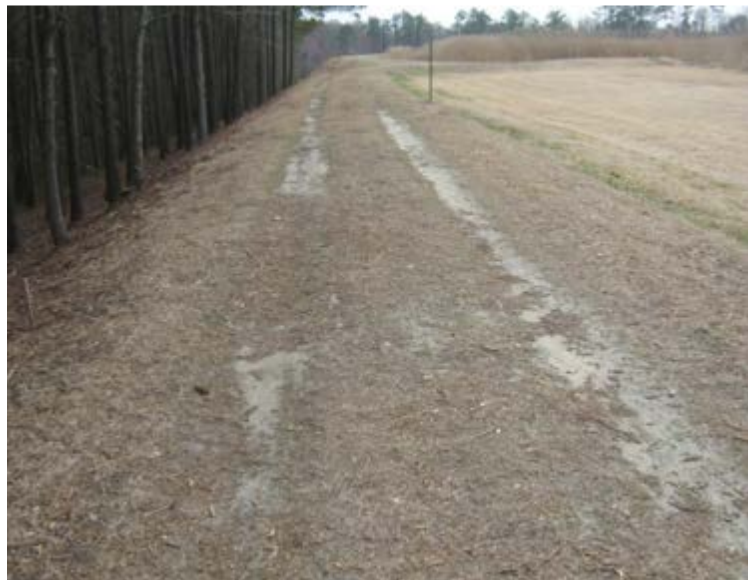
Crest showing minor rutting – Northern Ash Area
