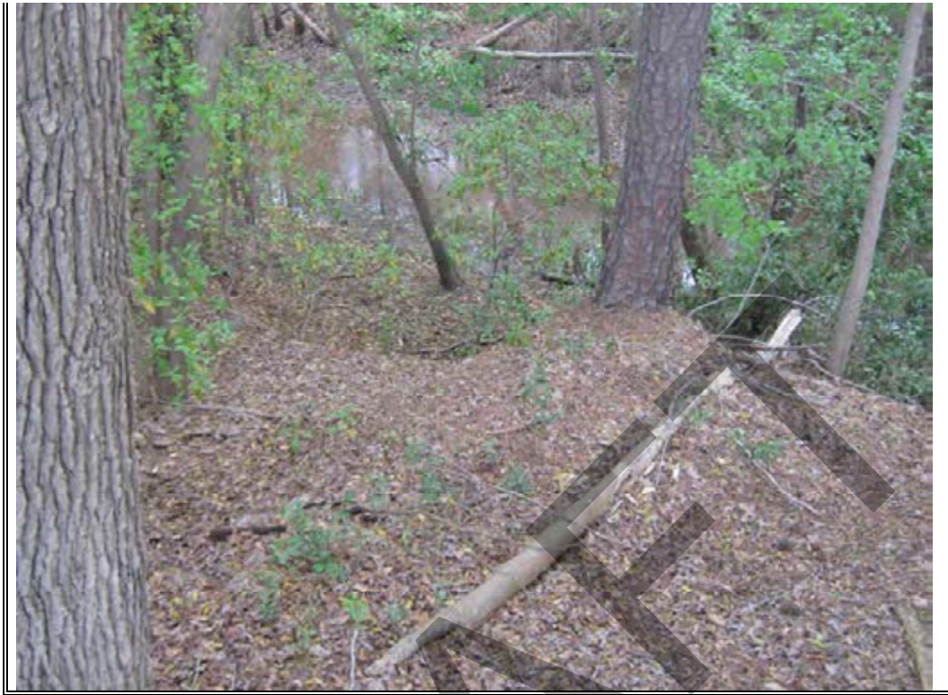
Photograph 9: Typical bench and tree growth – Northern Ash Area, west end north dike.
