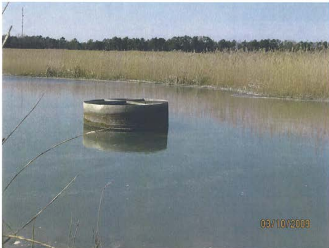
16. Ash Pond –Main Pond Skimmer on Riser
