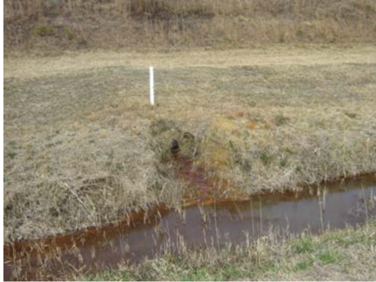
Toe drains – Southern Ash Area
