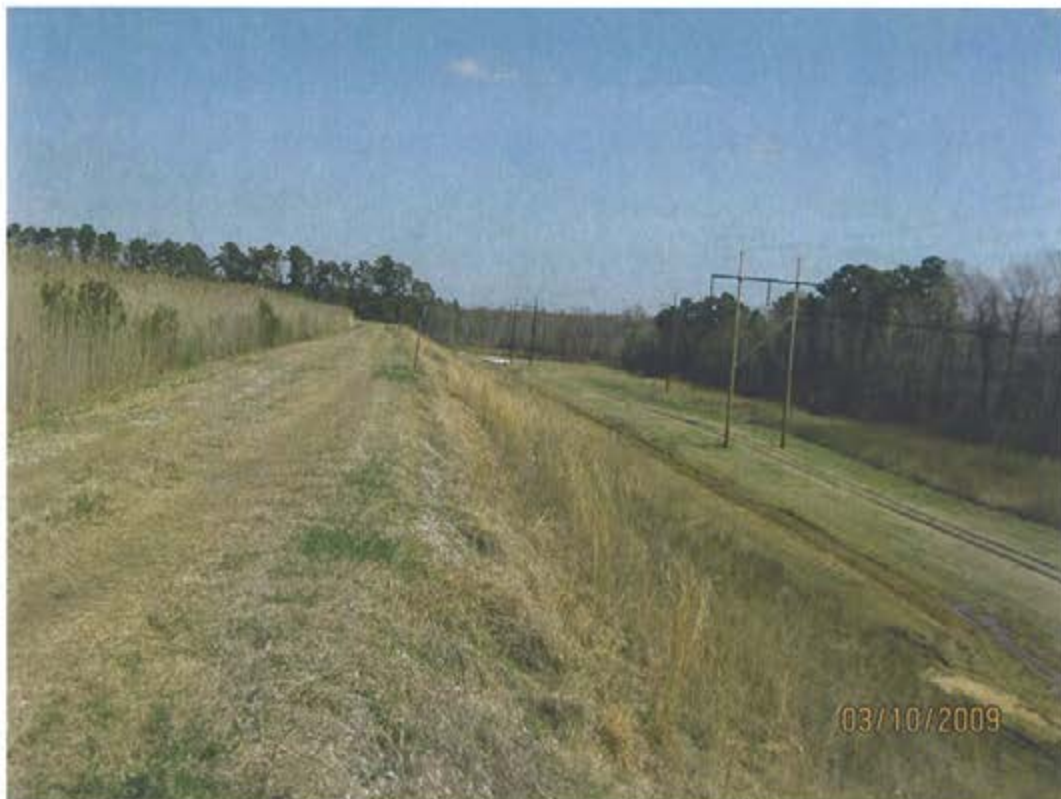
2. Ash Pond – Crest and exterior slope -South Dike looking East
