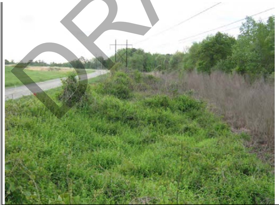
Photograph 6: Exterior slope – Northern Ash Area, west dike. Note vegetation.
