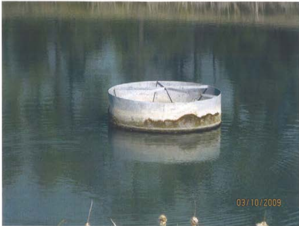
15. Ash Pond – Secondary Settlement Pond Skimmer on Riser
