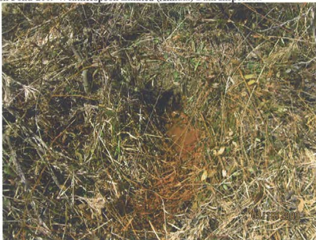
13. Ash Pond – Localized seep on south slope dike
