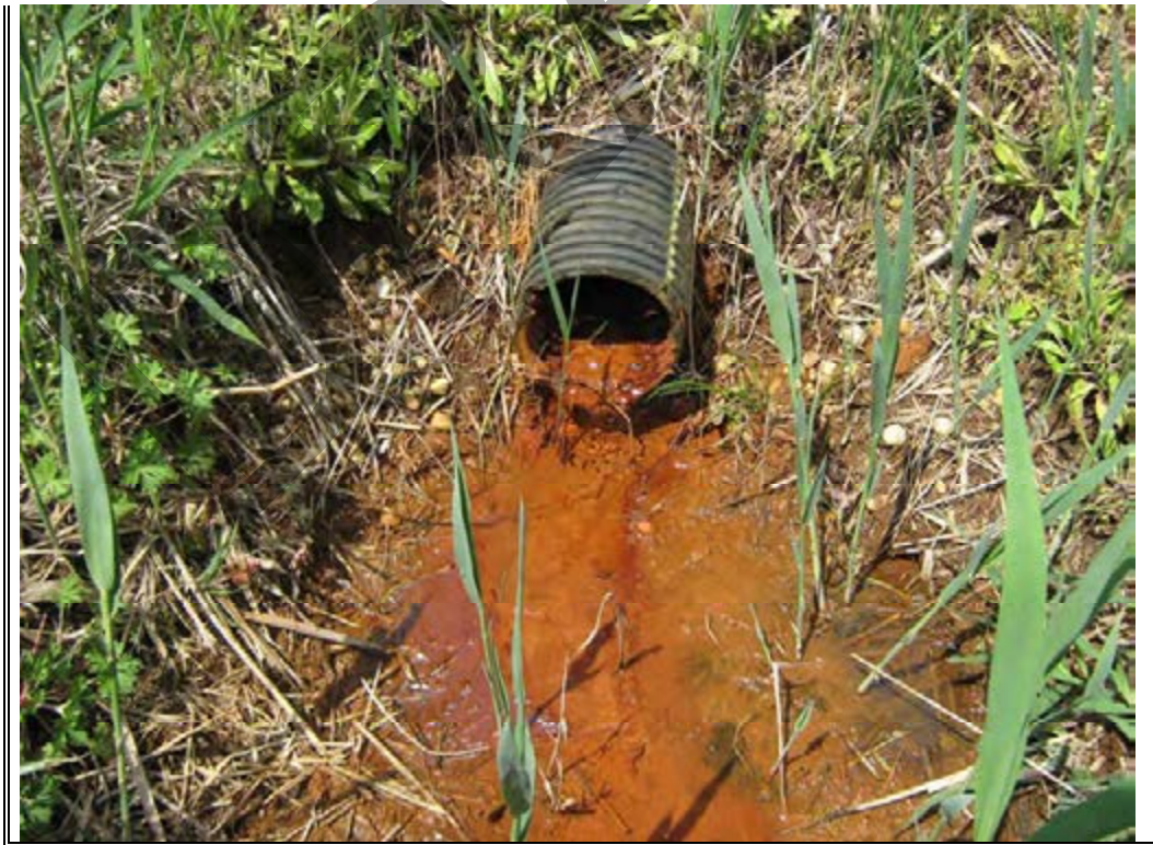
Photograph 26: Toe drain outlet pipe after cleaning – Southern Ash Area, south dike.
