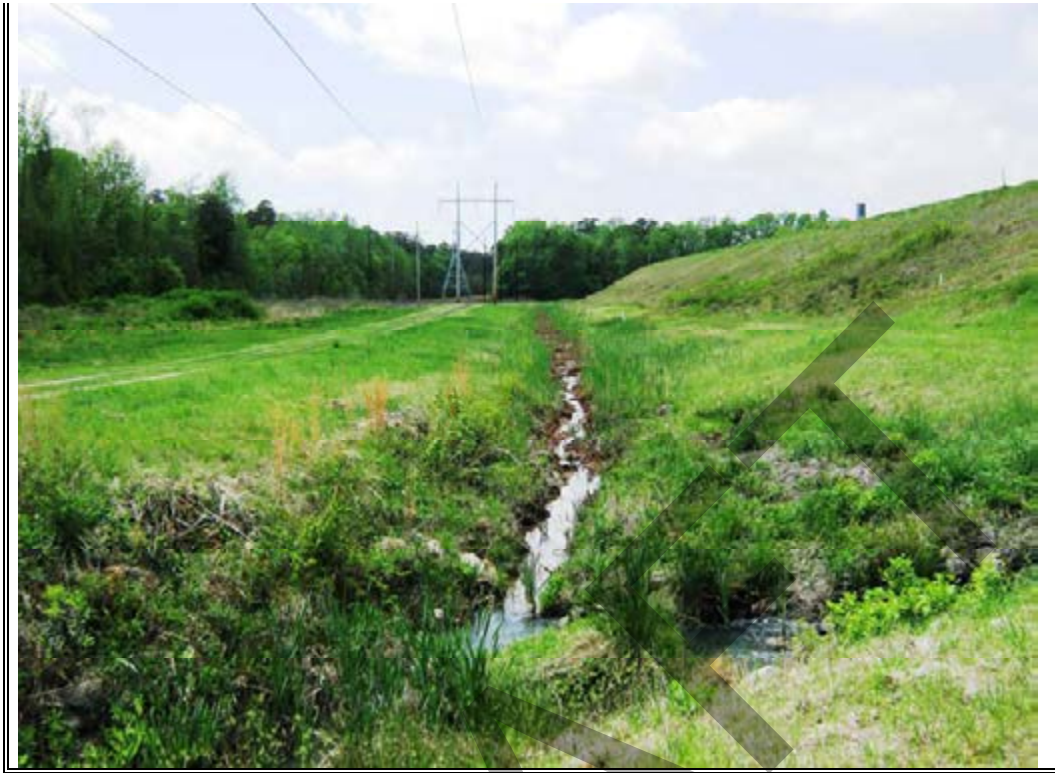
Photograph 27: Drainage swale along toe or south dike – Southern Ash Area.
