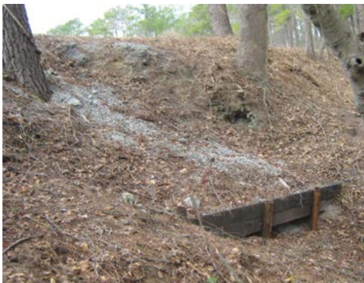
Downstream slope – Northern Ash Area
