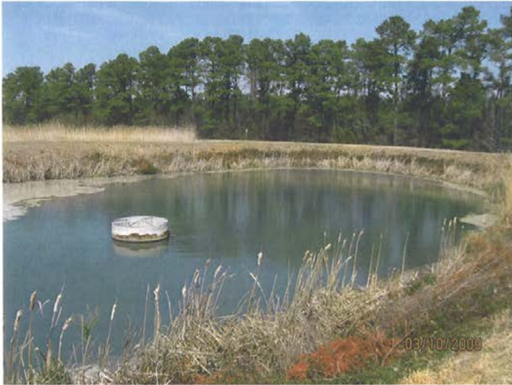
5. Ash Pond - Interior slope secondary settling pond dike
