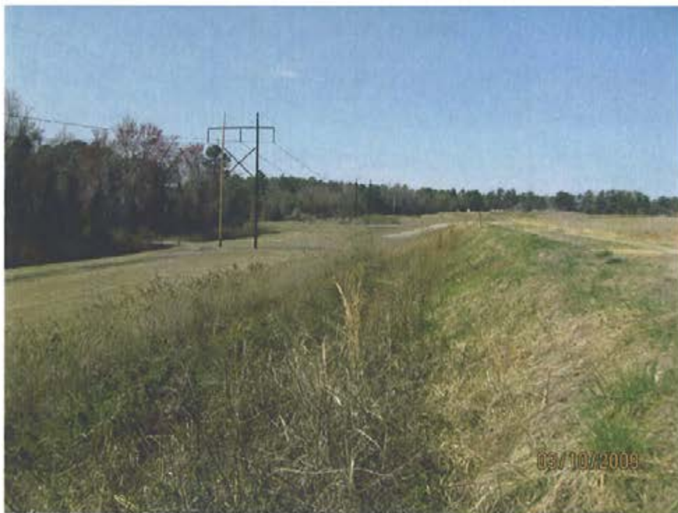
8. Ash Pond – West Dike-Exterior slope looking North
