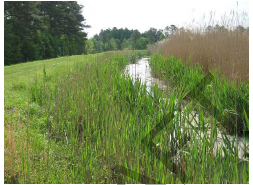
Photograph 15: Interior slope and ash/water channel – Southern Ash Area, east dike.
