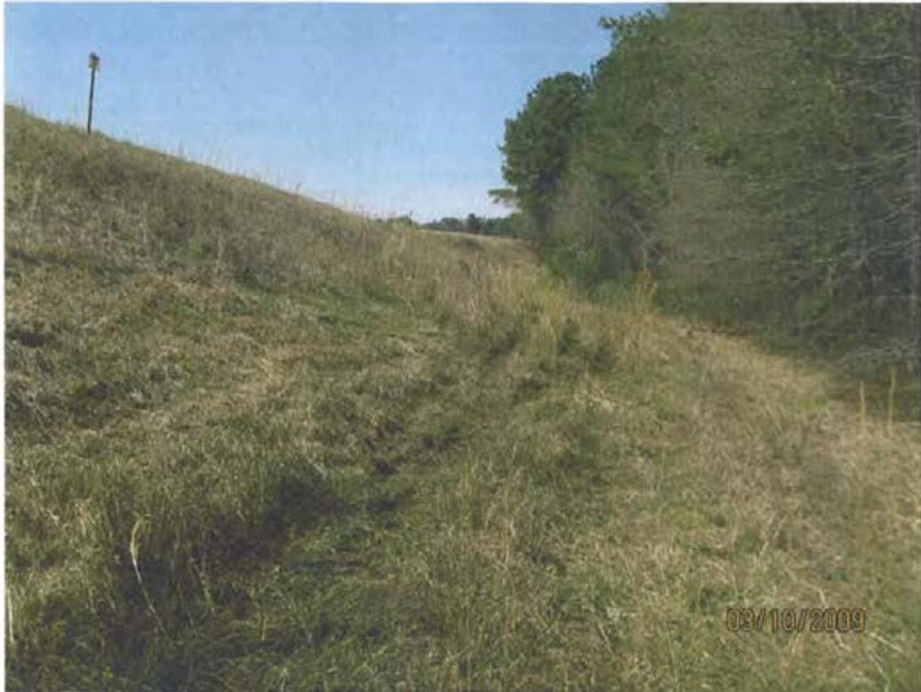
9. Ash Pond – East Dike-Exterior Slope looking North from south end
