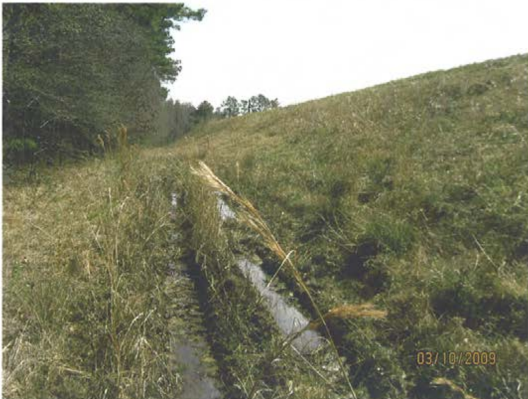
10. Ash Pond – East Dike looking south-Wet area at toe of slope
