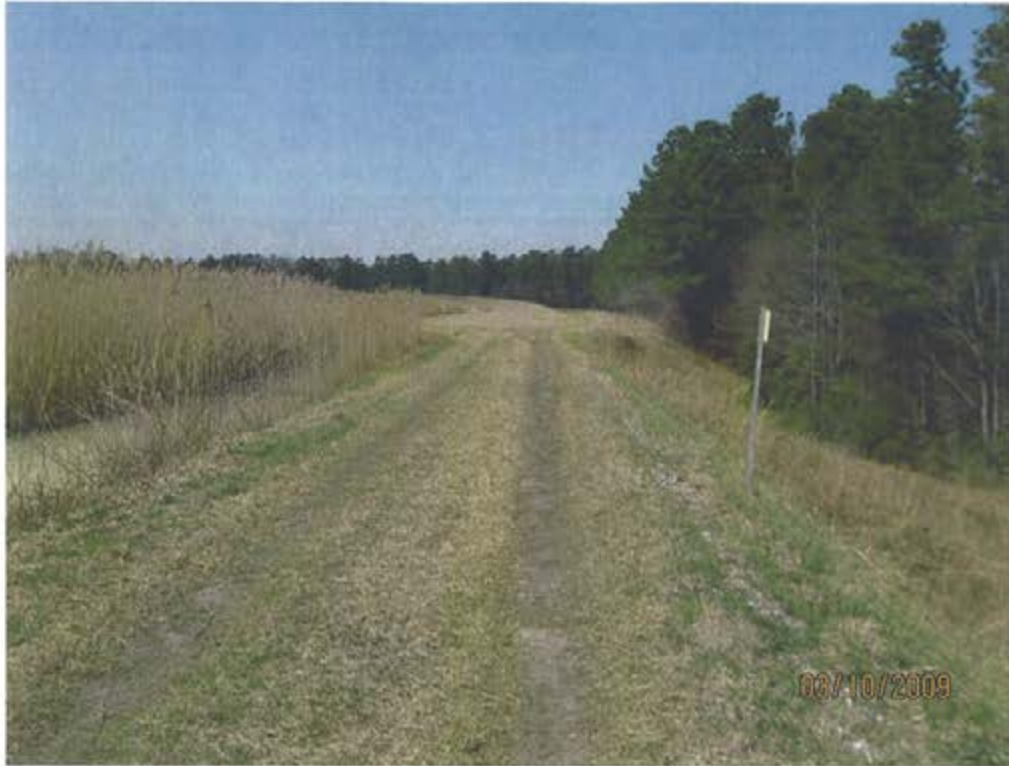
3. Ash Pond – Crest and interior slope -East Dike looking North
