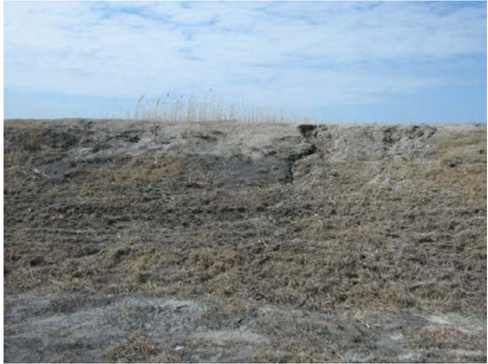
Rill erosion along downstream slope of internal dike of the 1984 Ash Pond
