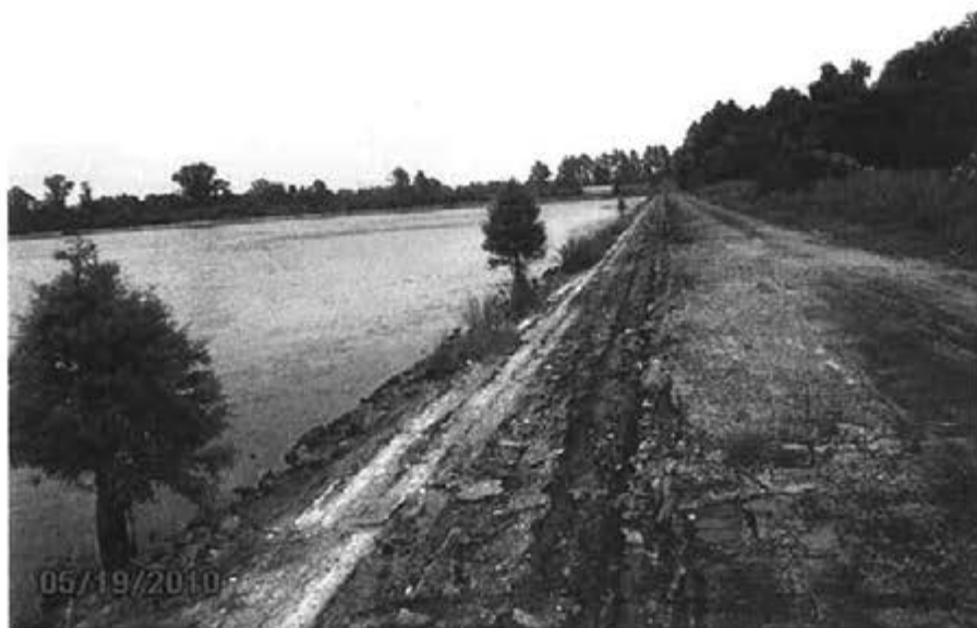
26. Cooling Pond – (Bay #1) View of crest and interior slope showing small trees growing at toe.
