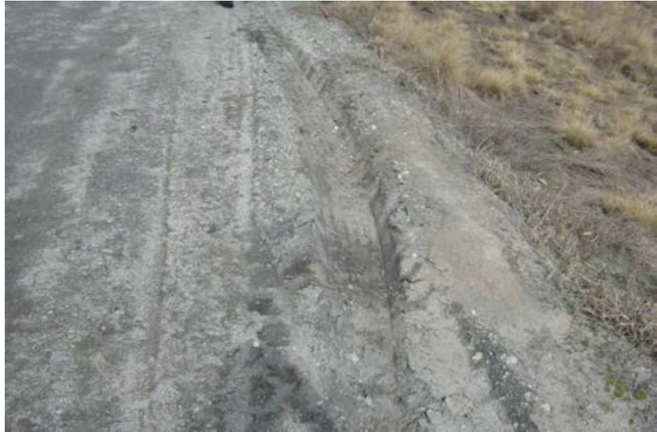
Vehicular rutting along crest of 1984 ash pond
