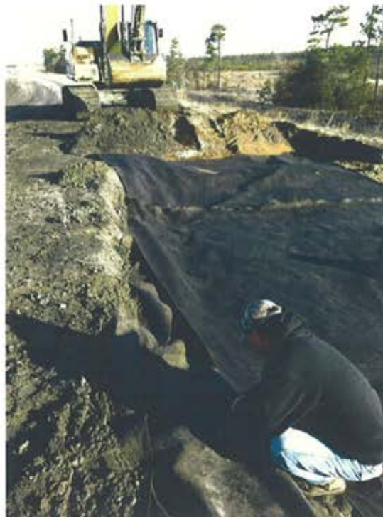
Photo 4. Placing geotextile in preparation for crest gravel.
