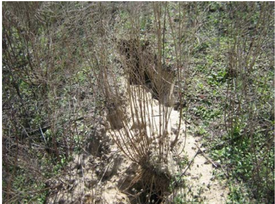
Animal burrows along downstream slope, 1984 Ash Pond
