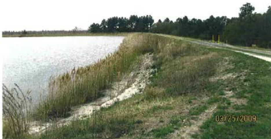
7. 1984 Ash Pond - View of riprap placed for interior slope on north side of pond.
