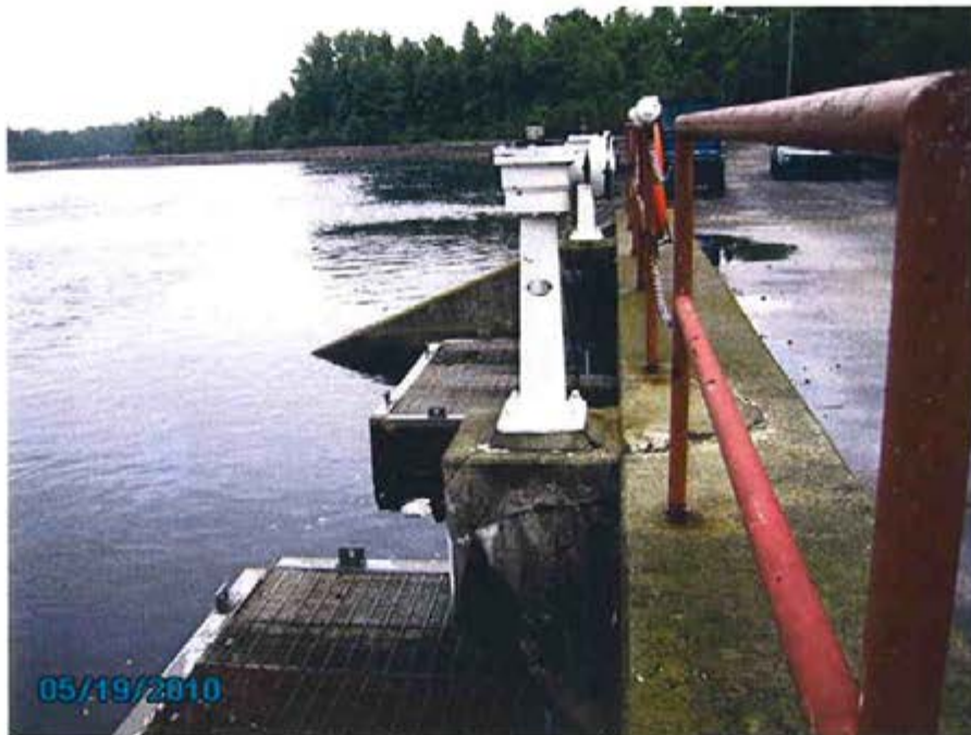
40. Cooling Pond – View of concrete cracking at sluice gate support on north side of discharge structure.
