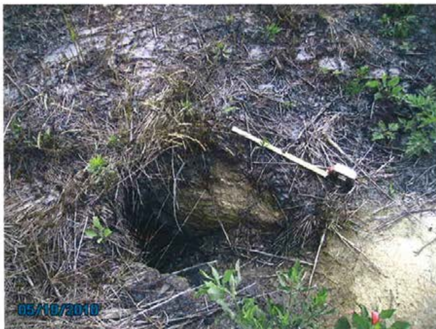
17. 1984 Ash Pond – View of animal burrow on the exterior slope for east dike (12 inch tape extension shown for scale).
