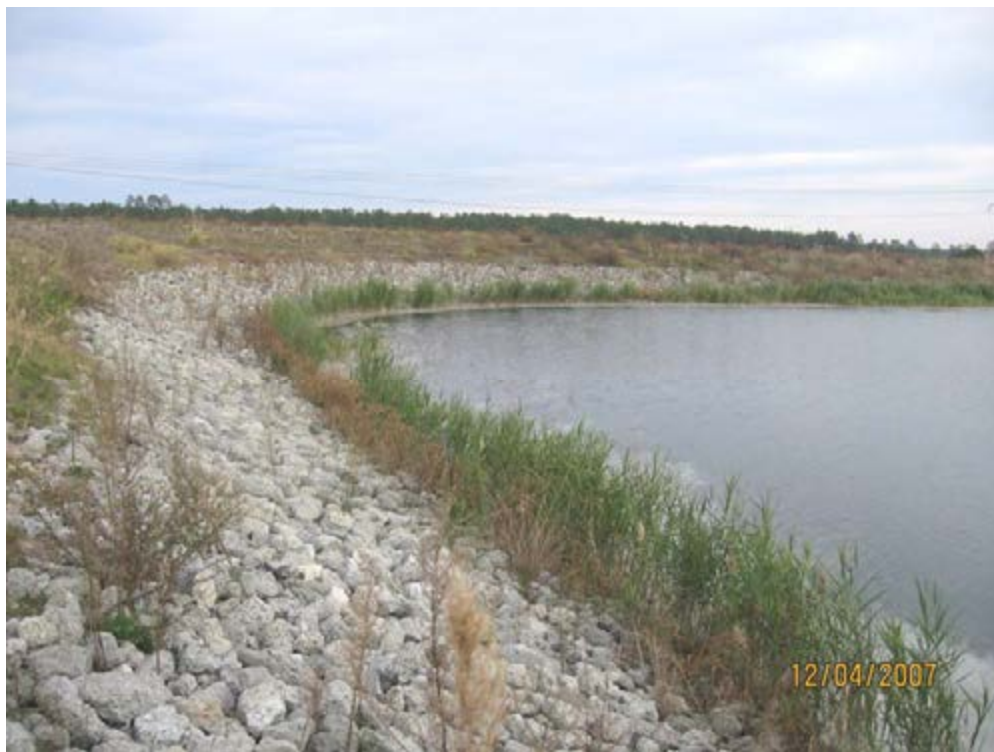
Photo 6. 1984 Ash Pond – Interior slope newly repaired with rip rap. Typical of section with good rip rap.
