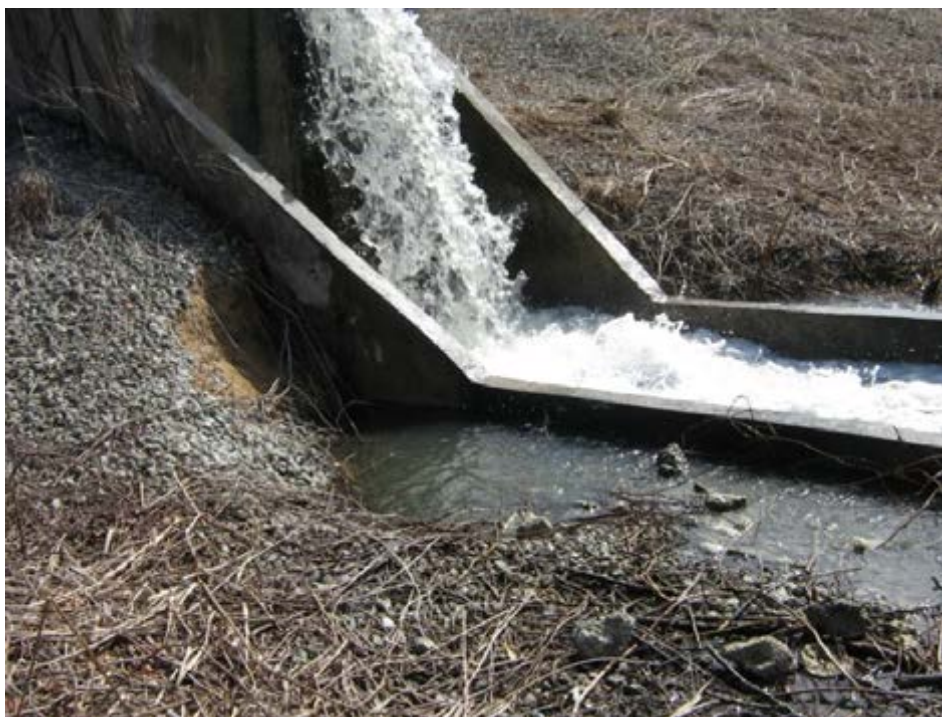
Concrete outfall of 1984 Ash Pond where undercutting is present
