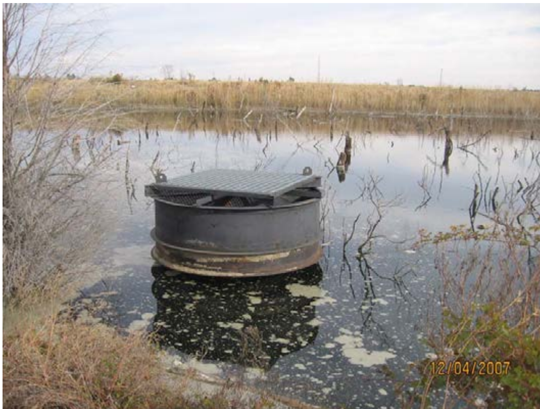
Photo 1. 1983 Ash Pond – Outlet riser and pond water.
