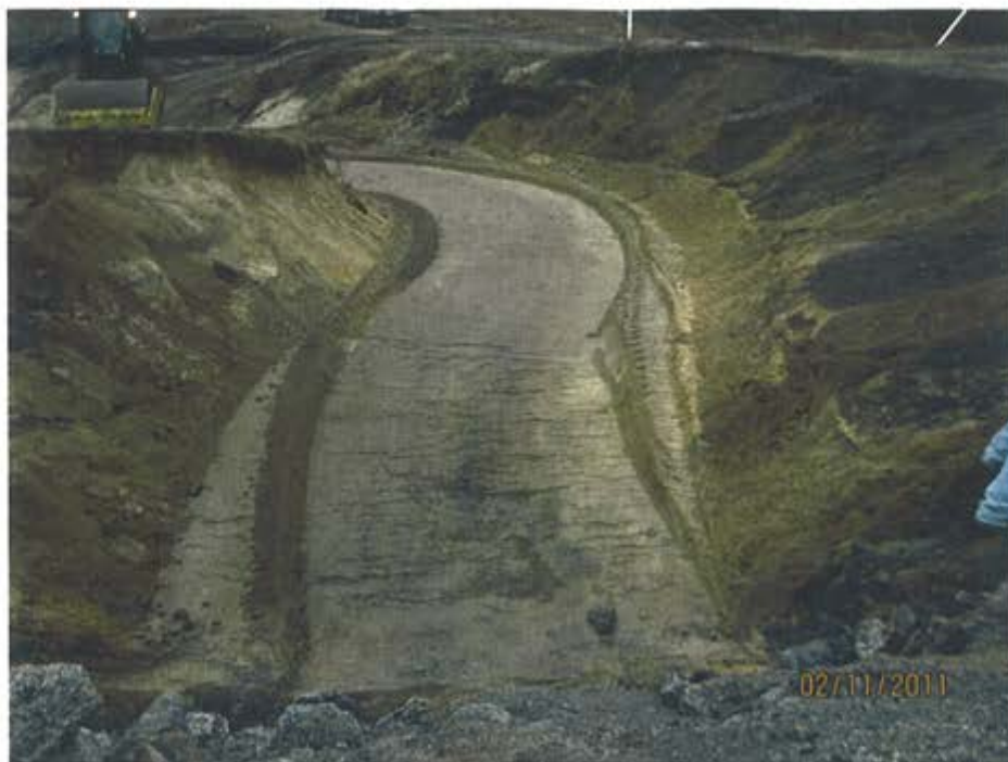
Photo 1. Breach bottom area after initial preparation.
