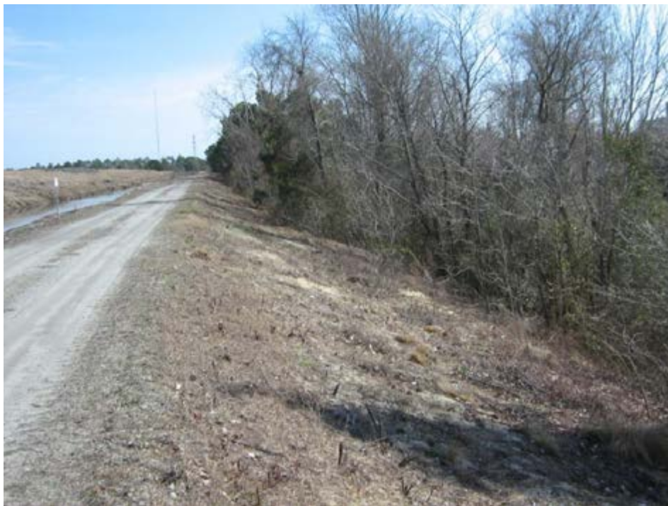
Trees along downstream south slope of 1971 ash pond.
