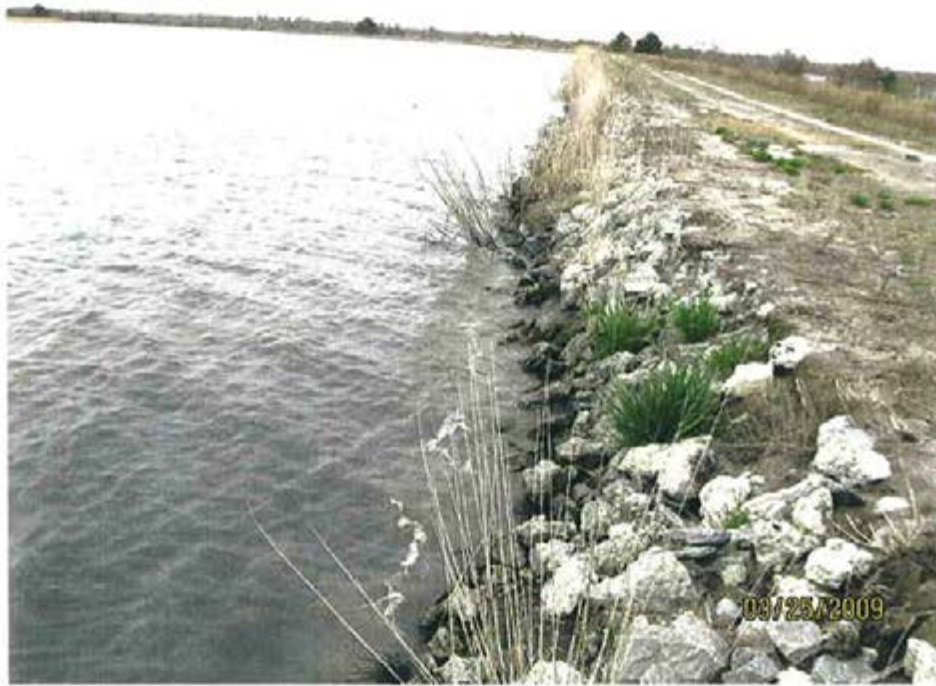
17. 1984 Ash Pond (Interior Storage Area) – View of riprap along interior slope on north side of pond.
