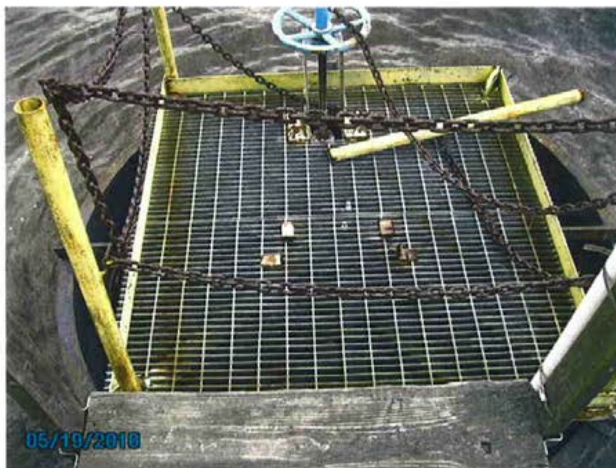
19. 1984 Ash Pond – View at top of platform mounted on skimmer for discharge structure.
