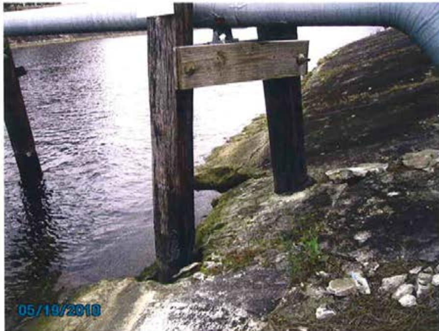
39. Cooling Pond – View of slope protection damage at pipe support on interior slope near the sluice gate structure.
