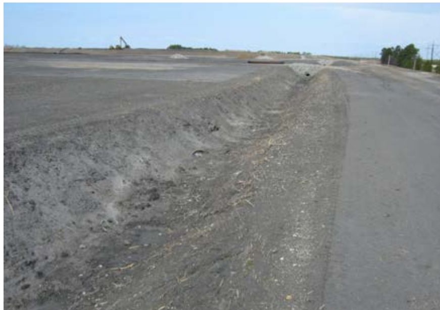
Upstream slopes along 1984 ash pond to be vegetated, Spring 2011. Work conducted in this area was to repair the small overflow from the 1984 ash pond
