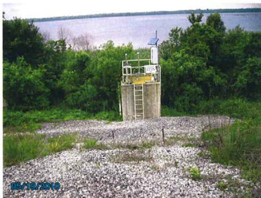
20. 1984 Ash Pond – View of discharge diversion structure at toe of west dike.
