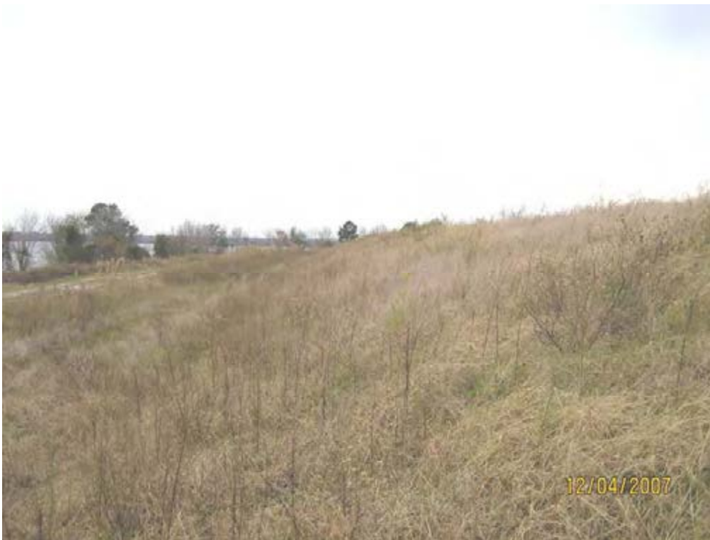
Photo 10. Ash Pond –Typical exterior slopes of 2006 dike.
