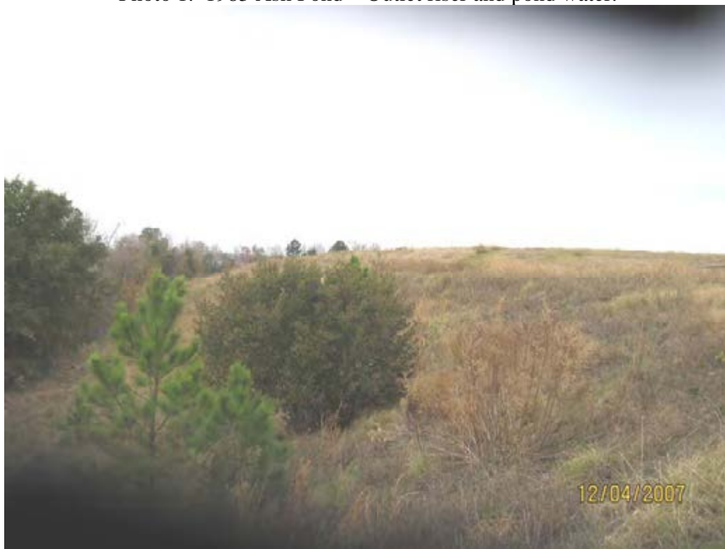
Photo 2. 1984 Ash Pond – Exterior Slope looking northwest.
