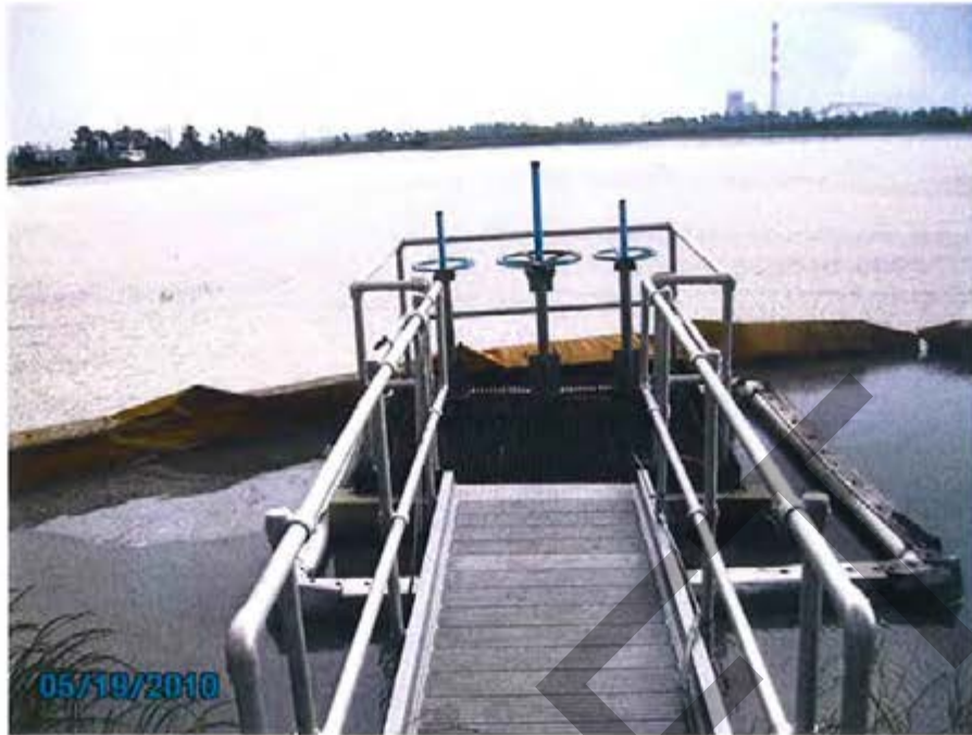
25. 1984 Ash Pond/Interior Storage – View of discharge structure from access platform.
