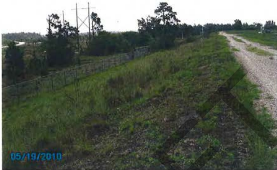
5. 1984 Ash Pond - View of exterior slope for east dike looking south.
