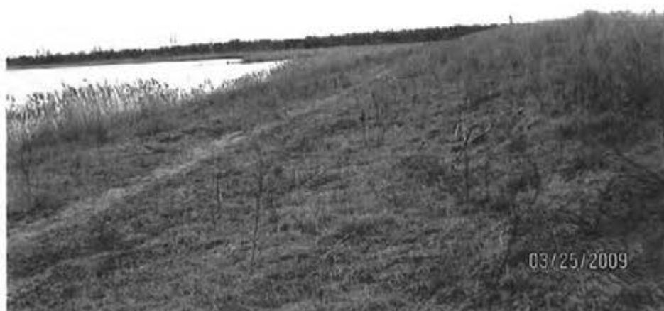
16. 1984 Ash Pond (Interior Storage Area) – View of along toe of north dike.
