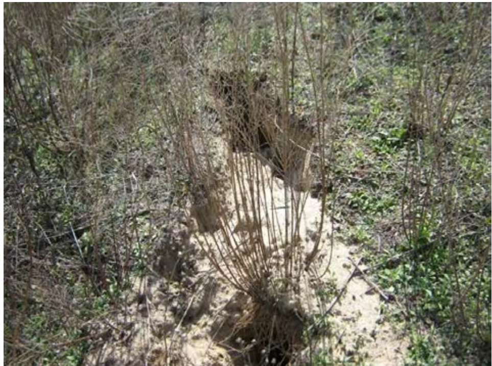
Animal burrows along downstream slope, 1984 Ash Pond
