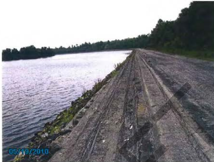
30. Cooling Pond – (Bay #3) View of crest and interior slope looking south.
