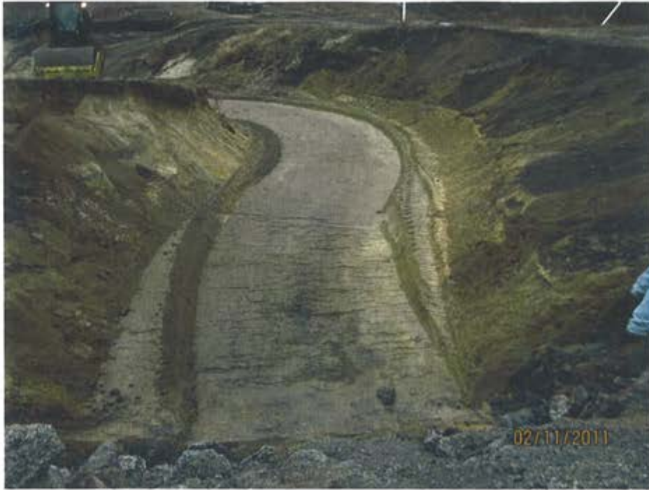
Photo 1. Breach bottom area after initial preparation.
