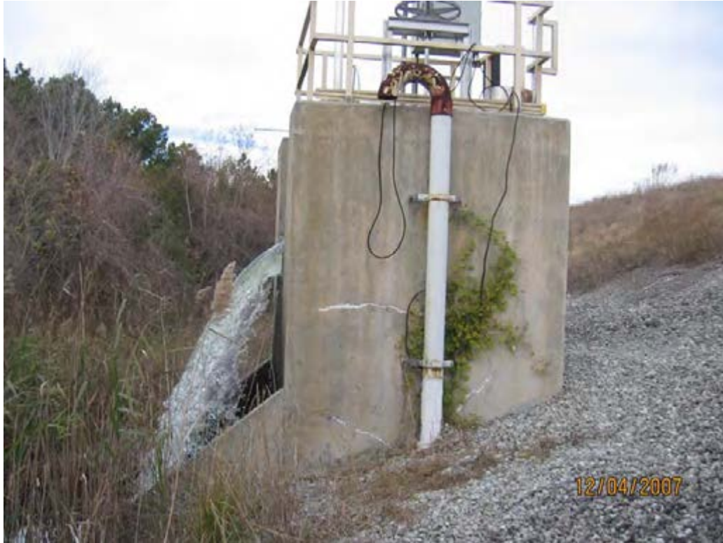
Photo 7. Ash Pond – Outlet drainage Structure looking northwest.
