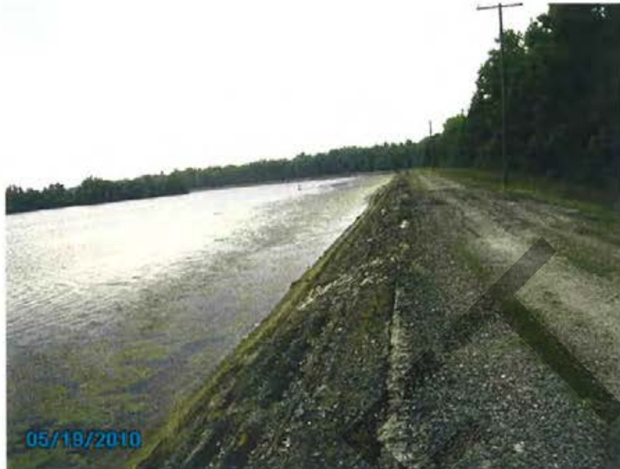
37. Cooling Pond – (Bay #6) View of crest and interior slope looking east.
