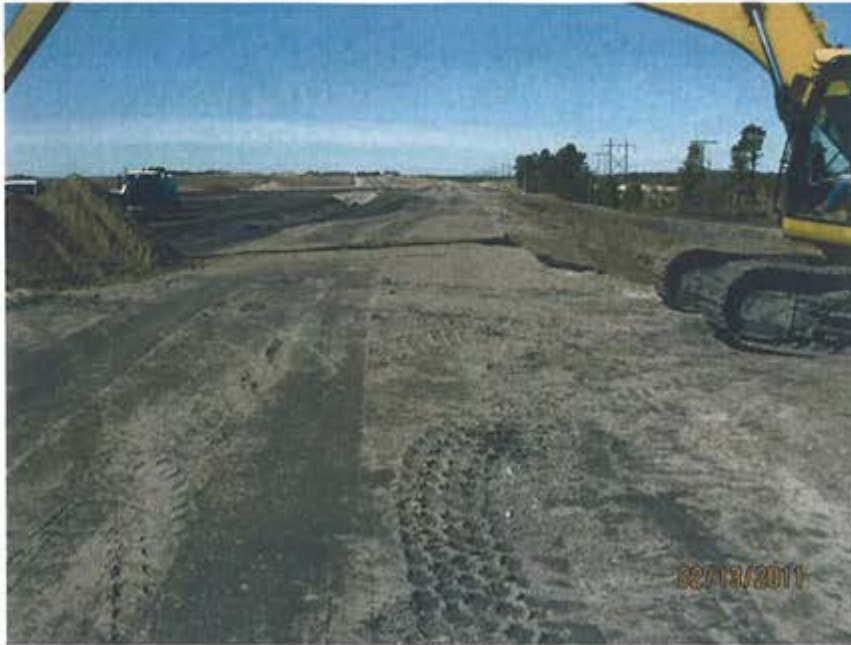
Photo 5. Crest at final grade.
