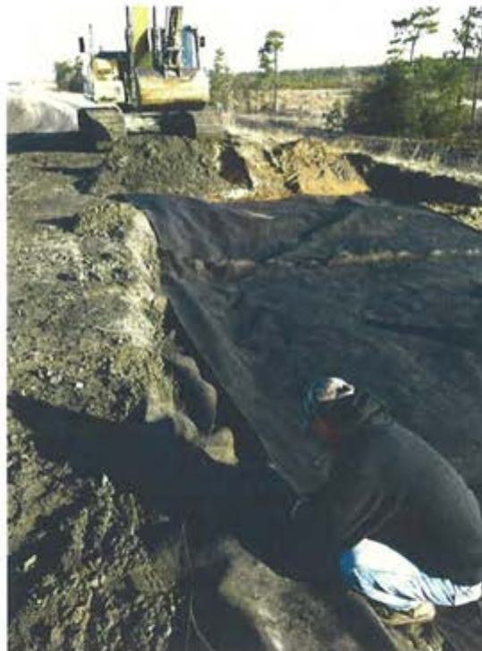
Photo 4. Placing geotextile in preparation for crest gravel.
