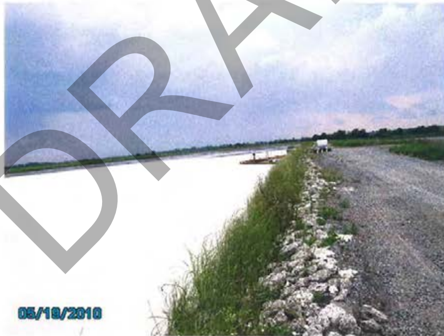
24. 1984 Ash Pond/Interior Storage – View of interior slope for containment dike and discharge structure looking west.
