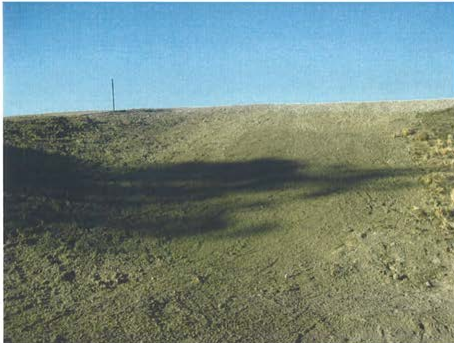
Photo 6. Completed repair slope.
