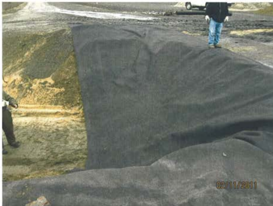
Photo 2. Placing geotextile across riprap face of emergency plug.
