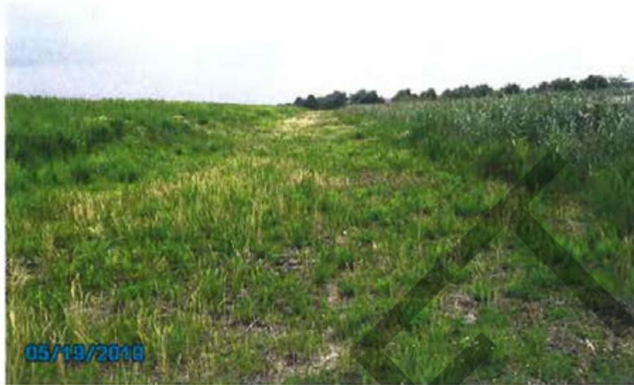
23. 1984 Ash Pond/Interior Storage – View of stability berm for containment dike looking west.
