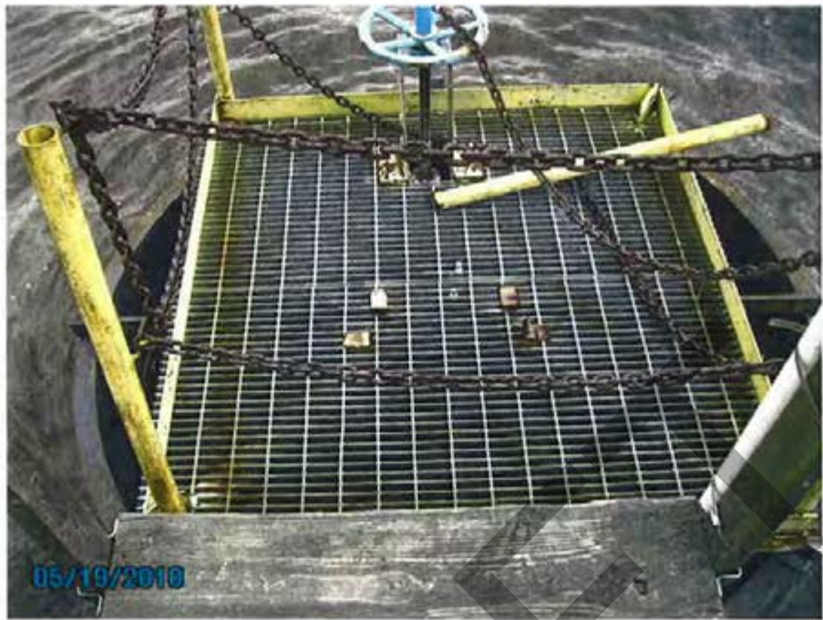
19. 1984 Ash Pond – View at top of platform mounted on skimmer for discharge structure.
