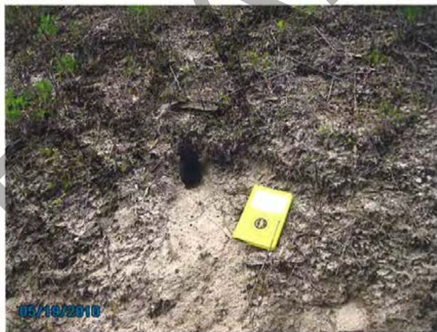
18. 1984 Ash Pond – View of animal burrow on the exterior slope for north dike (4" x 7" field book shown for scale).
