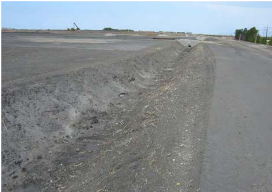
Upstream slopes to be vegetated, Spring 2011
