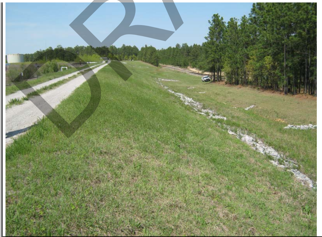
Photograph 51: Exterior of South Pond dike. Note good vegetative cover of slope and drainage ditch adjacent to dike toe.
