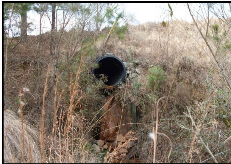
Photograph 5.9. HDPE outlet into outfall channel downstream of junction box, looking west. (Note steep bank and eroded small riprap around end of pipe,)
