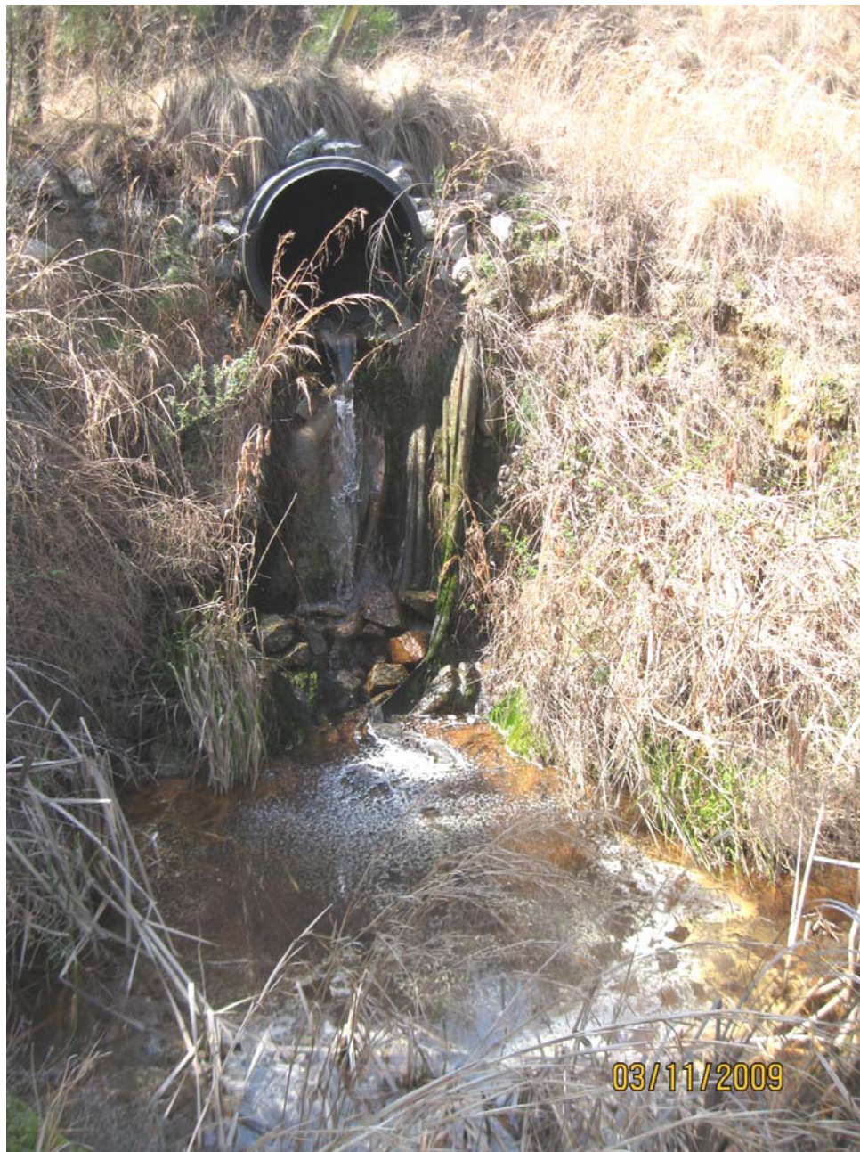
10. ASH POND – Outlet end of ash pond discharge pipe.
