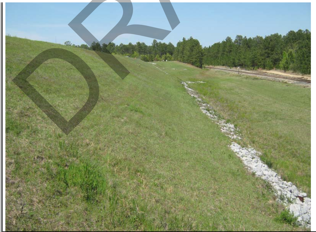
Photograph 53: Exterior slope and rock toe of North Pond dike.
