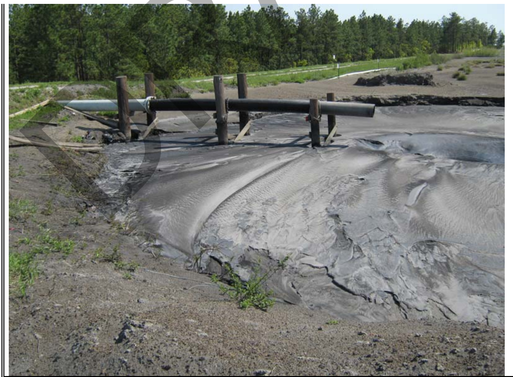
Photograph 59: Ash discharge line.
