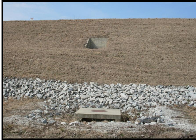
Photograph 5.8. Showing manhole access to outlet conduit on the slope, and covered catch basin at the downstream toe of the embankment of the ash pond dike, looking west.
