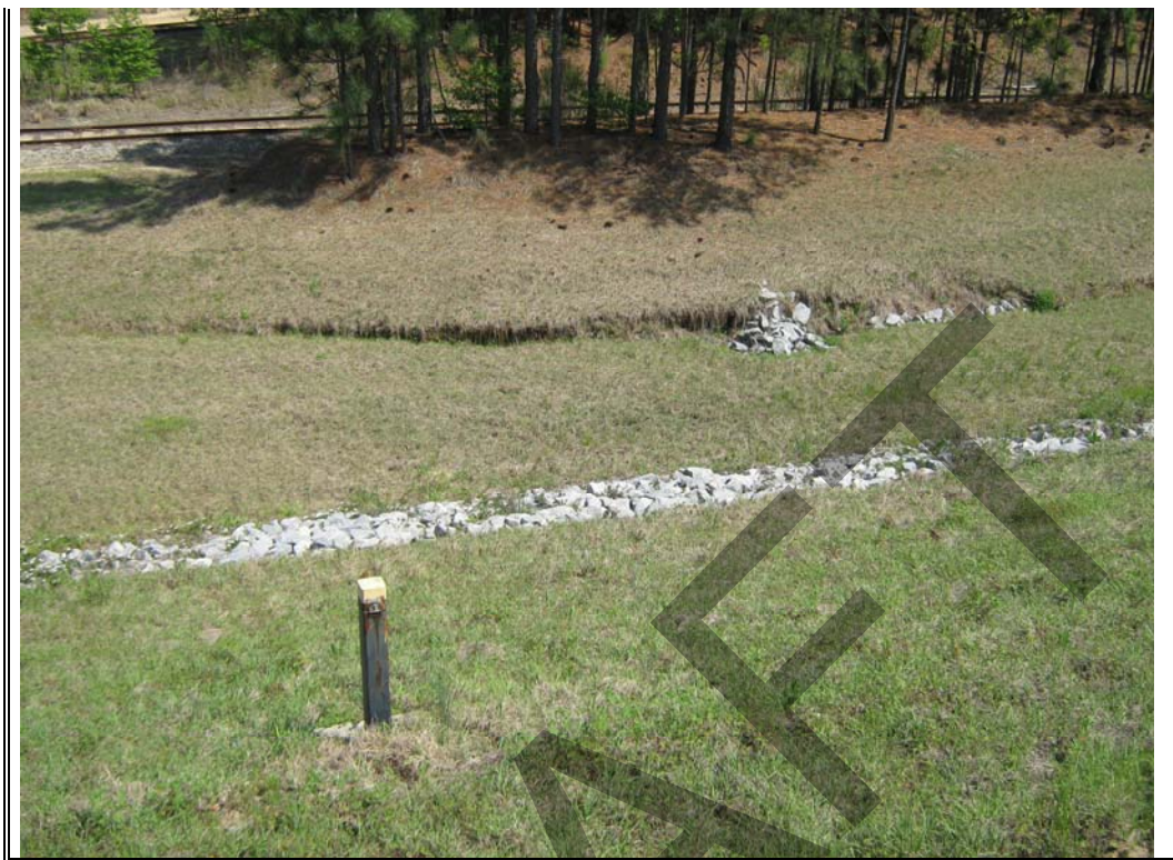
Photograph 52: Old erosion in drainage ditch area adjacent to South Pond dike toe.
