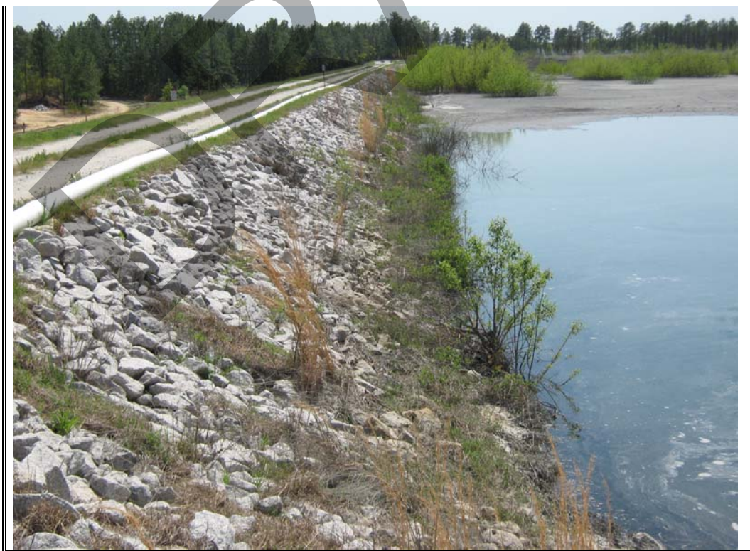
Photograph 47: Interior slope of North Pond dike. Note minor vegetation.
