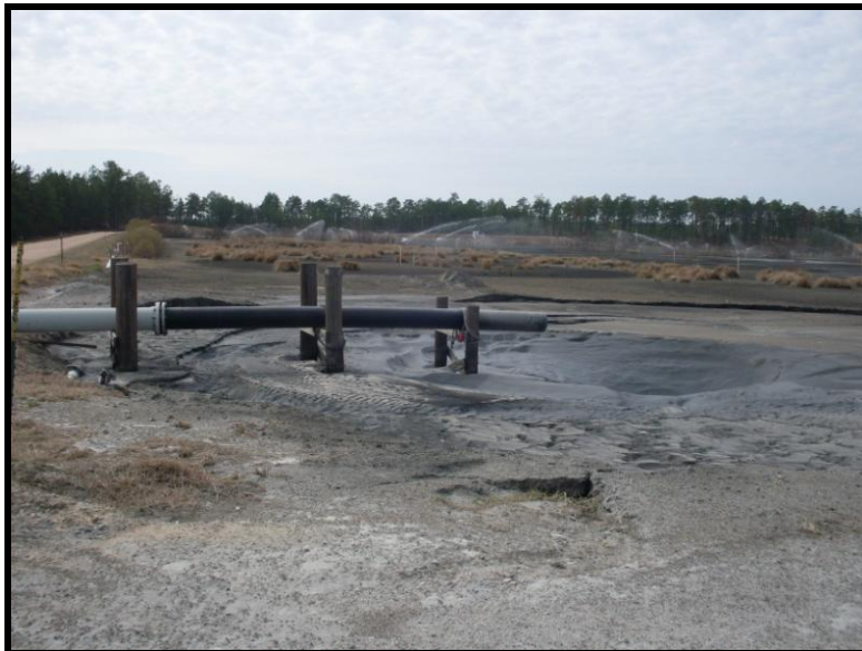
Photograph 5.3c. View of ash-sludge discharge line and ash-filled south portion of pond, looking south. (Note operation of sprinklers for dust control in south portion of pond).
