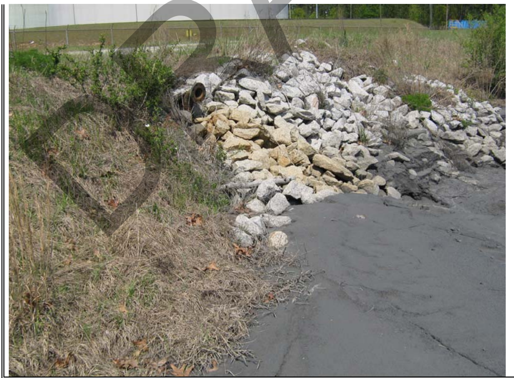
Photograph 49: Rip rap at Darlington County Plant water discharge pipe.
