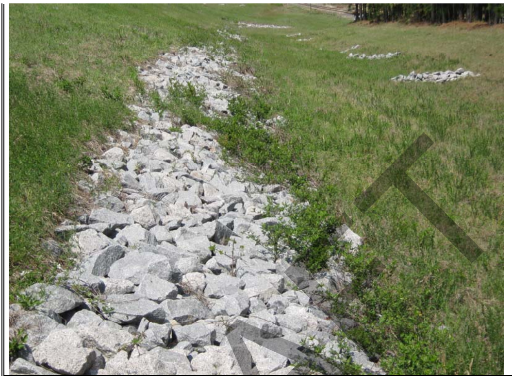
Photograph 56: Rock toe and rock check dams at toe of North Pond dike.
