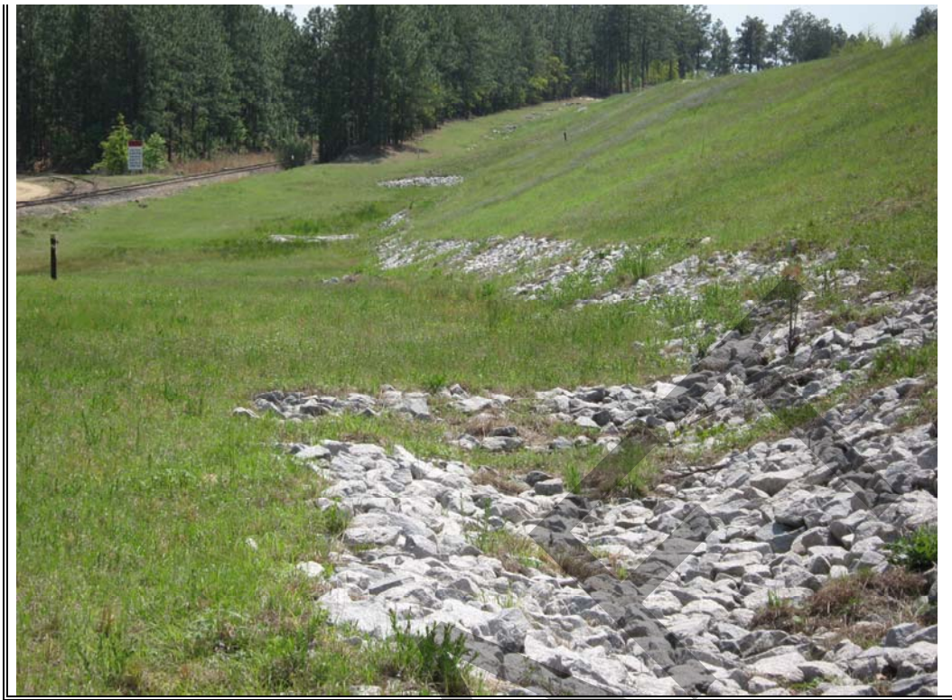
Photograph 54: Rock toe and rip rap blanket at culvert outlet near north end of North Pond dike. Note lack of erosion.
