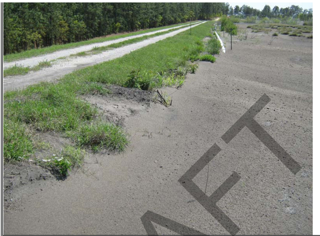
Photograph 46: Limited freeboard of South Pond dike near ash line discharge.
