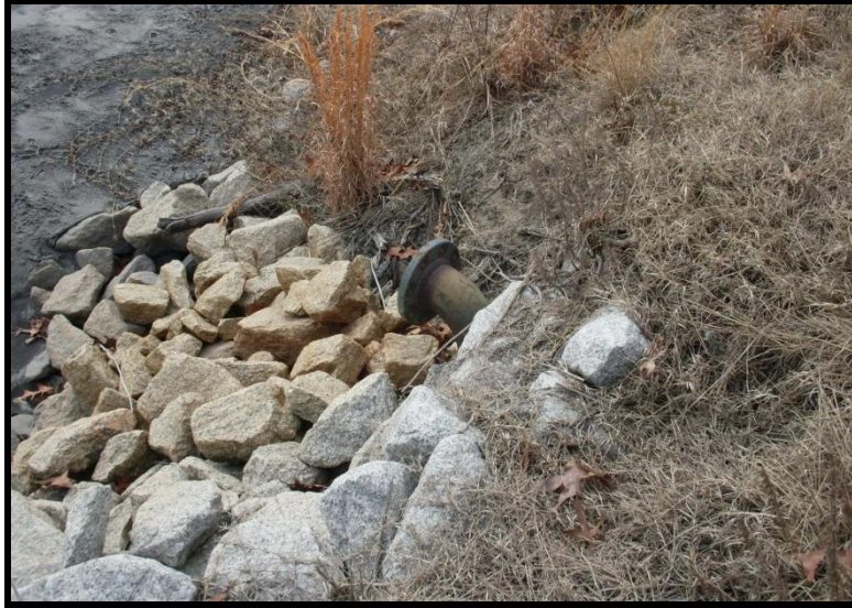
Photograph 5.3b. Discharge pipe from oil-water separator through north end of Ash Pond embankment.
