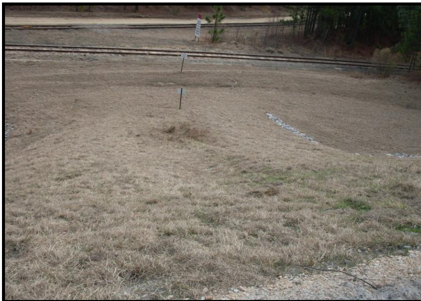
Photograph 5.5. Minor erosion observed along buried sluice line on the downstream slope, looking east.
