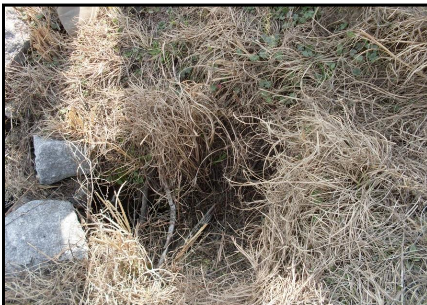
Photograph 5.6a. Hole due to soil material loss into riprap voids, observed on downstream slope above riprap at toe.
