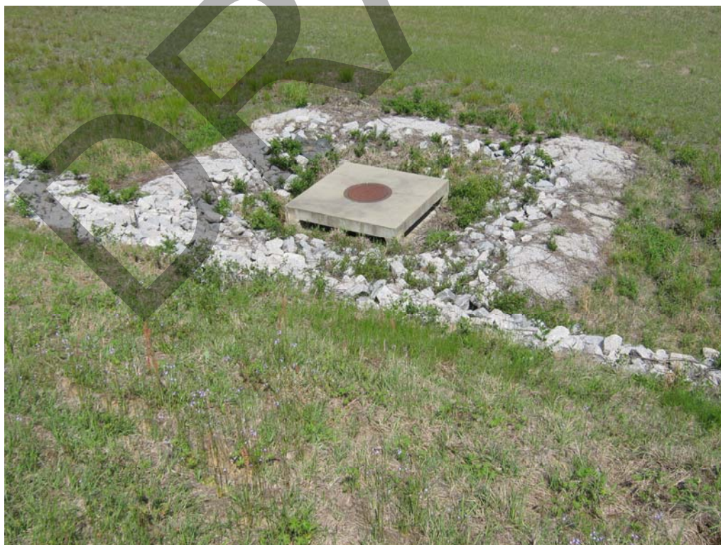
Photograph 57: Rock filter around catch basin over pipe outlet of discharge riser.
