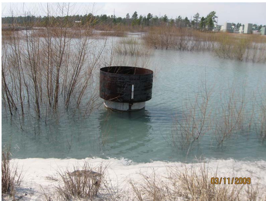
9. ASH POND – Vertical riser and trash guard at inlet point.
