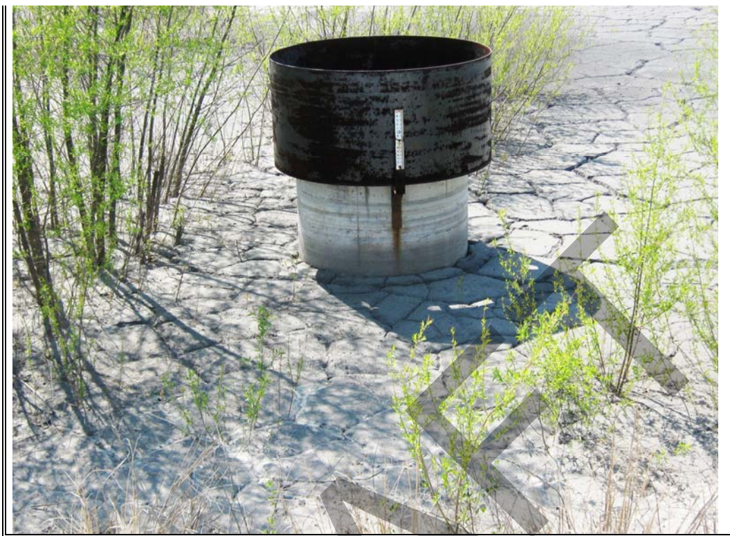
Photograph 60: Vertical riser and skimmer for ash pond discharge. Ash level is approximately 38 inches below top of riser.
