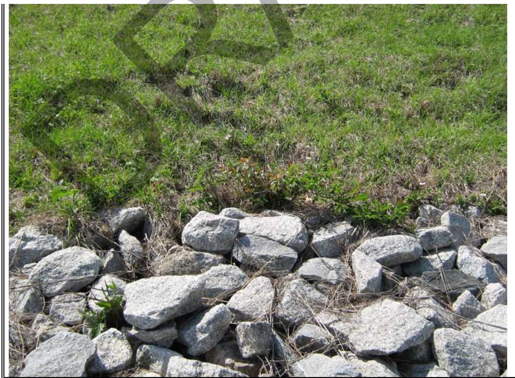
Photograph 55: Local spot in North Pond dike rock toe – soil slope where slight loss of material. Typical of conditions addressed as necessary by Plant.
