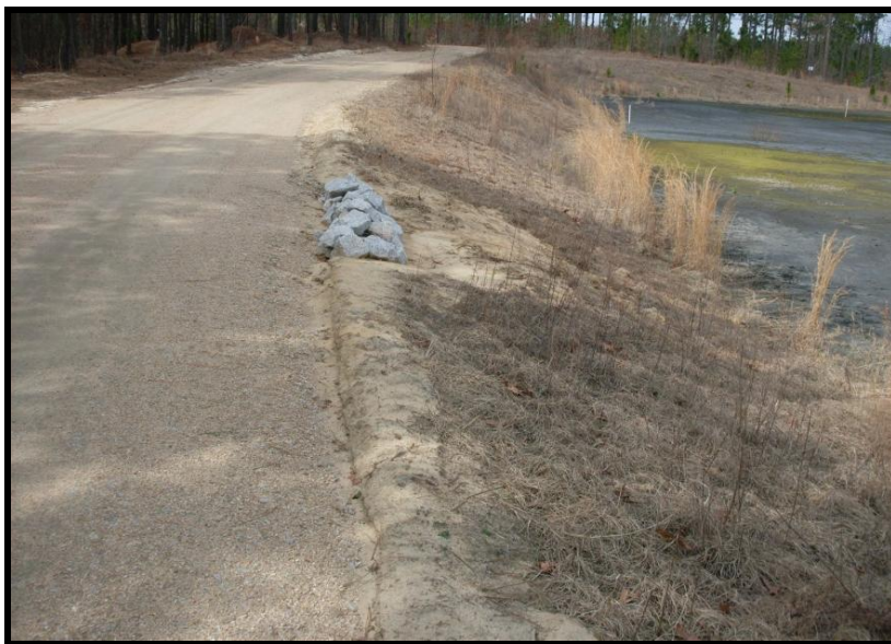
Photograph 5.2. Minor erosion at the upstream edge of crest at south side of embankment, looking west.
