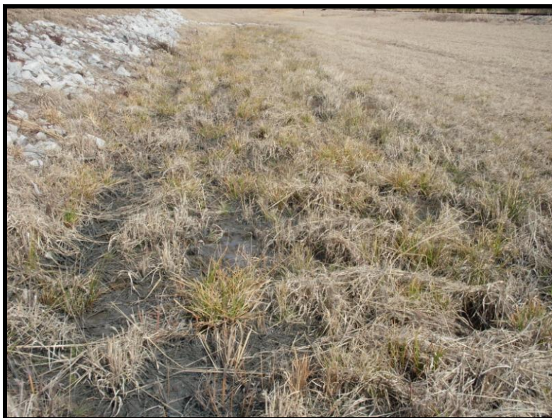
Photograph 5.6b. Wet soils in shallow swale along right (south) toe of dike embankment, looking north.
