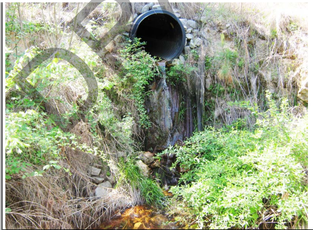
Photograph 61: Outlet end of discharge facility. Stormwater from Darlington Plant also discharges from this pipe.
