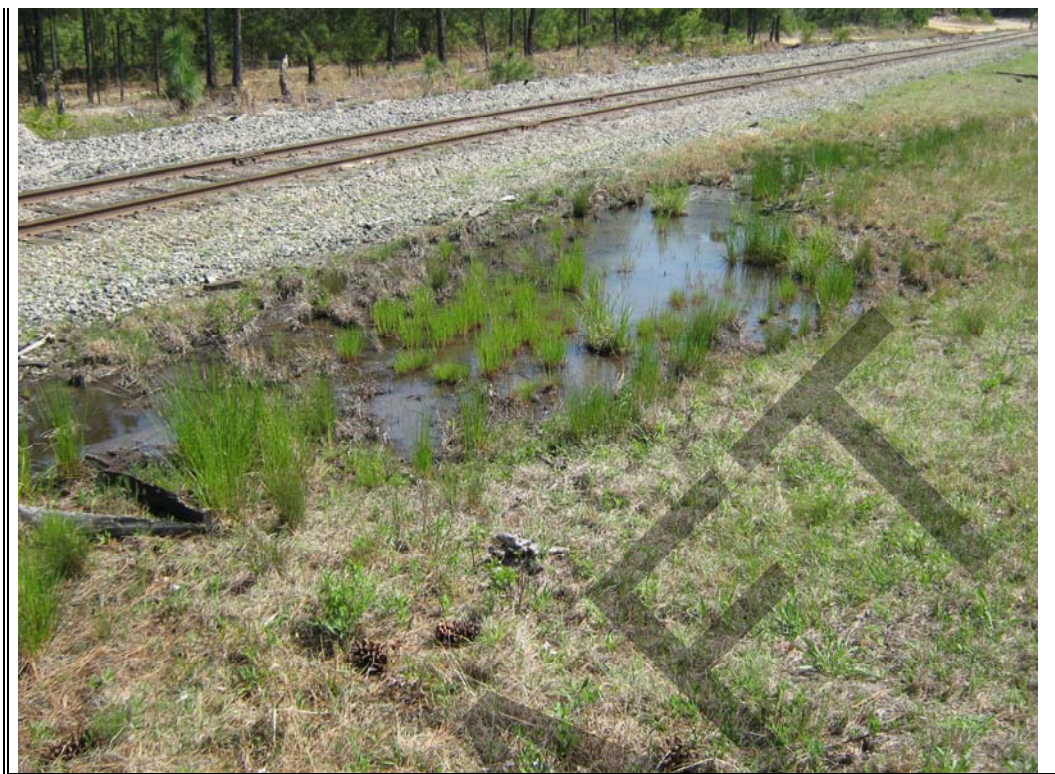
Photograph 58: Standing water adjacent to railroad in topographic low area. A normal condition not related to seepage.
