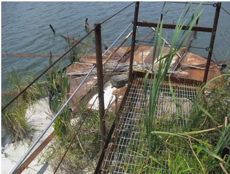
Photo 9: riser and skimmer at stilling pool, Photo: 079, 6/3/09
