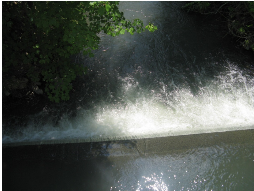
Photo 11 concrete overflow weir spillway, Photo: 068, 6/3/09
