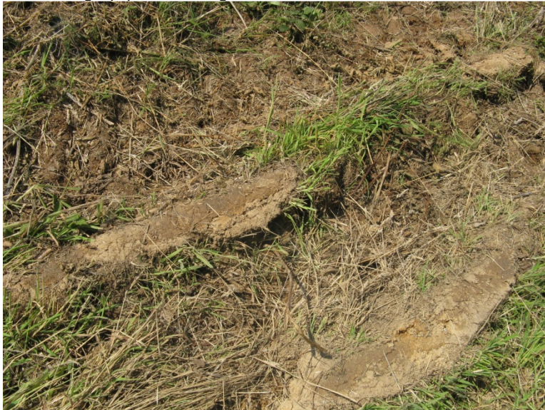
Photo 4: Mowing Equipment Rutting, Downstream Embankment, Photo: 007, 6/3/09
