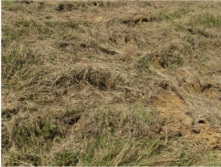
Photo 3: Bare Areas and Straw Build Up, Downstream Embankment, Photo: 004, 6/3/09
