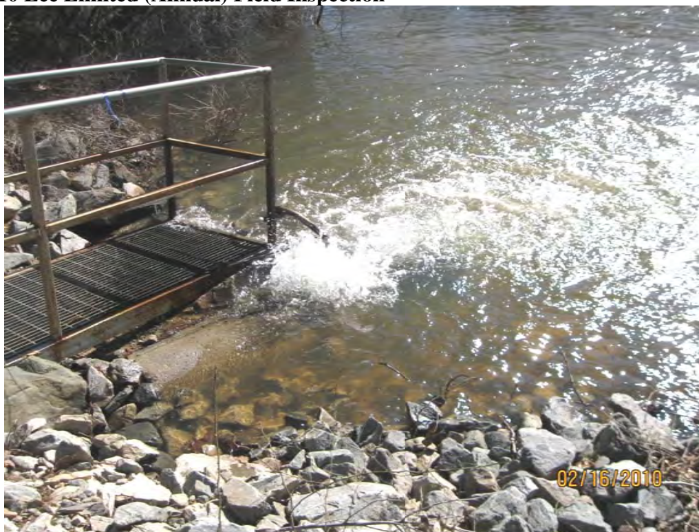
9. Ash Pond Dike – View of discharge from secondary settling basin at Neuse River.
