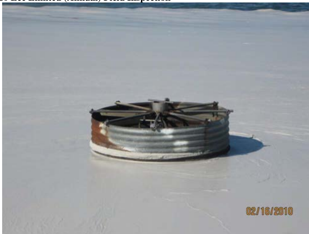
7. Ash Pond Dike – View of skimmer for ash pond discharge.
