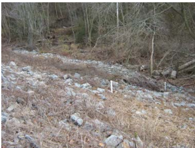
Riprap at seepage location that was repaired
