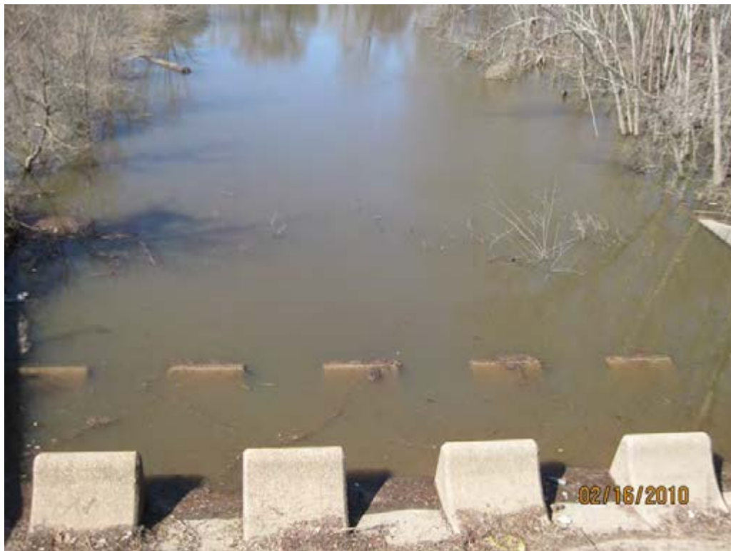
11. Cooling Lake Dike – View of energy dissipation blocks and downstream spillway channel with high tailwater conditions.
