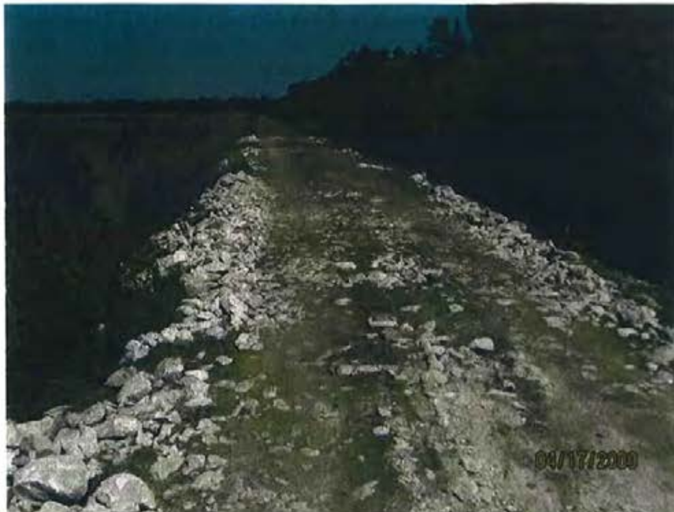
5. Crest condition 4-17-09. Additional cleanup of rip rap needed.
