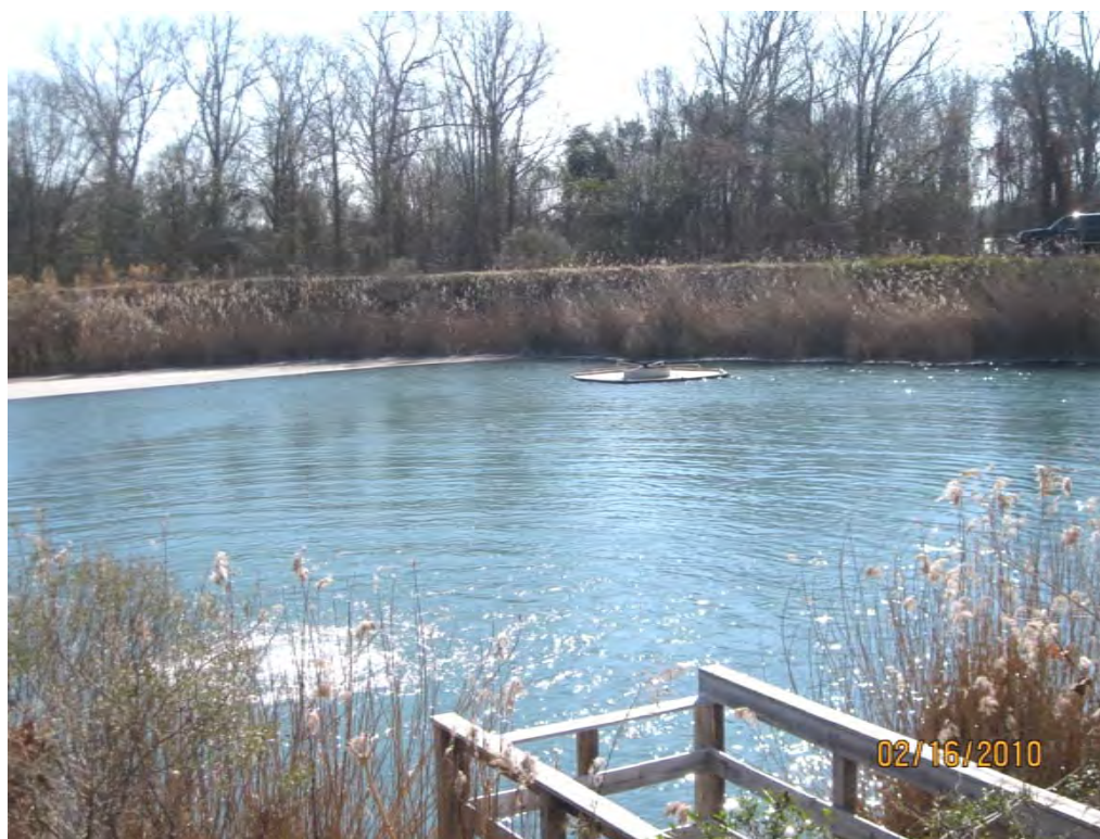
8. Ash Pond Dike – View of secondary settlement basin and skimmer for discharge riser. Turbulence is from ash pond discharge
