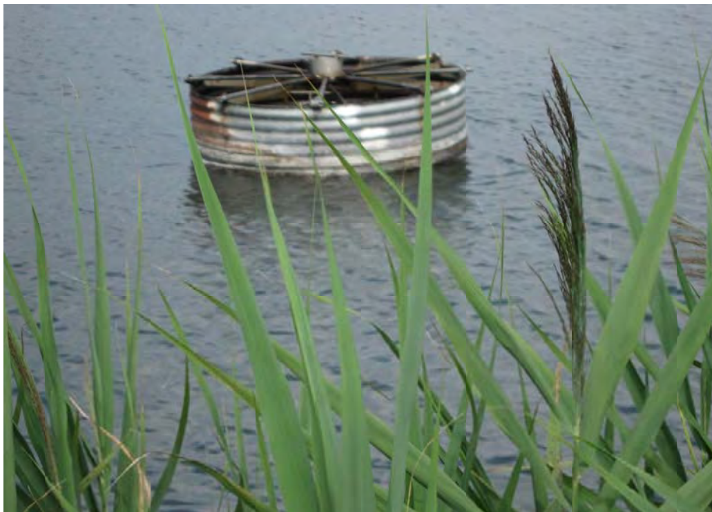
36. ASH POND-Skimmer structure on ash pond riser.
