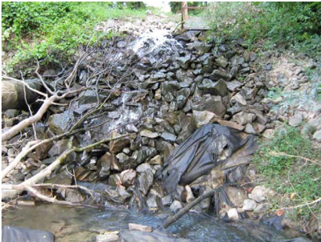
37. ASH POND-Discharge point for secondary settling pond outfall.
