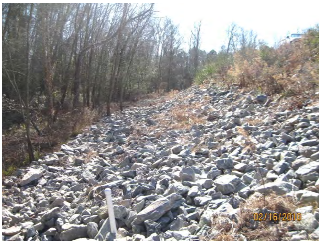
6. 6 Ash Pond Dike – View of riprap placed along toe of outside slope for secondary settling basin.
