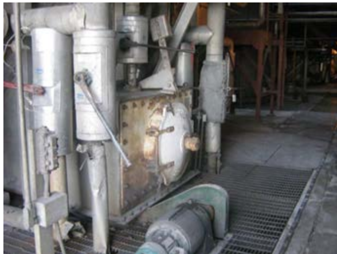
Boiler where boiler slag is discharged
