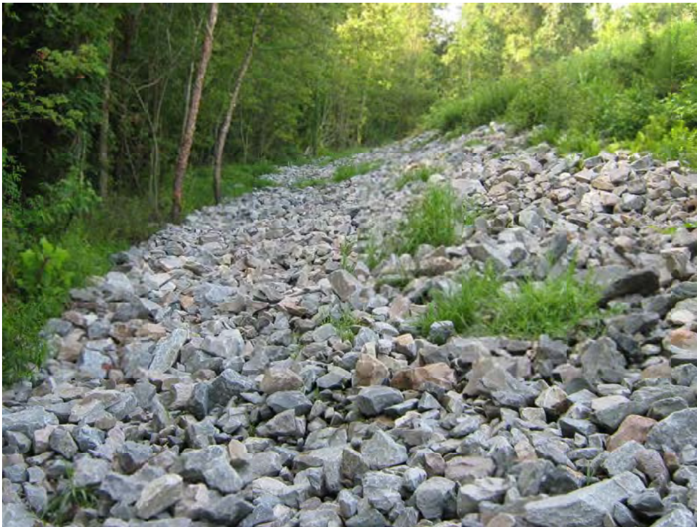
32. ASH POND- Drainage blanket at secondary settling pond-east slope
