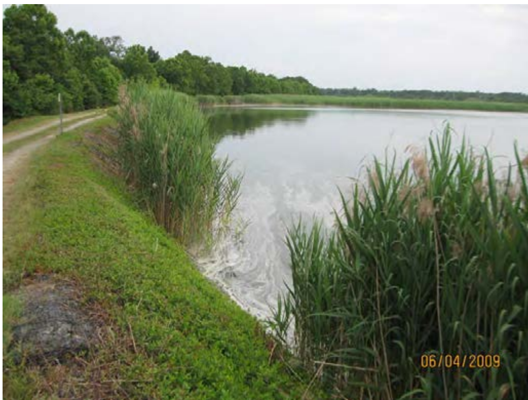
26. ASH POND- Interior slope of south dike. Note vegetation on erosion matting.
