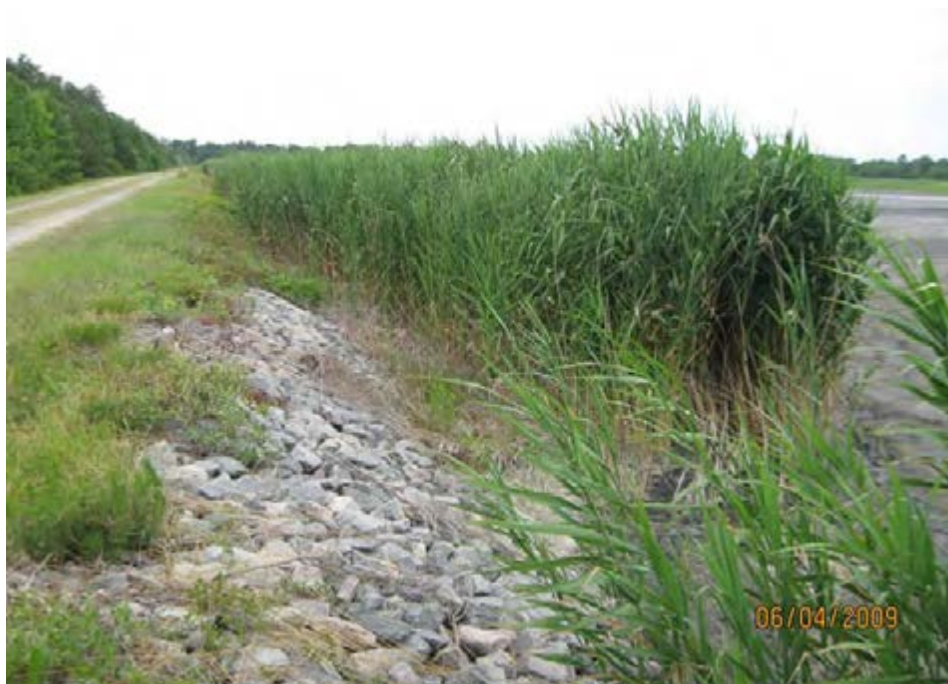
22. ASH POND- Crest and interior slope-east dike. Note good conditions of rip rap repair.
