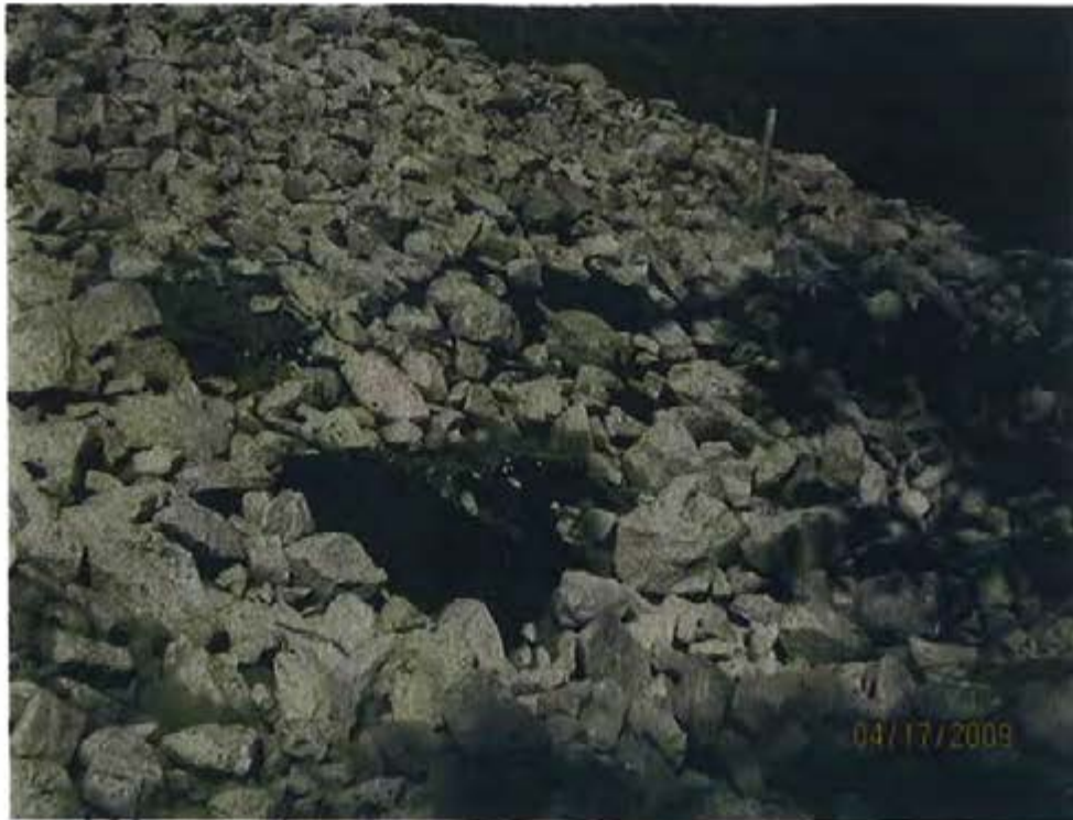
3. Areas within completed rip rap blanket where additional rip rap is needed 4-17-09.
