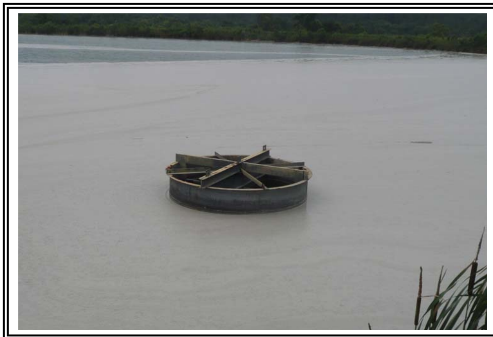
Outlet structure in the 1985 Ash Pond.
