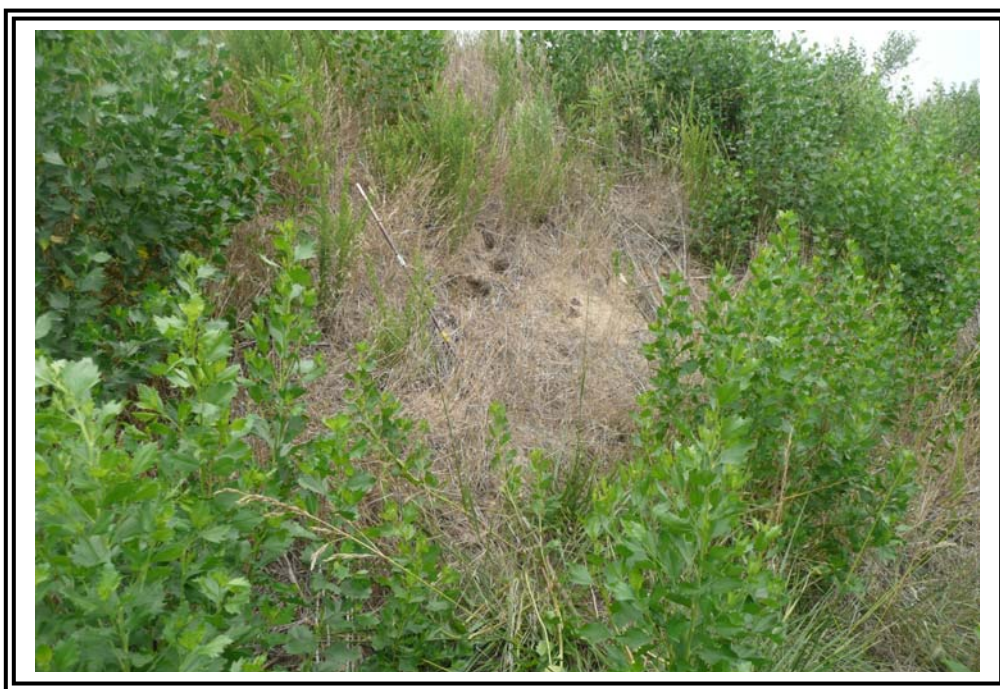
Scarp about 3 to 4 feet high near the top of the 1985 Ash Pond West Dike.
