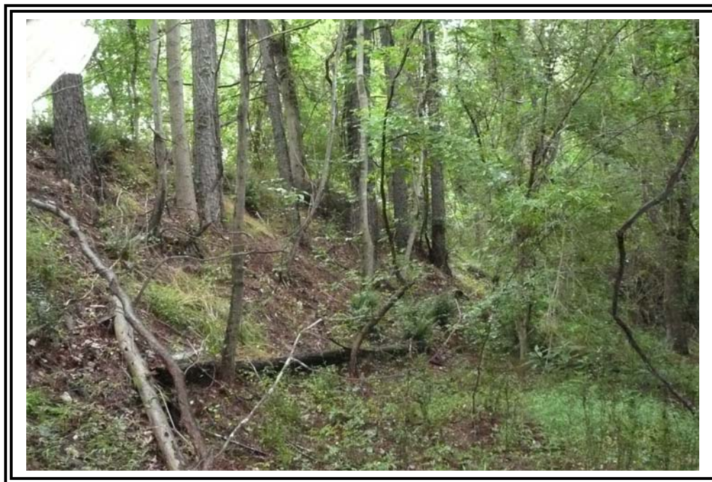
1970 Ash Pond downstream slope near southwest corner.
