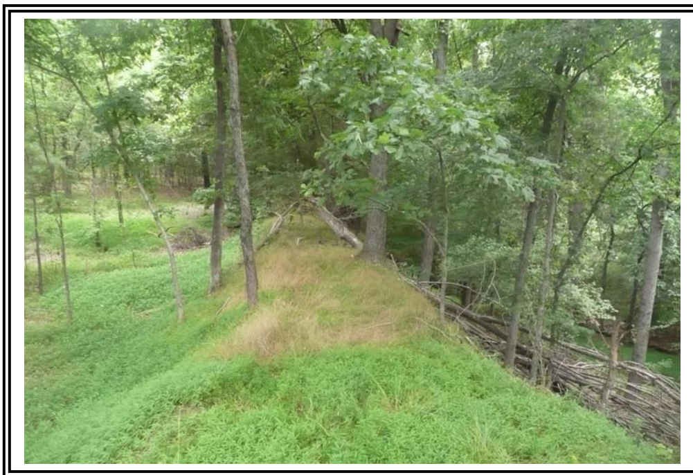
Crest of the 1956 Ash Pond Dike.
