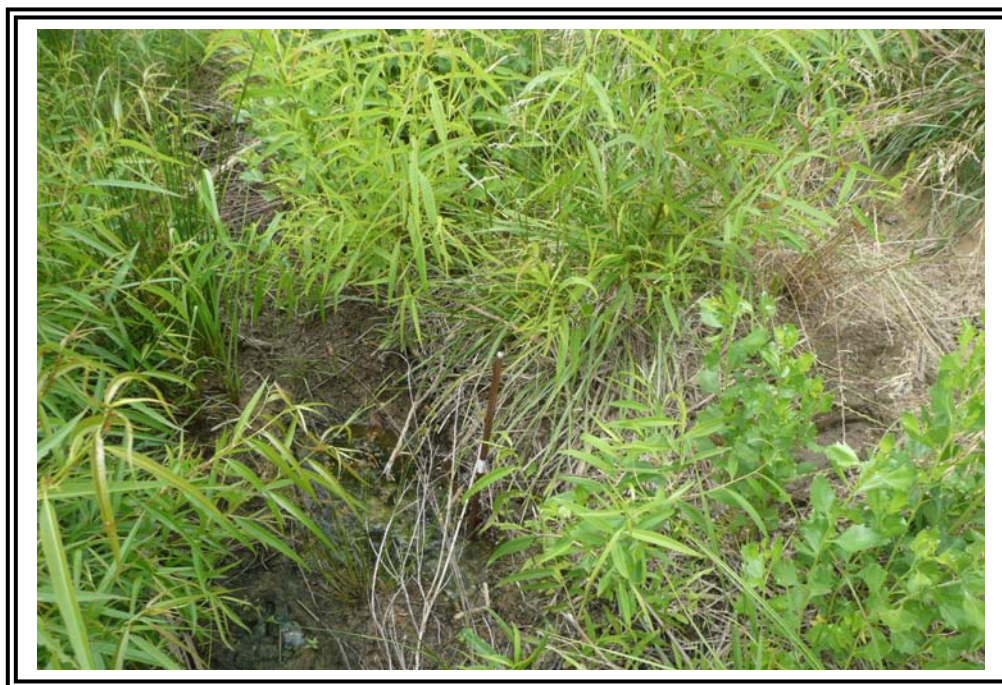
Soft soil at the toe of the 1985 Ash Pond West Dike. Probe pushed into the ground about 2 feet.
