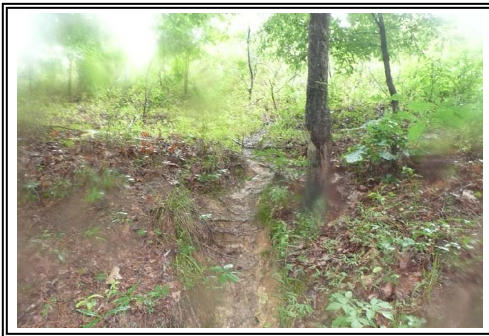
Animal slide (likely beaver or muskrat) on the downstream slope of the 1978 Ash Pond Dike.
