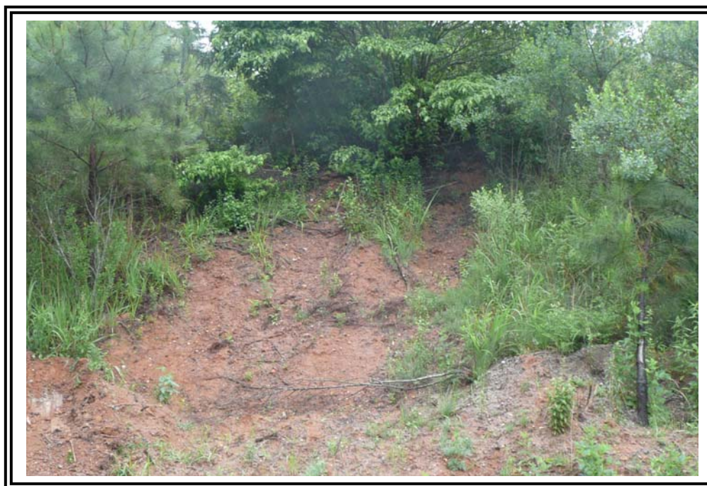
Example of poor vegetative cover, erosion, and probable human activity on the downstream slope of the 1978 Ash Pond Dike.
