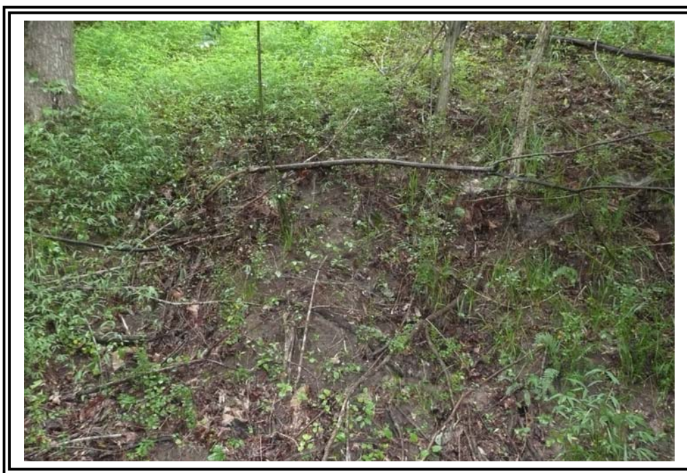
Surface erosion on 1970 Ash Pond west dike downstream slope.
