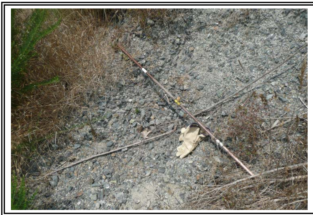
Stone filled erosion and /or abandoned rodent hole on the 1985 Ash Pond West Dike. Progress Energy reports filling rodent holes and erosion features with gravel.
