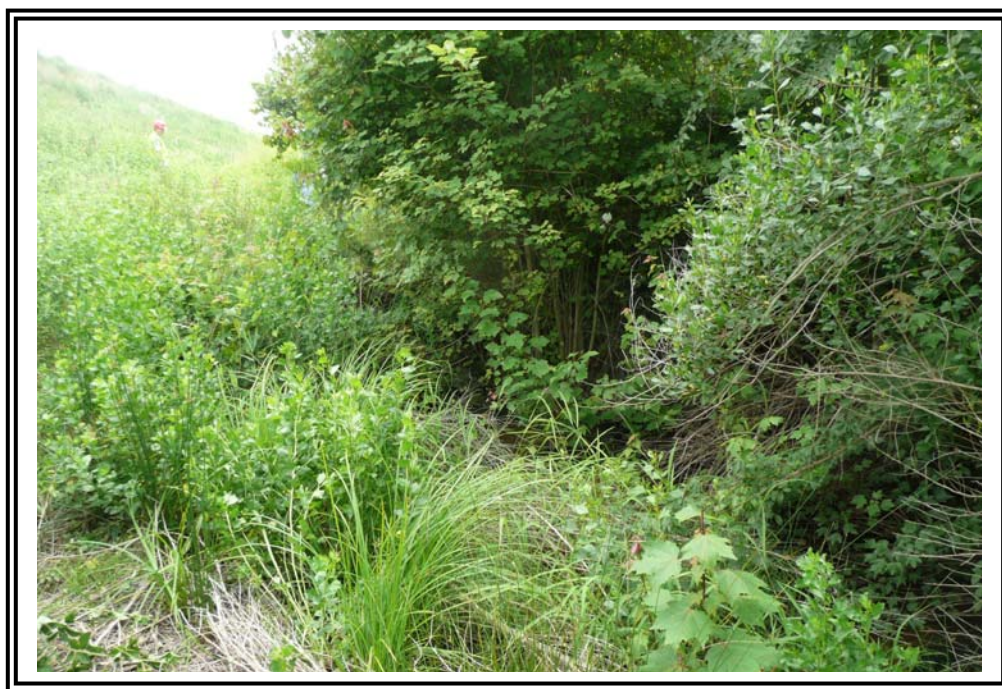
Tree growth at the toe of the 1985 Ash Pond West Dike.
