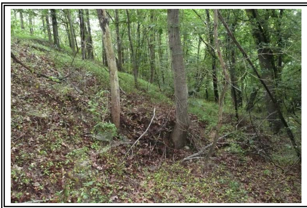
Steepened conditions on 1963 Ash Pond west dike from surface erosion and sloughing from the partially repaired 1982 slide.
