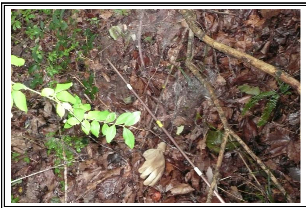
Erosion feature along 1970 Ash Pond west dike toe. Work glove placed below 4' probing rod supported at edge of feature for scale purposes.
