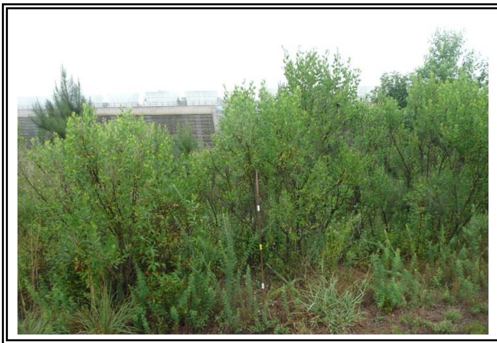
North end of 1978 Ash Pond Dike, downstream slope is covered with large brush.
