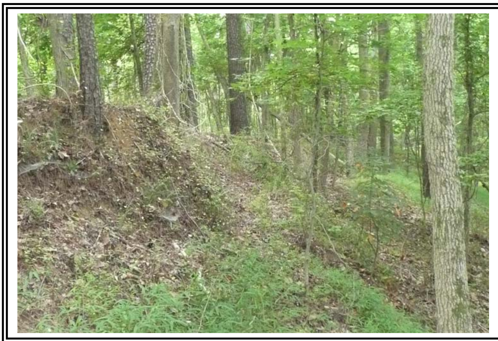
Typical of frequent areas of erosion on the downstream slopes of the 1956 Ash Pond Dikes.
