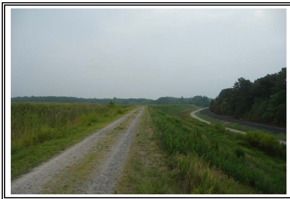
West Dike crest of the 1985 Ash Pond, looking southeast. Note: "Pond within a pond" to the upstream side of the crest. Ash in 1985 Ash Pond approximately at the crest of the dike.
