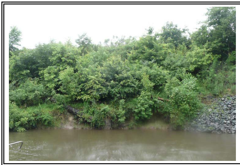
Erosion at the toe of the 1978 Ash Pond at discharge canal. Also note the fallen tree.
