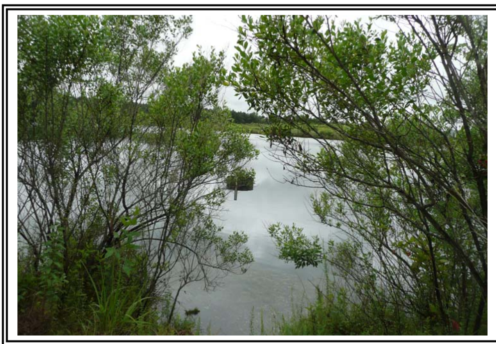
Outlet structure in 1978 Ash Pond.
