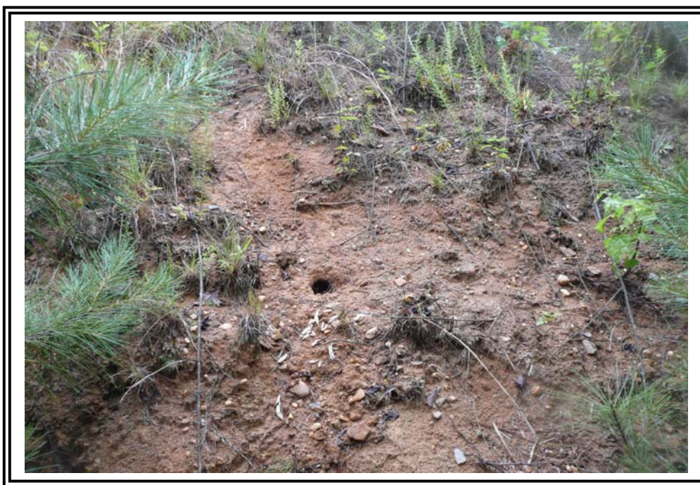
Evidence of animal burrow at the south end of the 1978 Ash Pond Dike.
