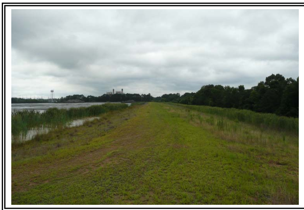
North Dike of "Pond within a pond" crest. Notice ash stockpiles within the pond.
