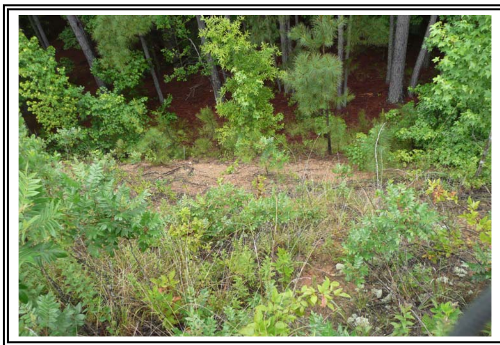
Downstream slope of the 1978 Ash Pond Dike. Note: Rows of trees are immediately beyond the toe.
