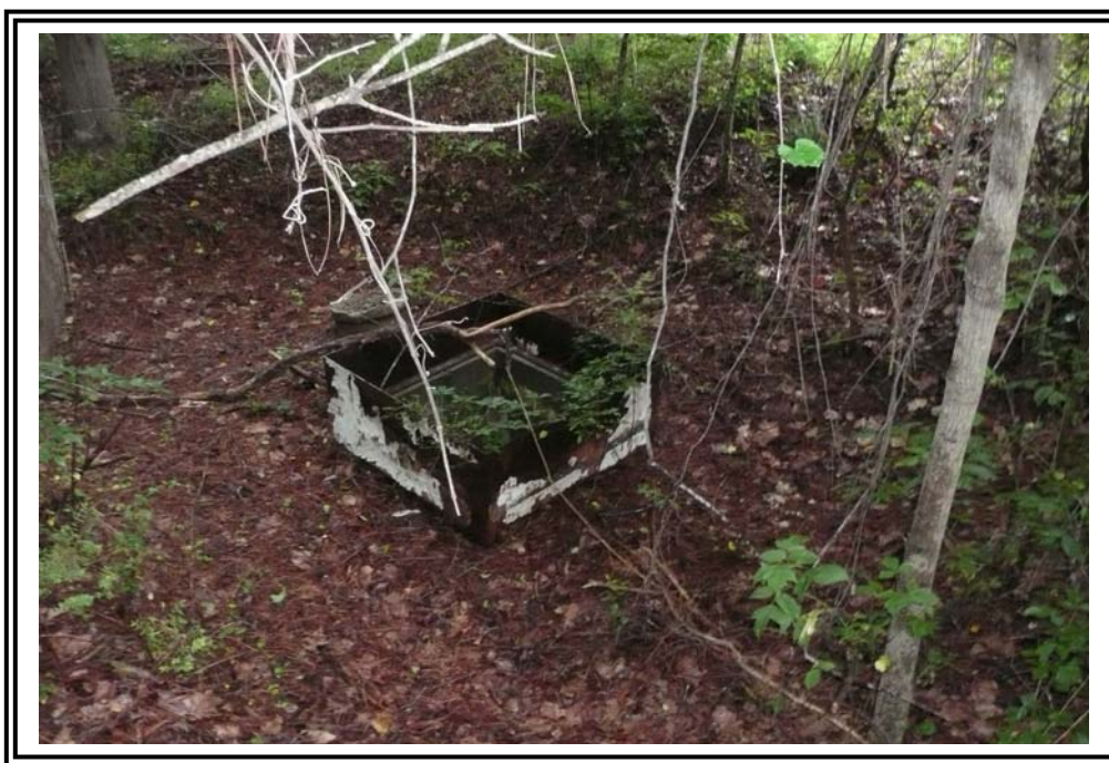
1970 Ash pond outlet control structure. Note: water level in south end of pond was several feet lower than outlet during our visit.
