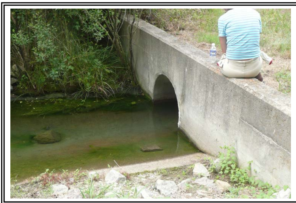
Culvert under the access road at the toe of the 1985 Ash Pond West Dike outlet channel.
