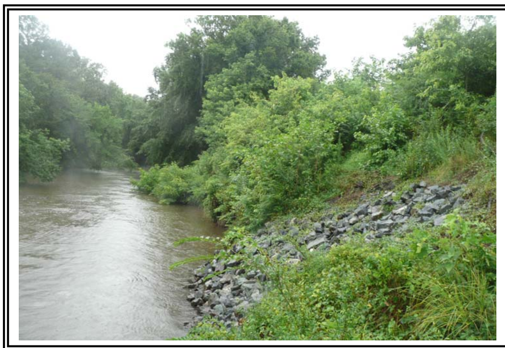
Rip Rap fill at the toe of the 1978 Ash Pond Dike along the discharge canal.
