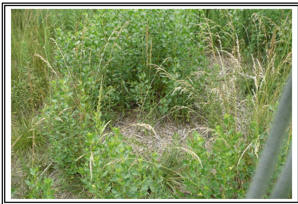
Sparse and weedy vegetation cover on the 1985 Ash Pond West Dike.
