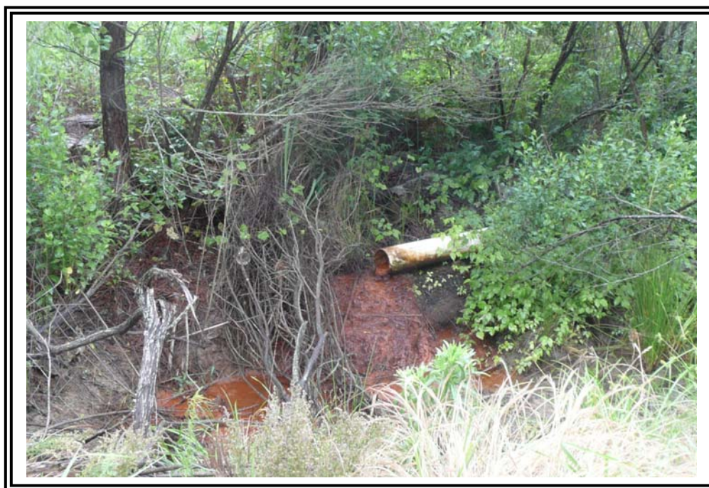
Apparent trench/field drain outlet at north dike toe on 1978 pond adjacent to cooling towers
