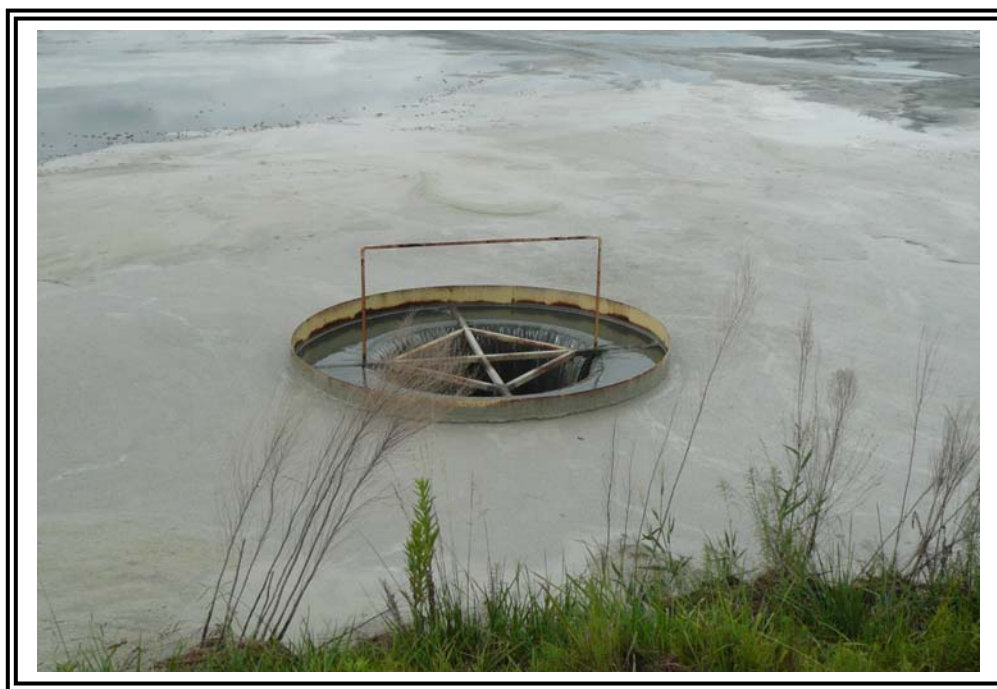
Close up of the outlet control structure in "Pond within a pond".
