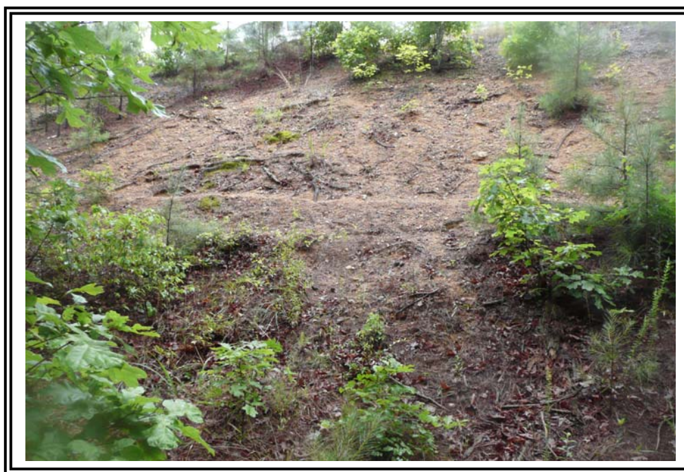
Downstream slope at the south end of the 1978 Ash Pond Dike is devoid of vegetation.
