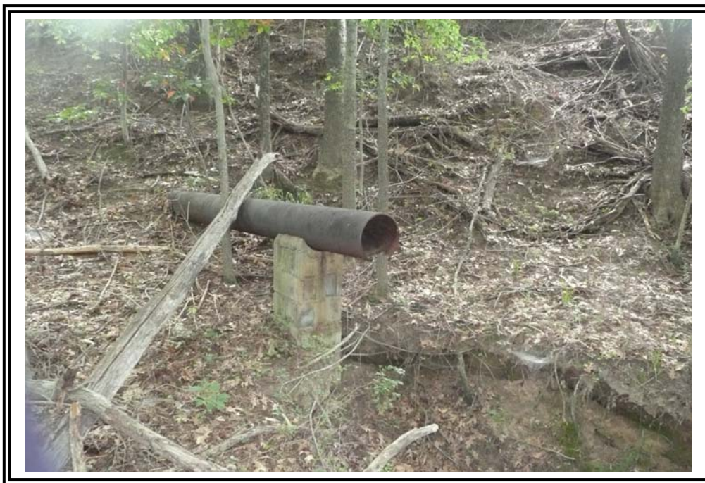
Former outlet pipe from 1956 Ash Pond. Pond no longer contains free water.
