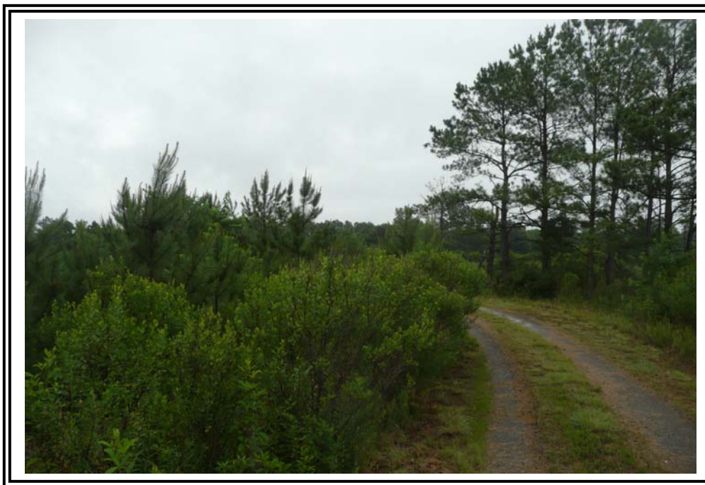
North end of 1978 Ash Pond Dike crest. Brush and small Pine trees are in the left of the photo and are on the downstream slope. Tall Pine trees on the right of the photo are in deposited ash within the pond.
