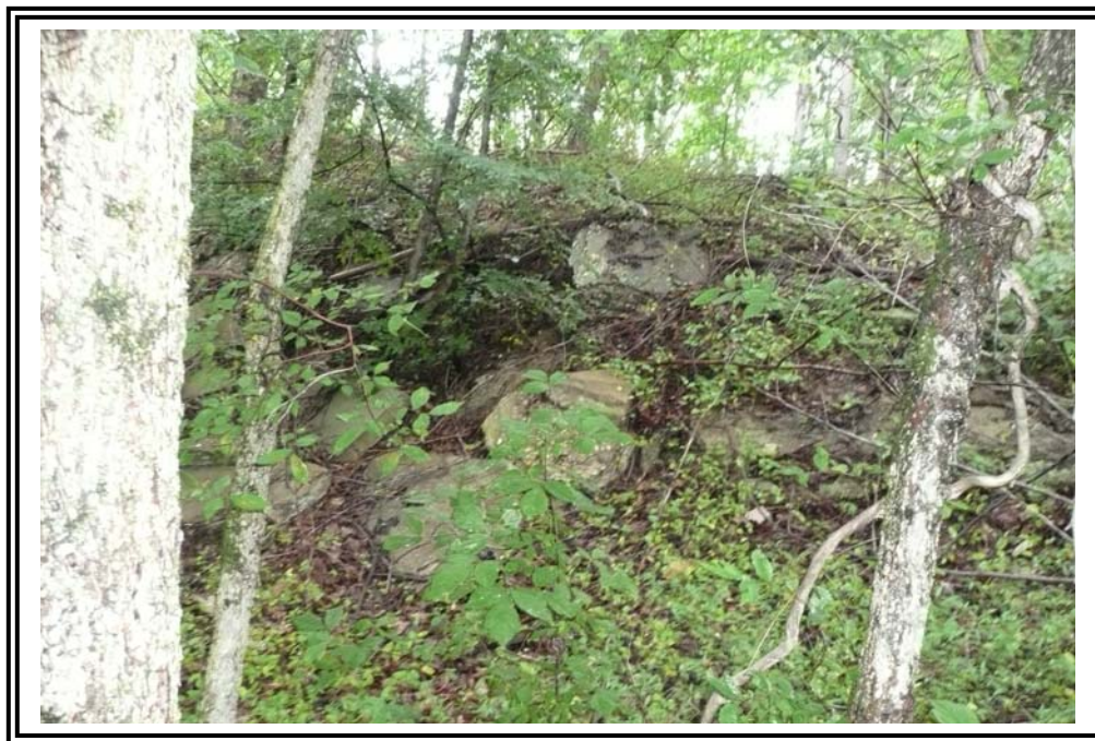
1970 Ash Pond downstream slope near outlet structure..
