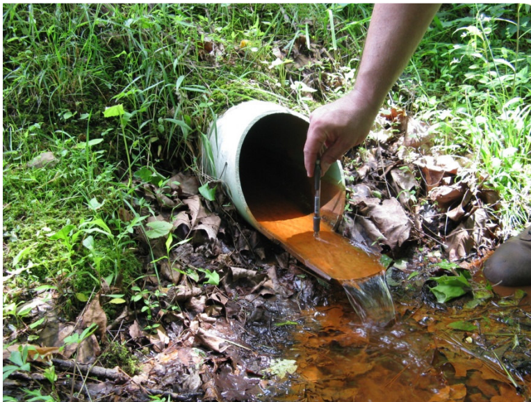
Photo 9: 1964 Dam – Internal Drain, Toe, Photo: 081, 5/29/09
