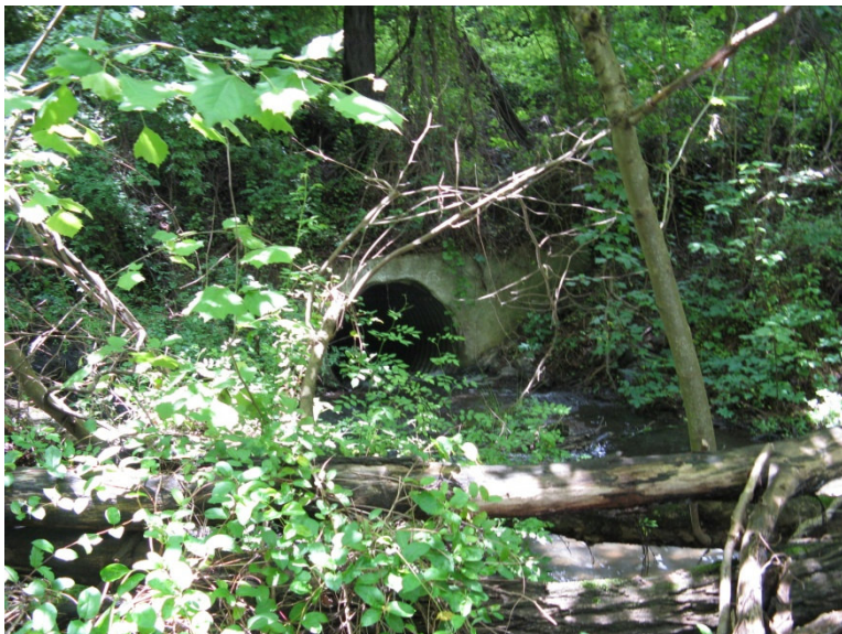
Photo 8: 1964 Dam - 60" CMP Underneath I-26, Toe, Photo: 087, 5/29/09
