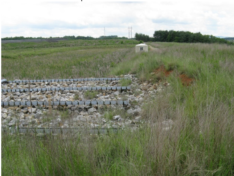
Photo 2: 1964 Dam - Upstream Wetland, Crest, Photo: 053, 5/29/09
