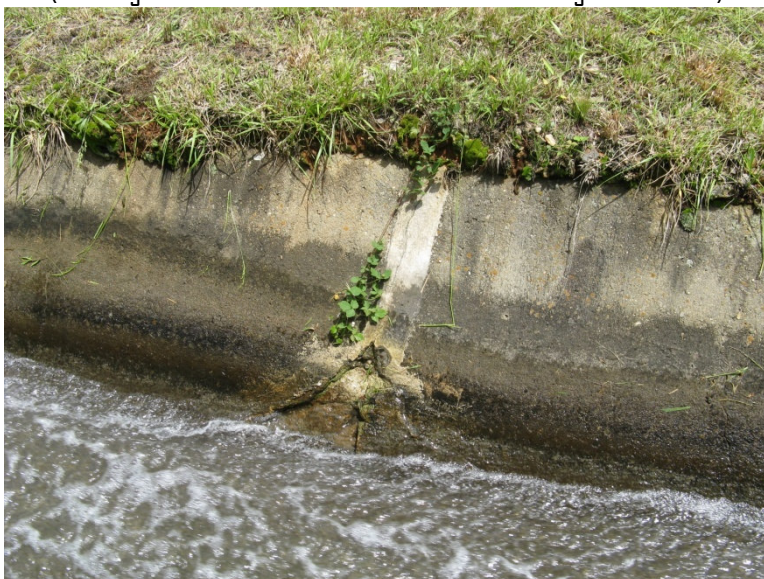
Photo 6: 1964 Dam - Concrete Flume Deterioration, Right Groin, Photo: 090, 5/29/09 (note: right and left are based on the observer facing downstream)
