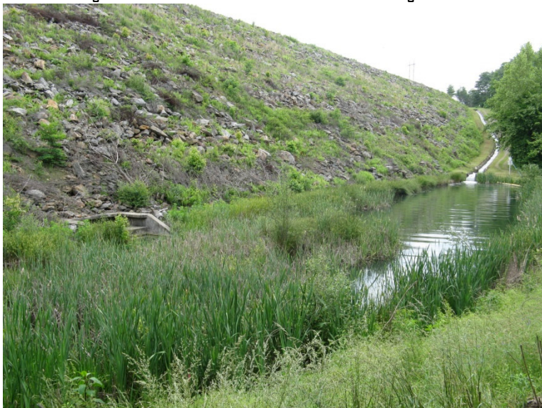
Photo 5: 1964 Dam - View of Stilling Pond/Embankment Right Groin, Toe, Photo: 063, 5/29/09 (note: right and left are based on the observer facing downstream)
