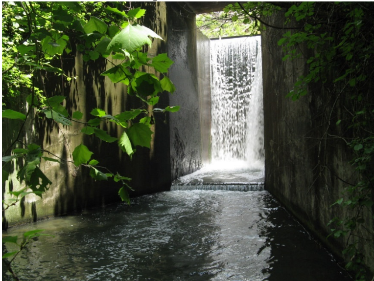
Photo 7: 1964 Dam - Stilling Pond Outfall, Toe, Photo: 086, 5/29/09
