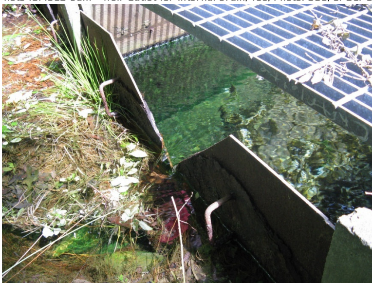
Photo 10: 1982 Dam - Weir Outlet for Internal Drain, Toe, Photo: 006, 5/29/09
