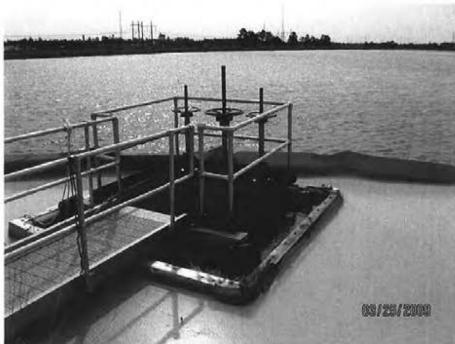
14. 1984 Ash Pond (Interior Storage Area) – View of discharge structure.
