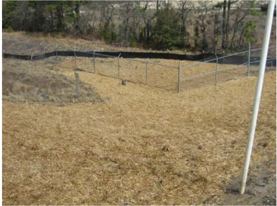
Repair along downstream east slope
