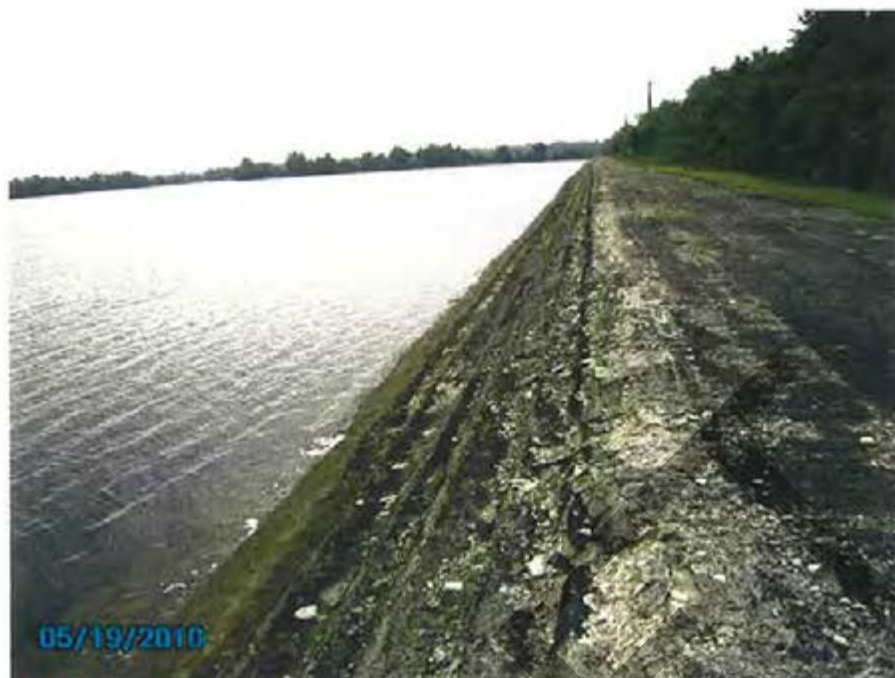
35. Cooling Pond – (Bay #5) View of crest and interior slope looking east.
