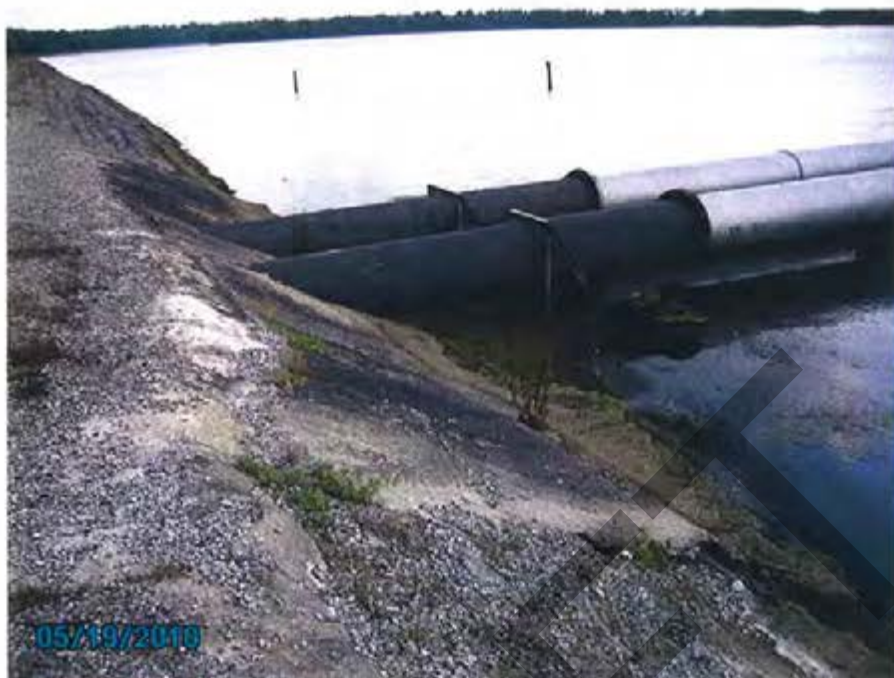
32. Cooling Pond – (Bay #4) View of makeup discharge pipes on upstream side of dike.
