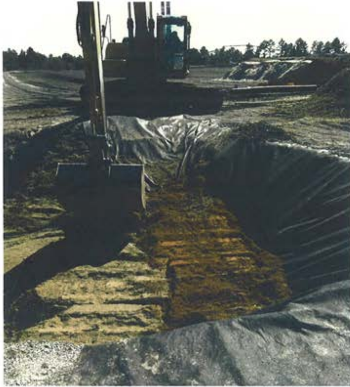
Photo 3. Sand and clay fill nearing top of repair zone.
