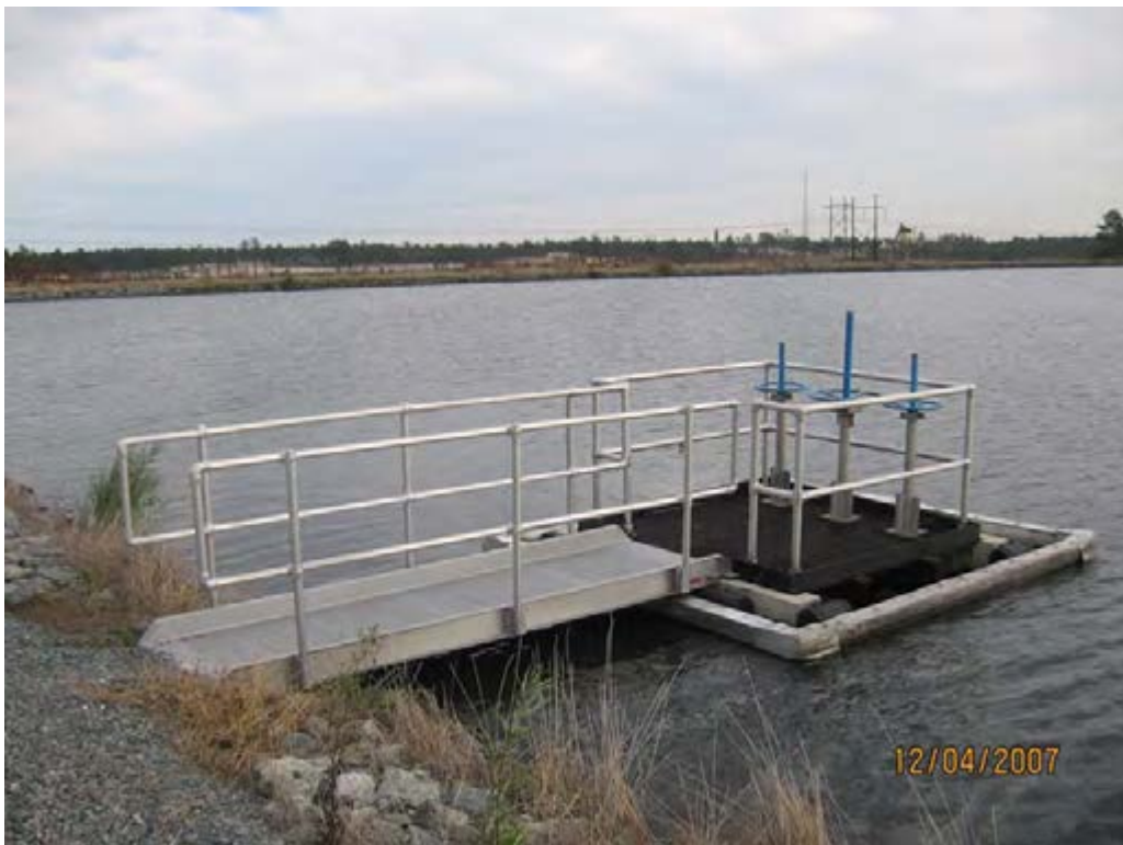
Photo 8. 2006 Interior Ash Pond Inlet looking east.
