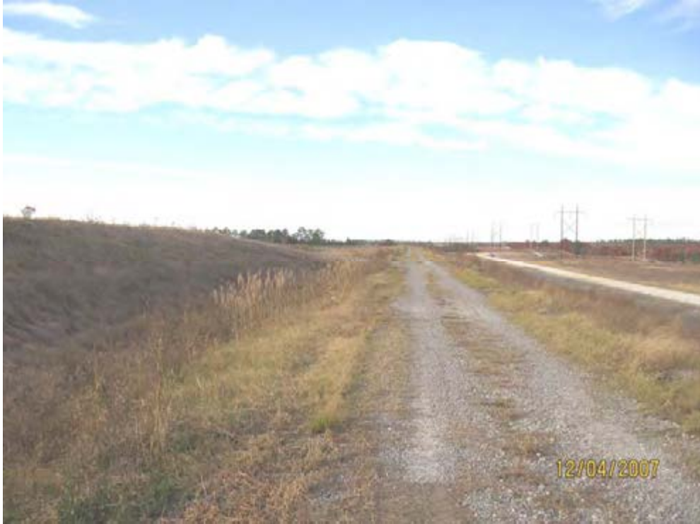
Photo 3. 1984 Ash Pond – Crest of 1984 dike and exterior slope of 2006 dike.
