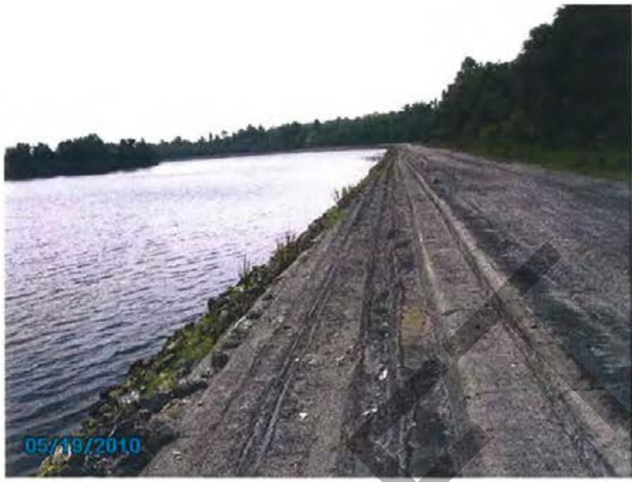
30. Cooling Pond – (Bay #3) View of crest and interior slope looking south.
