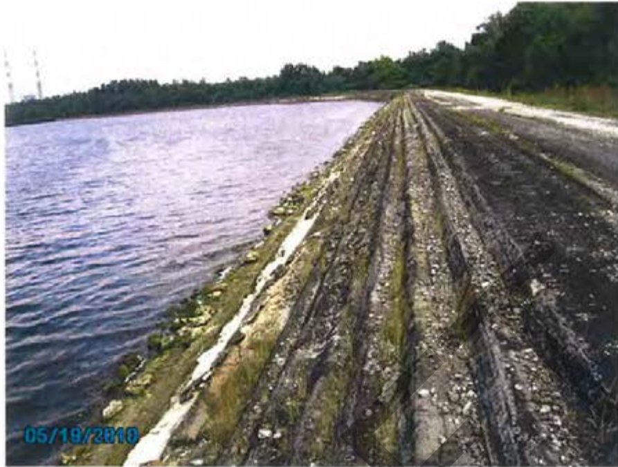
28. Cooling Pond – (Bay #2) View of crest and interior slope looking south.
