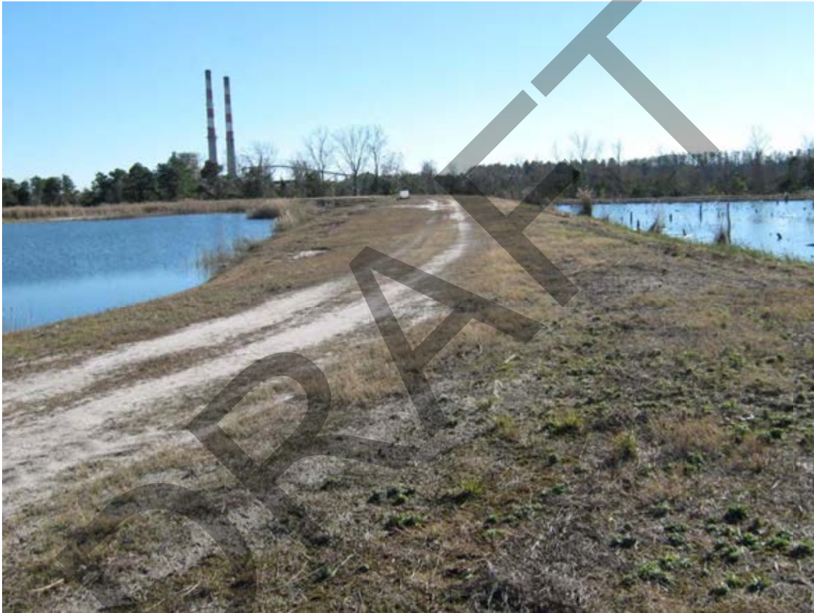
1983/1971 Ash Pond – View of containment berm for interior storage area (12/15/10)
