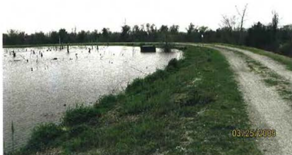
1. 1983 Ash Pond – View of interior slope, outlet riser and standing water near riser.
