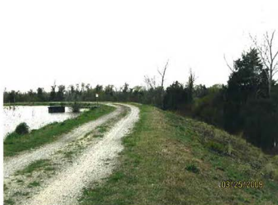
2. 1983 Ash Pond - View of dike exterior slope near outlet riser
