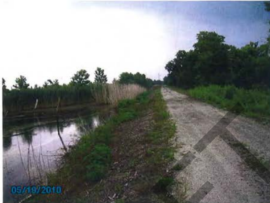
3. 1983/1971 Ash Pond – View of interior slope for south dike.
