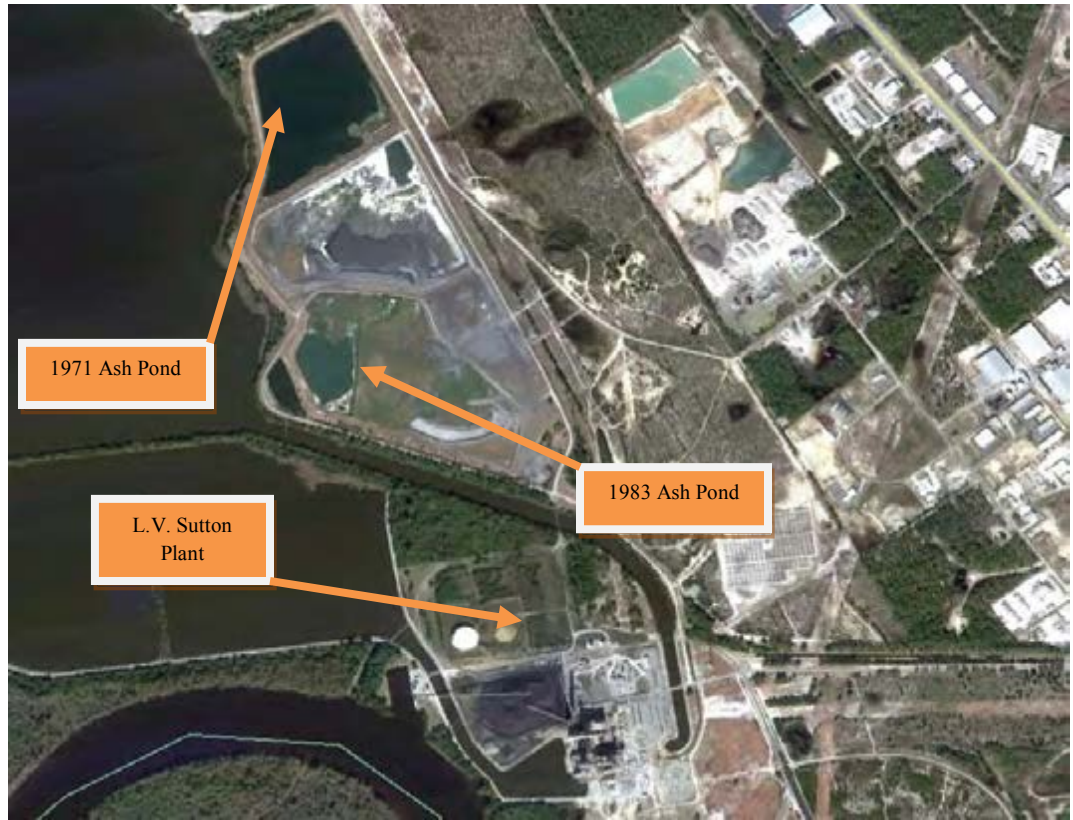
Figure 2.1b: L.V. Sutton Steam Electric Plant Aerial View
