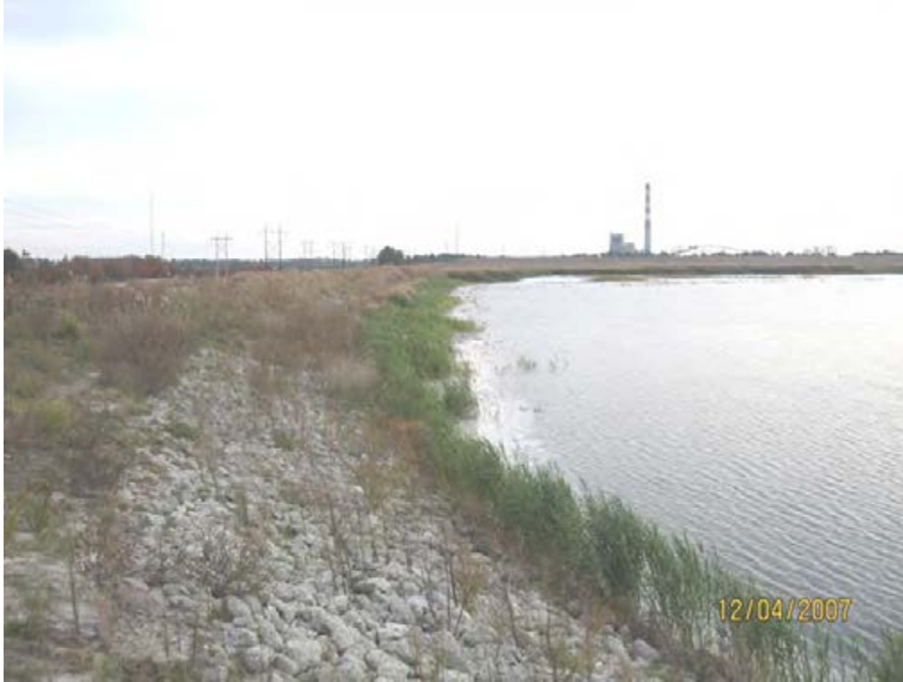
Photo 5. 1984 Ash Pond – Typical interior slope looking south. Note minor grass growth.
