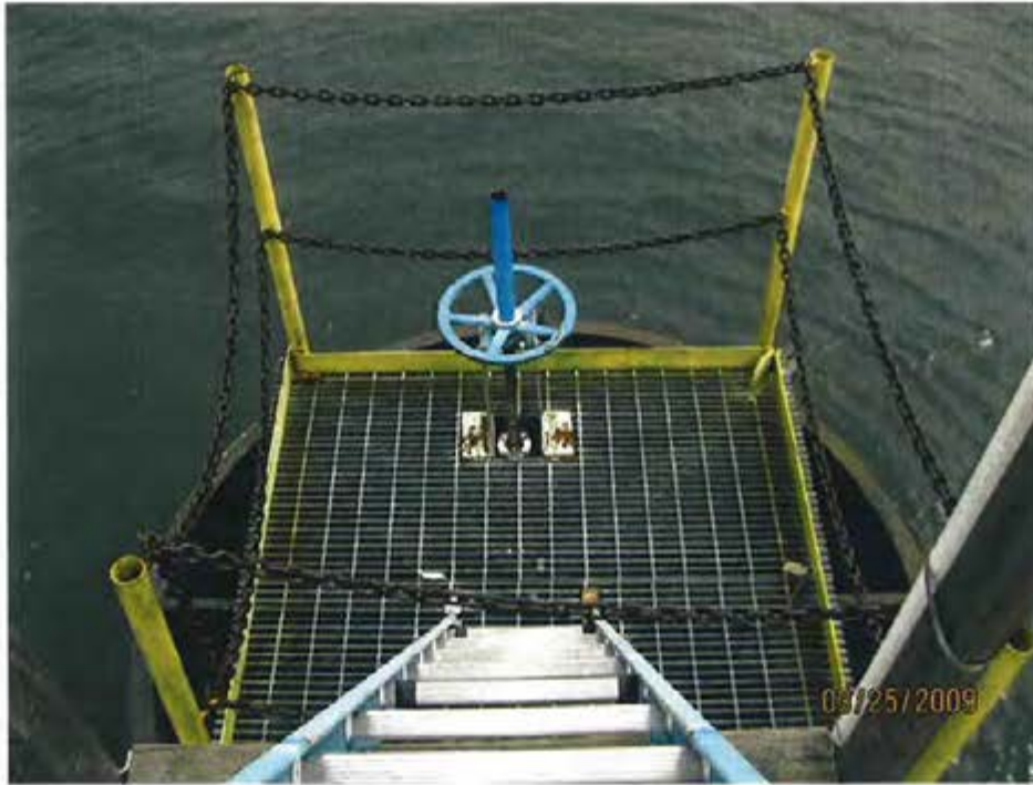
11. 1984 Ash Pond – View of top for discharge riser.
