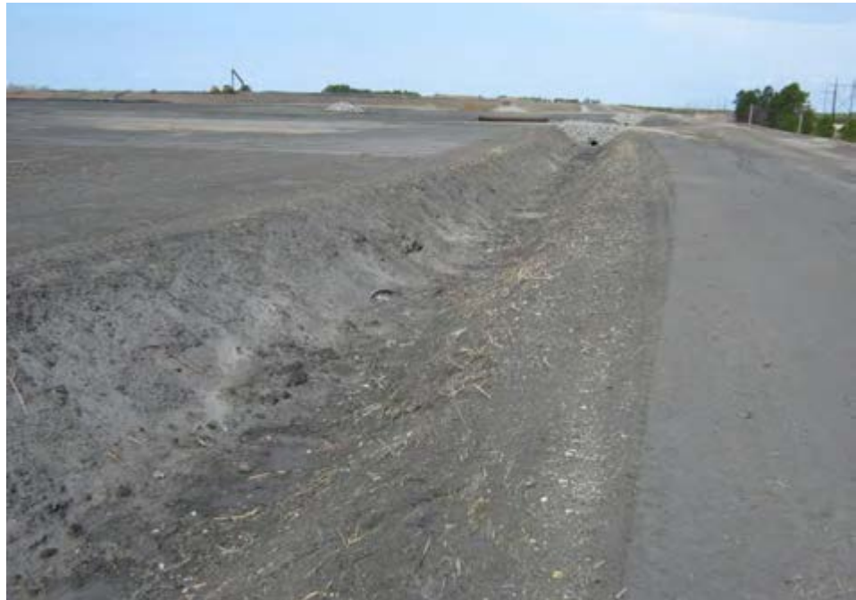
Upstream slopes to be vegetated, Spring 2011
