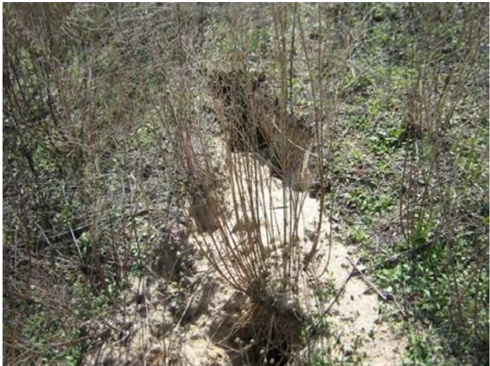
Animal burrows along downstream slope, 1984 Ash Pond
