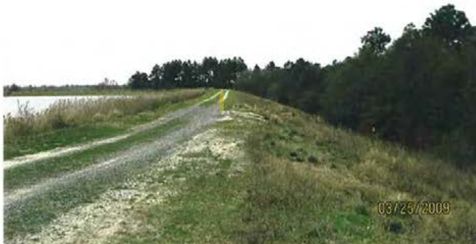
8. 1984 Ash Pond – View of exterior slope on north side of pond.
