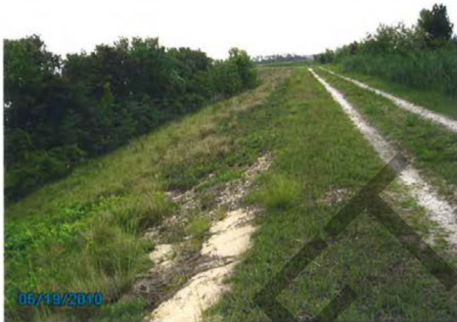
15. 1984 Ash Pond – View of exterior slope for west dike looking north.
