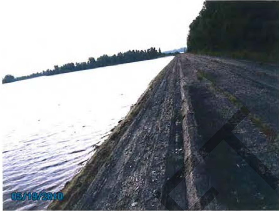
33. Cooling Pond – (Bay #4) View of crest and interior slope looking south.
