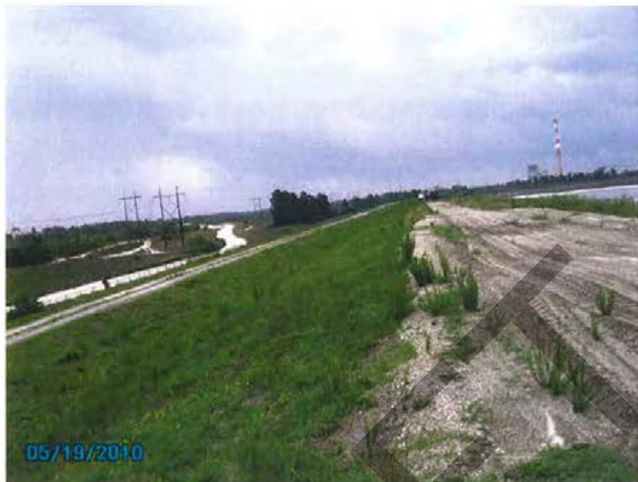
7. 1984 Ash Pond – View of exterior slope for east dike looking south (at northeast corner).
