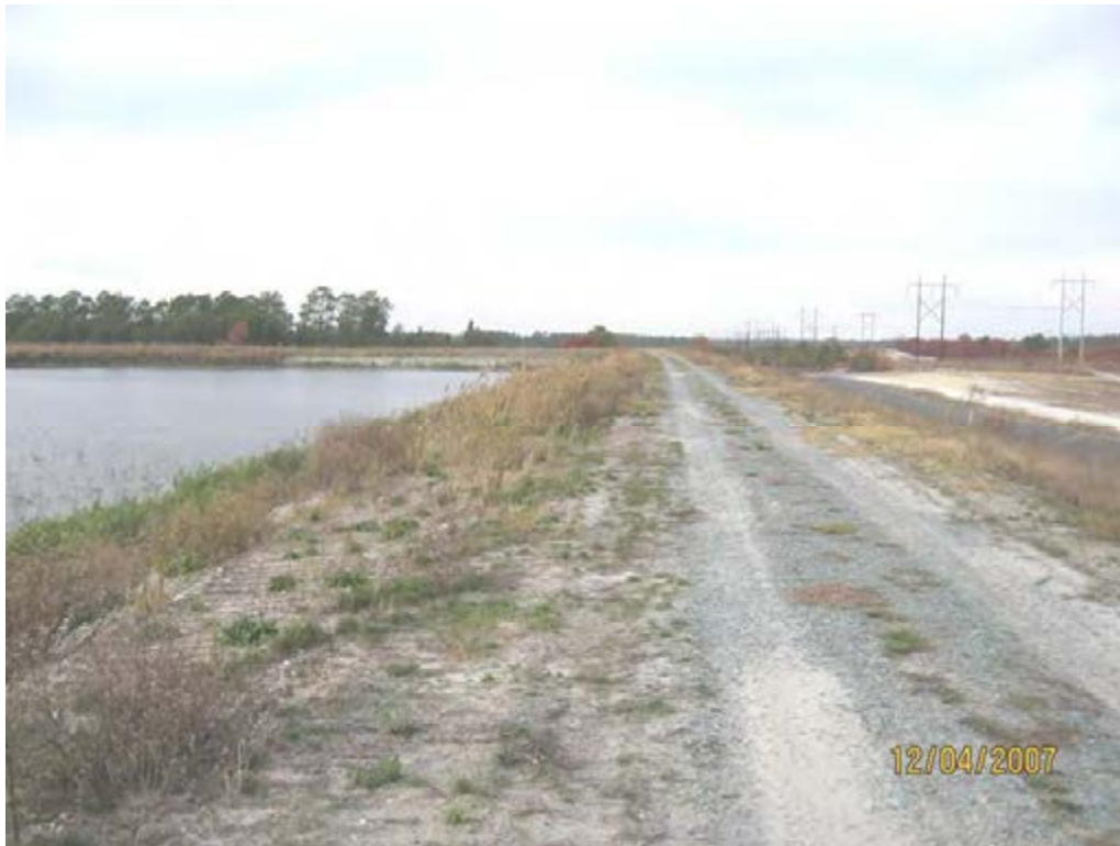
Photo 4. 1984 Ash Pond – Crest and interior slope looking north.
