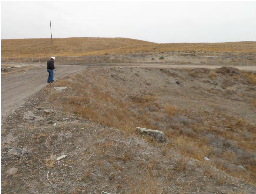
Photo 15: 4B Ash Pond east embankment dam downstream side. Topographic depression to right.
