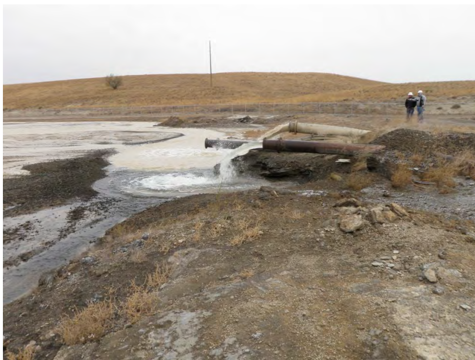
Photo 17: 4B Ash Pond inlet pipes at east margin of pond.
