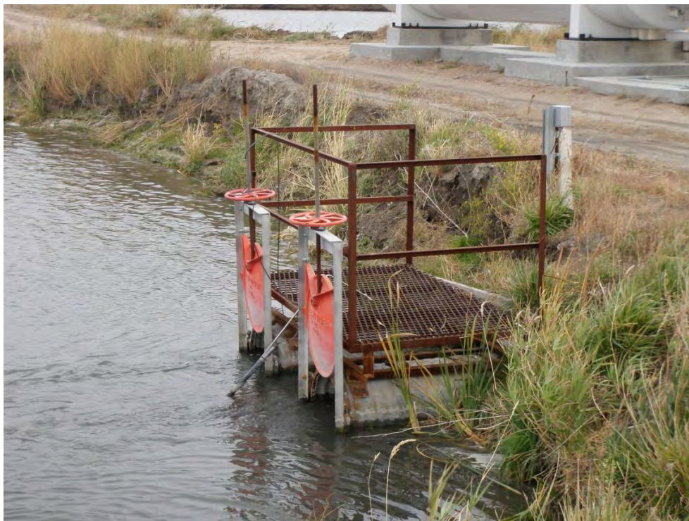
Photo 42: Intake culverts at southeast corner of 1A Clear Pond. Water flows from 1A to 1B Clear Pond through the interior dike and is treated with CO 2 to adjust pH.
