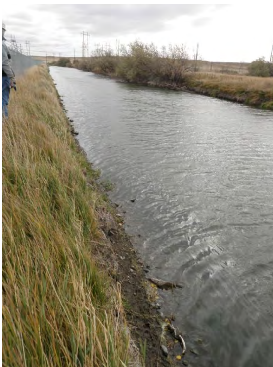
Photo 48: 1A / 1B Clear Pond south embankment dam downstream looking southeast showing steep downstream slope and Recirculation Canal.
