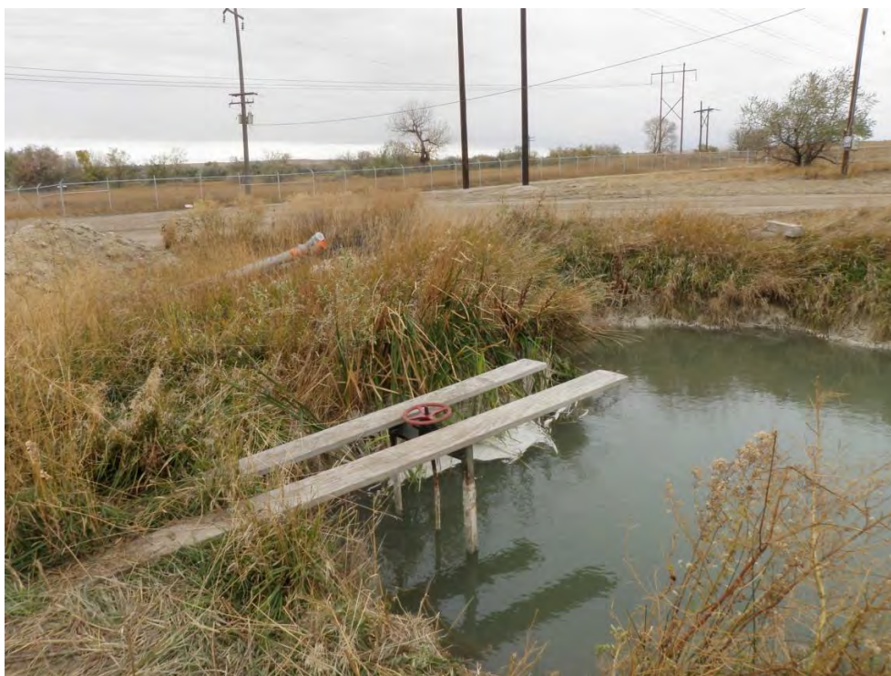
Photo 35: Blowdown Canal southwest corner showing outlet valve (discharge to 1B Ash Pond).
