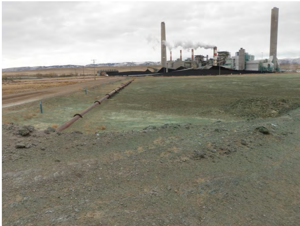
Photo 8: 4A Ash Pond east embankment dam upstream side looking south. Note that pond is full of CCW solids and not currently receiving wastewater.
