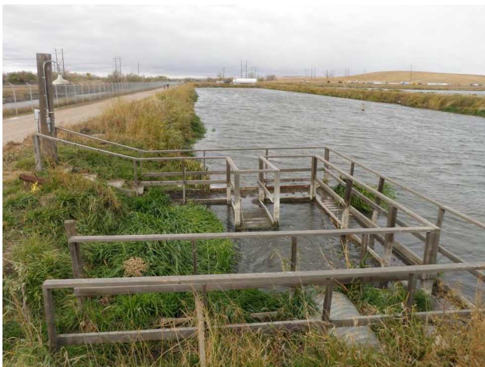
Photo 49: 1A / 1B Clear Pond south embankment dam upstream side looking northwest (1A Clear Pond drop-inlet pipe in foreground, Recirculation canal on left).
