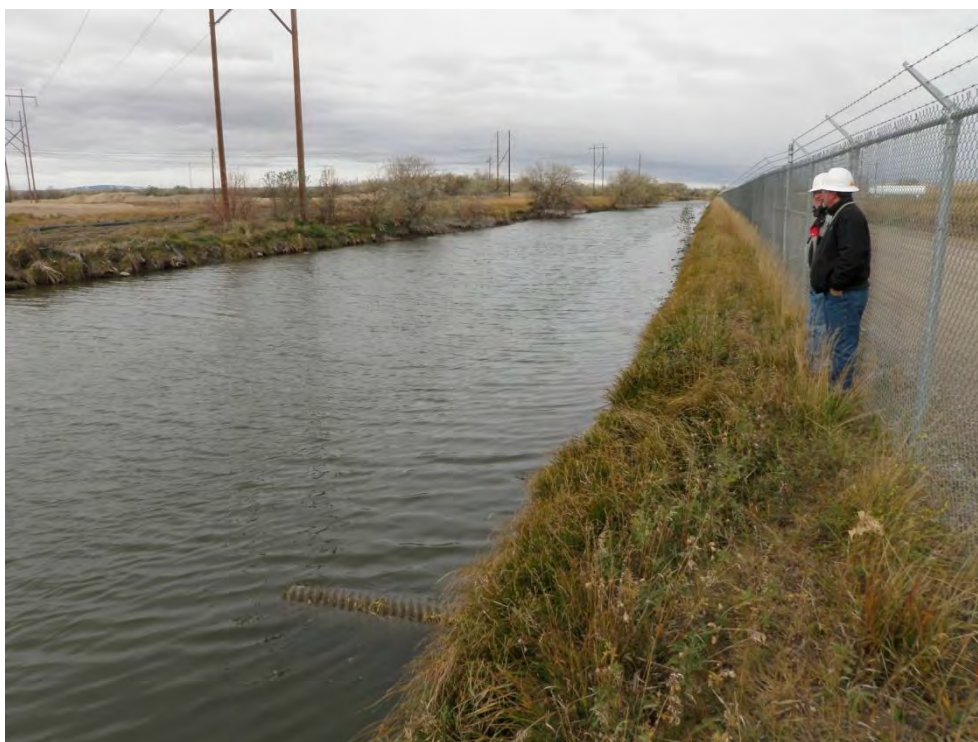
Photo 51: 1A / 1B Clear Pond south embankment dam downstream side looking northwest showing steep downstream slopes and Recirculation Canal. Inactive 008 Outfall in foreground left.
