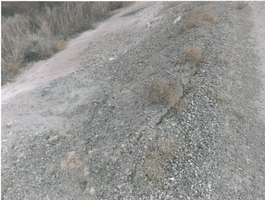
Photo 14: Pond F. Typical cracking and vegetation located along edge of crest and slope.
