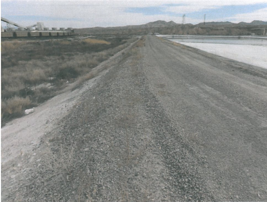
Photo 13: Looking southeast. North dike of Pond F. Typical soil cement slope protection. Muddy River located at left.
