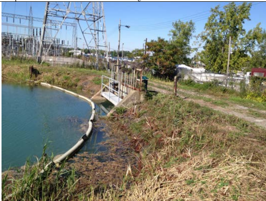
Photo 2: Caption- Pipe Outfall Retaining Wall and Embankment north side Pond 2
