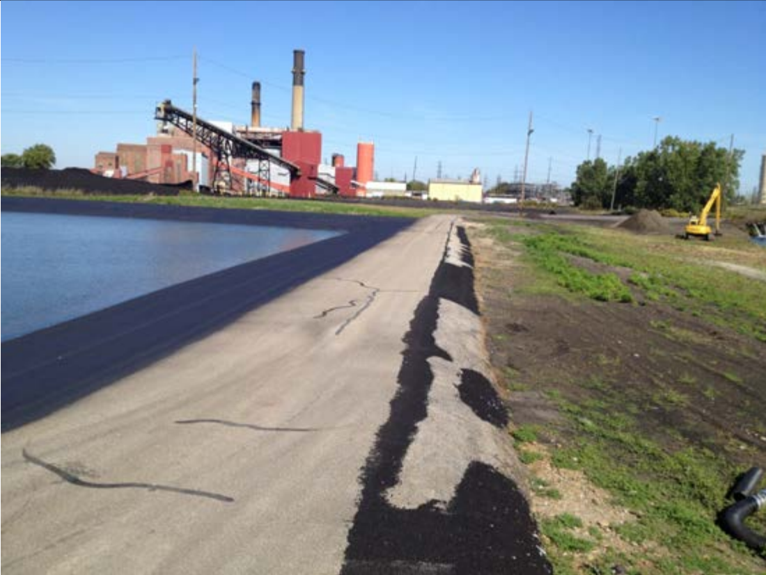
Photo 1: Caption- East Embankment North Equalization Basin. Note asphalt repair outer slope of embankment; sealant applied on basin interior and later applied on berm top and outside slope (see picture below).
