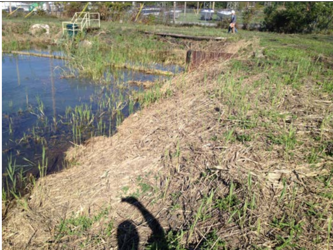
Photo 6: Caption- Incised East side of Pond 3 foreground, North embankment and outlet pipe background
