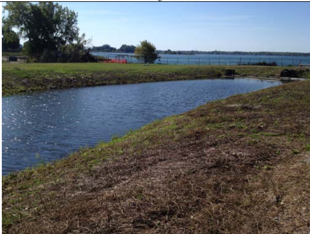
Photo 6: Caption- Incised Embankments West Outfall End of South Ash Settling Basin
