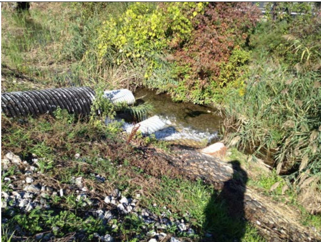
Photo 1: Caption- Pipe Outfall from Pond 2 into North side drainage ditch
