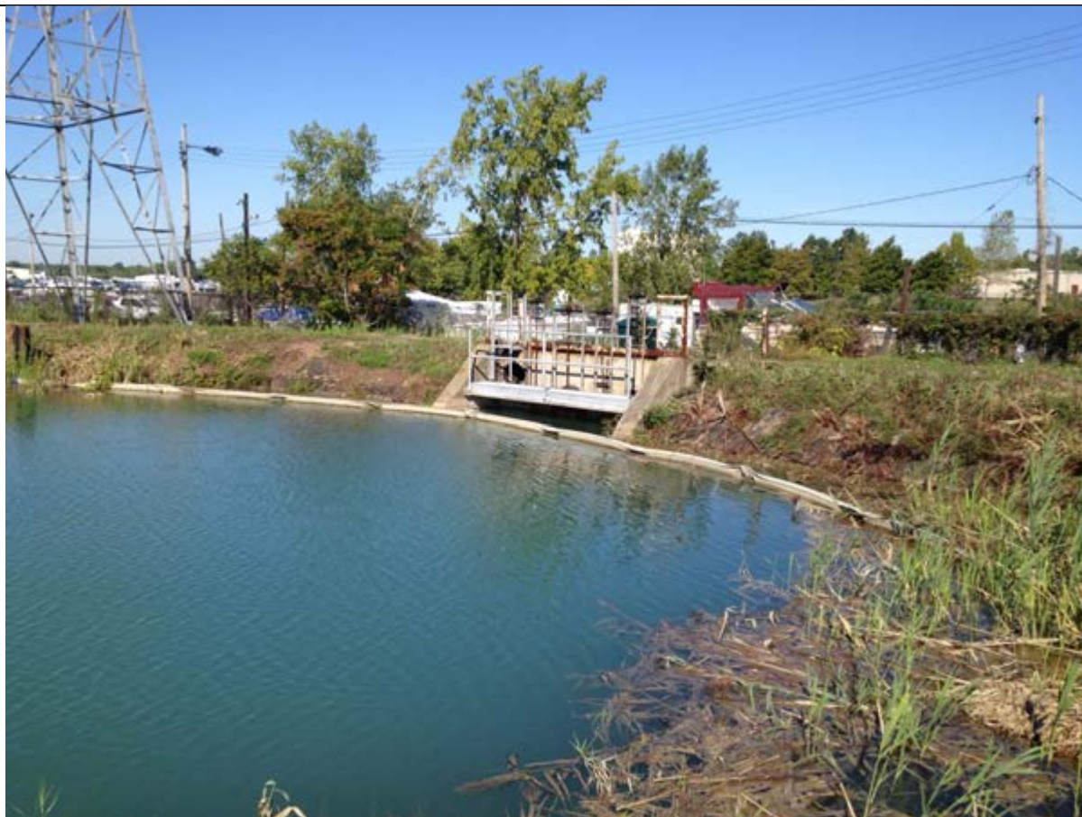
Photo 3: Caption- Pipe Outfall Retaining Wall and Embankment north side Pond 2
