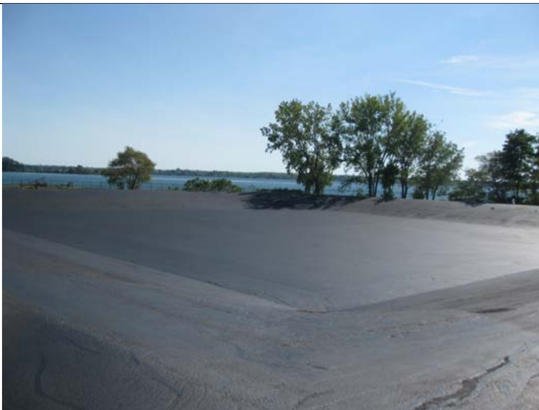
Photo 4: Caption- South Equalization Basin, newly applied asphalt sealant in basin bottom, berm tops and outside slopes.
