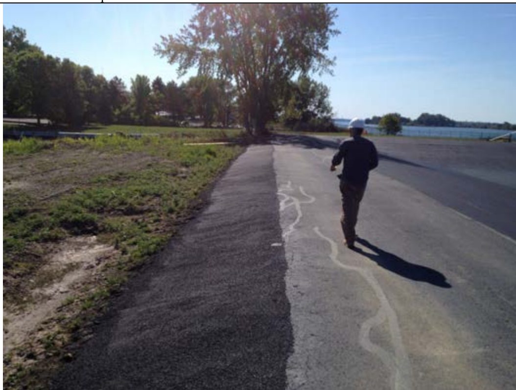
Photo 3: Caption- East Outside Embankment of South Equalization Basin. Note asphalt repair outer slope of embankment; application of sealant on basin interior in progress at time of photo and later applied on berm top and outside slope (see picture below).
