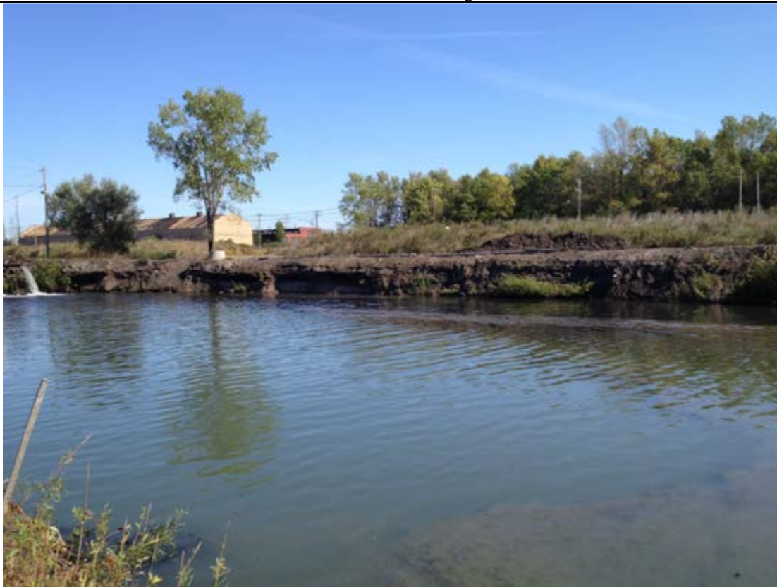
Photo 2: Caption- East Incised Embankment of South Ash Settling Basin
