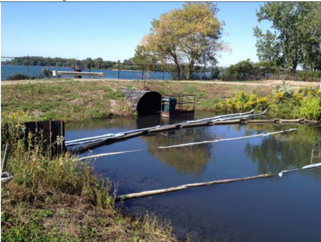
Photo 7: Caption- Outfall Pipe from South Ash Settling Basin to Niagara River
