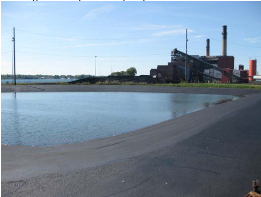
Photo 2: Caption- North Equalization Basin. Newly applied sealant in basin bottom, berm tops and outside slopes.
