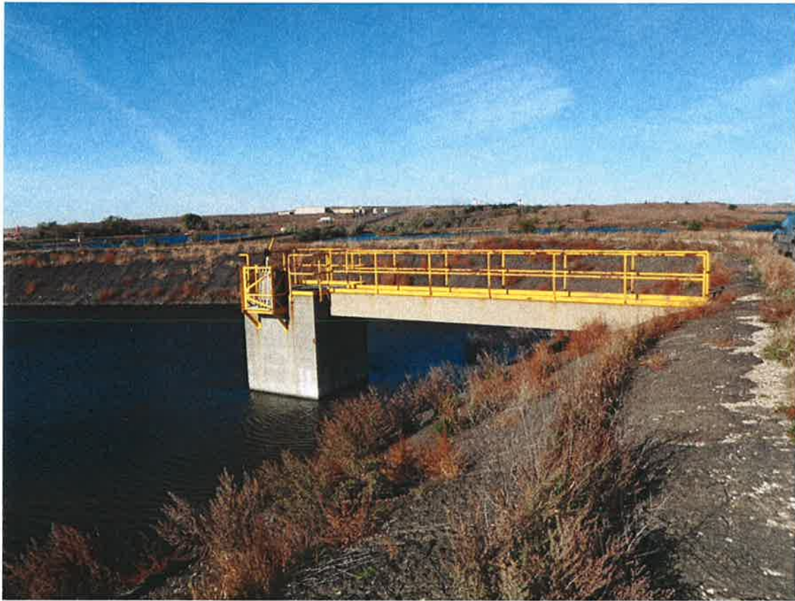
Photo 3: Alternate Bottom Ash Pond – Stop log structure on north dike, looking west
