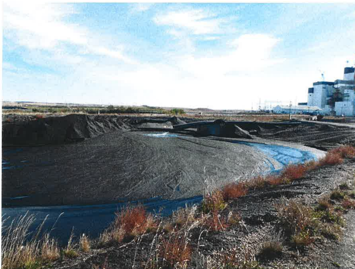
Photo 11: Alternate Bottom Ash Pond – East dike upstream slope and temporary inlet pipes, looking northeast
