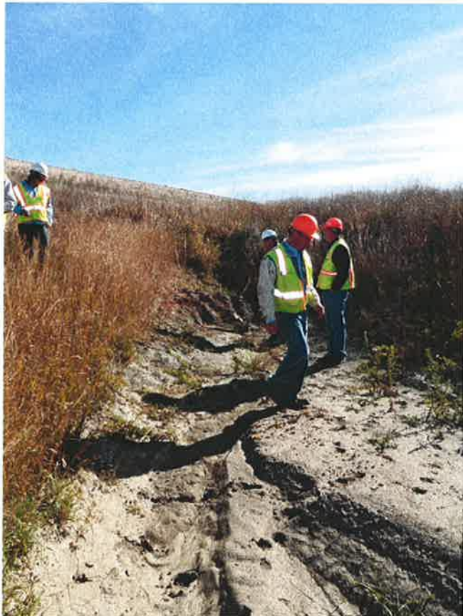
Photo 30: Cell 1 – Erosion channel near west dike downstream toe, looking south
