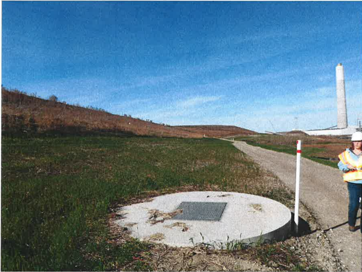
Photo 31: Cell 1 – East dike downstream slope and manhole for outlet pipes from Cell 2 returning to plant, looking north
