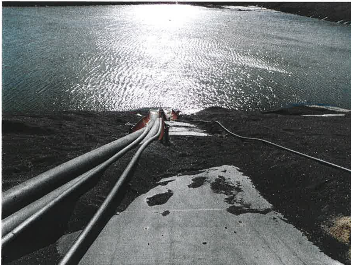
Photo 20: Cell 2 – North dike upstream slope, looking south, inlet pipes from Unit 1 and leachate collection from Butterfly Pond and Cell 1
