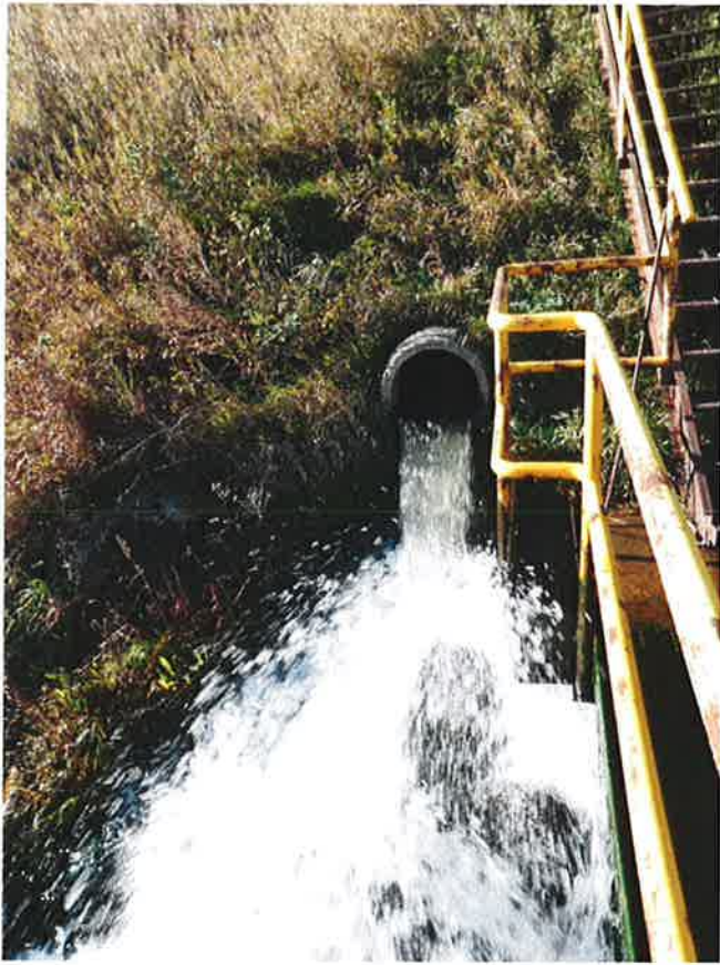
Photo 5: Alternate Bottom Ash Pond – 18" diameter RCP discharge to cooling canal, looking south
