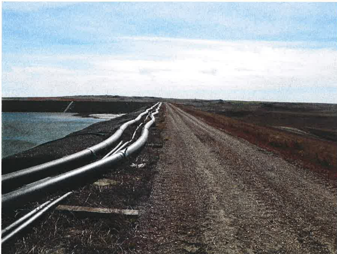
Photo 24: Cell 2 – West dike crest, looking south, inlet pipes from Unit 2
