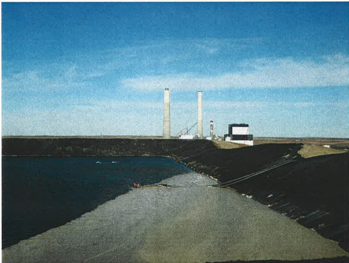
Photo 26: Cell 2 – East dike upstream slope, looking north, note siphon outlet pipes
