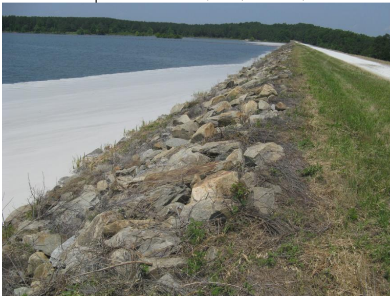
Photo 1: Upstream Embankment, Crest, Photo: 042, 6/3/09
