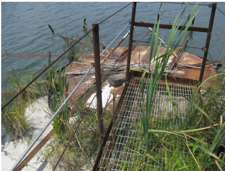
Photo 9: riser and skimmer at stilling pool, Photo: 079, 6/3/09
