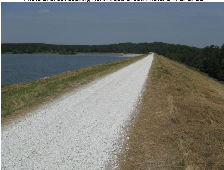
Photo 2: Crest Looking Northwest, Crest, Photo: 041, 6/3/09
