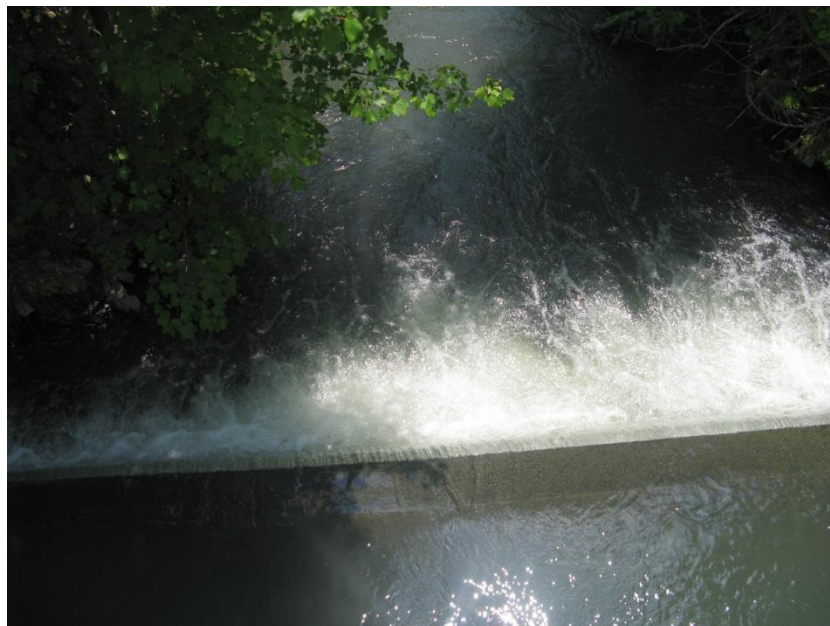
Photo 11 concrete overflow weir spillway, Photo: 068, 6/3/09
