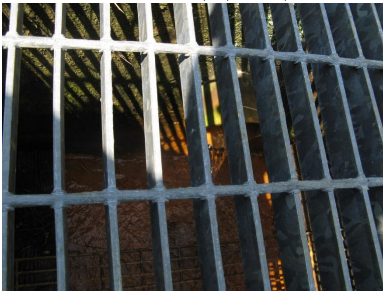
Photo 7: Internal Drain Outlet, Toe, Photo: 019, 6/3/09
