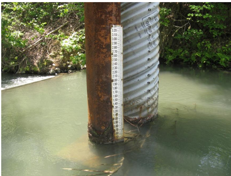
Photo 10: stilling pool staff gauge near spillway, Photo: 072, 6/3/09
