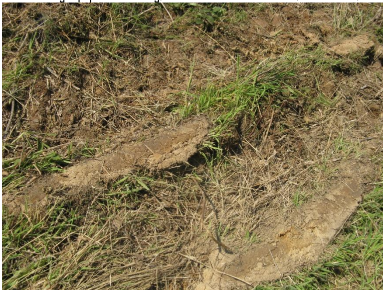
Photo 4: Mowing Equipment Rutting, Downstream Embankment, Photo: 007, 6/3/09
