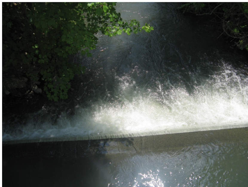
Photo 11 concrete overflow weir spillway, Photo: 068, 6/3/09
