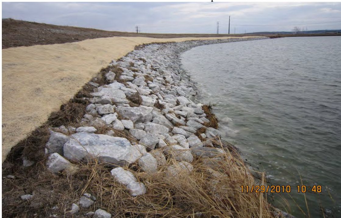
Photo 5 - Close up view of rip-rap protection North side of South Surface Impoundment
