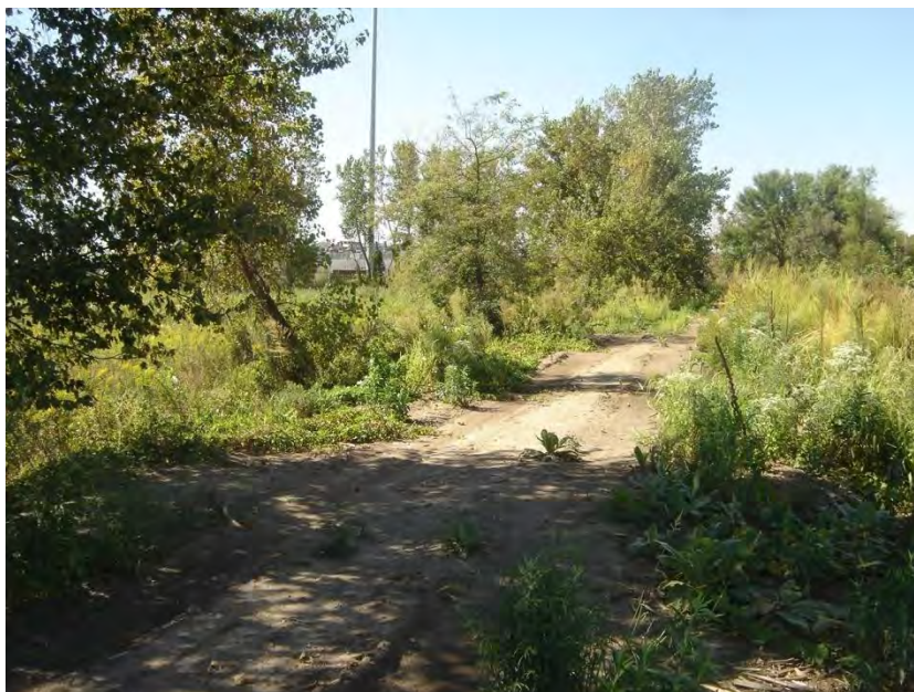
Figure 5.2.1: Crest and Slope of North Ash Pond dike.
