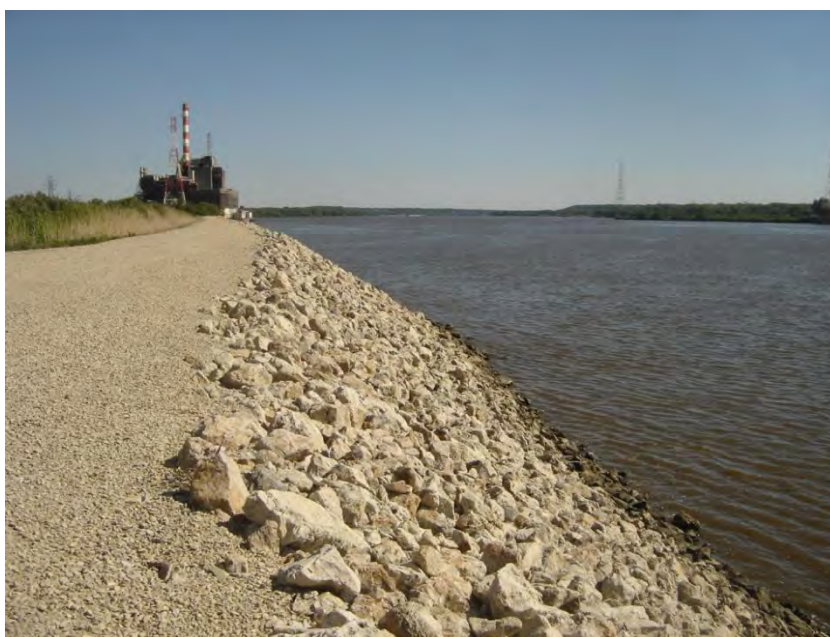
Figure 5.3.3: Downstream/Outside Slope of South Ash Pond dike.
