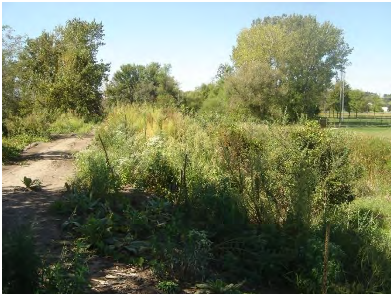
Figure 5.2.3a: Crest and Downstream/Outside Slope of North Ash Pond dike.
