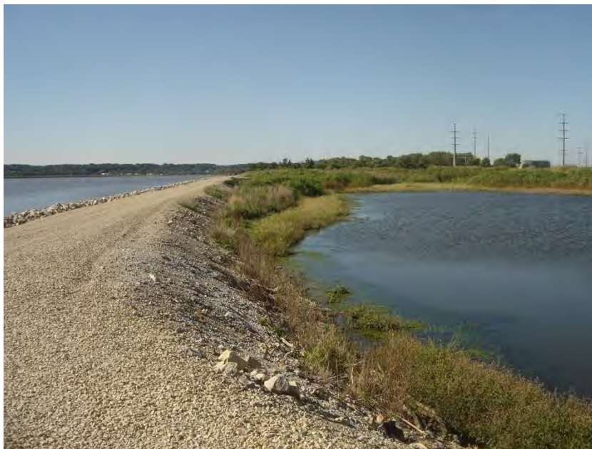
Figure 5.3.2: Upstream/Inside Slope of South Ash Pond dike.
