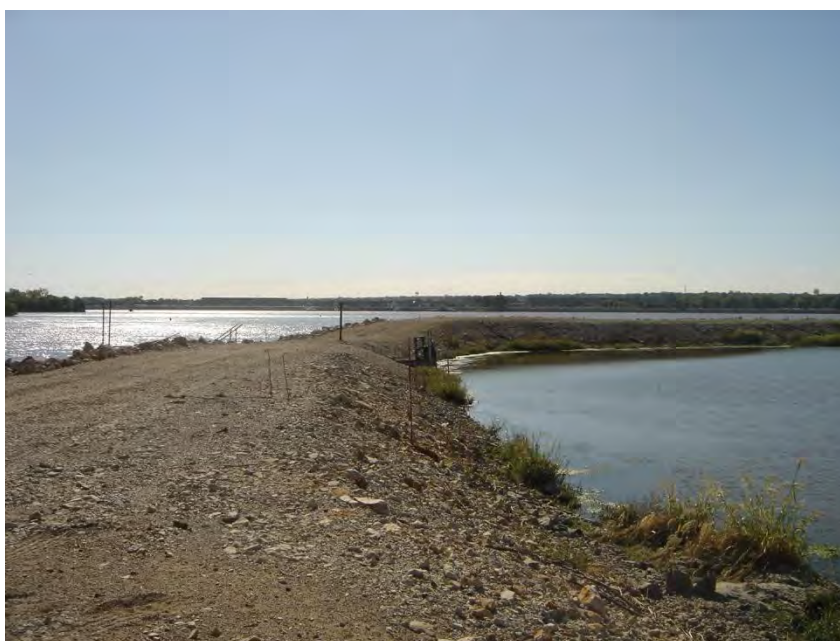
Figure 5.3.1: Crest and Upstream/Inside Slope of South Ash Pond dike.
