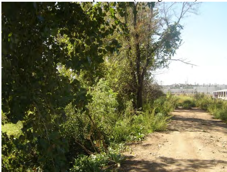
Figure 5.2.2: Crest and Upstream/Inside Slope of North Ash Pond dike.
